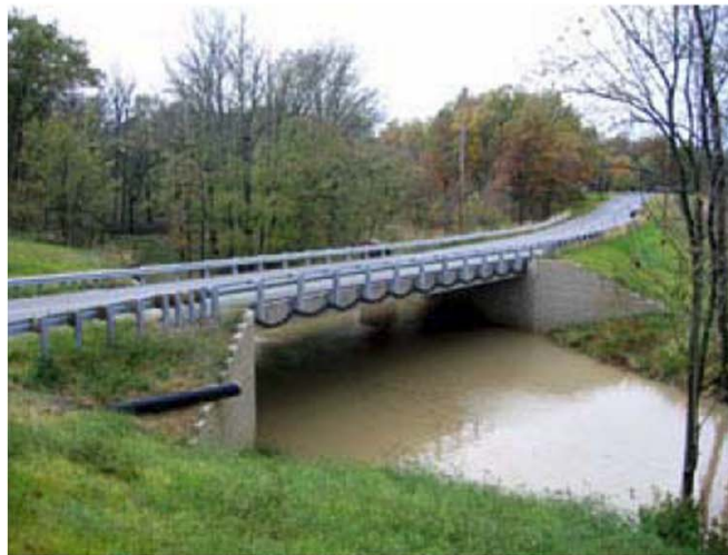
Bowman Bridge, Defiance County, Ohio
