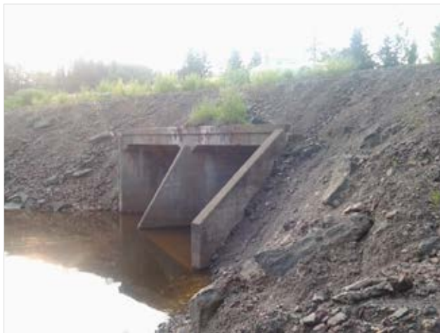
Figure 16: Photo of Culvert 5648, Downstream Side
