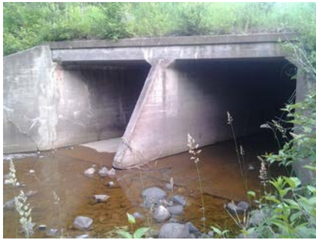
Figure 15: Photo of Culvert 5648, Upstream Side
