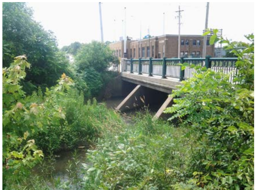
Figure 31: Photo of Culvert 5722, Downstream Side
