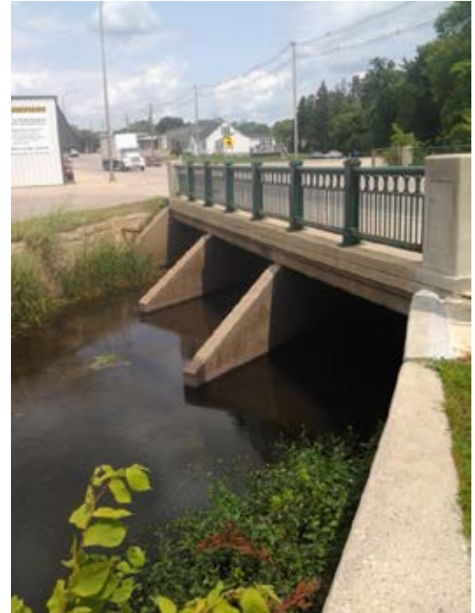
Figure 30: Photo of Culvert 5722, Upstream Side
