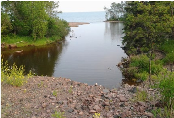
Figure 3: A view downstream from Culvert 5648
