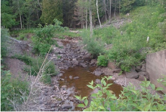
Figure 2: A view upstream from Culvert 5648
