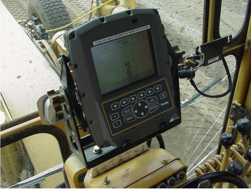
Operator's display for GPS inside of the Cab of a Grader.
