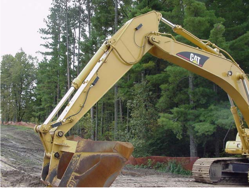
GPS on a Backhoe. Note the wiring to the bucket.
