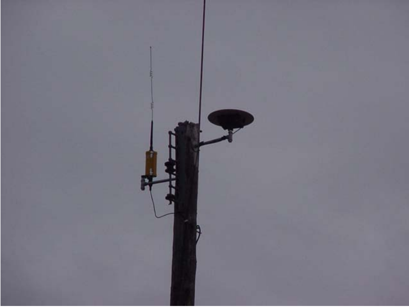
Close up of Contractors GPS Base.
