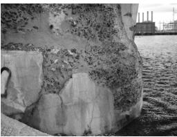
Figure 8. Looking east at the northernmost river pier. Shotcrete repairs to the pier have failed. Large spalled regions, with water draining out of the deteriorated area, were visible during the site visit.
