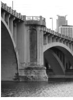
Figure 7. Staining and concrete spalls are visible on the north face of the west end of the pier between the barrel and rib arches.
