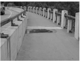
Figure 3. Looking north at the north end of the east sidewalk. Localized ponding adjacent to a reconstructed sidewalk expansion joint is visible. Staining on the vehicle barrier from the metal railing components and anchorages is typical.
