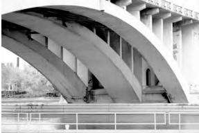
Feature 1. Melan-system reinforced-concrete arches. The Melan system, patented in 1894, uses steel Ibeams bent approximately to the shape of the arch axis and laid in a parallel series near the undersurface of the arch. The Third Avenue Bridge has seven large Melan arches, including two barrel arches and five three-rib arches, including the example in this photograph. It is considered to be the last major reinforced-concrete bridge constructed in the Twin Cities using the Melan system.
