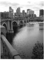
Figure 2. Looking south along the west side of the bridge from the west sidewalk. Stained, deteriorated concrete on the pier below the overlook is visible.
