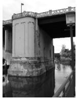
Figure 5. Looking east at the southernmost river pier. Deteriorated concrete is visible in many locations, primarily near the water line. The weathering steel beams supporting the south approach spans are also visible.
