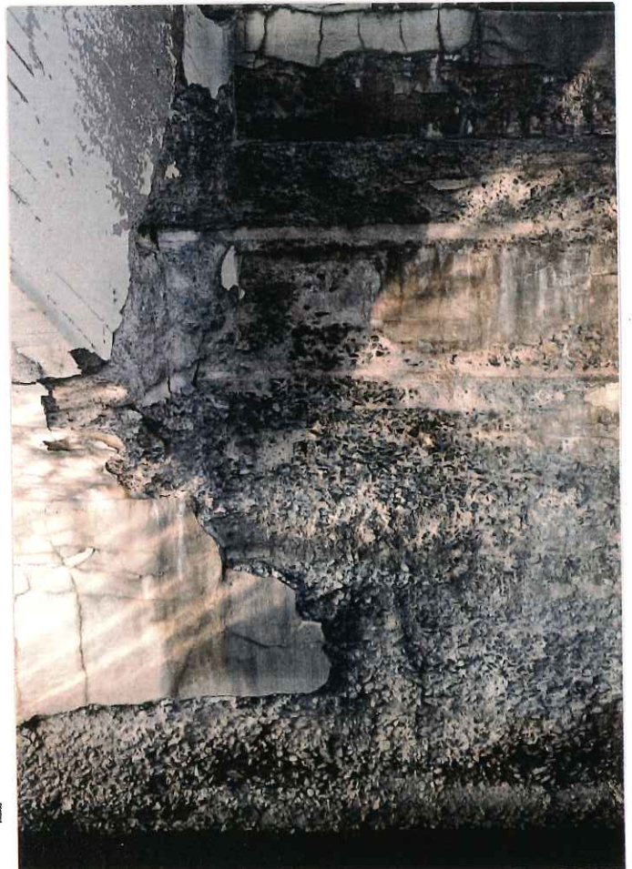
Pier 1 - Between Center and North Arches (Scaling)
