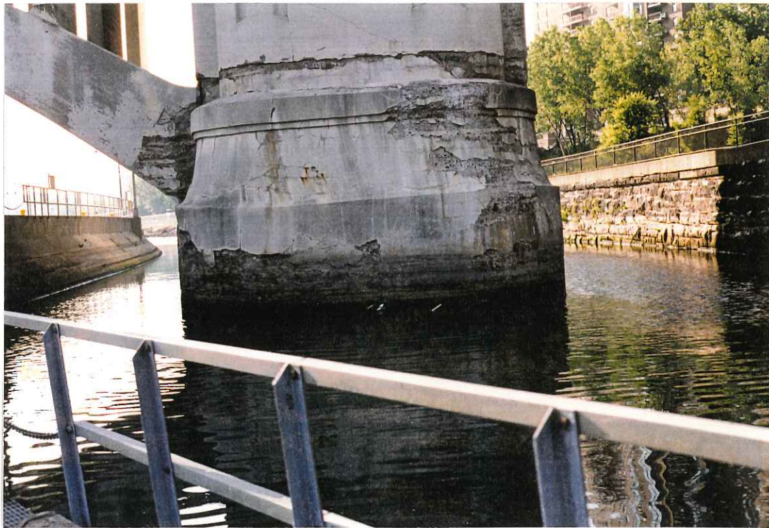
Pier 1 - Upstream Nose (Scaling)
