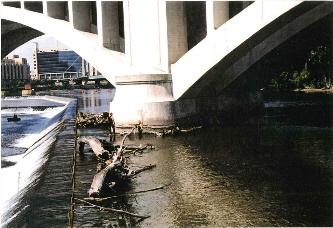
Pier 5 - Downstream End (Debris and Scaling)
