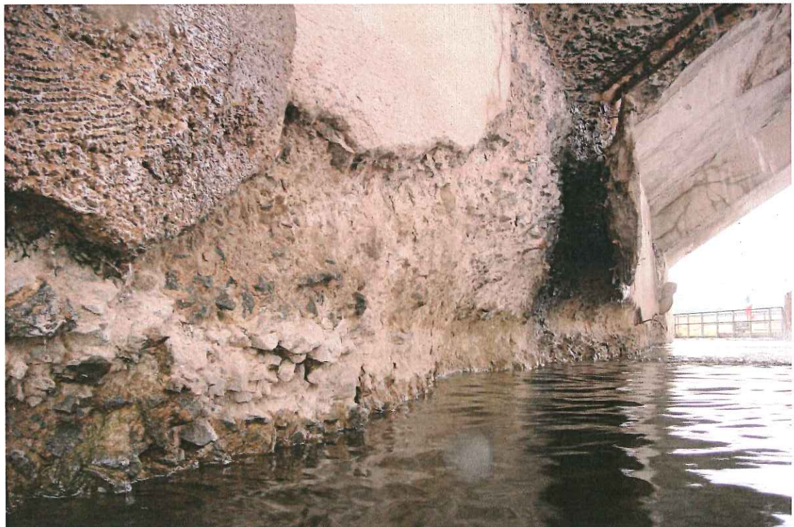
Photograph 10. View of typical concrete deterioration on the East face of Pier 1, Looking Northwest.
