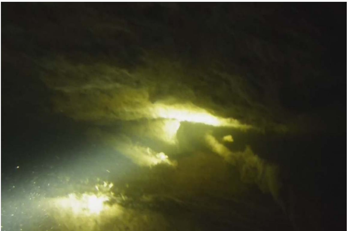
Photograph 10. View of Undermined (Undercutting) cavity at Pier 5, Looking South.
