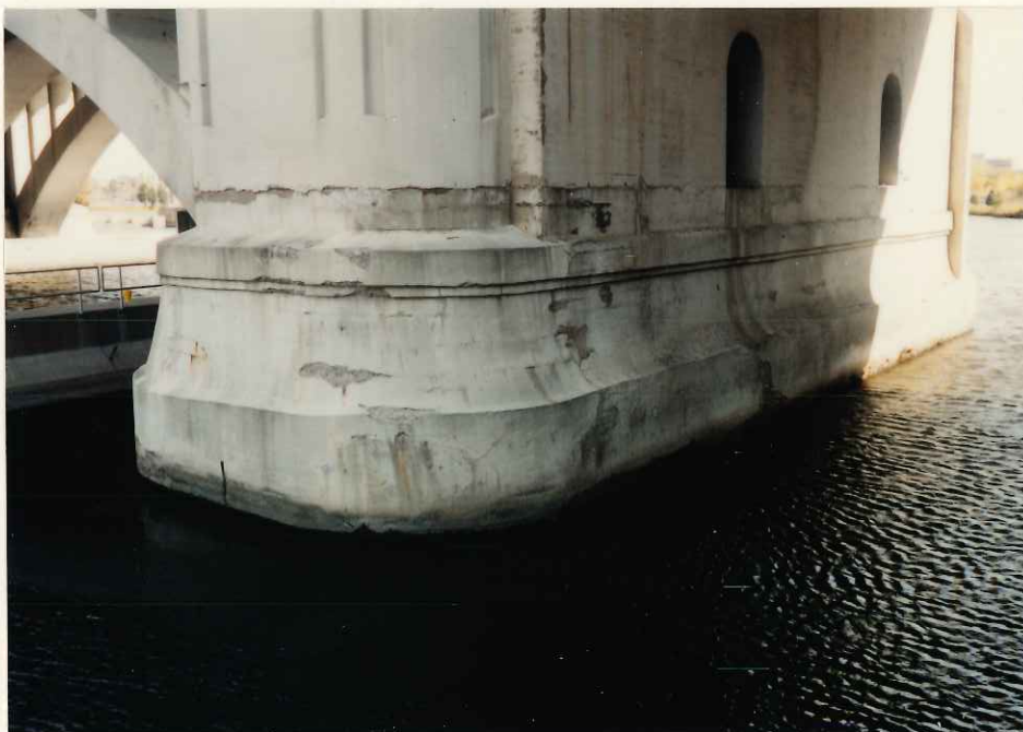
Photograph 1. Bridge No. 2440, 10/11/91. View of Pier 1 Looking Northeast.
