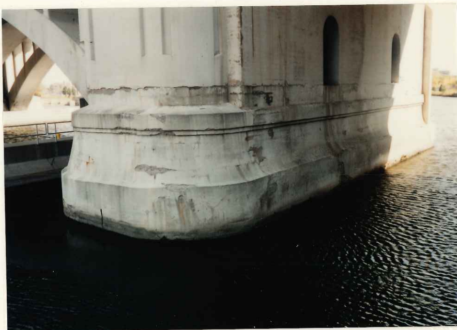
Photograph 1. Bridge No. 2440, 10/11/91. View of Pier 1 Looking Northeast.
