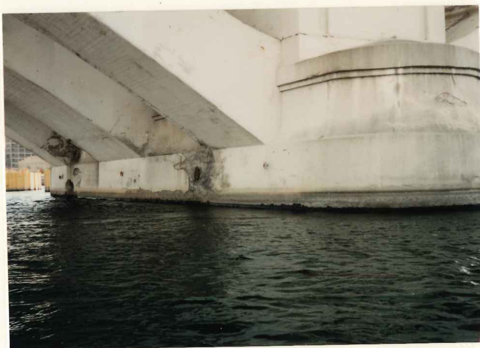
Photograph 2. Bridge No. 2440, 10/11/91. View of Pier 2 Looking East.
