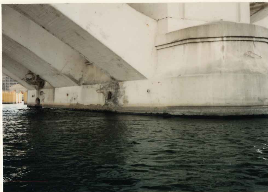
Photograph 2. Bridge No. 2440, 10/11/91. View of Pier 2 Looking East.
