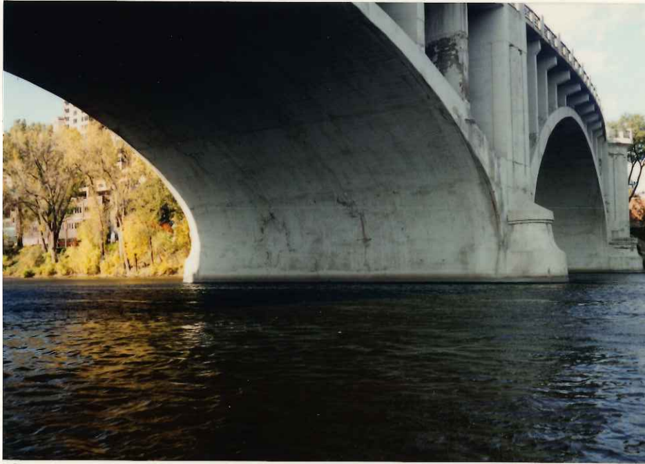
Photograph 5. Bridge No. 2440, 10/11/91. View of Pier 7 Looking North.
