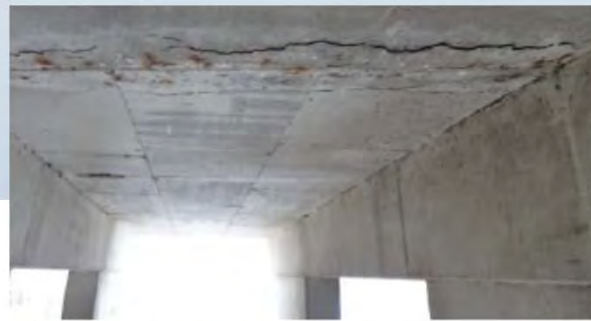
Figure 4.14. Slab underside delamination at manhole.
