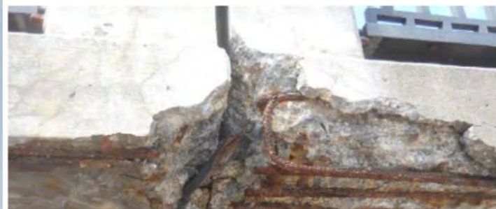
Figure 4.17. Slab underside spalls and rebar section loss at manholes in southbound lane.
