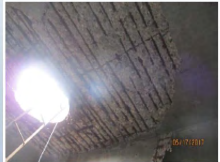
Figure 4.17. Slab underside spalls and rebar section loss at manholes in southbound lane.
