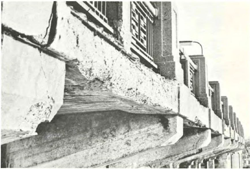
II-14. Areas of spall at the bridge railing posts, sidewalk deck, and spandrel cantilevers.
