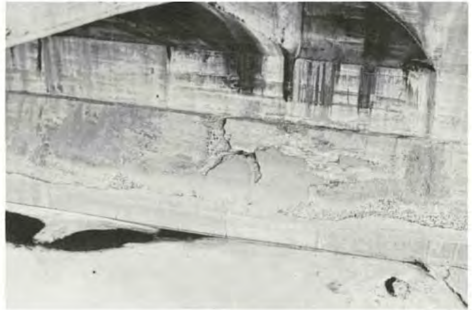
II-29. Deterioration to the south wall of Pier 4.
