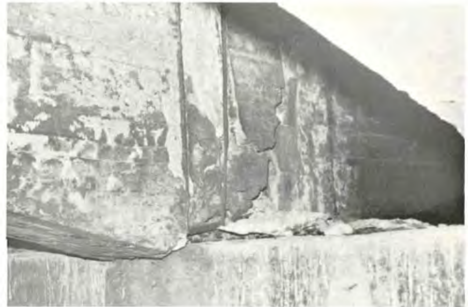
II-19. Crushed concrete at a beam haunch above Bent 5.
