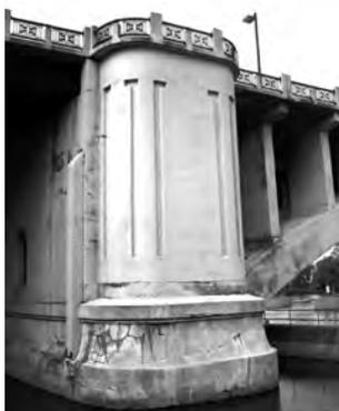
Feature 3. Classical Revival aesthetic treatment. A gateway structure, the Third Avenue Bridge received a Classical Revival aesthetic treatment. Classical elements include piers and the projecting pedestrian bays, which were restored or reconstructed in the 1979-80 deck-replacement project, and the 1939 ornamental railing.
