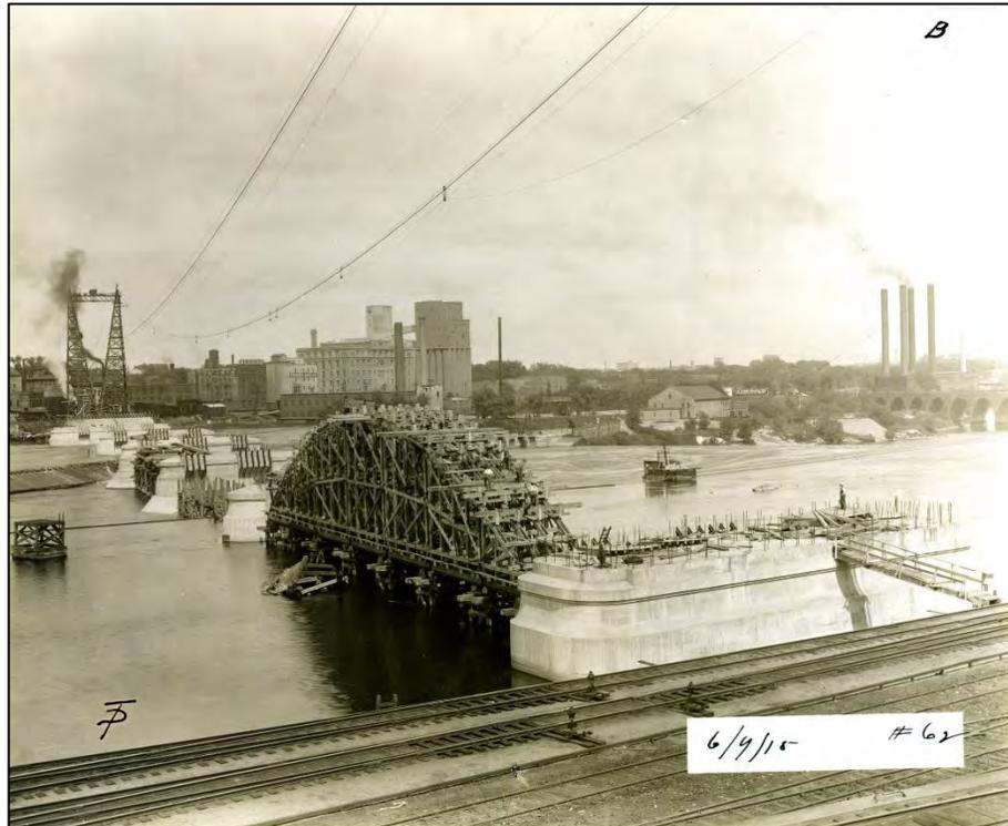
**Figure 11.** June 9, 1915 – Arch falsework, looking northeast
