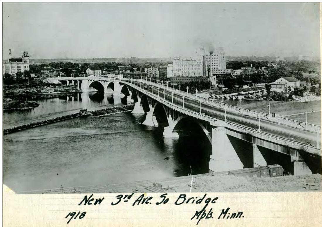
**Figure 17.** 1918 – Third Avenue Bridge with steel-girder west approach spans in foreground, looking northeast
