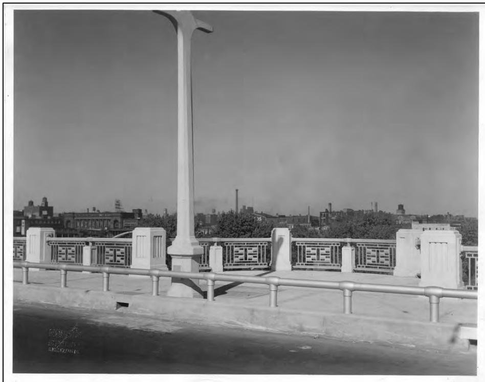
**Figure 24.** 1939 – New sidewalk, railing, and traffic barriers after renovation
