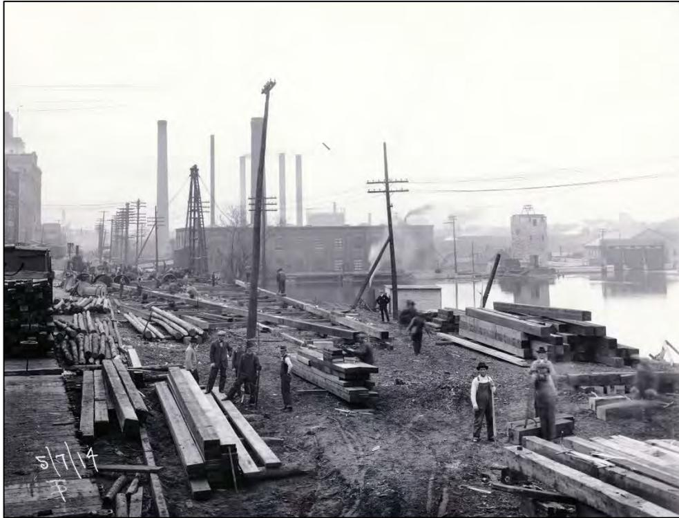
**Figure 4.** May 7, 1914 – Building the timber tower on the east bank, looking southeast
