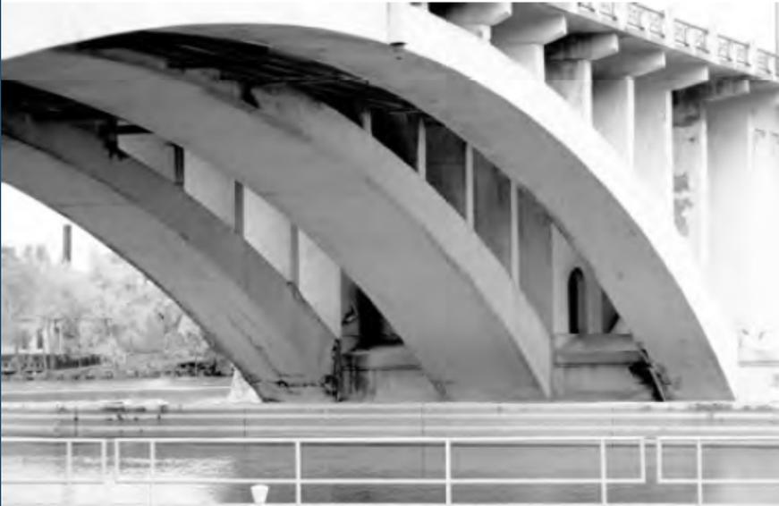
Feature 1. Melan-system reinforced-concrete arches. The Melan system, patented in 1894, uses steel I-beams bent approximately to the shape of the arch axis and laid in a parallel series near the undersurface of the arch. The Third Avenue Bridge has seven large Melan arches, including two barrel arches and five three-rib arches, including the example in this photograph. It is considered to be the last major reinforced-concrete bridge constructed in the Twin Cities using the Melan system.
