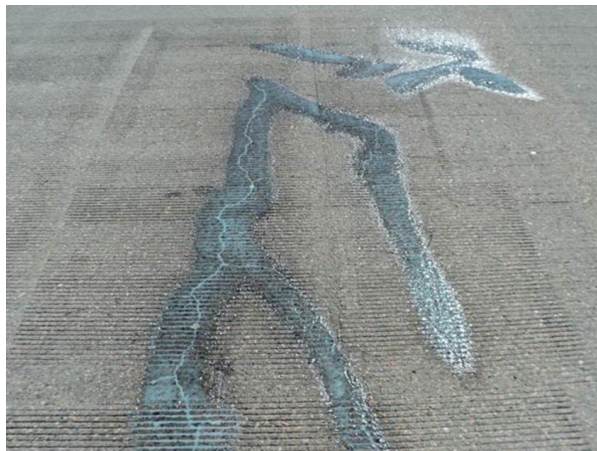
Figure 1: Prefilling cracks .040" and larger
