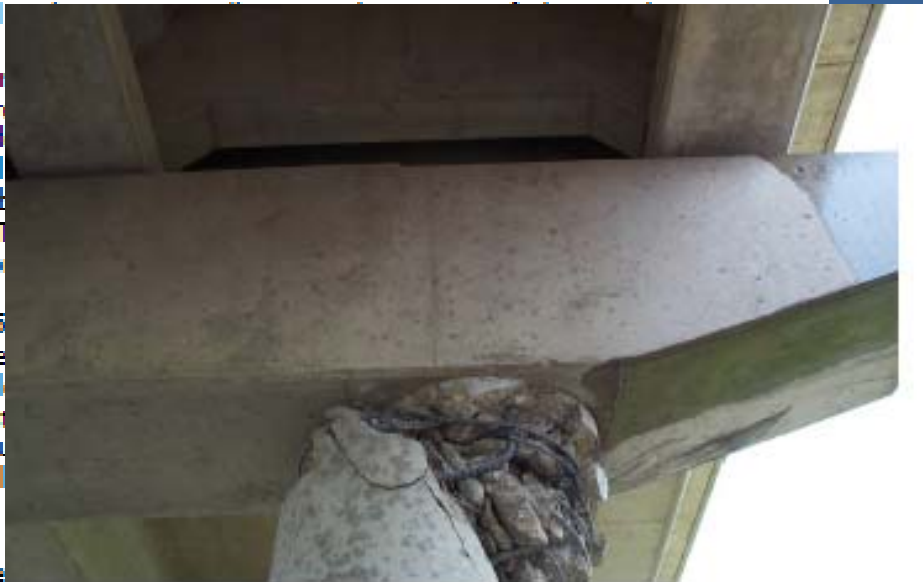
Figure 2.10. Truck Accident – IH-90 Bridge, #53812, Minnesota.
