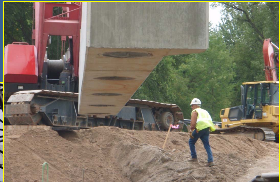
Photo courtesy of MnDOT
