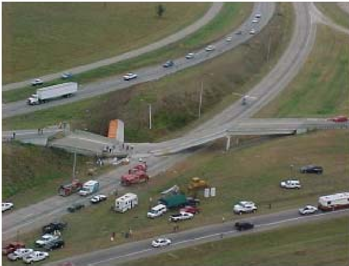
Figure 2.7. Truck Accident – SH 14 Bridge over IH-45, Corsicana, Texas.
