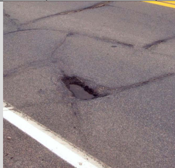
Condition State 4 Pothole (2" deep) in bituminous overlay
