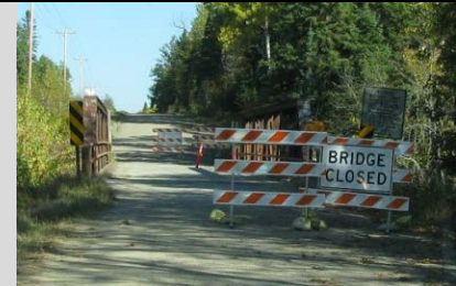
Condition State 4 Closed bridge not properly barricaded
