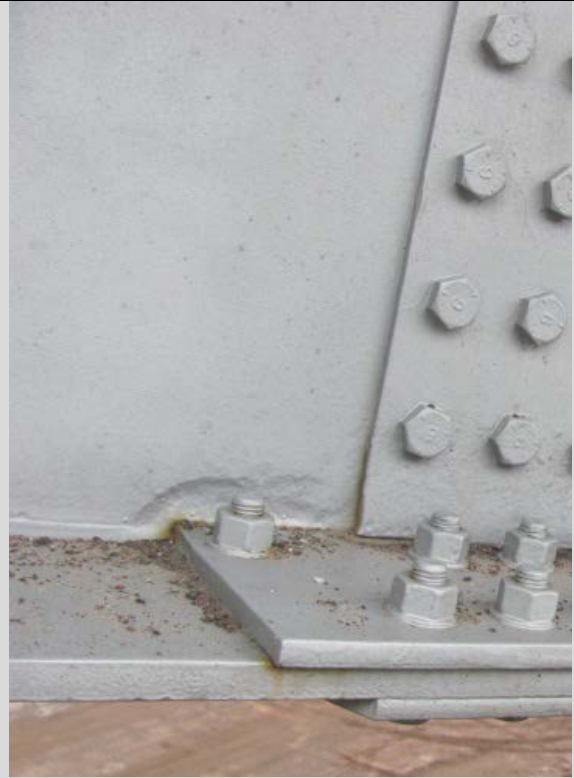
Condition State 3 Pitting in girder web at splice (painted over)
