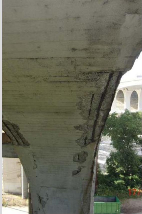
Condition State 3 Spalling on a reinforced concrete arch
