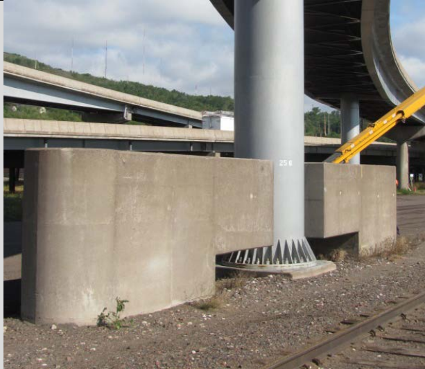
Condition State 1 Concrete wall protecting a steel pier column adjacent to a railroad track
