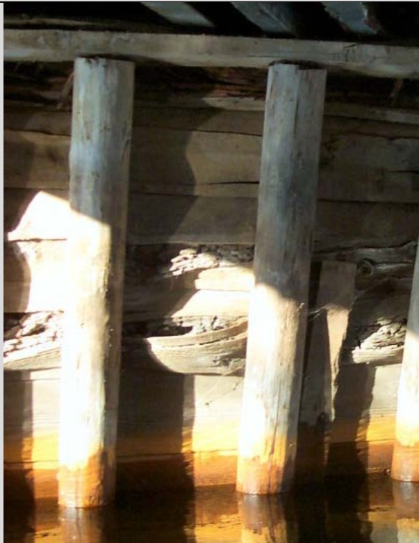
Condition State 4 Failure of abutment backing planks
