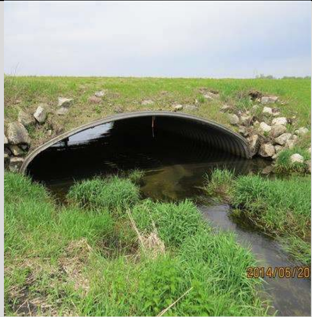
Condition State 1 Aluminum Box Culvert
