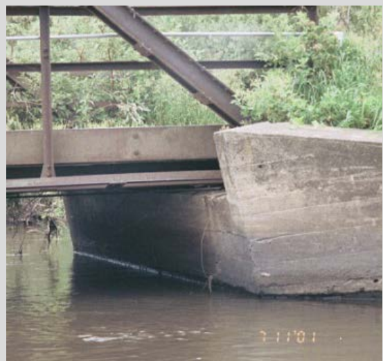
Condition State 4 Abutment severely tipped
