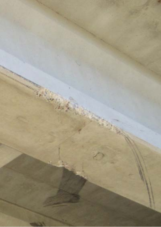
Condition State 2 Impact damage (minor spall) on a prestressed concrete beam
