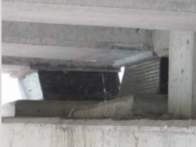
Condition State 2 Elastomeric pads tipped in opposite directions
