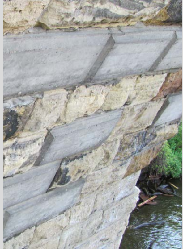
Condition State 2 Concrete repairs on a masonry arch
