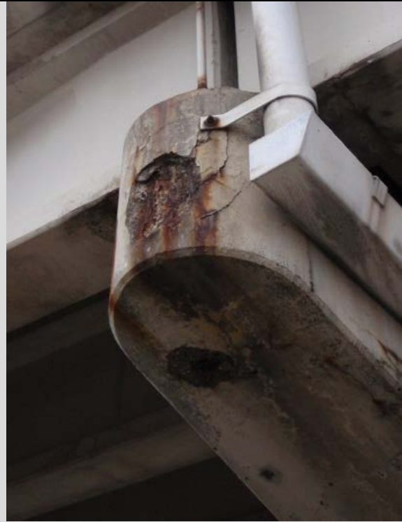
Condition State 3 Spalling on a reinforced concrete pier cap
