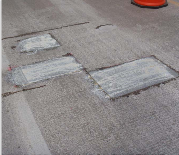
Condition State 2 Sound concrete patches on a low slump overlay
