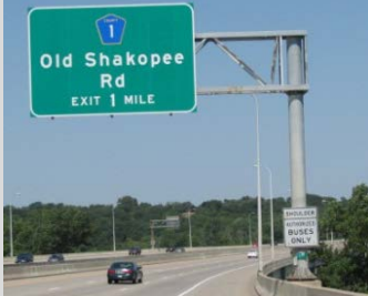
Overhead sign structure mounted on bridge railing
