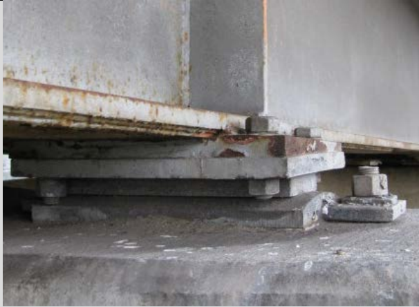
Condition State 2 Minor corrosion on a curved plate fixed bearing
