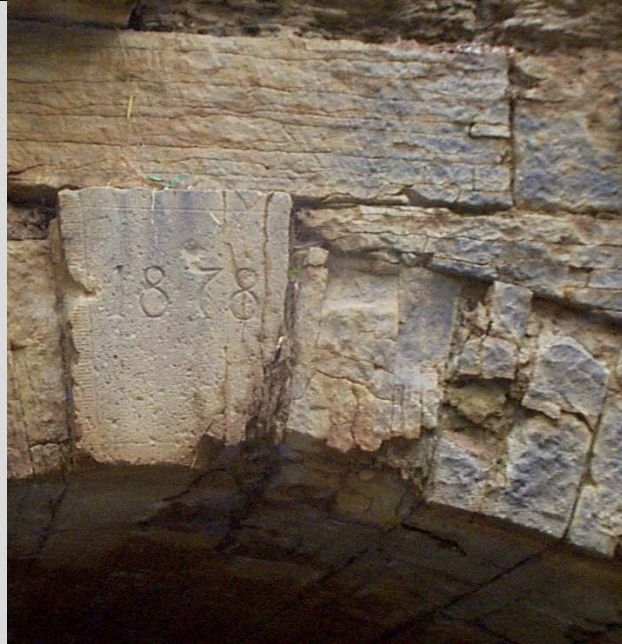
Condition State 2 Weathering of fascia blocks on a masonry arch culvert
