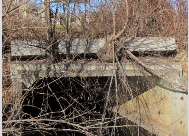
Condition State 3 Precast headwall separated due to tree growth
