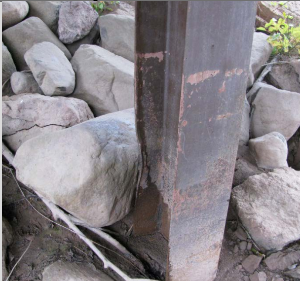
Condition State 3 Steel H-piling bent due to rock impact
