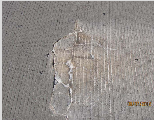
Condition State 3 Delamination on a low slump concrete overlay
