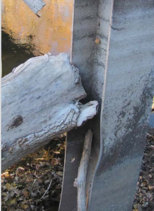
Condition State 2 Impact damage (bent flange) on a steel H-pile
