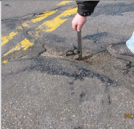
Condition State 3 Significant cracking on a bituminous overlay
