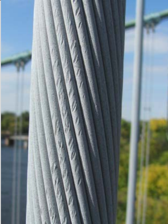
Condition State 2 Minor wear on steel strand hanger cable
