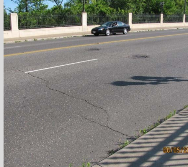
Condition State 1 Minor cracking in a bituminous roadway above a masonry arch culvert
