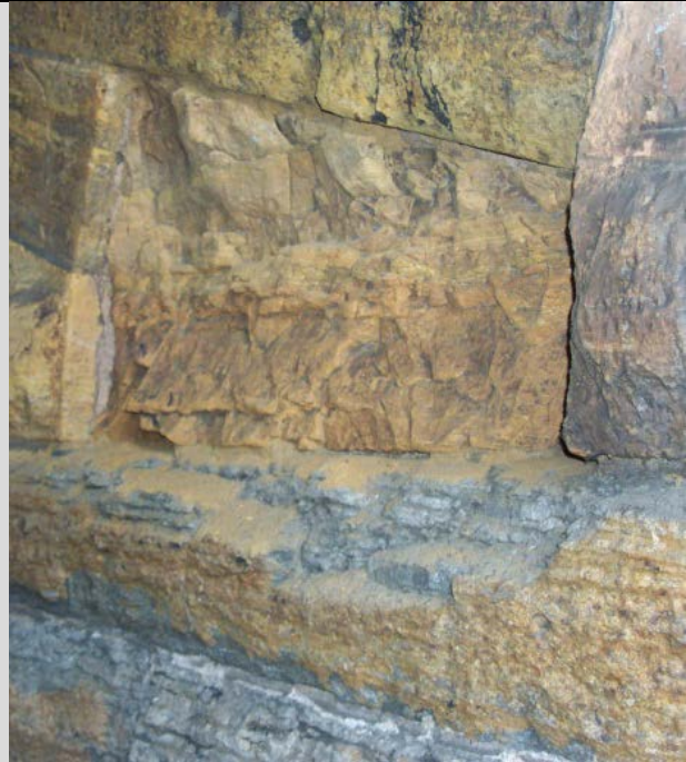
Condition State 3 Spalling on a masonry arch block (10% to 25% of block thickness)
