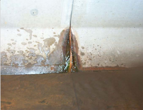
Condition State 2 Minor leakage between the segments of a precast box culvert
