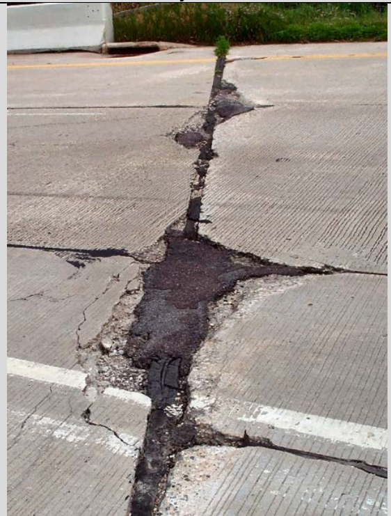
Condition State 4 Severe spalling (temporary patch) along approach relief joint
