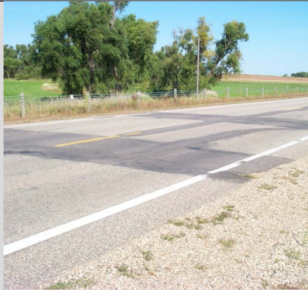
Condition State 2 Bituminous patches (due to settlement) along both sides of a concrete box culvert
