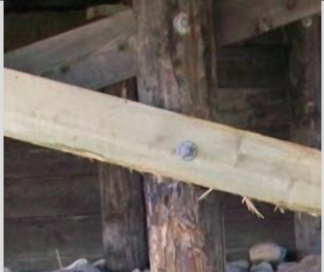
Condition State 2 Minor ice abrasion on a timber pier bracing plank
