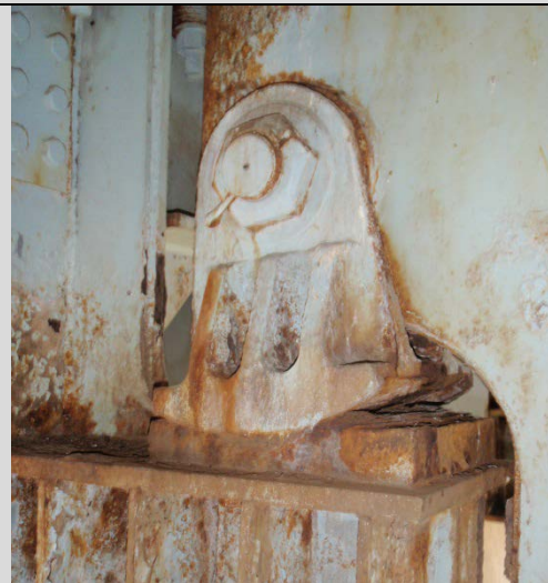
Condition State 3 Pack rust under a rocker expansion hinge
