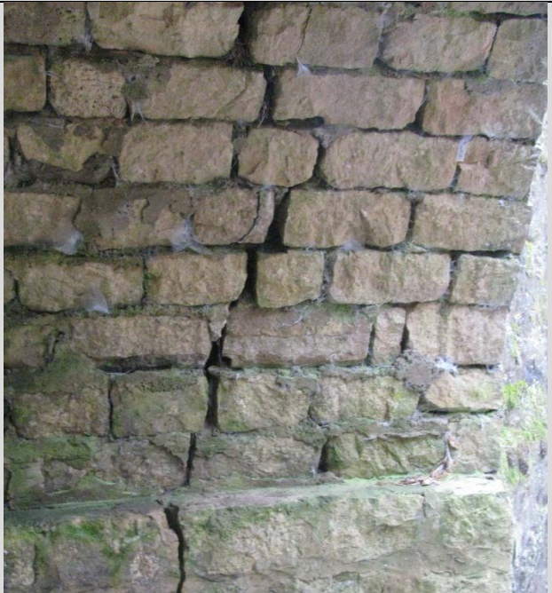
Condition State 4 Severe vertical fracture (with blocks misaligned and loose) on a masonry arch culvert
