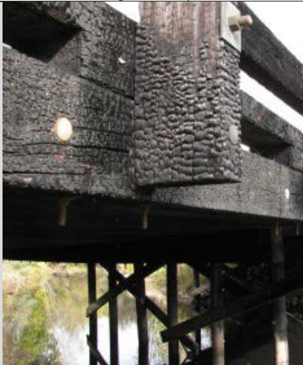
Condition State 3 Fire damage (significant charring) on a timber slab
