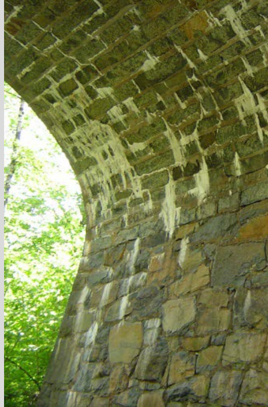
Condition State 3 Leaching through joints on a masonry arch
