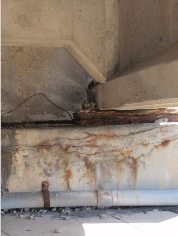
Condition State 3 Horizontal cracking with delamination and rust stains on the face of a reinforced concrete abutment
