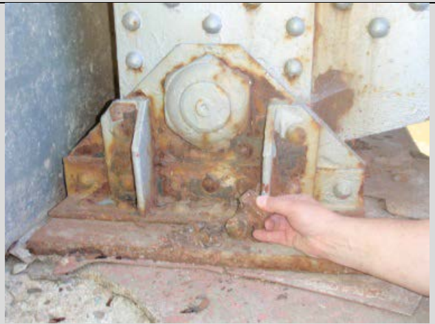
Condition State 4 Anchor bolt failure on a fixed pin bearing (masonry plate has slid back to the parapet)
