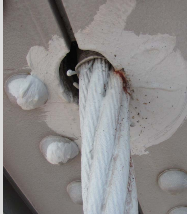
Condition State 3 Active abrasion at contact point (steel wire rope hanger cable wearing against a steel batten plate)
