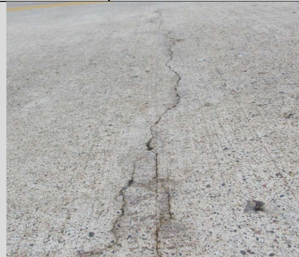
Condition State 3 Crack in a concrete wearing surface (width between 1/16" and 1/4")
