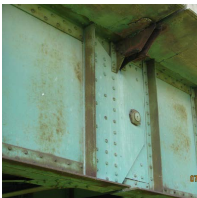
Fixed Pin Assembly on a Riveted Steel Girder Bridge
