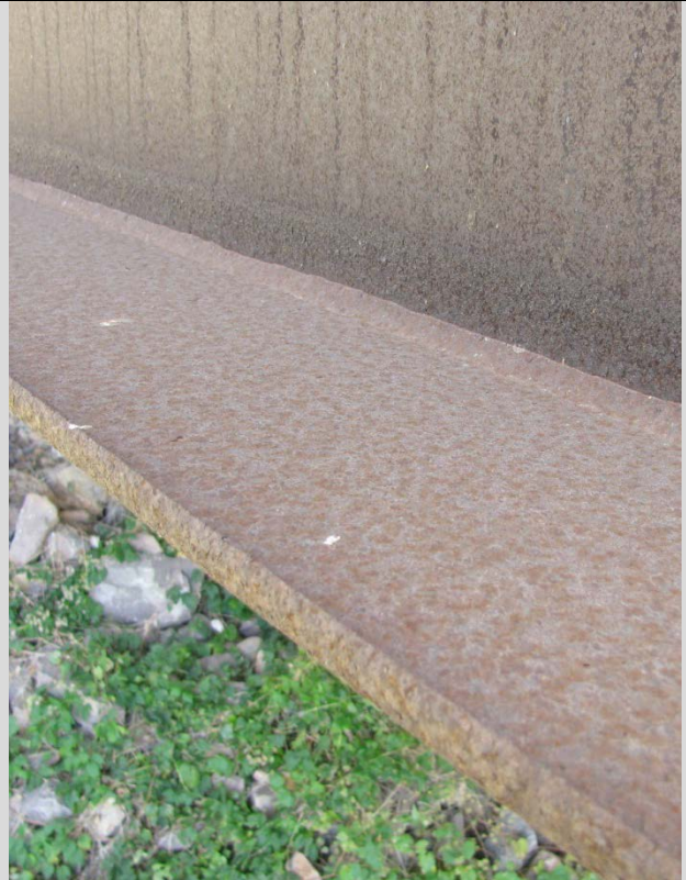
Condition State 2 Weathering steel patina is slightly uneven - surface is granular and dusty
