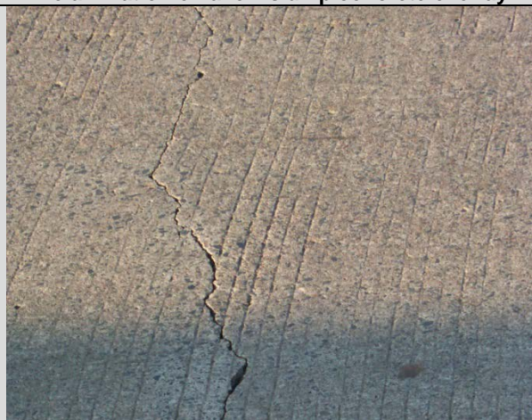
Condition State 3 Unsealed crack in a low slump overlay (1/8" wide)
