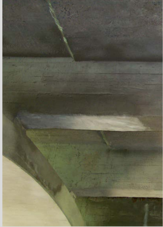
Condition State 2 Patching on a concrete arch spandrel cap
