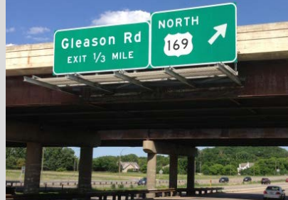
Signs mounted on bridge fascia
