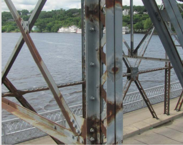
Condition State 2 Heat-straightened truss vertical member
