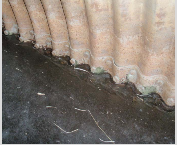
Condition State 2 Extensive surface corrosion
