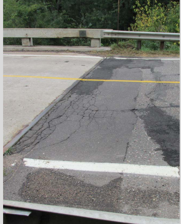
Condition State 3 Extensive deterioration on a bituminous approach roadway (settlement, cracking, and patching)
