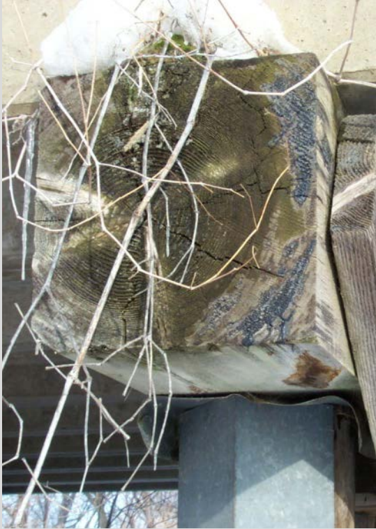
Condition State 2 Checking on the end of a timber pier cap
