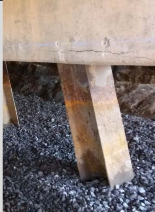
Condition State 3 Flaking rust on a steel H-Pile
