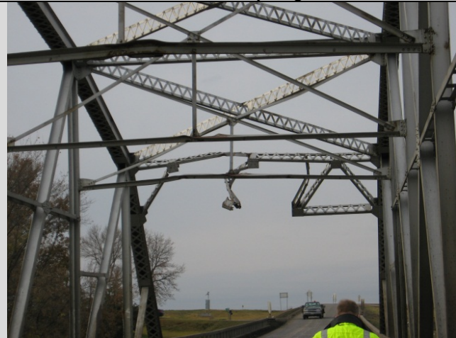
Condition State 4 Truss portal brace severely damaged
