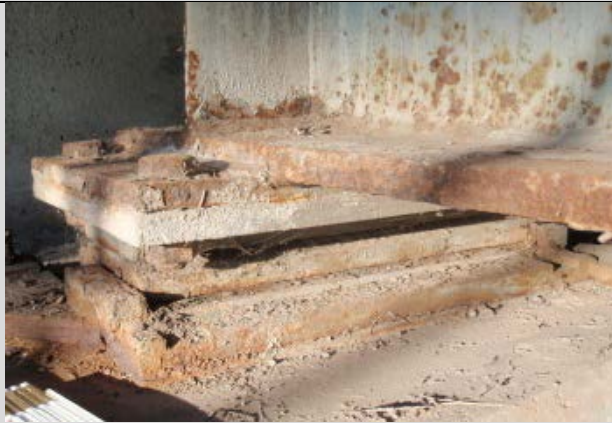
Condition State 2 Debris and surface corrosion on sliding plate bearing
