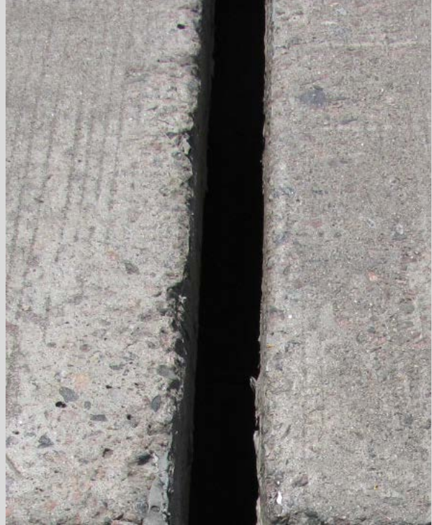
Condition State 3 Compression seal gland has dropped out of joint
