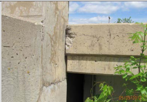
Deck corner contacting the abutment end post due to abutment movement
