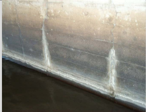
Condition State 2 Leaching cracks on a cast-in-place (CIP) concrete box culvert
