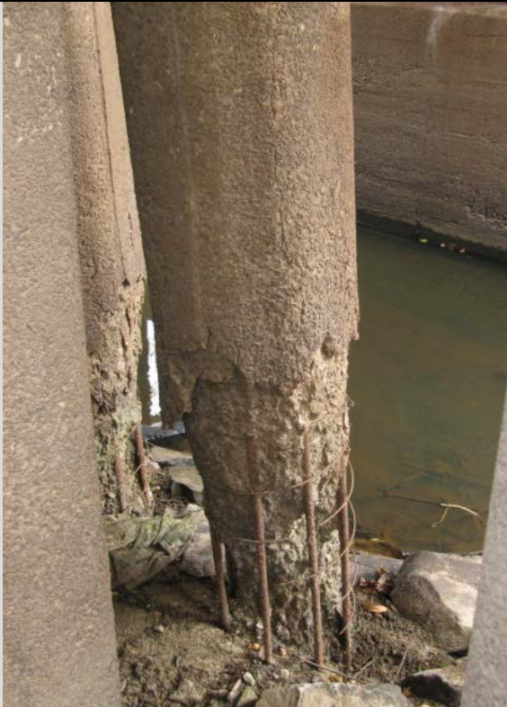
Condition State 4 Severe scale/spall on a reinforced concrete pile
