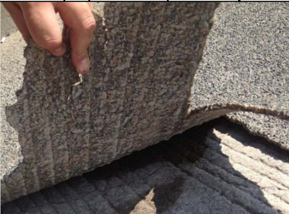
Condition State 4 Chip seal overlay peeling off (loose)
