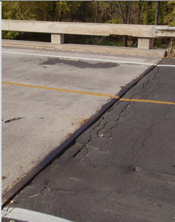
Condition State 3 Significant settlement on a bituminous approach roadway (along the bridge deck)
