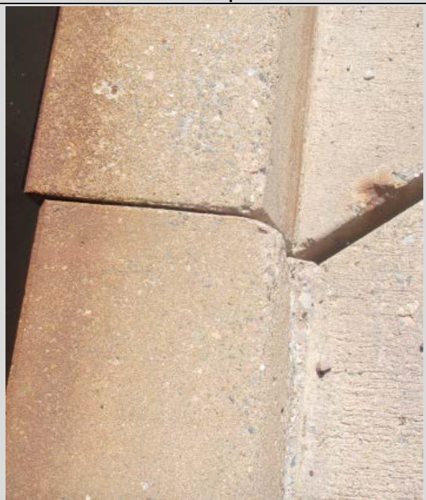
Condition State 4 Open joint contacting at curb (no further expansion is permitted) – deck is offset laterally
