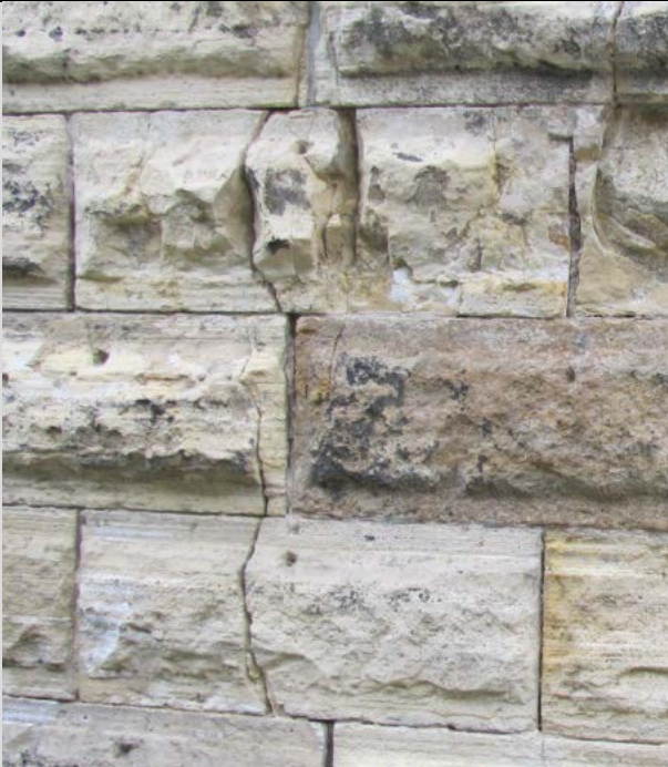
Condition State 3 Fracture in a masonry block continuing into adjacent courses
