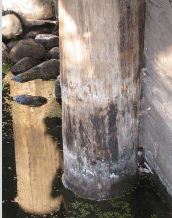
Condition State 2 Timber piling with decay at waterline (less than 10% section loss)
