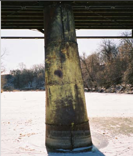
Condition State 4 Steel tube pier column severely tipped
