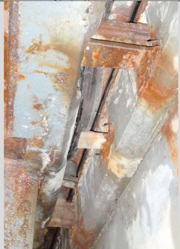
Condition State 4 Support missing from underside of modular joint - gland has fallen out and is hanging down
