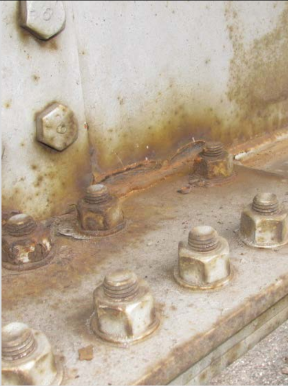
Condition State 3 Flaking rust (and pitting) in girder web at splice
