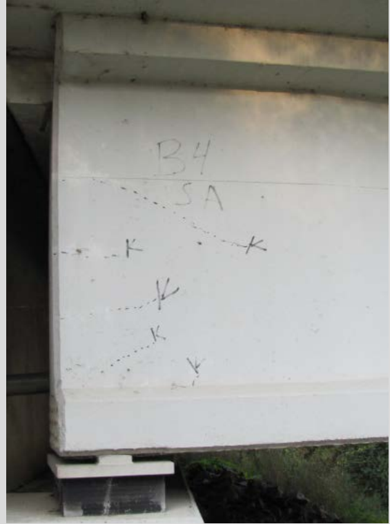
Condition State 2 Draped strand cracking in the end a prestressed concrete beam
