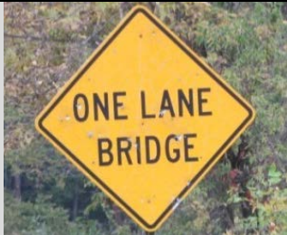
Condition State 2 One Lane Bridge sign with several bullet holes
