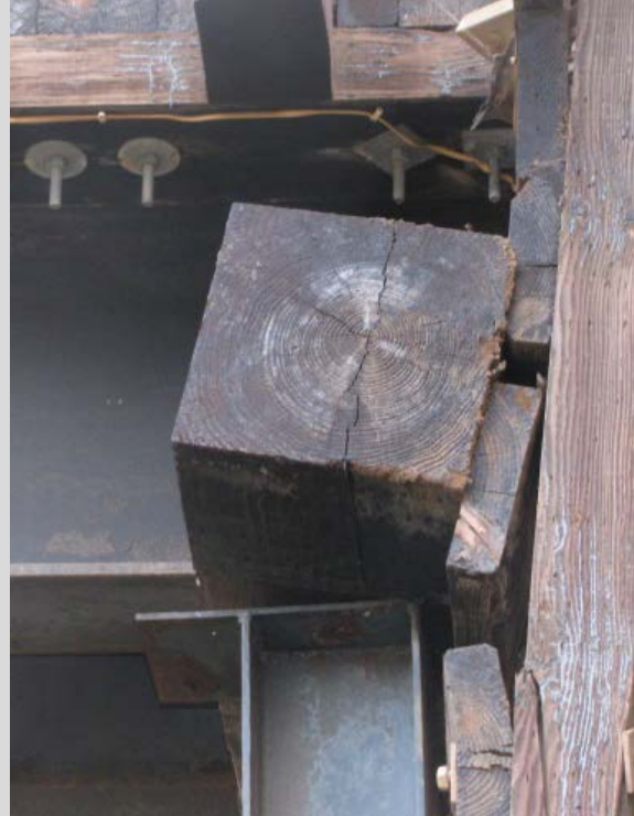
Condition State 3 Timber cap with significant misalignment (tipped) – not bearing fully on the steel piling
