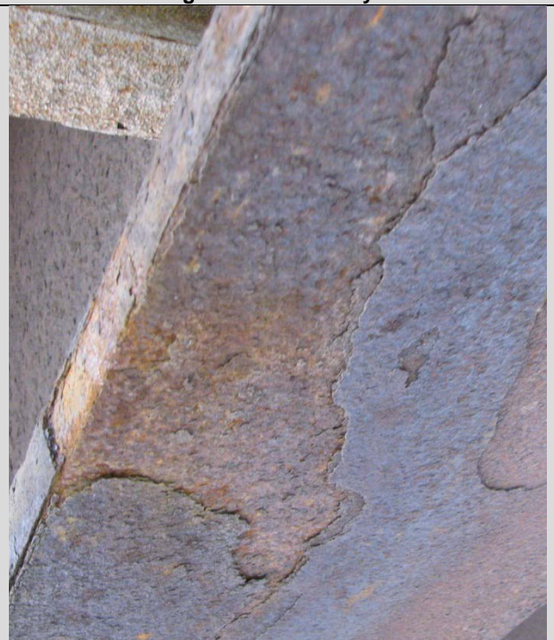
Condition State 4 Weathering steel patina has failed – large areas of surface layer flaking off.
