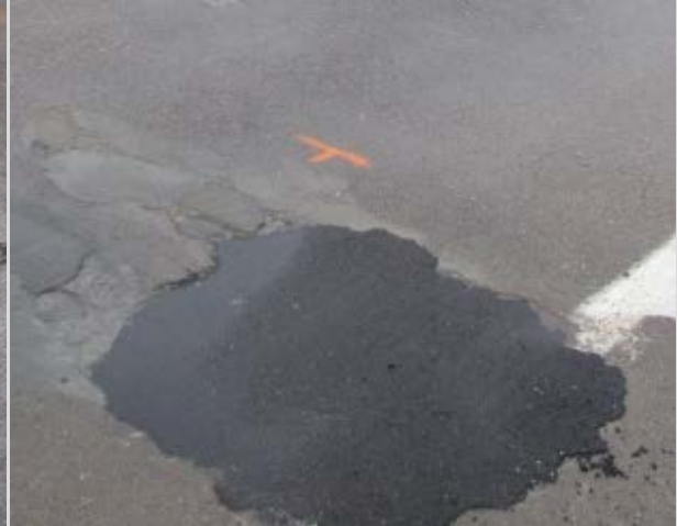
Condition State 3 Bituminous patch on a bare concrete deck
