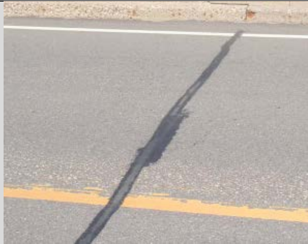
Condition State 2 Sealed crack on a bituminous overlay
