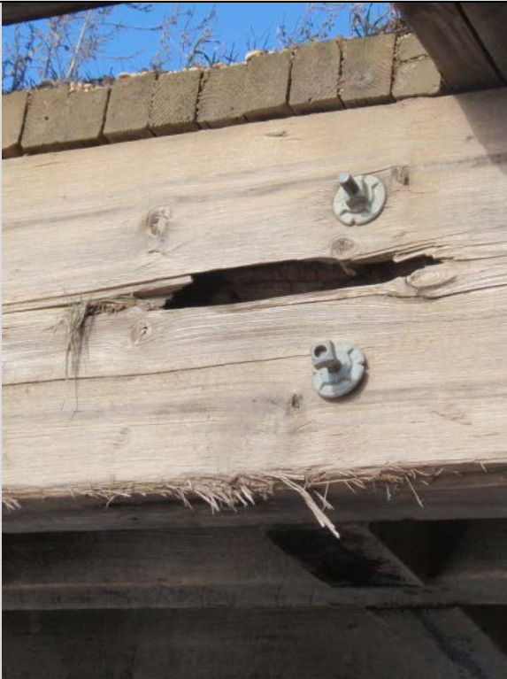
Condition State 4 Severe internal decay on a sawn timber beam
