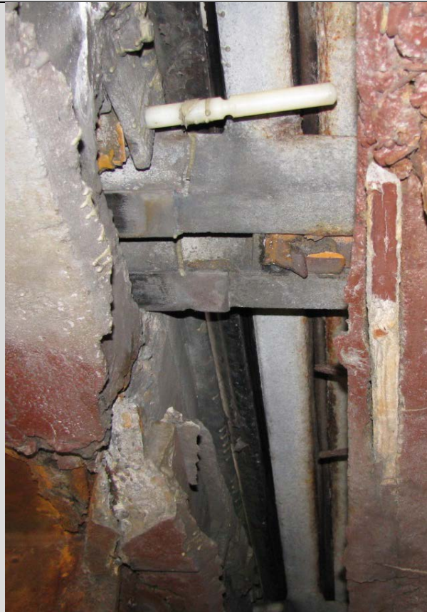
Condition State 3 Teflon pin on equalizer has nearly fallen out
