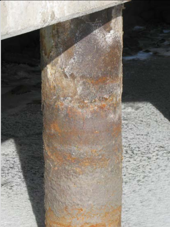
Condition State 3 Flaking rust on a CIP Pile
