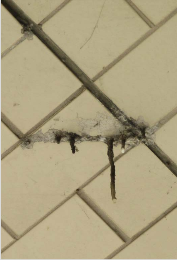
Condition State 2 Leaching crack in a tunnel ceiling
