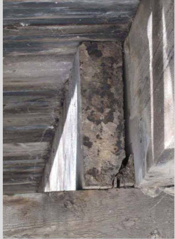
Condition State 3 Sawn timber beam – bottom corner fractured at pier bearing
