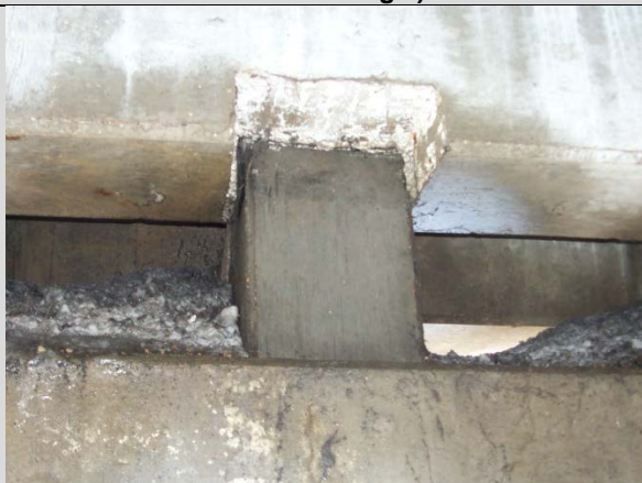
Concrete diaphragm offset excessively at shear key due to pier movement
