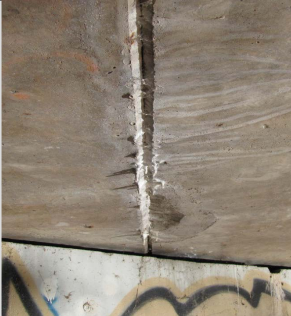
Condition State 2 Light leaching along joint between prestressed voided slab panels
