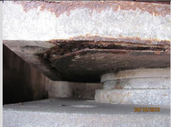
Condition State 3 Pack rust on the sliding plate on a free expansion pot bearing
