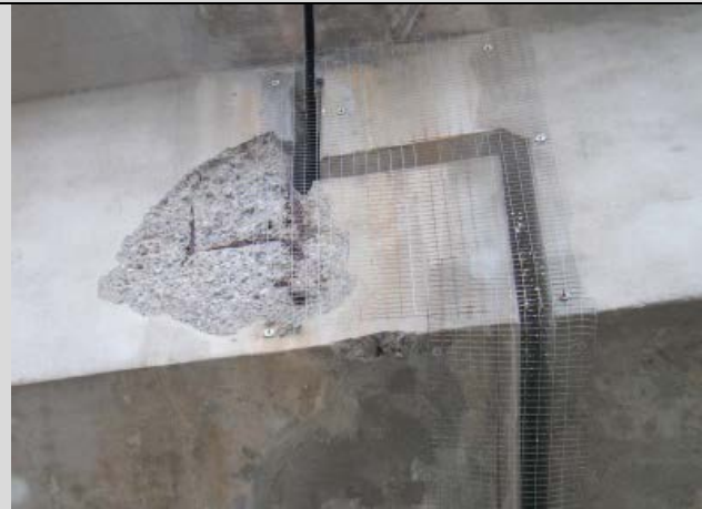
Condition State 3 Spalling on concrete box girder adjacent to hinge
