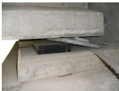
Severe malfunction of an elastomeric bearing
