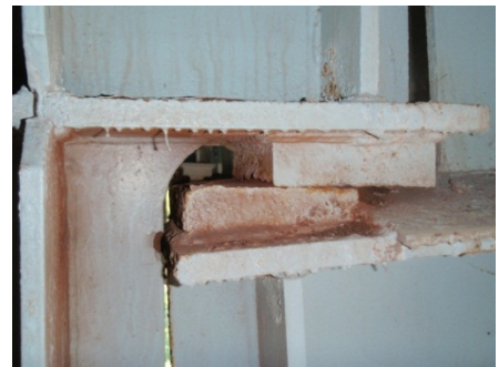
Hinge bearing in full expansion (beam ends contacting)
