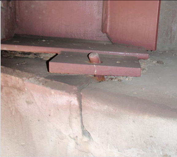
Condition State 3 Anchor bolt bent (and abutment seat spalled) on a fixed pad bearing
