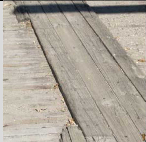
Condition State 4 Section of timber wearing plank missing
