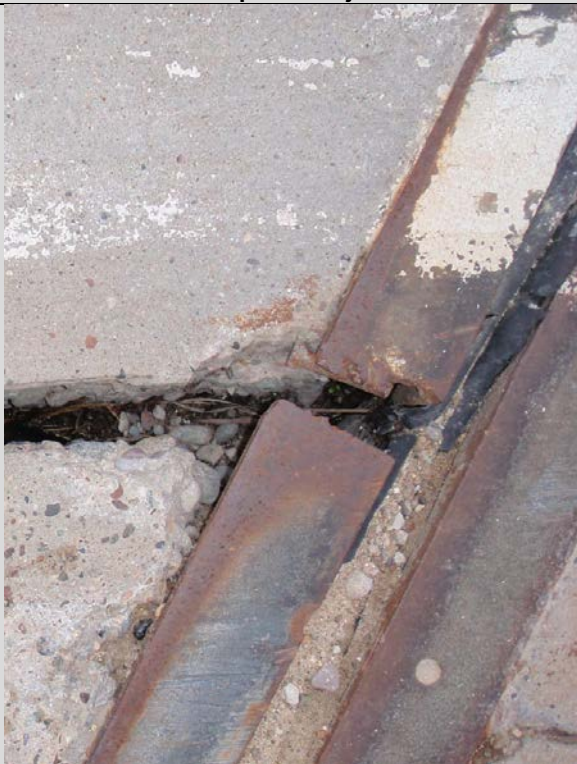
Condition State 4 Steel protection angle on a compression seal joint fractured and separated
