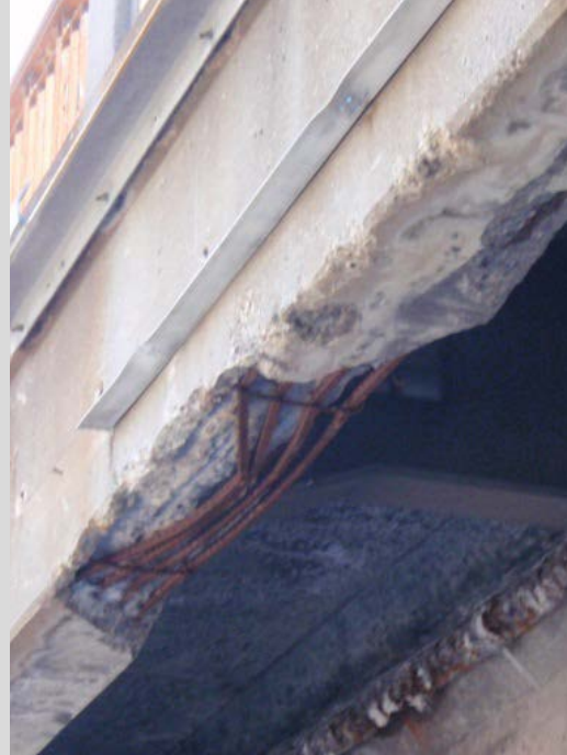
Condition State 4 Severe impact damage (exposed and bent reinforcement) on a cast-in-place concrete T-girder
