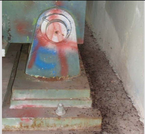
Condition State 3 Bats droppings on an abutment bearing seat
