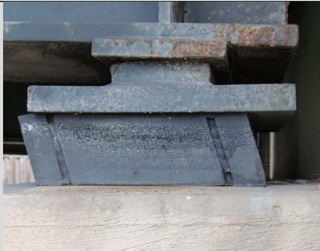
Condition State 3 Pad has moved out from beneath the sole plate (more than 1/2" but less than 2")
