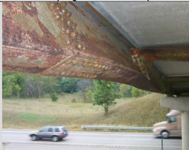
Condition State 4 Steel beam severely bent due to high load impact
