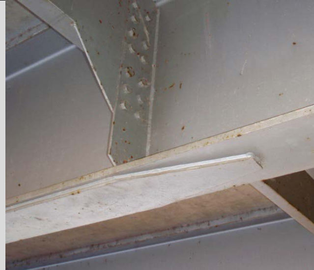
Condition State 1 Welded cover plate on the bottom flange of a rolled steel beam (fatigue prone detail)
