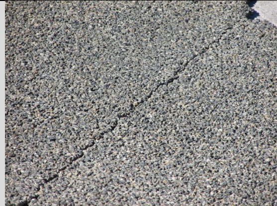
Condition State 3 Significant cracking on a chip seal overlay
