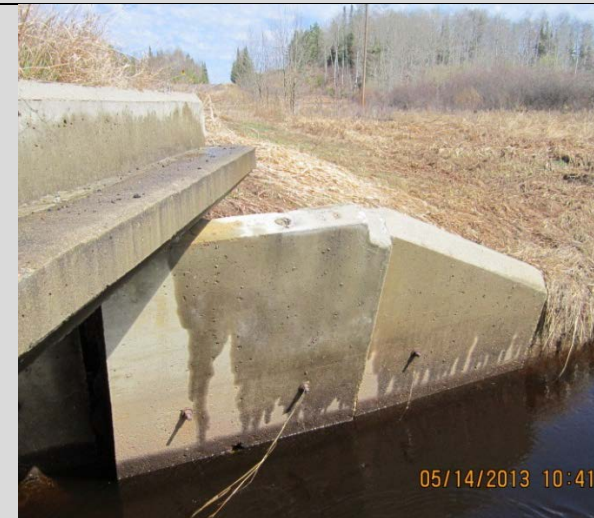
Condition State 3 Failed wingwall on a precast concrete box culvert
