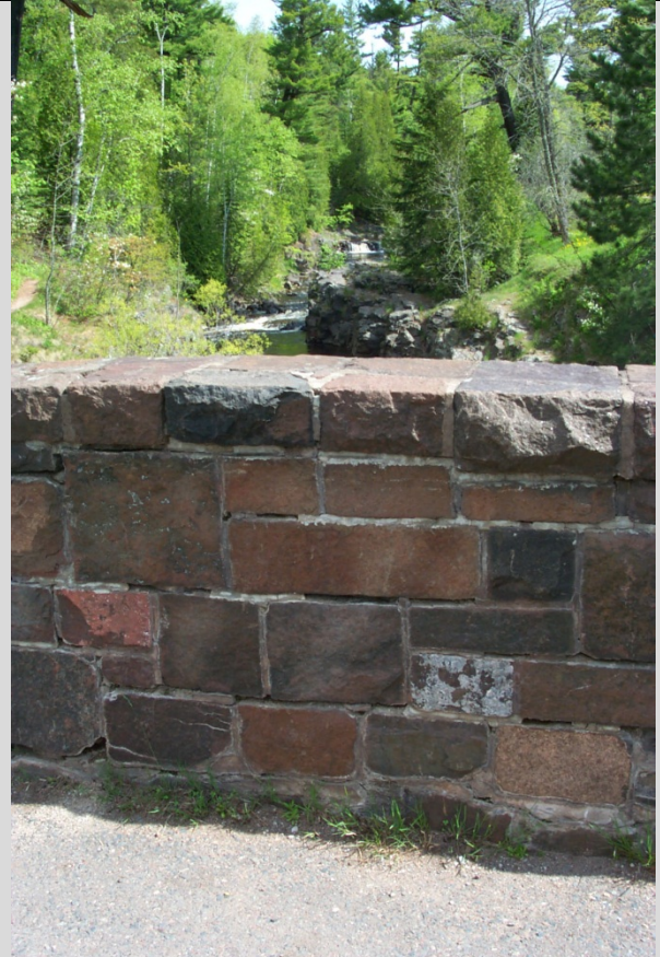
Condition State 3 Extensive mortar breakdown on a masonry bridge railing
