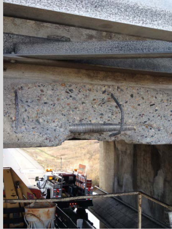
Condition State 3 Impact damage (spalling) on a post-tensioned concrete beam
