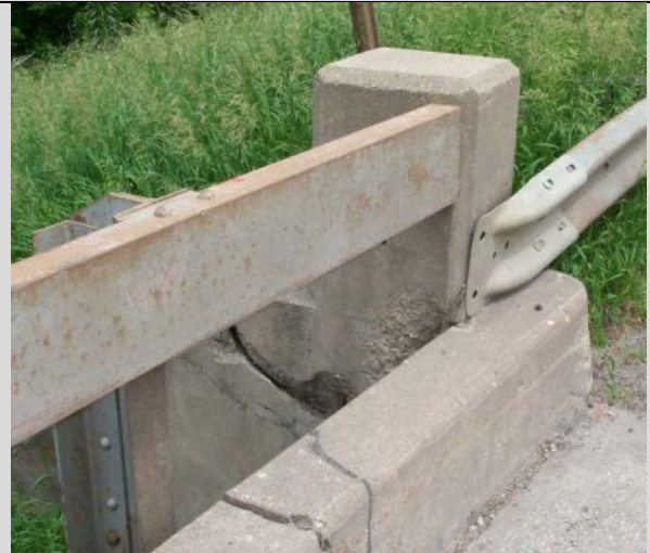
Condition State 3 End post fractured due to contact with deck & railing (abutment movement)
