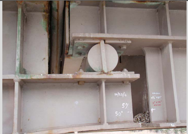
Condition State 2 Minor corrosion on a sliding plate hinge
