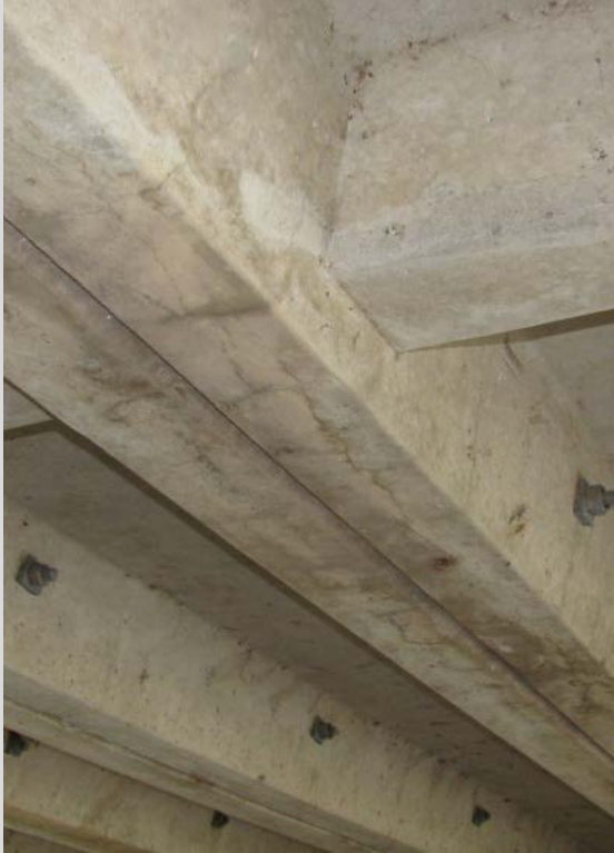
Condition State 2 Cracking on precast concrete channel beams
