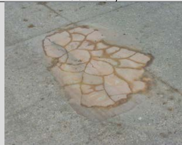
Condition State 3 Deteriorated patch on a bare concrete deck
