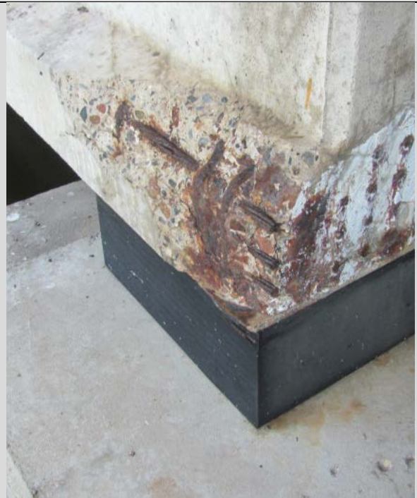
Condition State 3 Spalling on a bottom flange of a prestressed concrete beam
