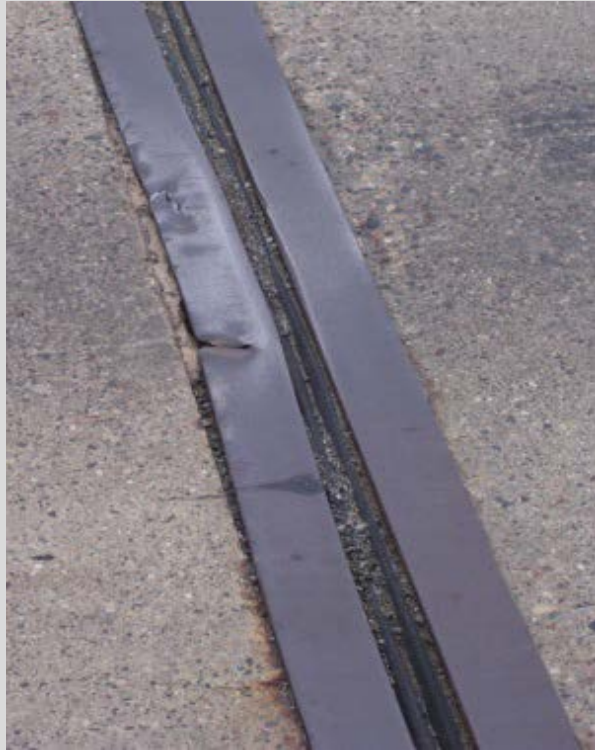
Condition State 2 Plow damage on steel protection angle along compression joint
