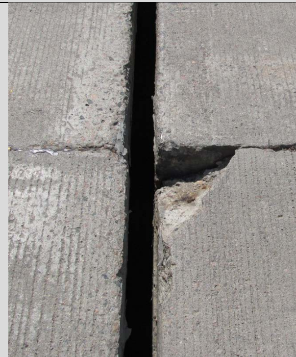
Condition State 3 Moderate spalling along an open deck joint (does not impact function or present a safety hazard)
