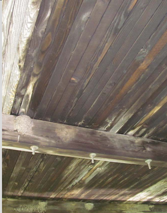
Condition State 2 Staining on the underside of a timber slab
