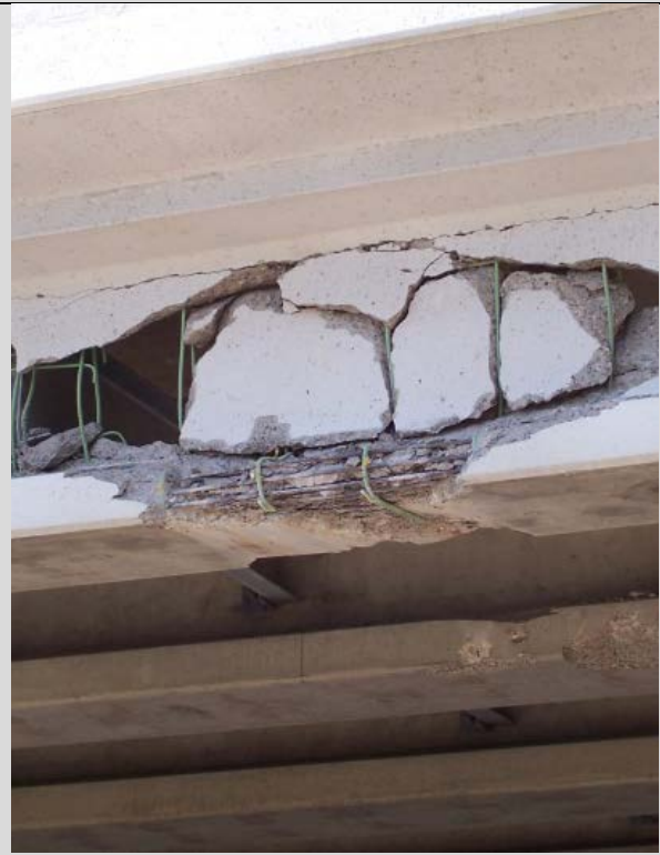
Condition State 4 Severe impact damage on a prestressed concrete beam
