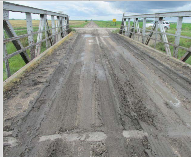
Condition State 3 Significant rutting on gravel wearing surface
