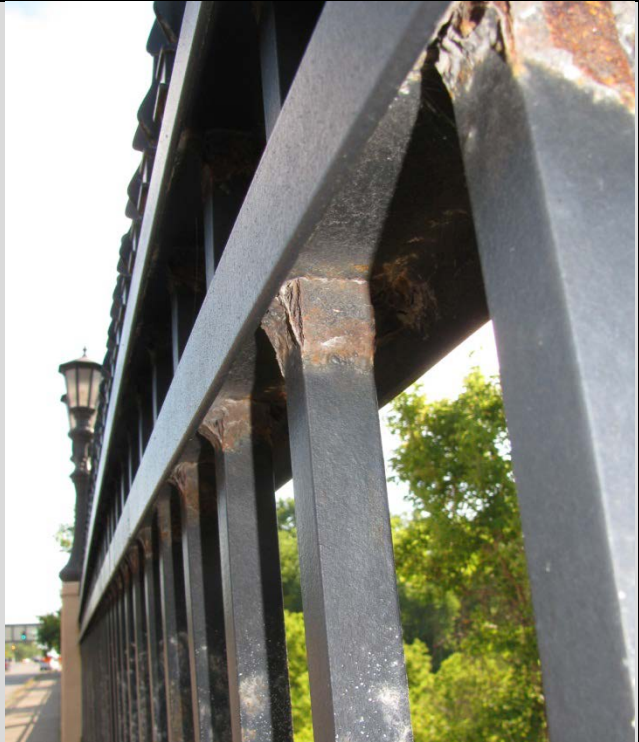
Condition State 4 Complete failure of a Duplex system on a steel railing (isolated locations)
