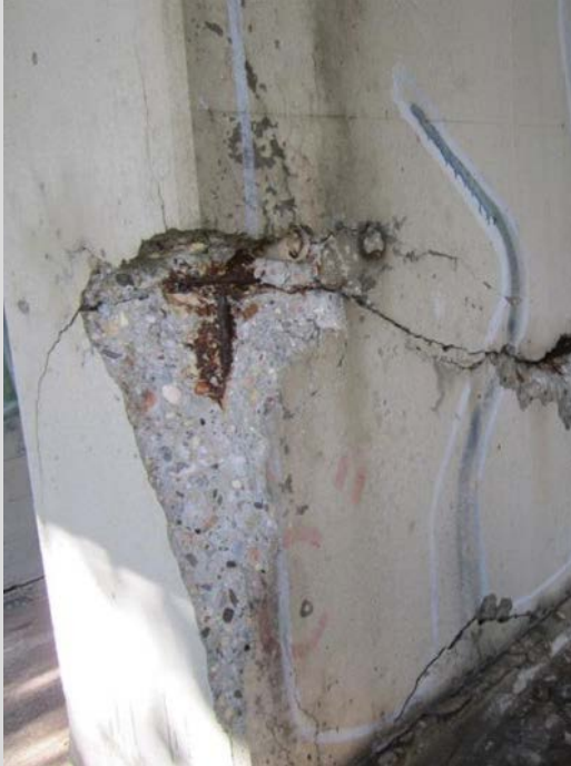
Condition State 4 Severe spalling (and fracture) on a concrete arch spandrel wall
