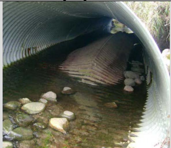
Condition State 4 Severe barrel distortion
