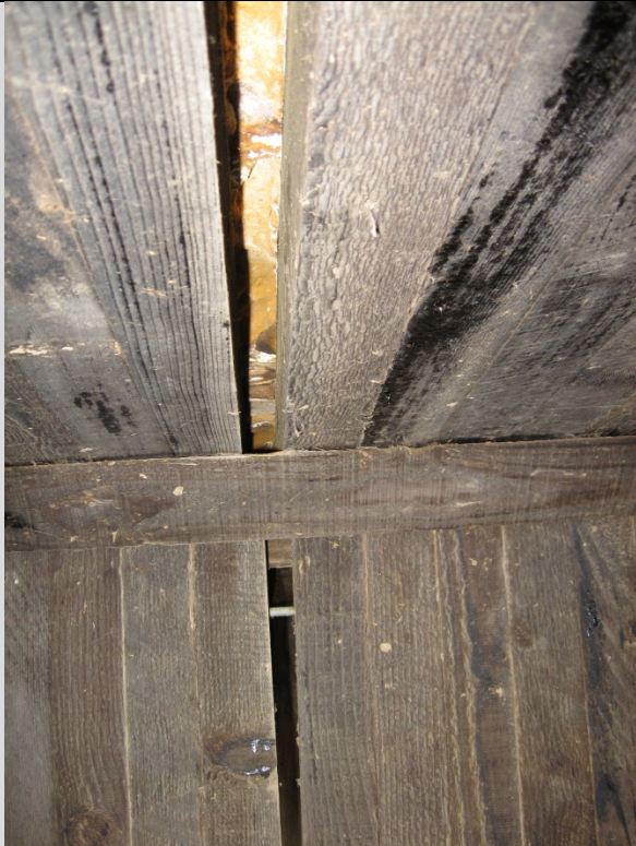
Condition State 2 Separation between timber members on a timber box culvert (no backfill infiltration)
