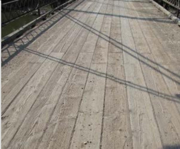
Condition State 1 Minor weathering on timber wearing planks
