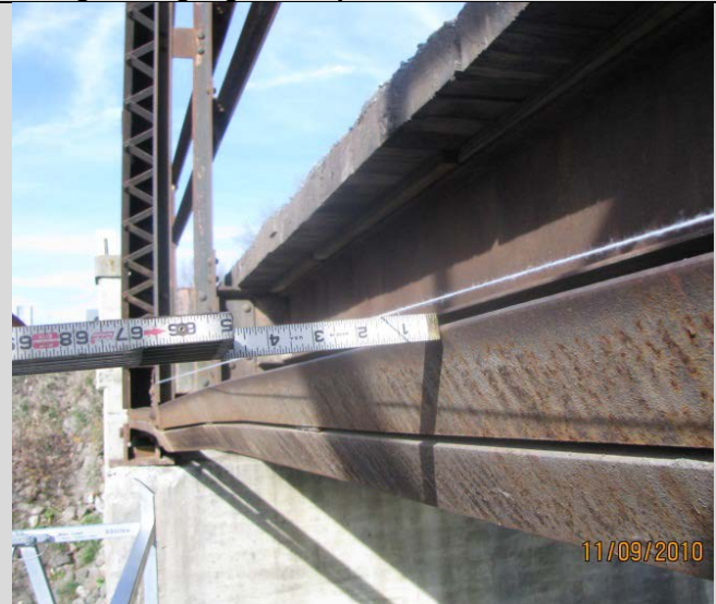
Condition State 3 Ice or flood damage to a truss bottom chord
