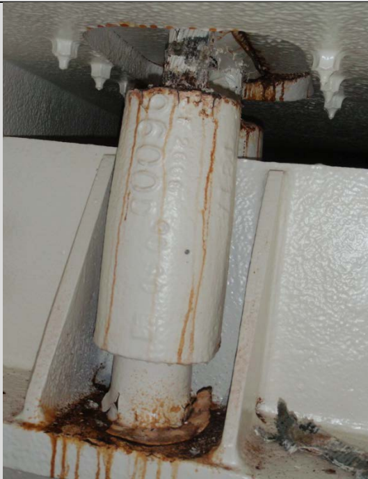
Condition State 3 Corrosion on steel strand hanger cable just above the anchorage socket
