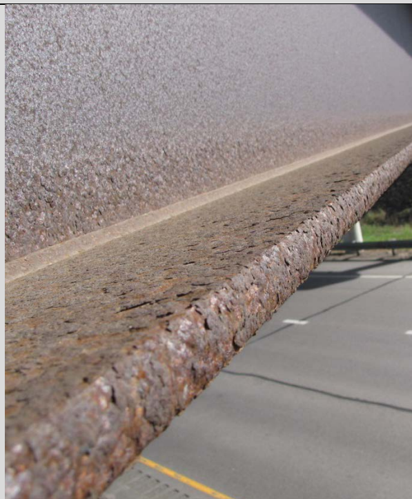
Condition State 3 Weathering steel patina has flaking (less than 1/2" diameter) along the bottom flange
