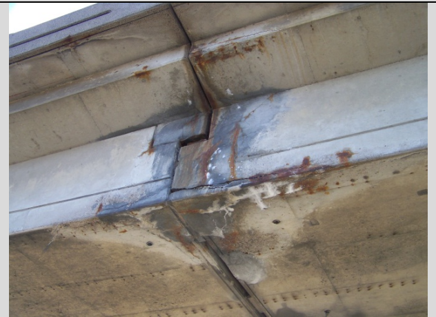
Condition State 3 Rust staining and cracking in concrete box girder at hinge joint
