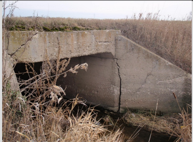
Condition State 3 Fractured wingwall on a cast-in-place (CIP) concrete box culvert
