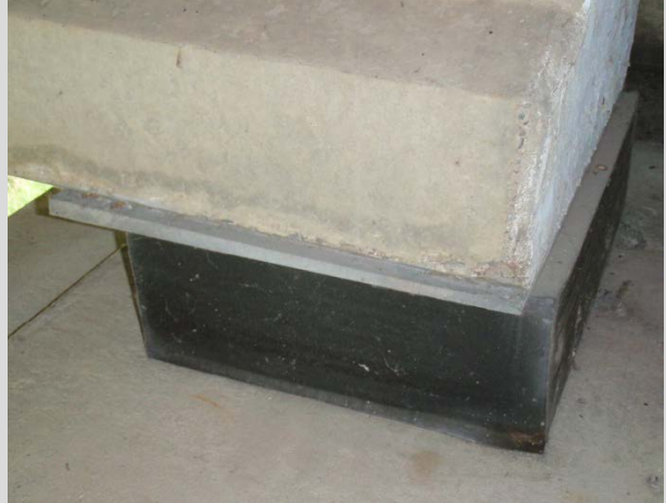
Condition State 2 Pad rolled up slightly on the bottom edge and moved from beneath sole plate (less than 1/2")
