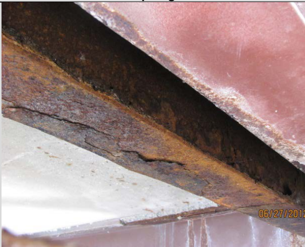
Condition State 3 Flaking rust (section loss) on a steel diaphragm
