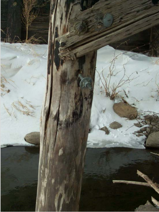
Condition State 3 Timber pile with splitting and decay at a bracing connection
