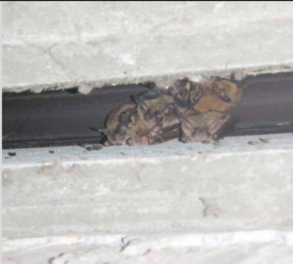
Condition State 3 Bats on the underside of a strip seal deck joint
