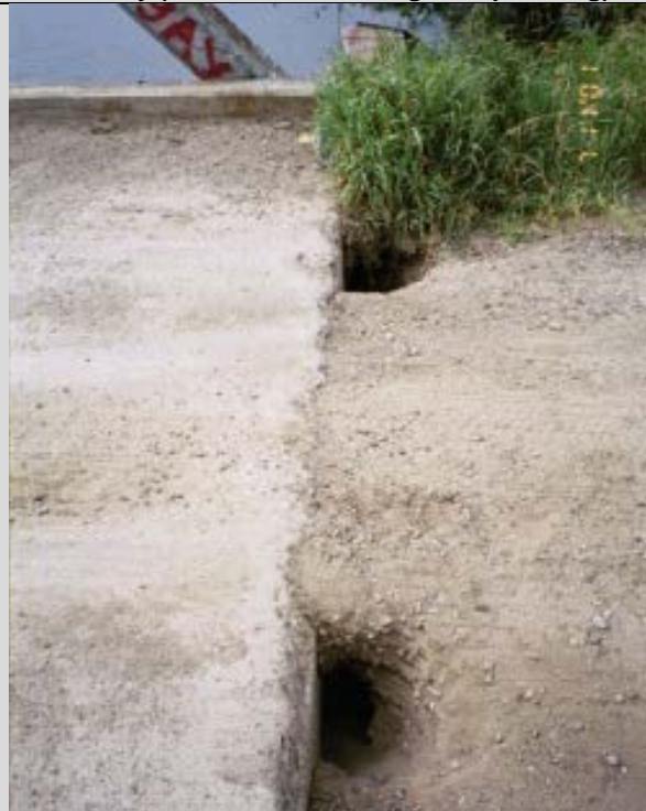
Condition State 4 Severe washouts on a gravel approach roadway (traffic hazard)
