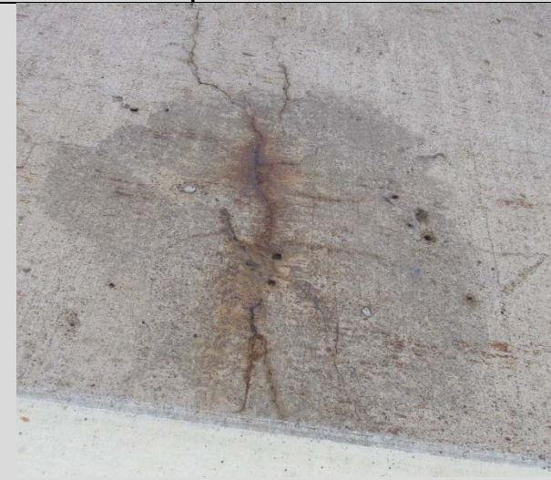
Condition State 3 Map cracked area with rust staining on a bare concrete deck
