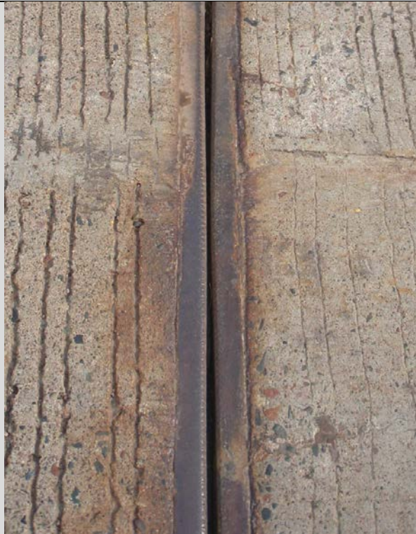
Condition State 4 Strip seal deck joint closed to less than a 1/2" gap
