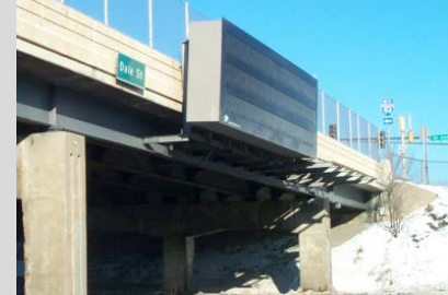
Dynamic Message Sign (DMS) mounted on bridge fascia
