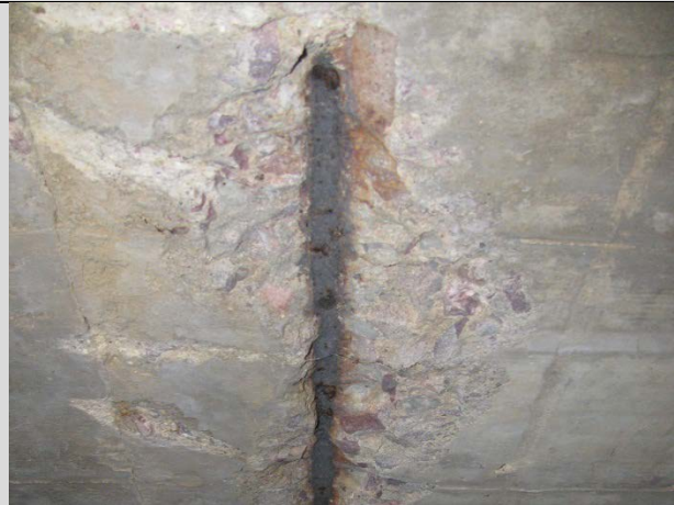
Condition State 3 Spalling (exposed rebar) on a cast-in-place (CIP) concrete box culvert
