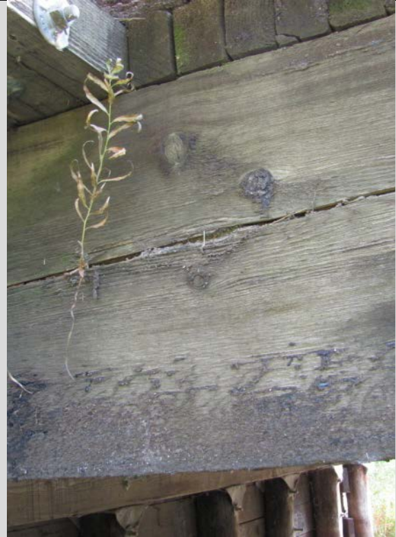
Condition State 3 Horizontal splitting with internal decay (plant growth) on a sawn timber beam
