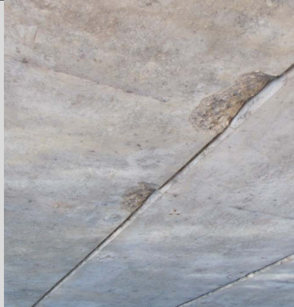
Condition State 2 Minor spalling (no exposed steel) along the edge of a prestressed voided slab panel
