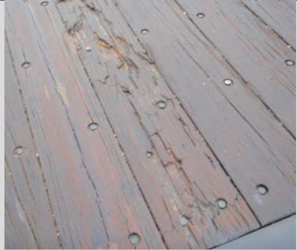
Condition State 2 Moderate weathering on a timber wearing plank
