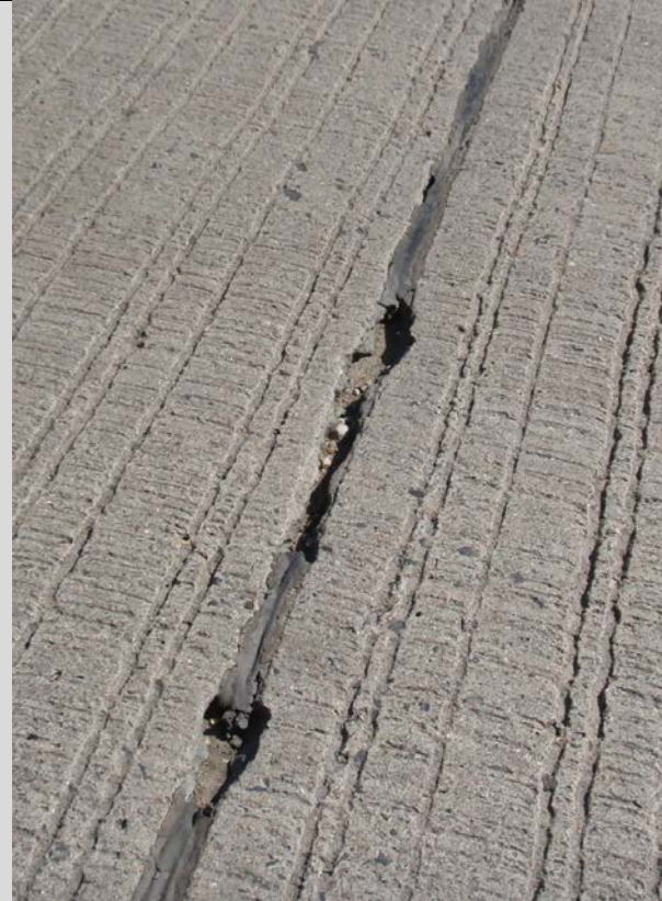
Condition State 3 Section of poured seal missing
