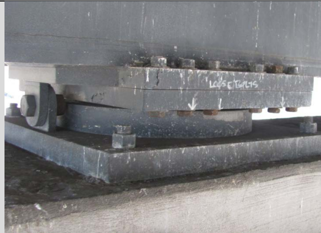
Condition State 2 Loose sole plate bolts on a fixed pot bearing
