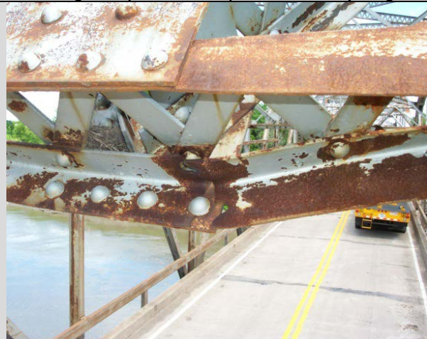
Condition State 4 Truss portal brace fractured
