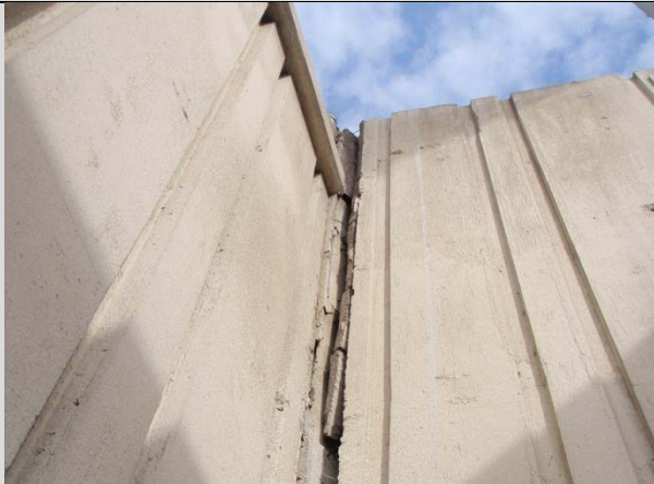
Condition State 2 Wingwall separation due to abutment movement
