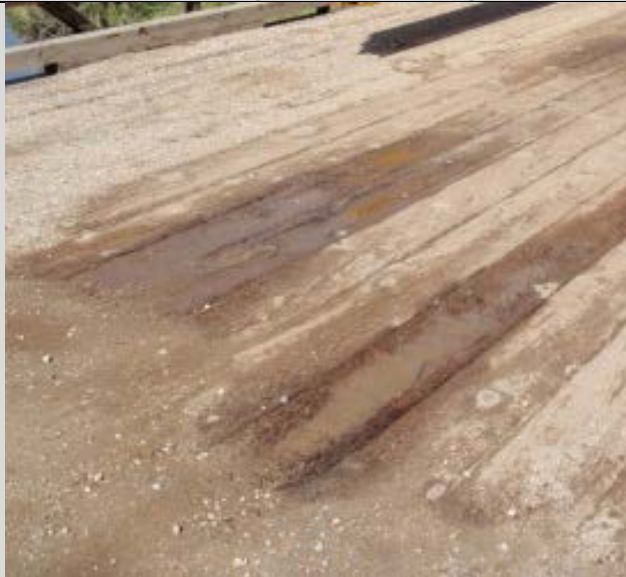
Condition State 3 Significant weathering/decay on timber wearing planks
