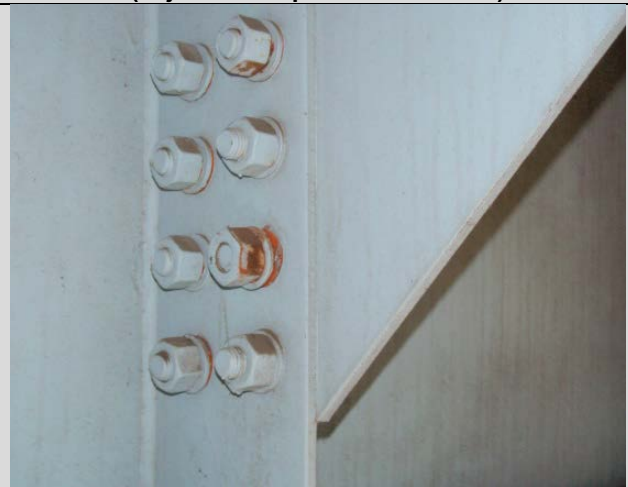
Condition State 3 Loose bolts on a steel diaphragm connection
