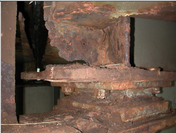
Condition State 4 Severe corrosion on a sliding plate hinge (severe section loss in beam web above hinge)
