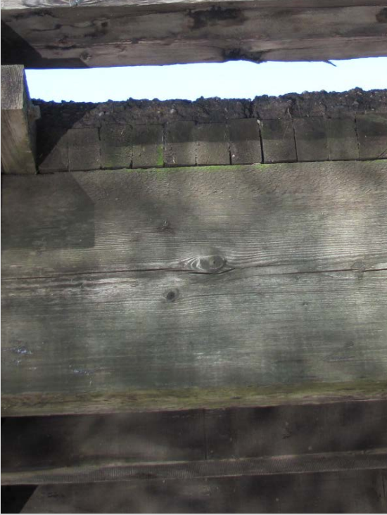
Condition State 2 Moderate horizontal splitting on a sawn timber beam
