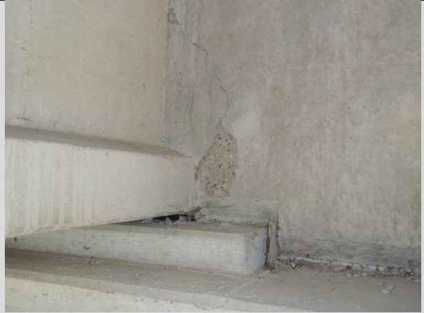
Condition State 2 Delamination and spall on a concrete end diaphragm (adjacent to a prestressed beam)
