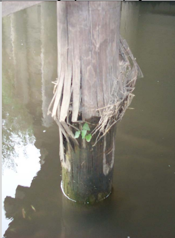
Condition State 4 Timber pile with severe decay and crushing
