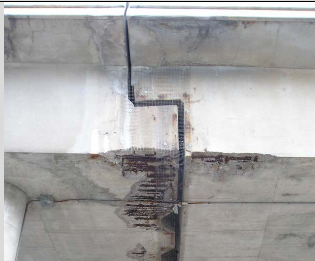
Condition State 4 Extensive (and severe) spalling on concrete box girder adjacent to hinge
