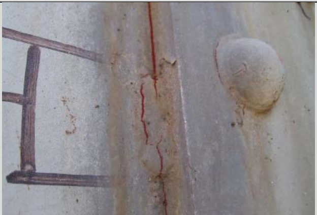
Condition State 2 Partially cracked tack weld along connection plate (could potentially propagate into base metal)
