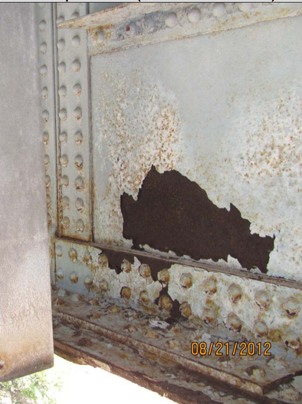
Condition State 4 Paint system failure (exposed steel)
