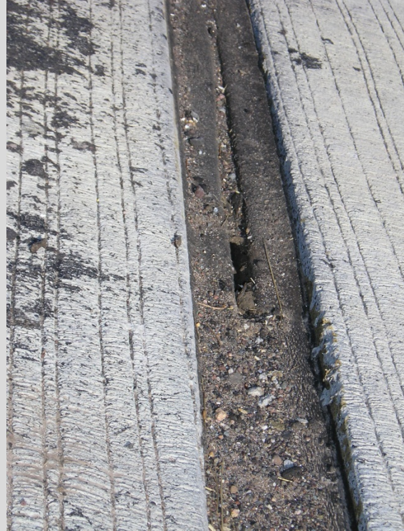
Condition State 2 Partial failure of poured seal on an approach relief joint
