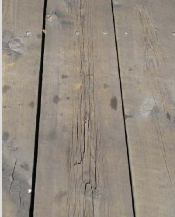
Condition State 2 Weathering on timber plank deck
