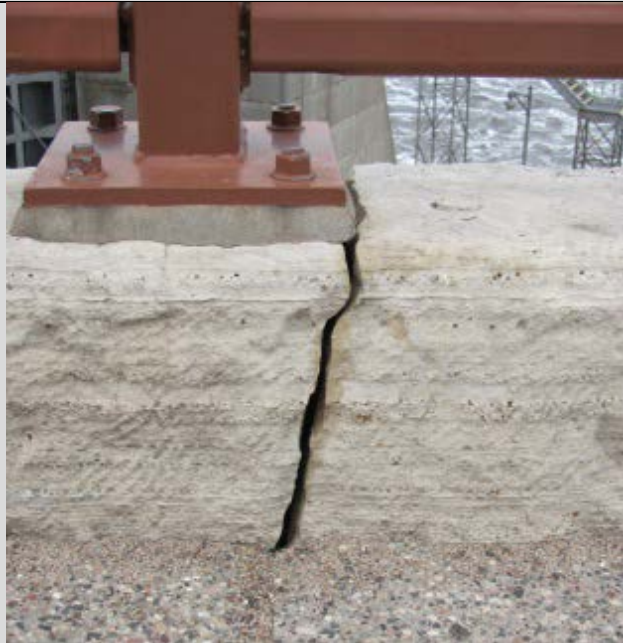
Condition State 3 Block split on a masonry parapet
