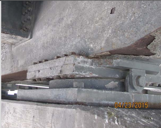
Condition State 2 Paint/galvanizing failure and surface corrosion on a fixed pot bearing
