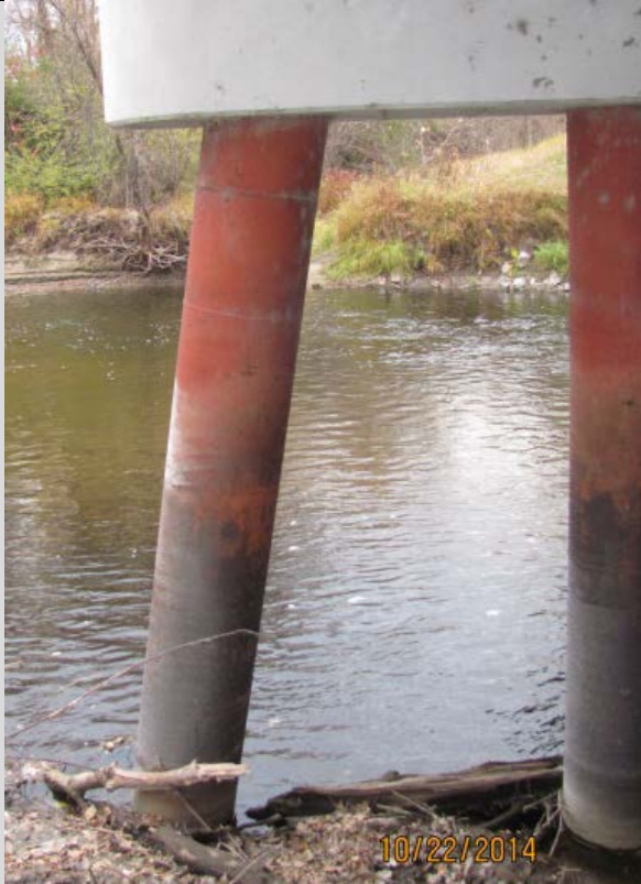
Condition State 2 Paint failure and surface corrosion on a CIP Pile
