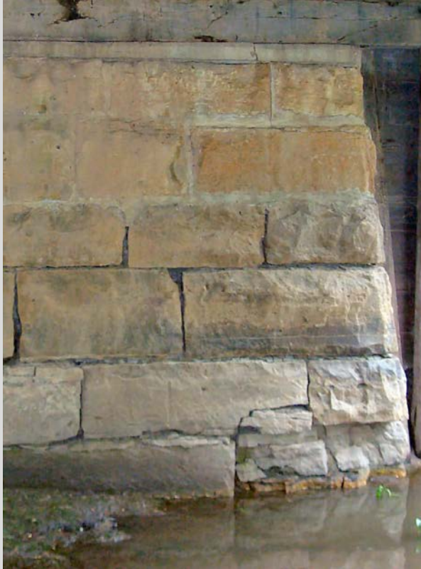
Condition State 3 Mortar failure and spalling on masonry block (10%-25% of block thickness)
