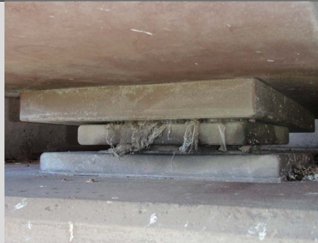
Condition State 3 Teflon shavings due to wear on the sliding surface of a free expansion pot bearing
