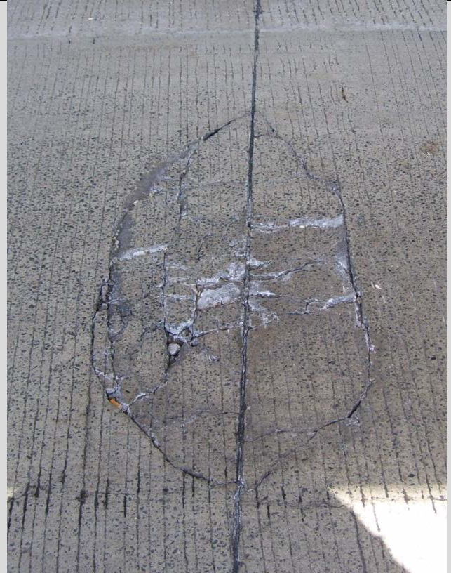
Condition State 4 Cracking and delamination adjacent to a transverse poured deck joint
