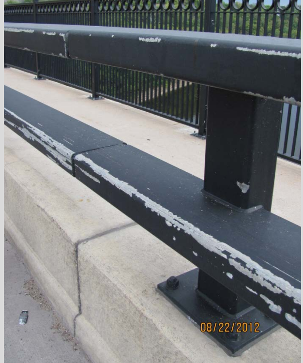
Condition State 3 Finish paint coat (Duplex system) has been scraped off, the galvanized layer below remains intact
