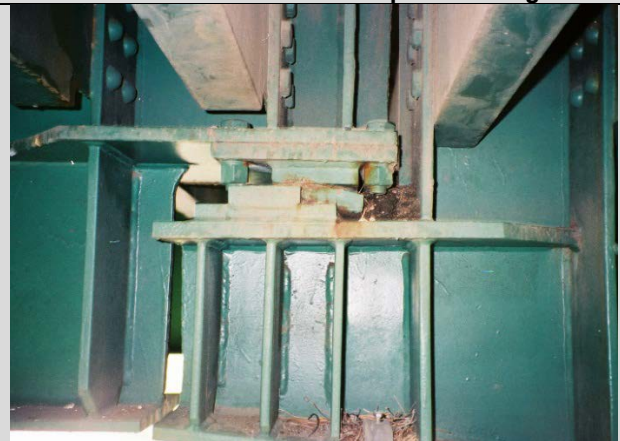
Condition State 4 Sliding plate hinge locked in expansion (curved slide plate tipped)
