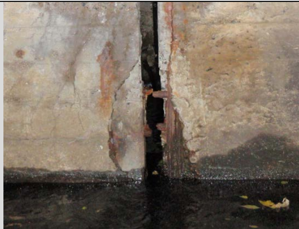
Condition State 4 Severe separation and deterioration at a construction on a cast-in-place (CIP) concrete box culvert
