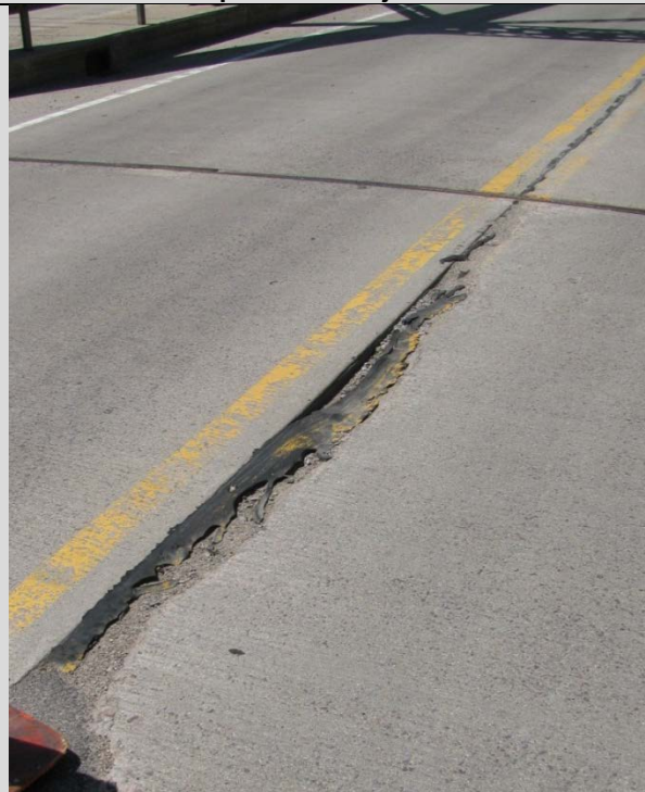
Condition State 4 Severe spalling along a longitudinal poured joint
