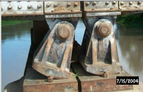
Bearing misalignment due to substructure movement (the rockers should be tipped in opposite directions at the same angle)
