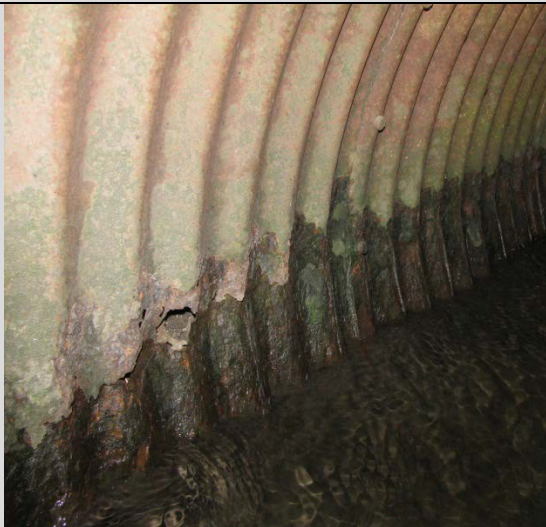
Condition State 4 Through corrosion along the waterline
