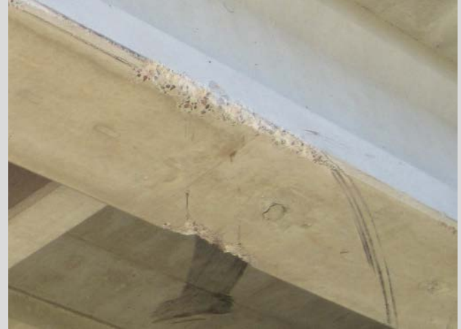
Condition State 2 High load gouges on a prestressed concrete beam
