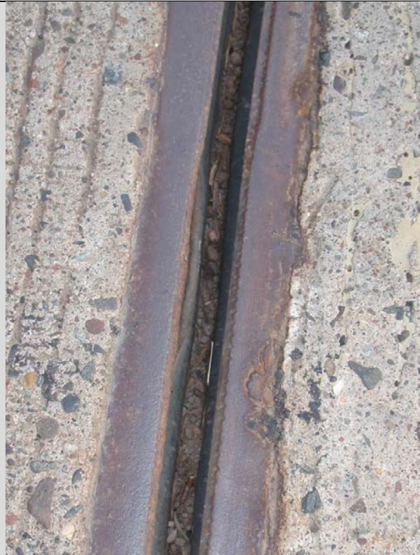
Condition State 2 Strip seal gland partially pulled out
