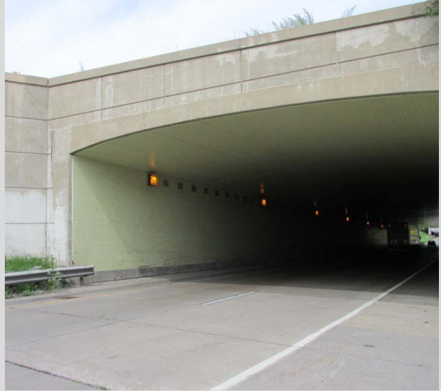
Condition State 1 Concrete roadway through a tunnel
