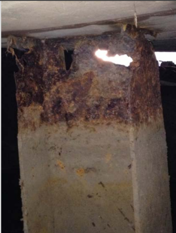
Condition State 4 Severe corrosion and section loss on a steel h-pile
