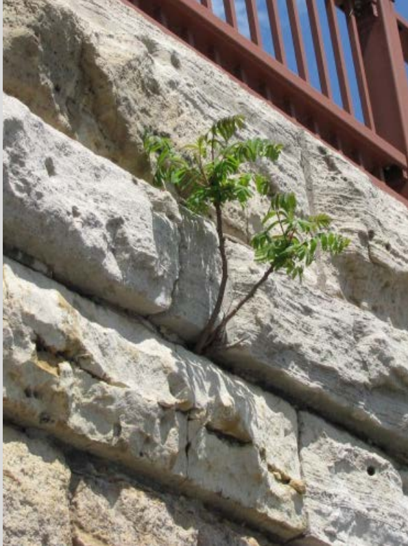
Condition State 2 Mortar breakdown (plant growing in masonry joint)
