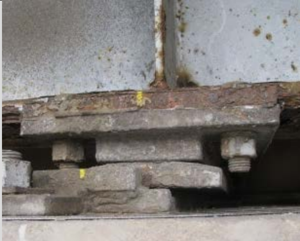
Condition State 3 Sliding plate bearing near expansion limits (slide plate extends well beyond the masonry plate)
