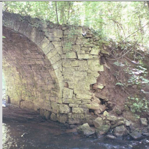
Condition State 4 Wingwall failure on a masonry arch culvert
