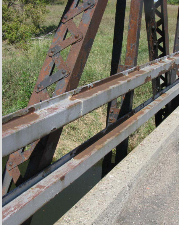
Condition State 2 Surface corrosion on steel rail beams
