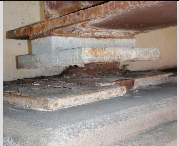
Condition State 3 Flaking rust on a free expansion pot bearing
