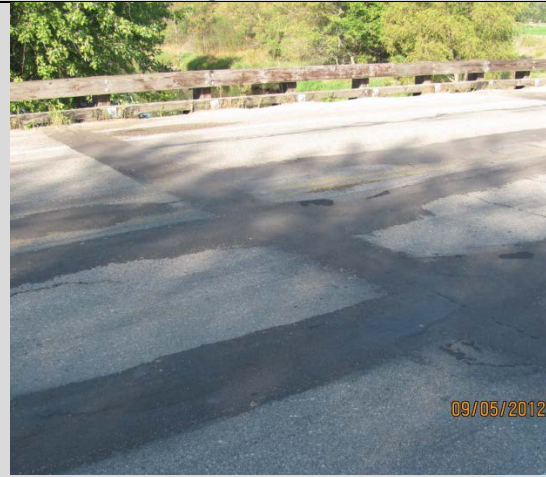
Condition State 2 Sound patches on a bituminous overlay
