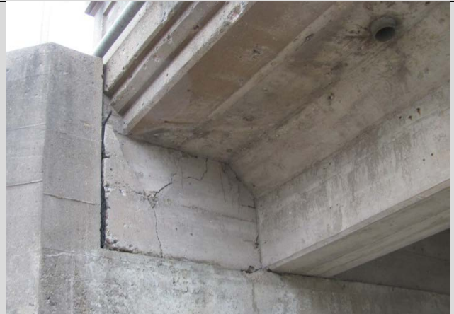
Condition State 2 Abutment end diaphragm offset and fractured due to abutment movement
