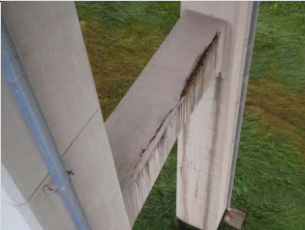
Condition State 3 Spalling on a concrete pier strut
