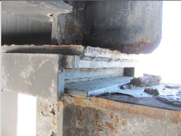
Condition State 2 Minor corrosion on a sliding plate hinge
