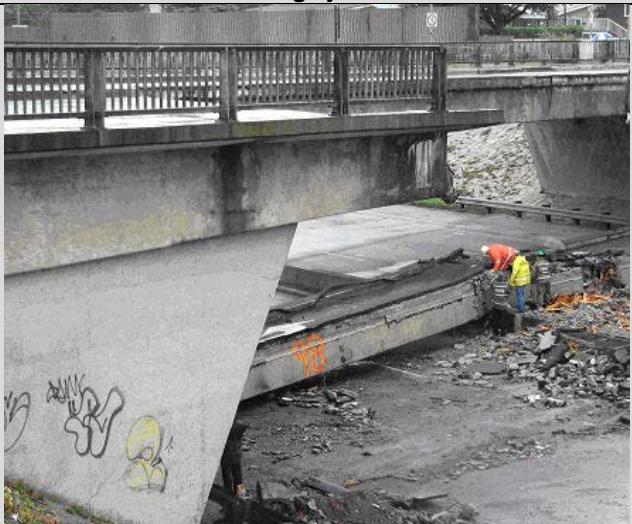
Bridge collapse in Montreal Canada (2006) due to failure of concrete hinge resulted in 5 fatalities
