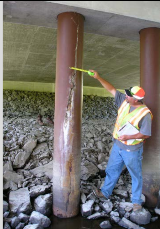
Condition State 4 Fracture in steel shell of a CIP Piling
