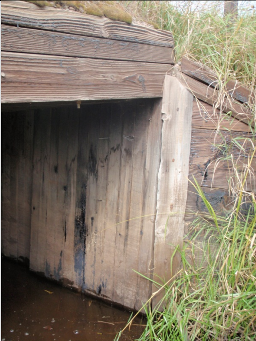
Condition State 3 Wall section misaligned on a timber box culvert
