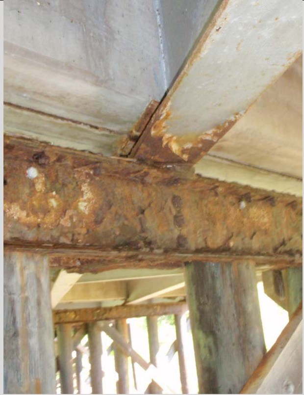
Condition State 3 Leakage through and open deck joint resulting in severe corrosion of superstructure below
