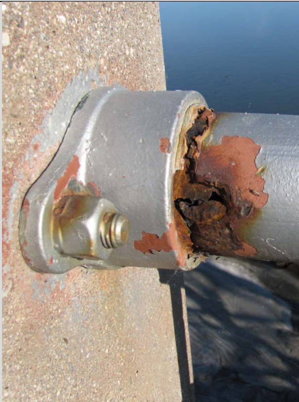
Condition State 4 Horizontal steel rail pipe rusted through at connection to a concrete post
