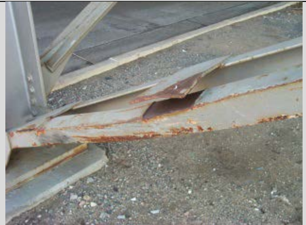
Condition State 3 Steel pier brace bent (batten plate detached)
