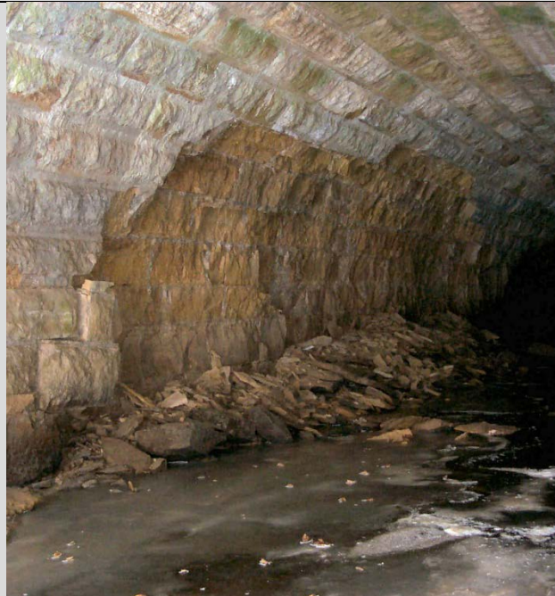
Condition State 4 Severe (and extensive) spalling on a masonry arch culvert
