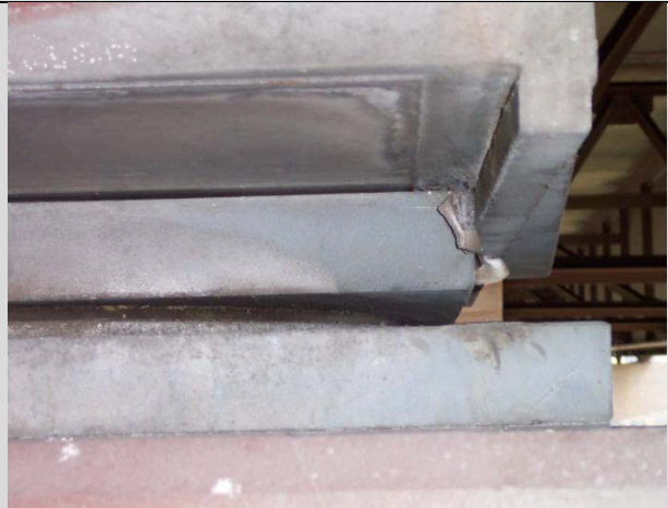
Condition State 2 Teflon stop peeling off from the guide bar on a guided expansion pot bearing
