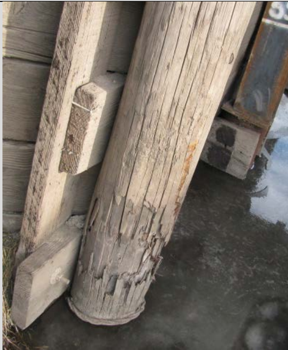
Condition State 3 Shell damage on a timber piling (section loss between 10% and 40%)
