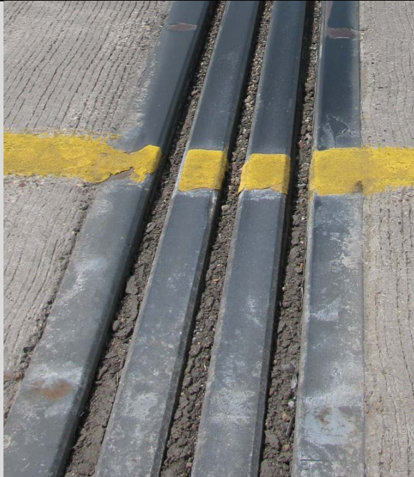
Condition State 2 Modular joint seals filled with debris
