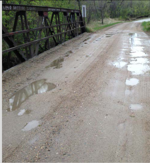
Condition State 2 Moderate ponding on a gravel wearing surface
