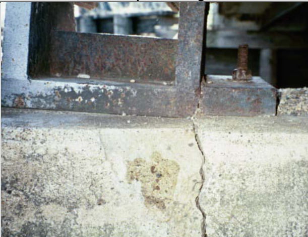
Condition State 4 Masonry plate cracked (and supporting pier fractured) on a fixed pin bearing
