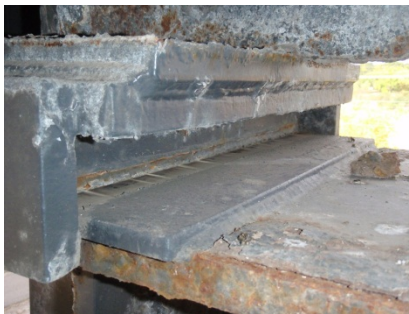
Scrape marks on a sliding plate hinge bearing indicate recent movement
