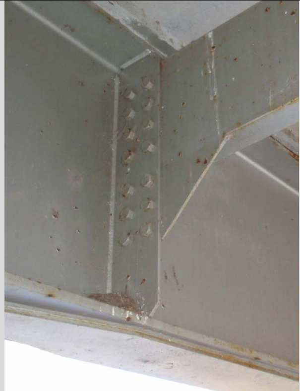
Condition State 2 Minor paint failure (Isolated – less than 3%)
