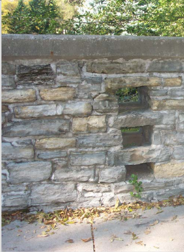
Condition State 2 Minor mortar breakdown on a masonry bridge railing
