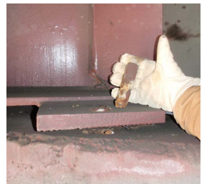
Anchor bolt failure on a fixed bearing
