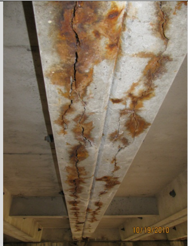
Condition State 3 Cracking, delamination, and rust staining a precast concrete channel beam
