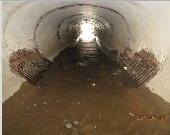
Condition State 4 Severe spalling on a precast concrete elliptical culvert
