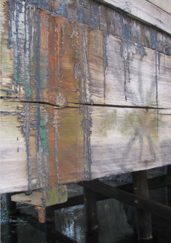
Condition State 3 Significant horizontal splitting on a sawn timber beam
