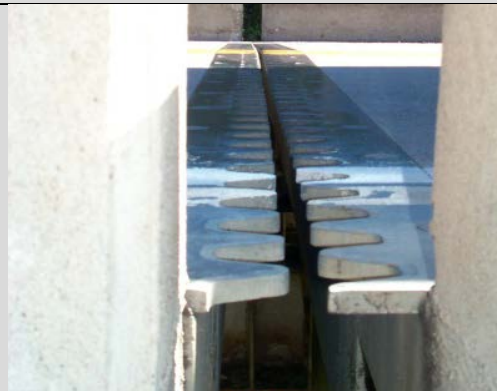
Finger joint open beyond design limits due to substructure movement
