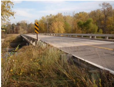
1). Roadway across Bridge
