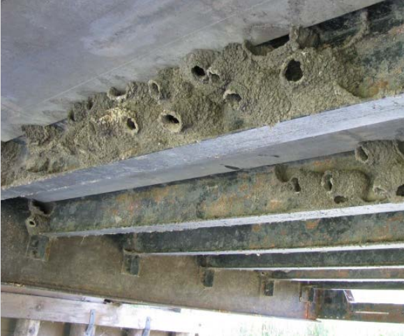
Condition State 2 Cliff Swallow nests present on the underside of a bridge
