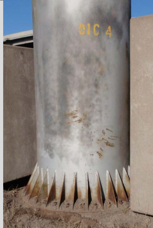
Condition State 2 Paint failure and surface corrosion on a steel column
