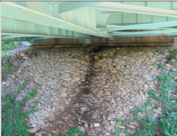
Condition State 3 Bats droppings on a slope below a deck median joint
