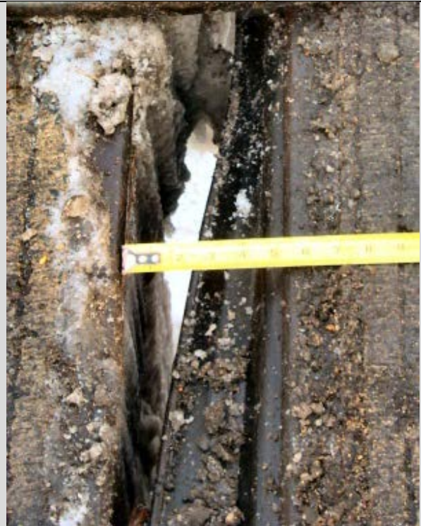
Condition State 4 Joint open beyond design limits (5" gap) - the gland has pulled out of the steel extrusion
