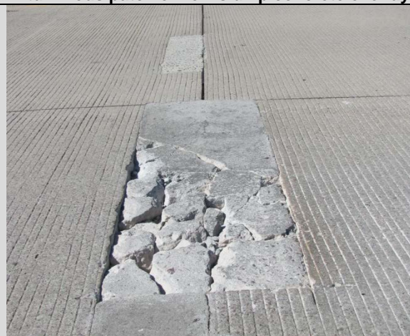
Condition State 4 Failed patch on low slump concrete overlay
