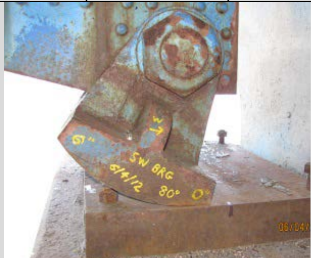
Condition State 4 Rocker bearing locked and sliding on the masonry plate
