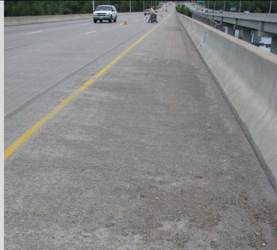
Condition State 2 Scaling on low slump concrete overlay
