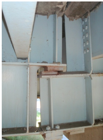
Misaligned hinge bearing
