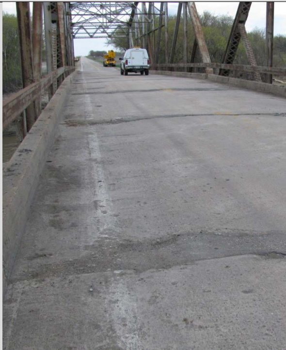
Condition State 4 Extensive deck deterioration (bituminous patching) along transverse poured deck joints
