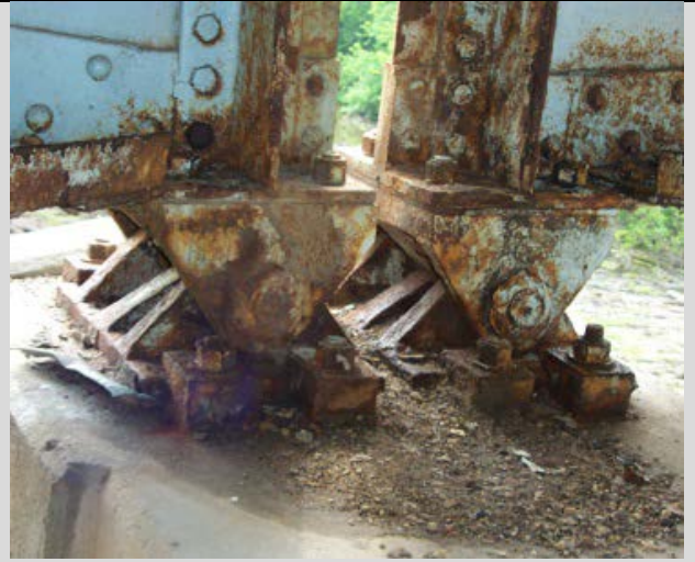
Condition State 3 Flaking rust and debris on two fixed pin bearings
