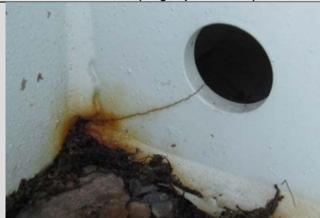
Condition State 2 Crack in girder web has arrested with a drilled hole
