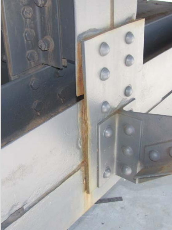
Condition State 3 Pack rust along truss connection
