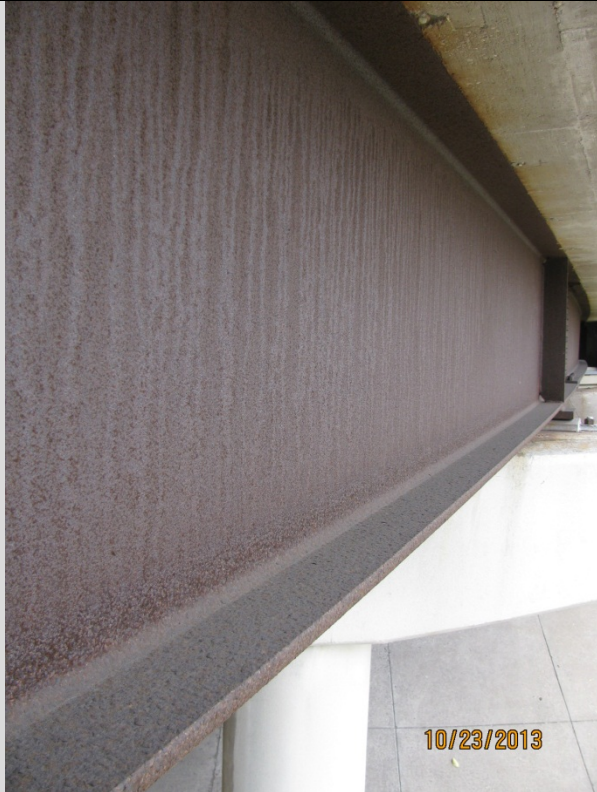
Condition State 1 Weathering steel patina is uniform and tightly adhered to the steel beam
