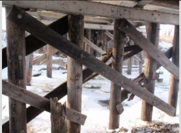
Condition State 4 Severe ice damage to timber pier bracing planks
