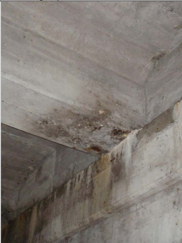
Condition State 3 Water saturation, rust staining, and spalling on a cast-in-place concrete T-girder
