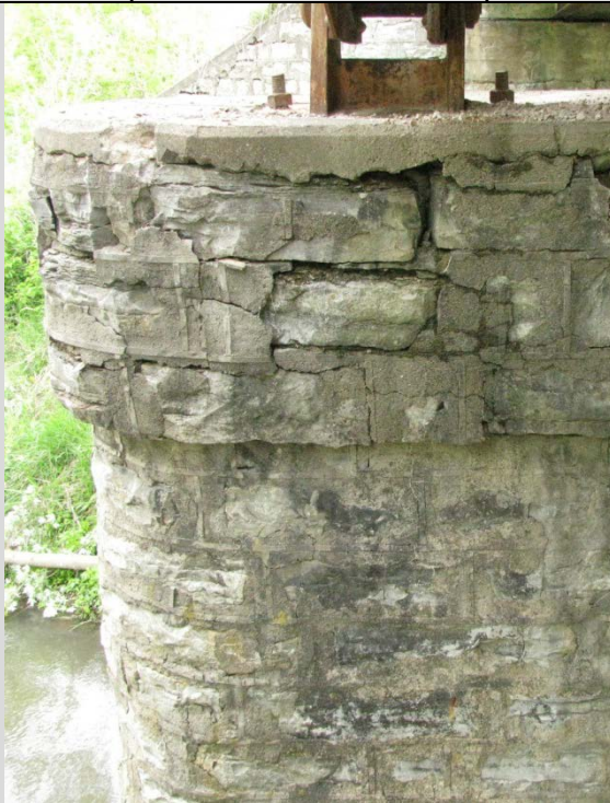
Condition State 4 Masonry pier wall severely deteriorated below a truss bearing
