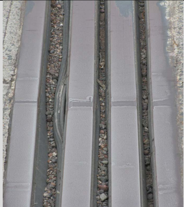
Condition State 3 Modular joint gaps are uneven (equalizer system is not functioning properly) - one gland is pulled out.
