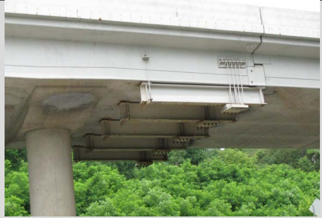
Condition State 2 Structural retrofit at a hinge joint in a concrete box girder
