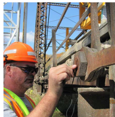
Ultrasonic Examination of a Pinned Truss Connection
