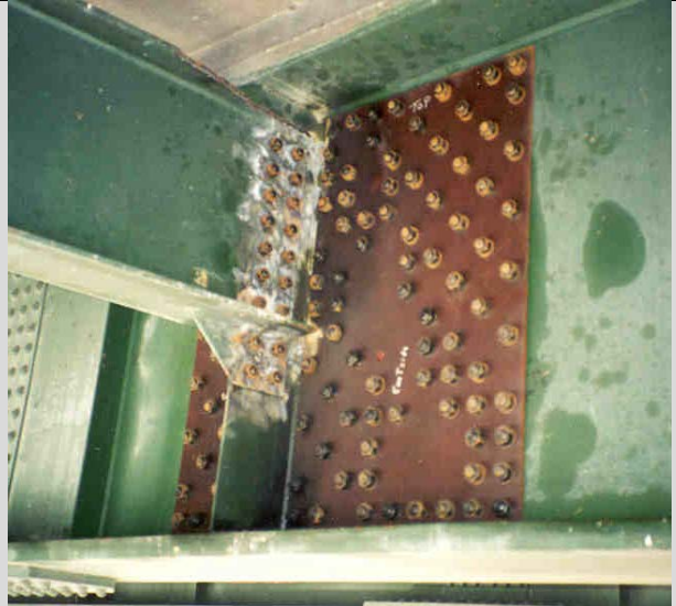
Condition State 2 Fractured beam web reinforced with bolted plates
