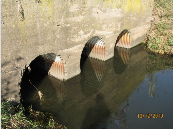
Condition State 2 Cracking and scale on a concrete headwall (3-barrel steel pipe culvert)
