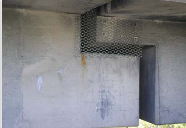
Condition State 2 Cracking on concrete adjacent to hinge adjacent concrete
