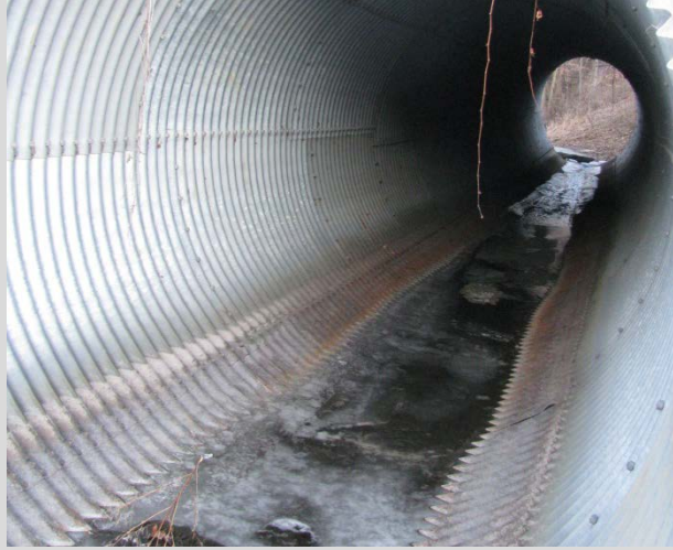
Condition State 2 Minor surface corrosion along the waterline
