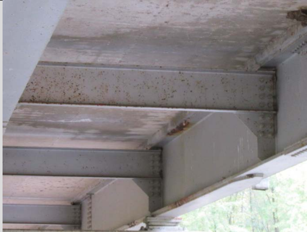
Condition State 2 Surface corrosion (freckled rust) on a steel diaphragm
