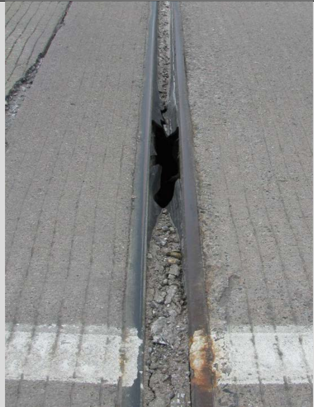
Condition State 3 Hole in strip seal gland
