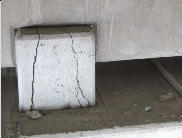
Condition State 3 Fractured shear key on a concrete pier cap
