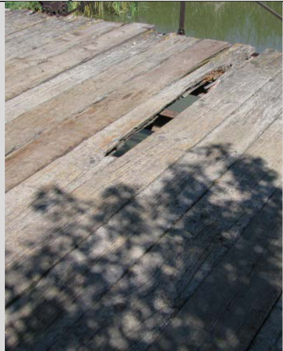
Condition State 4 Hole in a timber plank deck
