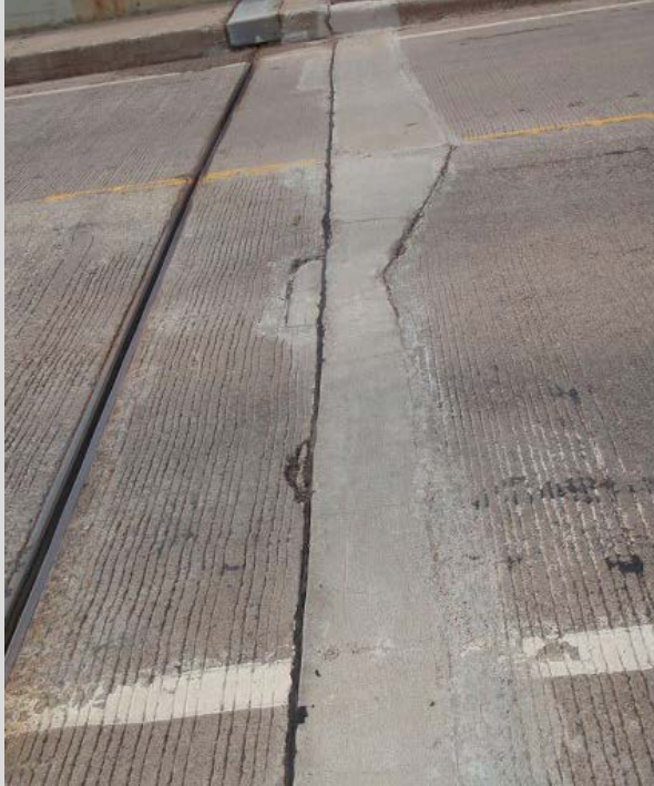
Condition State 2 Concrete patch on a concrete approach panel (along the end block joint)
