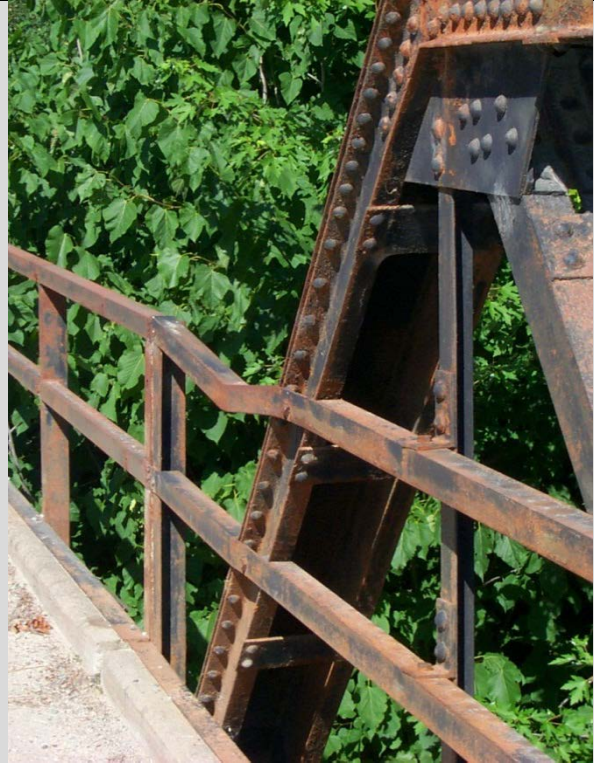
Condition State 3 Steel angle railing bent significantly
