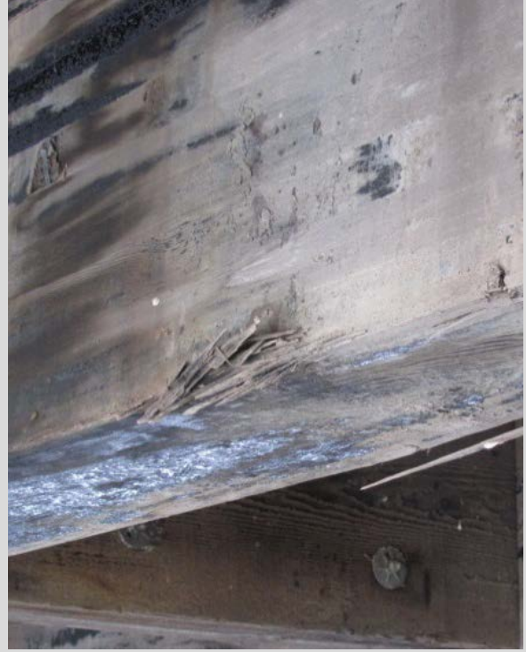
Condition State 2 Minor impact damage on a Glulam timber beam
