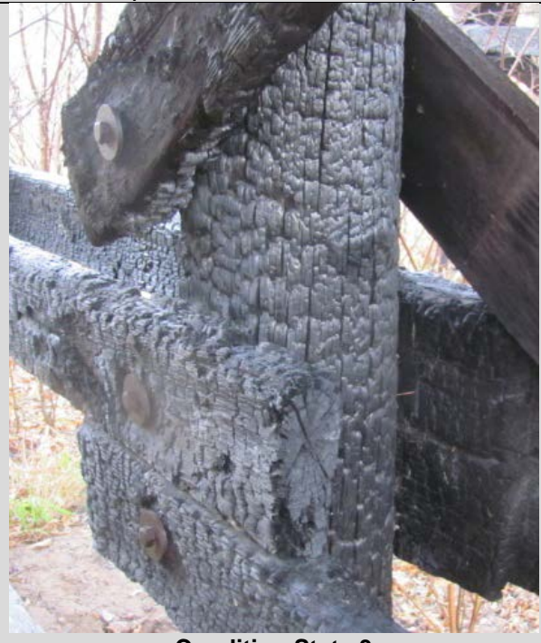
Condition State 3 Fire damage on a timber piling (section loss between 10% and 40%)
