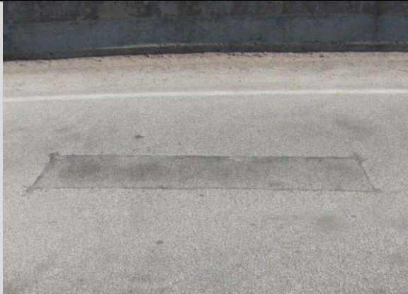
Condition State 2 Repair patch on a chip seal overlay
