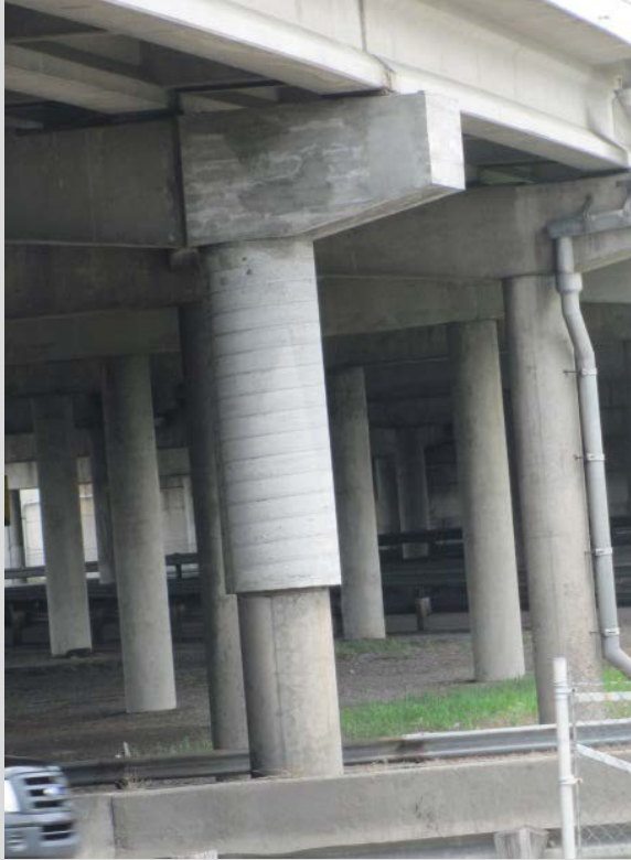
Condition State 2 Repair on a reinforced concrete column & pier cap
