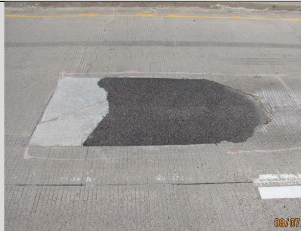
Condition State 3 Bituminous patch on low slump concrete overlay
