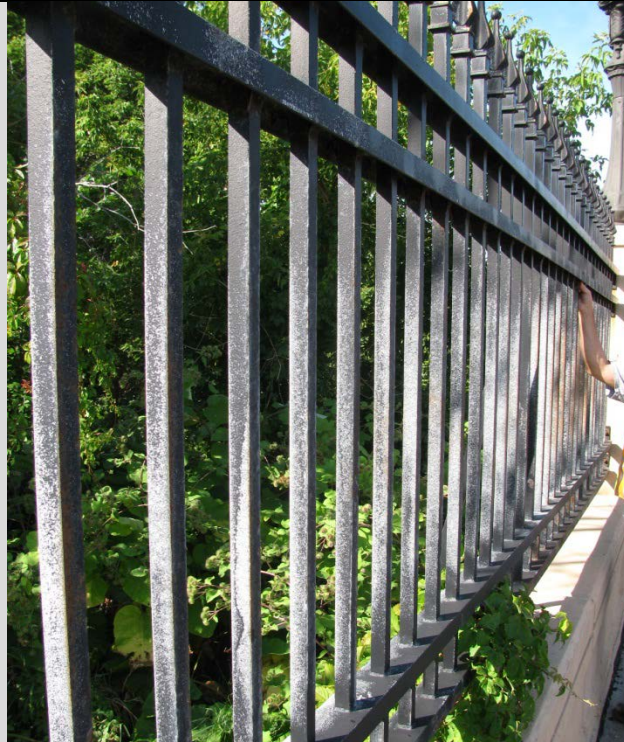
Condition State 3 Finish paint coat (Duplex system) has extensive failure, the galvanized layer below remains intact
