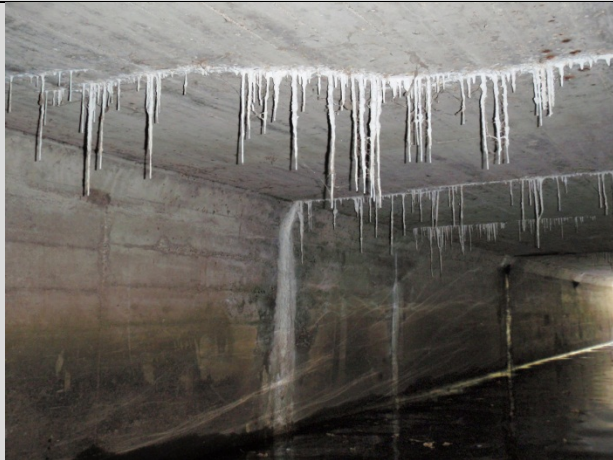
Condition State 3 Heavy leaching on a cast-in-place (CIP) concrete box culvert
