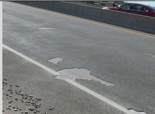
Condition State 4 Chip seal overlay missing
