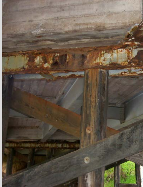
Condition State 3 Flaking rust and pack rust on a steel channel pier cap
