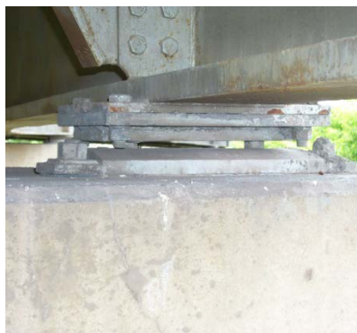
Uplift (gap) on a curved plate fixed bearing
