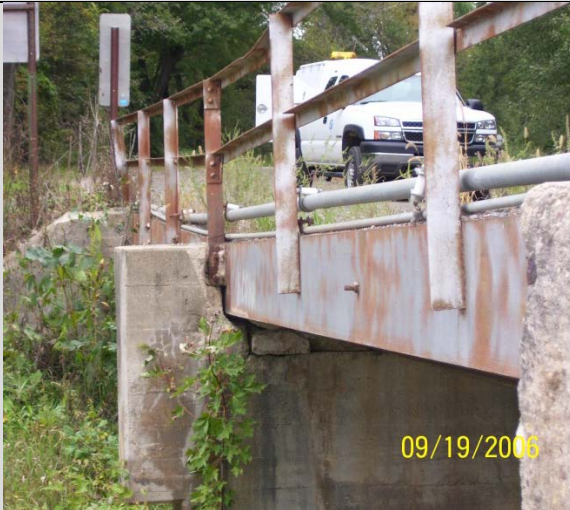
Condition State 3 Significant settlement of a concrete approach pier
