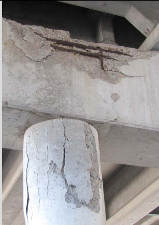
Condition State 4 Severe spalling on a reinforced concrete pier cap
