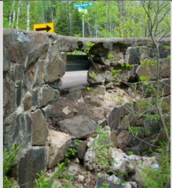
Condition State 4 Severe impact damage on a masonry railing
