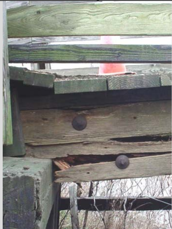
Condition State 4 Severe crushing (failure) of a sawn timber beam
