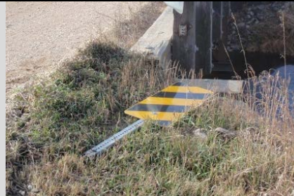
Condition State 3 Type III Object Marker on ground
