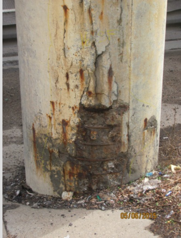
Condition State 3 Spalling (exposed & corroded reinforcement) on a reinforced concrete column
