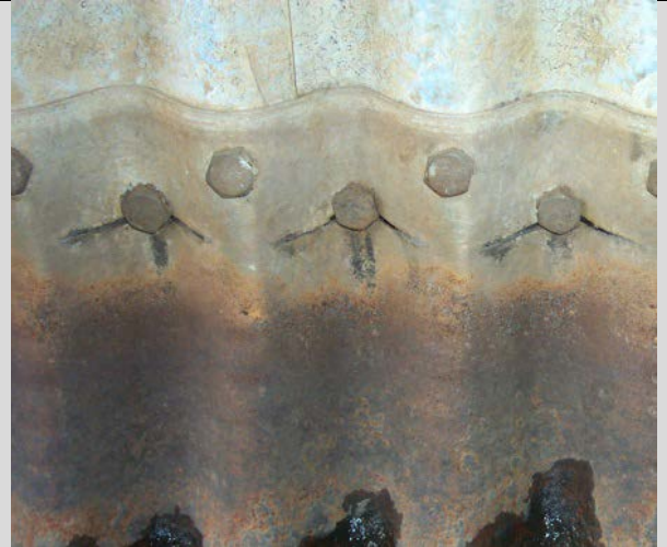
Condition State 3 Cracking along a bolted seam
