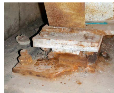
Corroded (possibly frozen) sliding plate bearing
