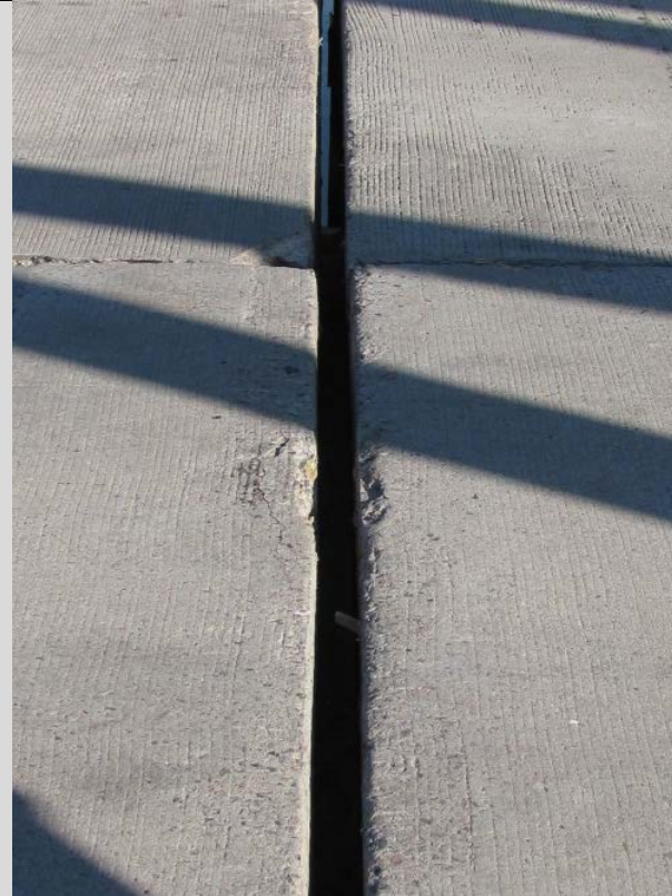
Condition State 2 Minor spalling along an open deck joint
