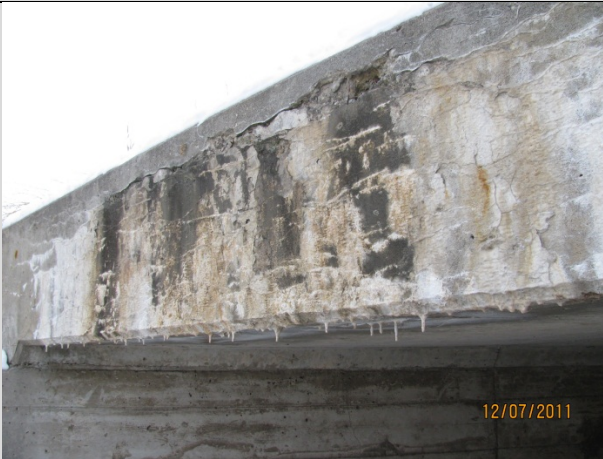
Condition State 3 Extensive leaching cracks on the headwall of a cast-in-place (CIP) concrete box culvert
