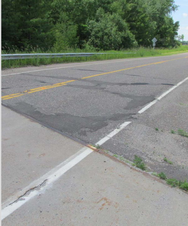
Condition State 2 Moderate deterioration on a bituminous approach roadway (cracking and patching)
