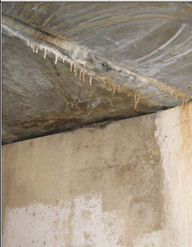
Condition State 3 Cracking with significant leaching on the underside of a prestressed voided slab panel
