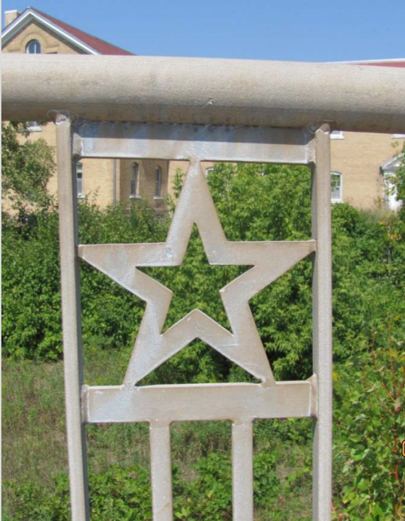
Condition State 2 Galvanized coating on bridge rail is faded
