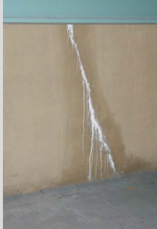
Condition State 2 Leaching crack in the parapet wall on a reinforced concrete abutment
