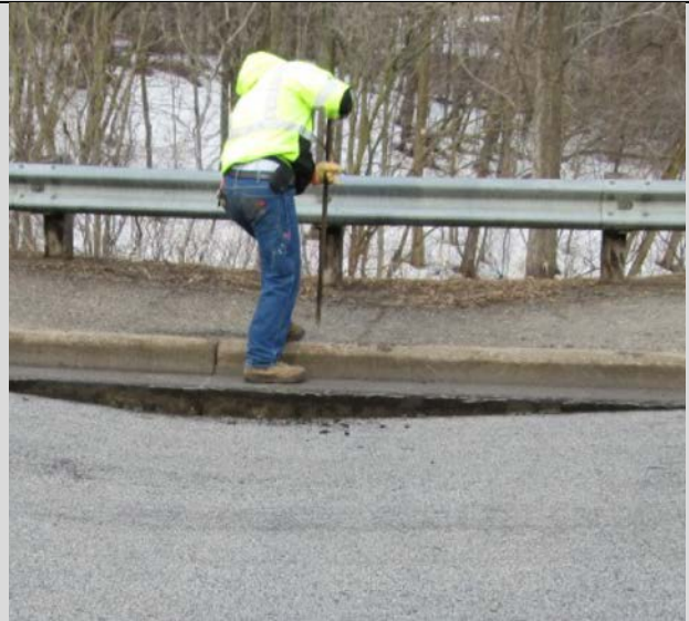
Condition State 4 Severe settlement of a bituminous roadway above a failed steel culvert
