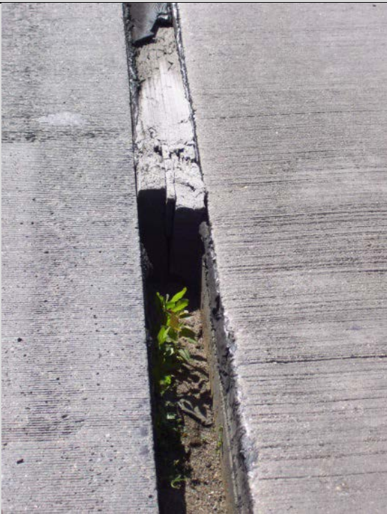
Condition State 3 Poured seal and foam filler missing from an approach relief joint
