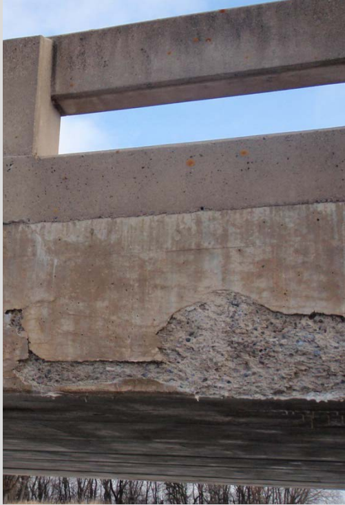
Condition State 3 Scale/spall on the fascia of a prestressed concrete box beam
