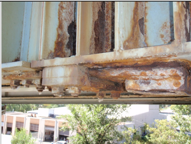
Condition State 3 Lateral guide below hinge bearing is severely corroded (possibly restricting movement)
