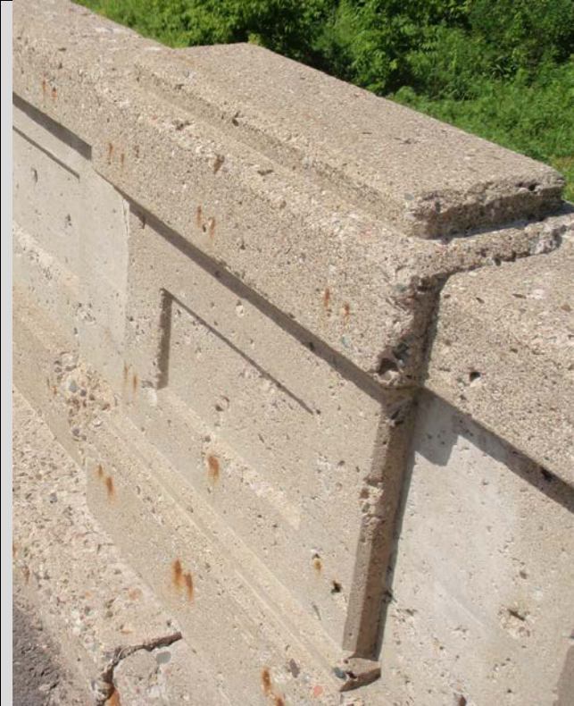
Condition State 2 Scale and pot-outs on a solid concrete parapet railing
