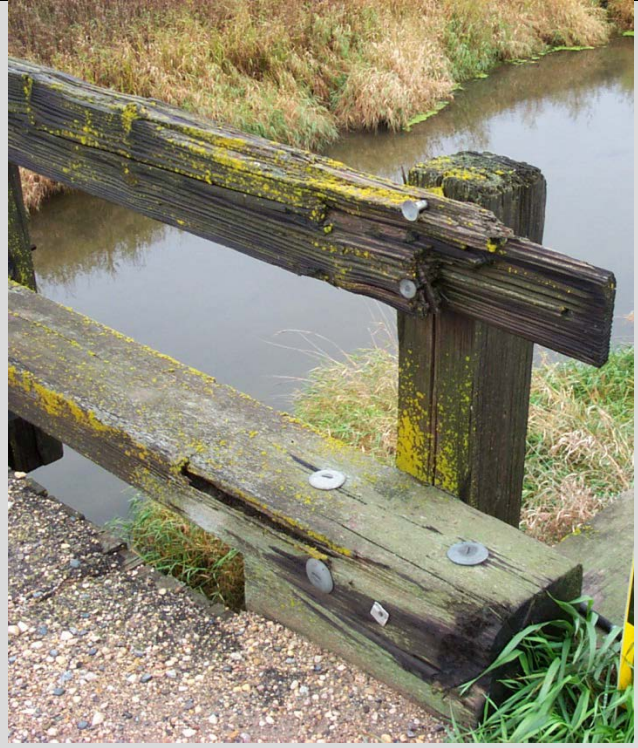
Condition State 3 Significant decay on a timber rail beam
