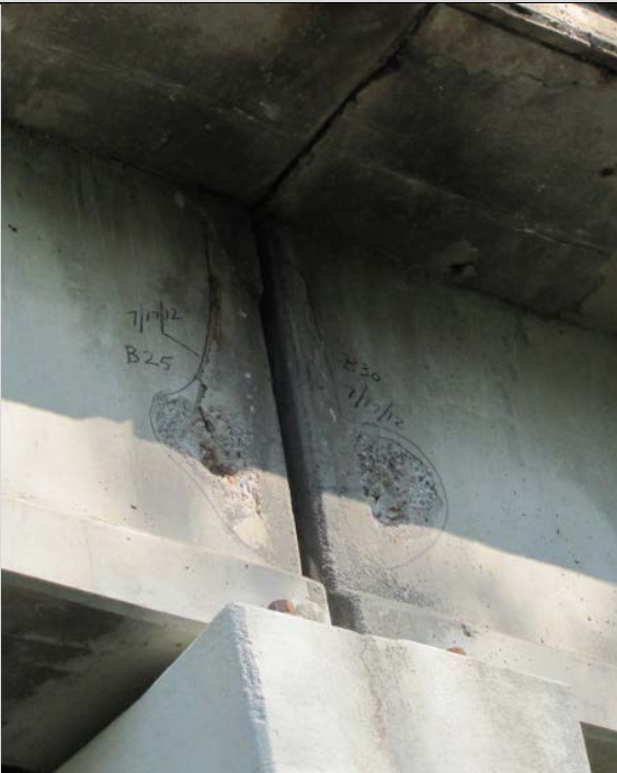
Condition State 3 Spalling on the web of a prestressed concrete beam
