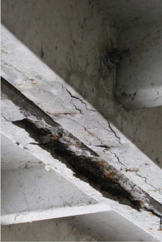
Condition State 3 Spalling on a precast concrete channel beam
