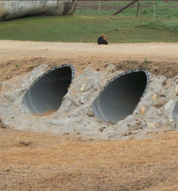
Condition State 1 Plastic pipe culvert (DWPE - Double Wall Polyethylene)
