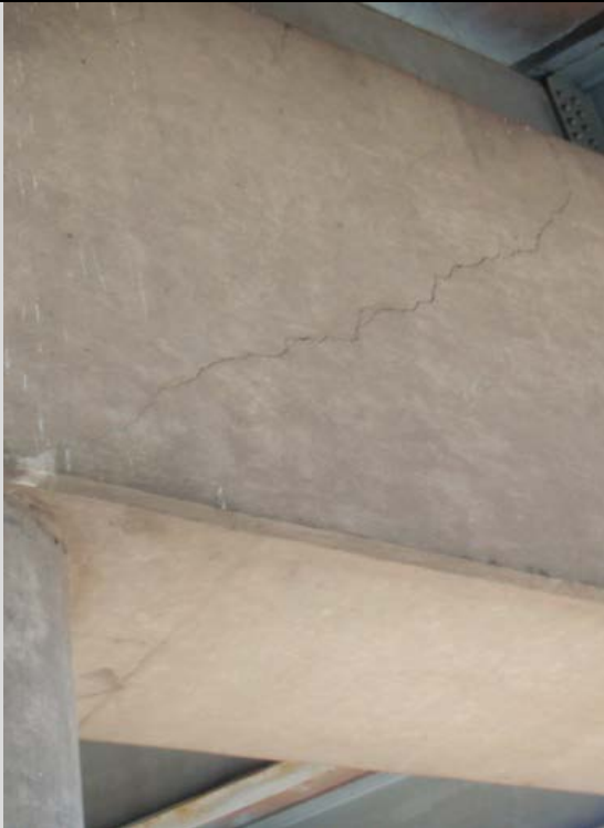
Condition State 3 Shear crack in a reinforced concrete pier cap
