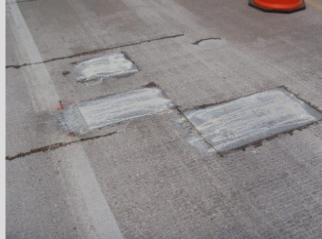
Condition State 2 Sound concrete patches on a bare concrete deck
