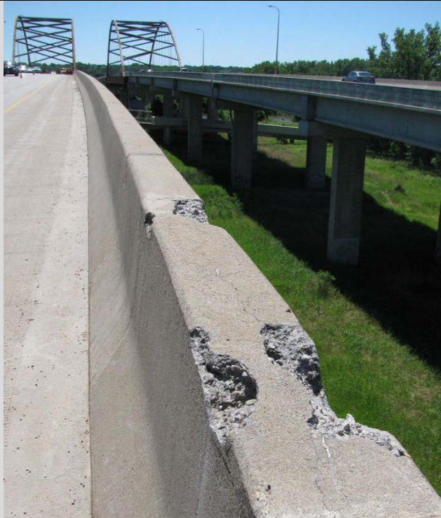
Condition State 3 Spalling along the top of a concrete J-rail
