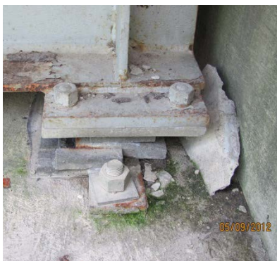
Sliding plate bearing near the design limits of expansion
