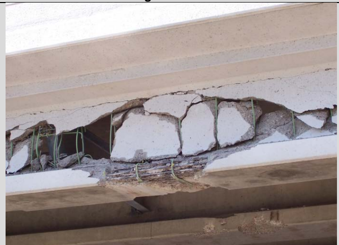
Condition State 4 Prestressed beam severely damaged by high load impact
