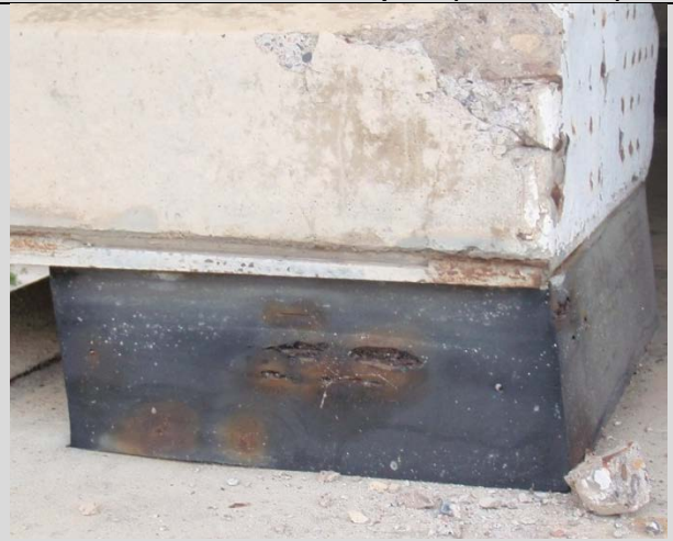
Condition State 3 Pad covering torn, internal plates rusting
