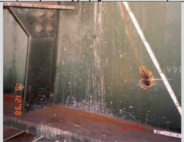
Condition State 4 Fatigue crack has propagated through beam web
