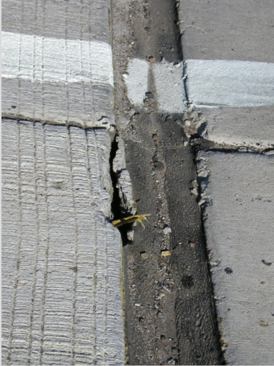
Condition State 2 Minor spalling along an approach relief joint
