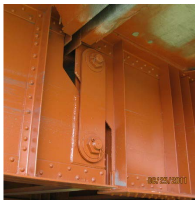
Pin & Hanger Assembly on a Riveted Steel Girder Bridge
