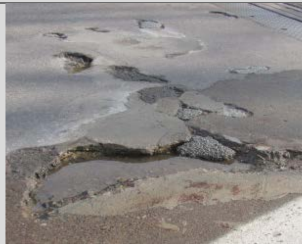
Condition State 4 Spalling 2" or deeper on a bare concrete deck
