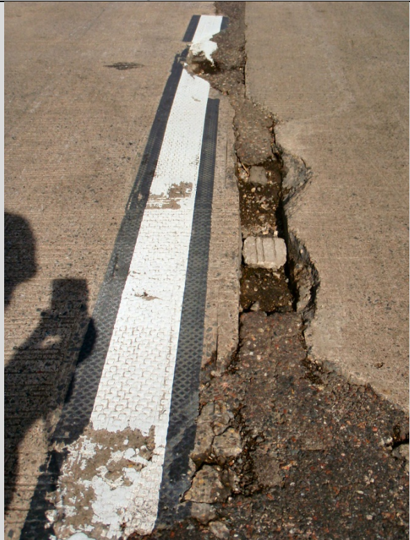
Condition State 4 Severe spall along centerline of a concrete approach panel
