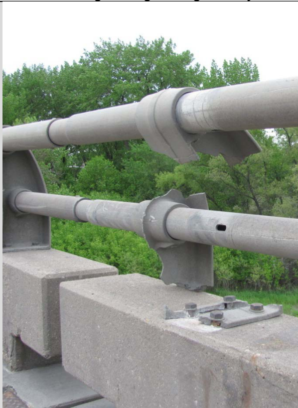
Condition State 4 Aluminum post severely damaged
