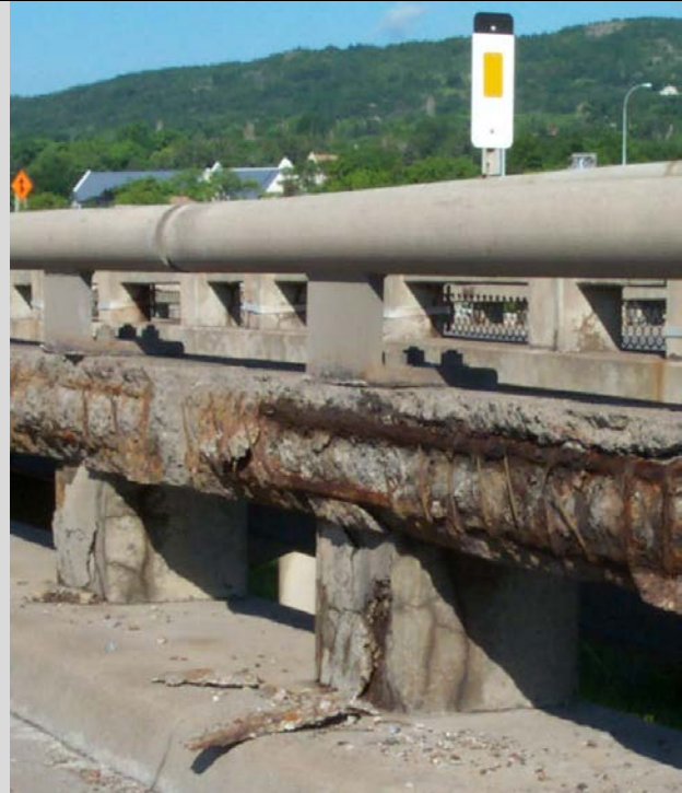
Condition State 4 Severe spalling on the concrete rail base of a combination railing
