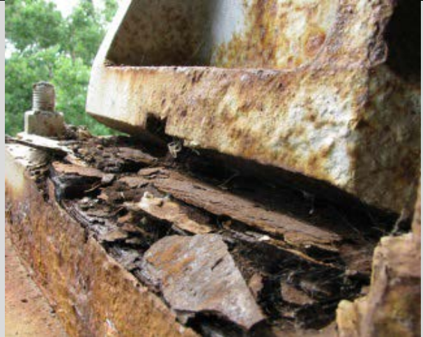
Condition State 3 Flaking rust and debris below rocker bearing (restriction of movement)
