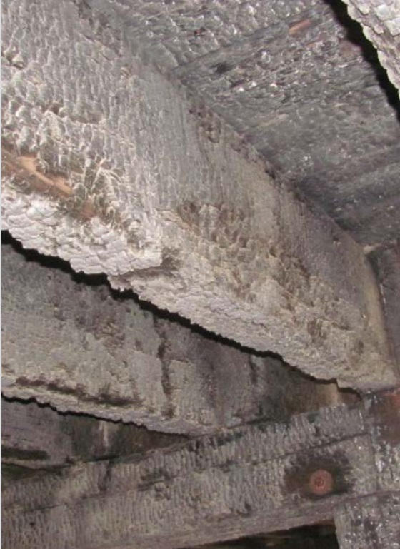
Condition State 3 Fire damage on a sawn timber beam
