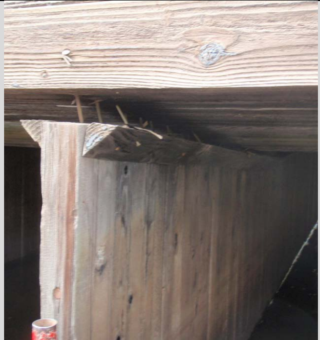
Condition State 4 Separation (connection failure) between wall and ceiling on a timber box culvert
