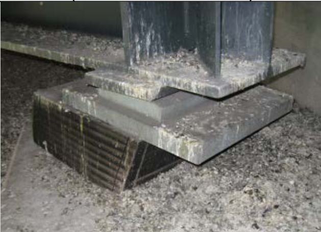
Condition State 4 Pad has moved from beneath the curved pintle plate (nearly fallen off)
