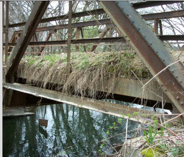
Condition State 4 Excessive gravel on a deck (more than 6" depth)
