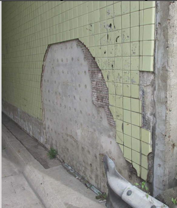
Condition State 3 Tiles missing from a tunnel wall
