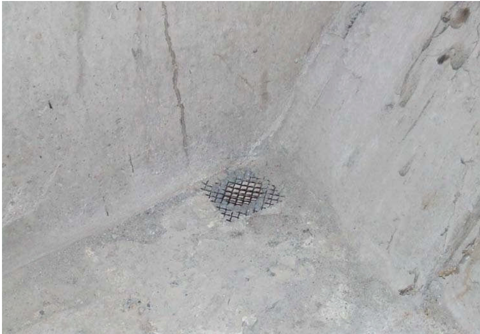
Figure 9.11.37 Concrete Box Girder Drain Hole with Screen
