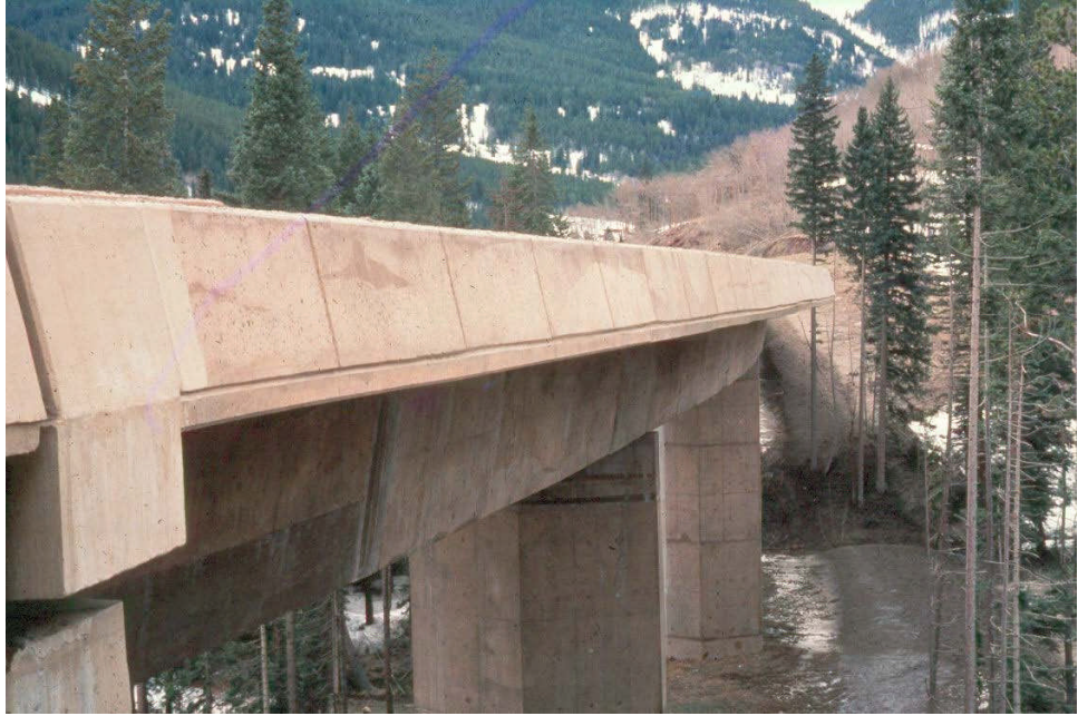
Figure 9.11.4 Cast-in-place Concrete Box Girder Bridge
