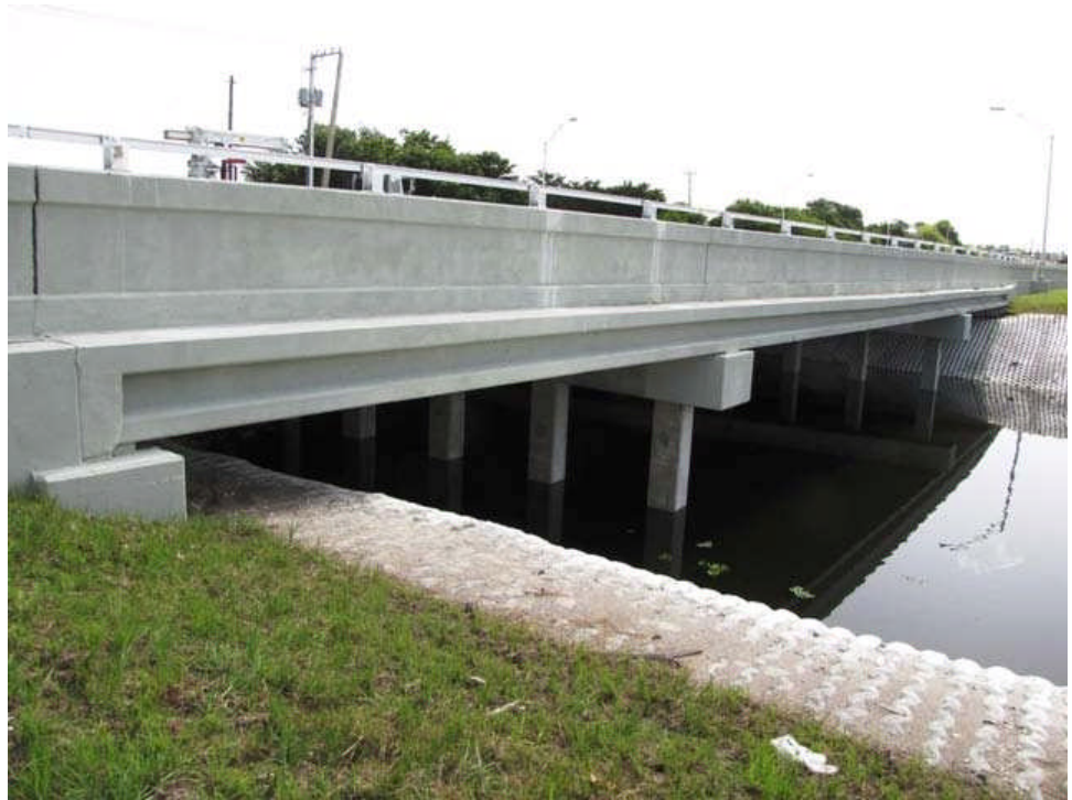
Figure 9.7.3 Poutre Dalle Precast Slab Bridge
