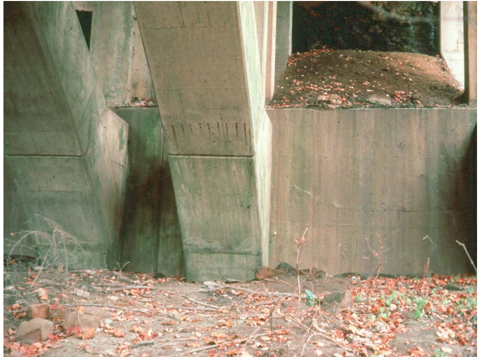
Figure 9.5.12 Arch/Skewback Interface
