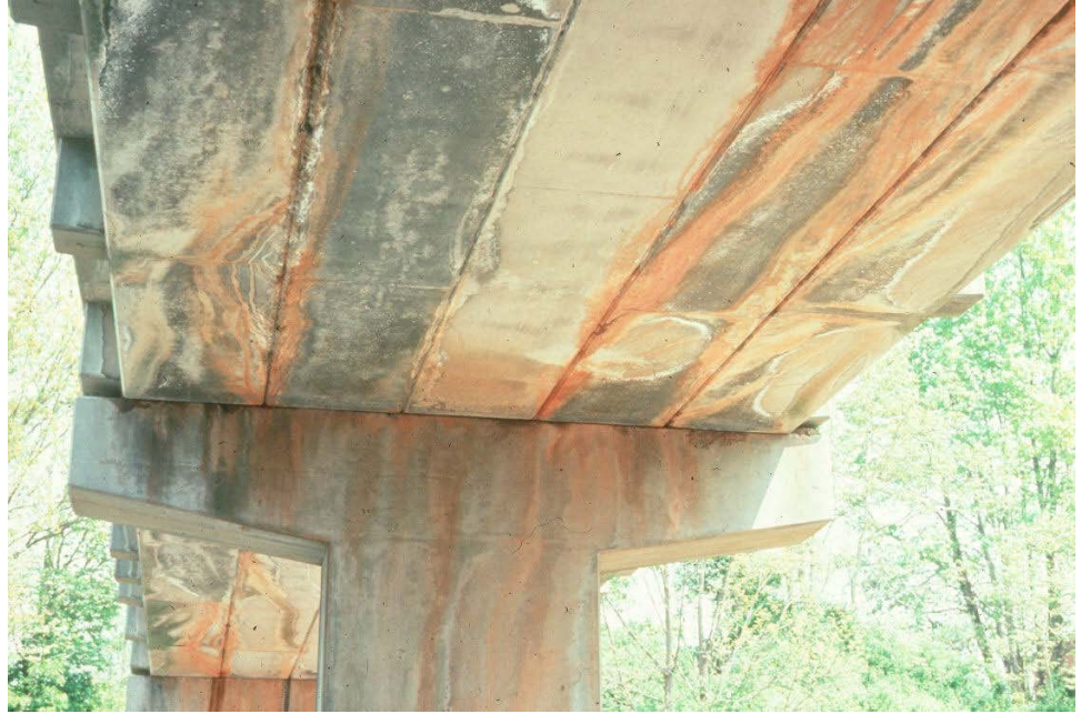
Figure 9.10.17 Joint Leakage and Rust Stain
