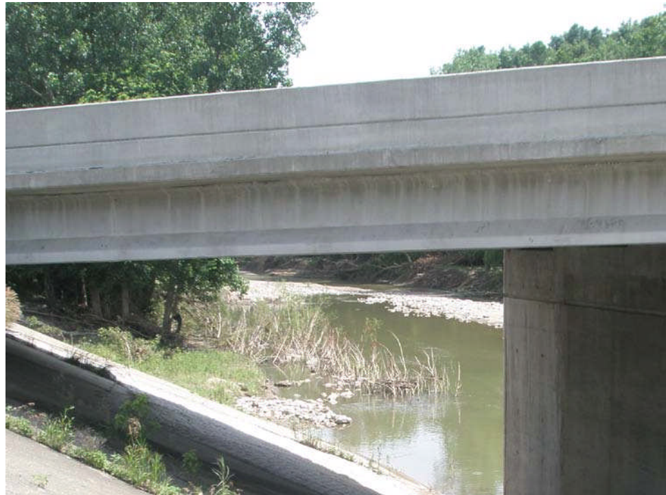
Figure 9.9.3 AASHTO Prestressed I-beam Bridge
