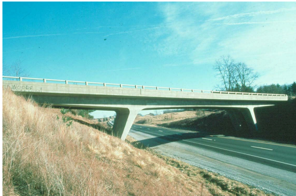
Figure 9.6.3 Three Span Concrete K-frame Bridge
