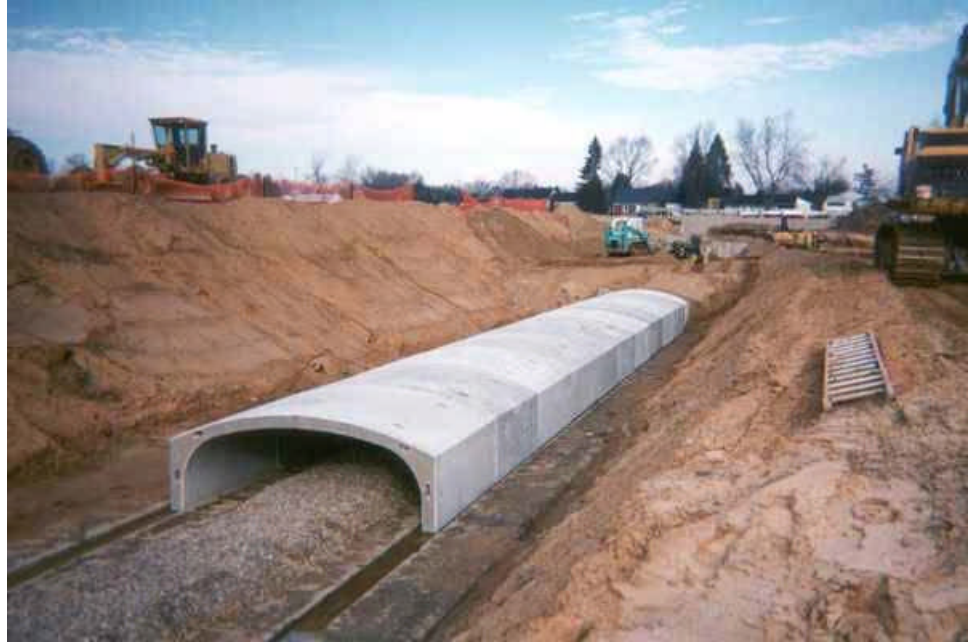
Figure 9.5.4 Precast Concrete Arch with Integral Vertical Legs
