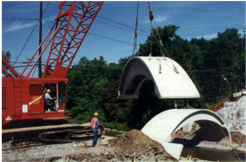
Figure 9.5.5 Precast Segmental Concrete Arch
