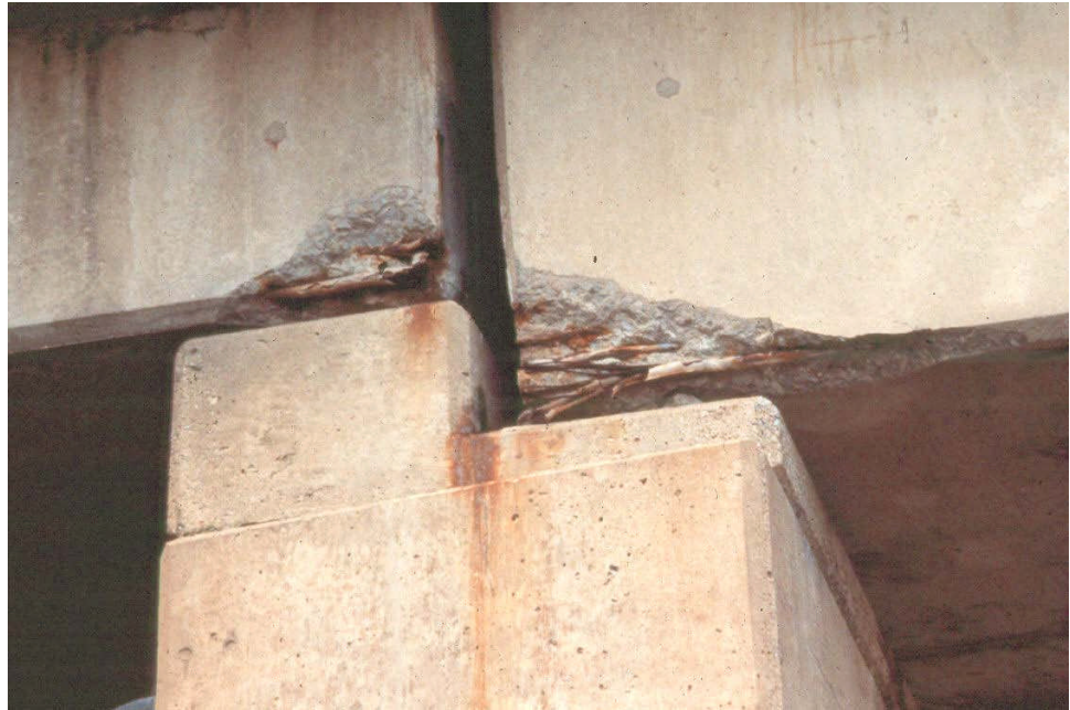
Figure 9.10.11 Spalled Beam Ends with Exposed Prestressing Reinforcement
