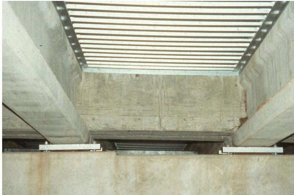
Figure 9.9.18 Concrete End Diaphragm
