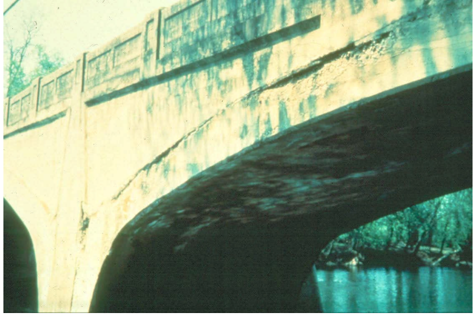
Figure 9.5.15 Deteriorated Arch/Spandrel Wall Interface
