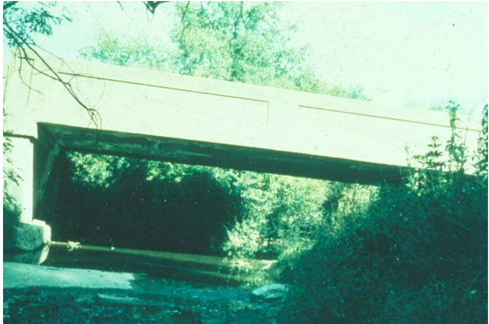
Figure 9.3.4 Concrete Through Two-Girder Elevation View
