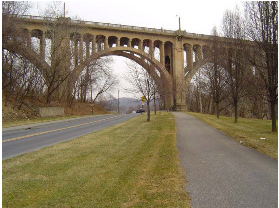
Figure 9.5.1 Open Spandrel Arch Bridge
