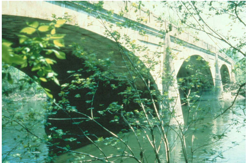
Figure 9.5.2 Multi-span Closed Spandrel Arch Bridge
