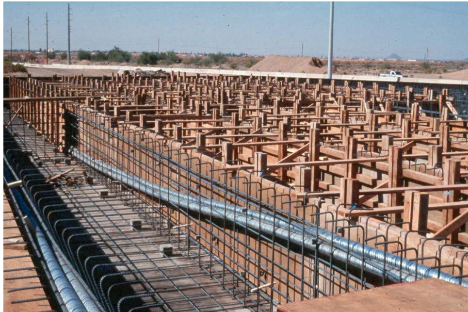
Figure 9.11.41 Post-tensioning Tendon Duct
