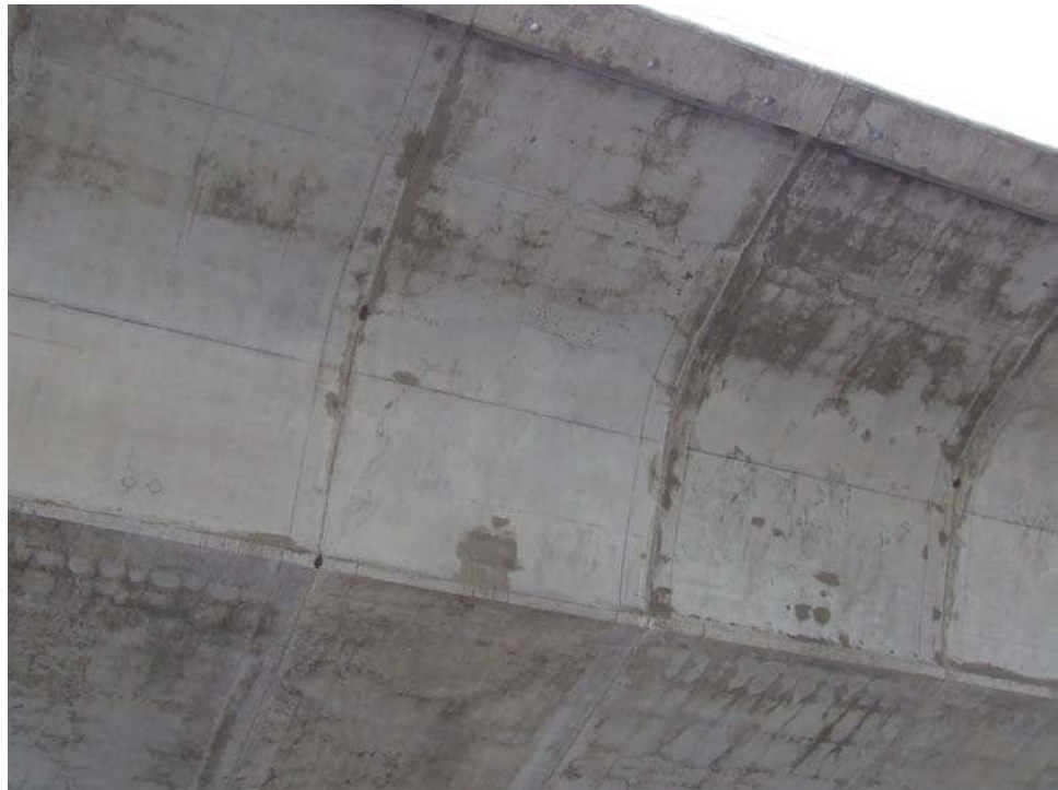
Figure 9.11.15 Close-up of Box Girder Segments
