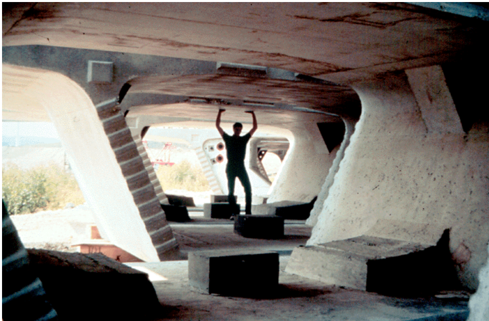
Figure 9.11.16 Box Girder Segment
