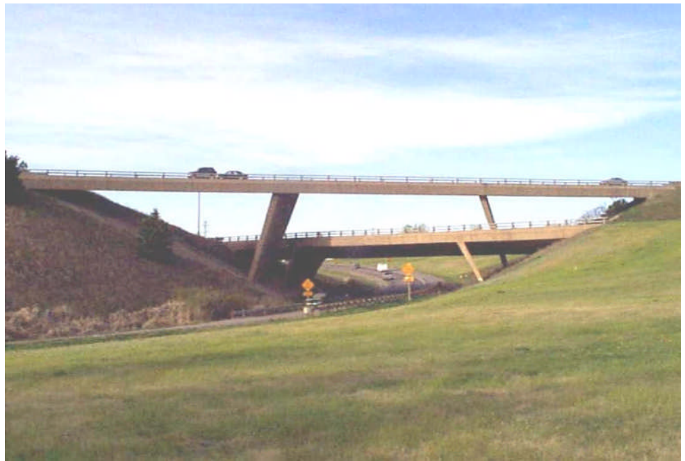
Figure 9.6.1 Multi-span Concrete Rigid Frame Bridges
