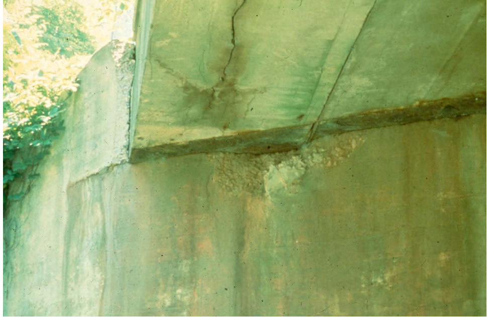
Figure 9.10.13 Longitudinal Cracks in Bottom Flange of Beam
