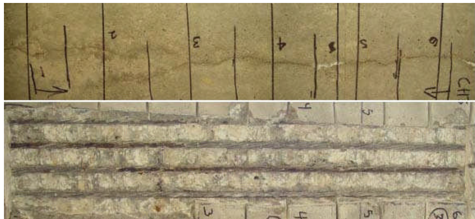
Figure 9.10.26 Longitudinal Cracks (Top) and Corresponding Corroded Prestressing Strands after Concrete Removed (Bottom)
