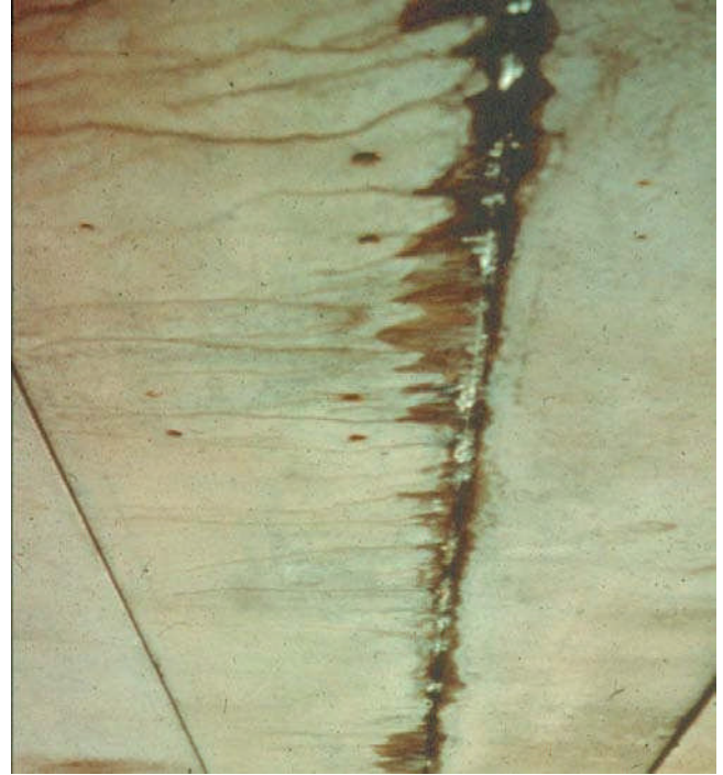
Figure 9.7.6 Leaking Joint between Adjacent Slab Units
