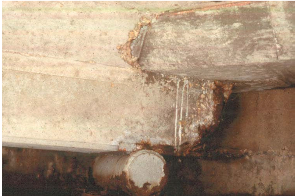
Figure 9.2.9 Spalled Tee Beam End
