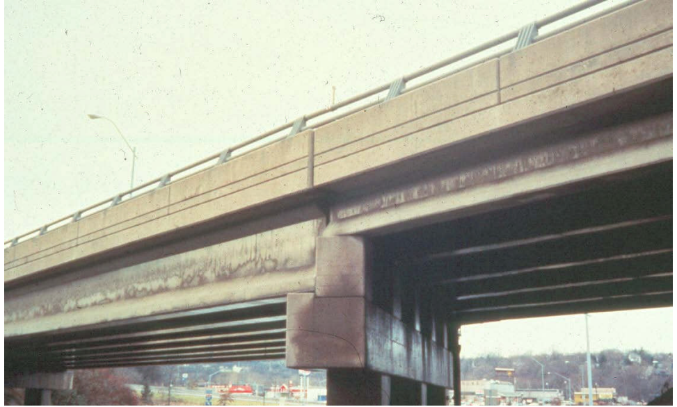
Figure 9.9.19 Leakage of Water at Joint between Spans
