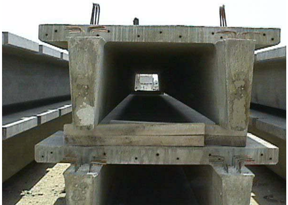
Figure 9.8.1 Typical Prestressed Double Tee Beam
