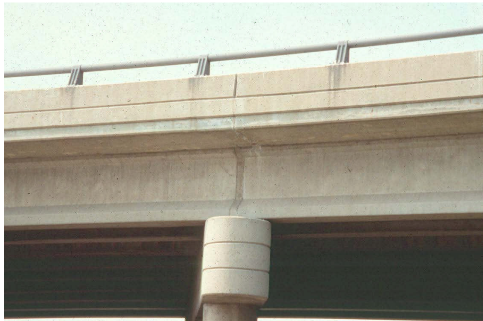
Figure 9.9.9 Continuous Prestressed I-Beam Bridge
