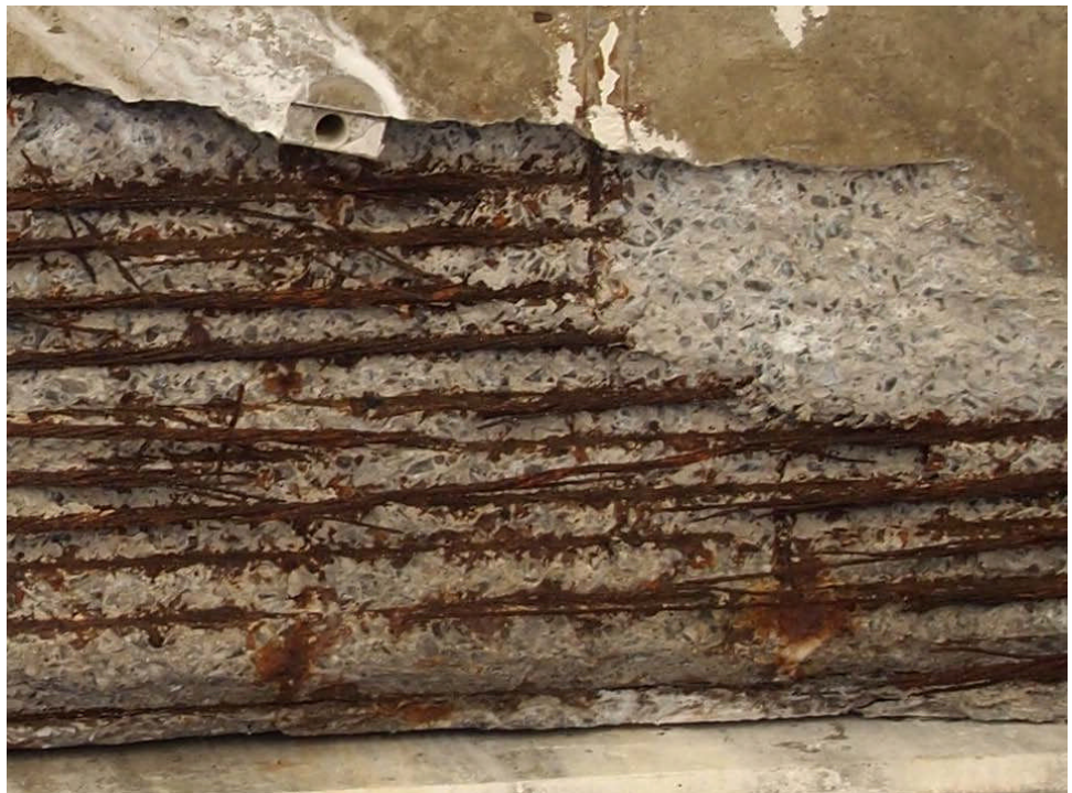
Figure 9.10.16 Close-up of Failed Strands due to Corrosion
