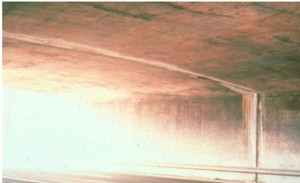
Figure 9.6.14 Longitudinal Joint Between Slab Frames
