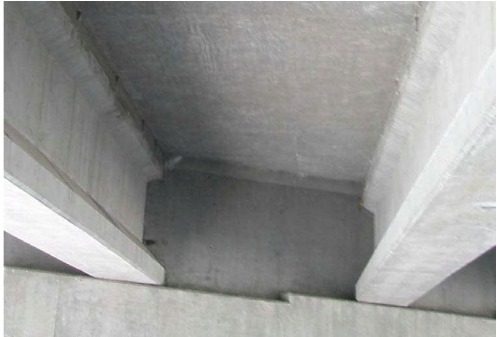
Figure 9.9.15 Bearing Area of a Typical Prestressed I-beam
