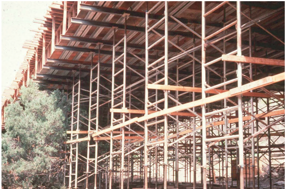
Figure 9.11.5 High Level Casting Formwork on Falsework
