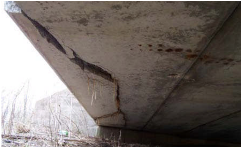
Figure 9.10.18 Close-up of Box Beam Collision Damage
