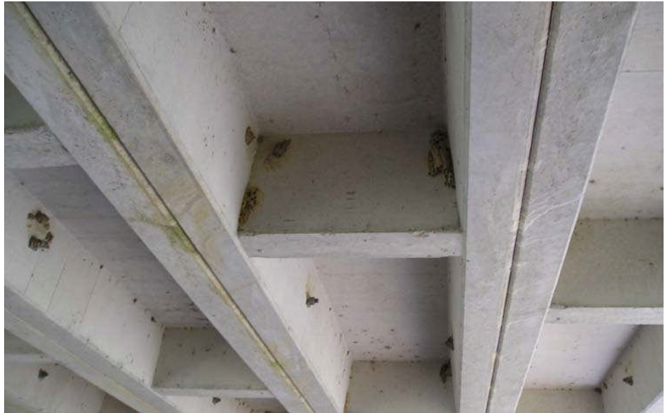
Figure 9.4.1 Underside View of Precast Channel Beam Bridge
