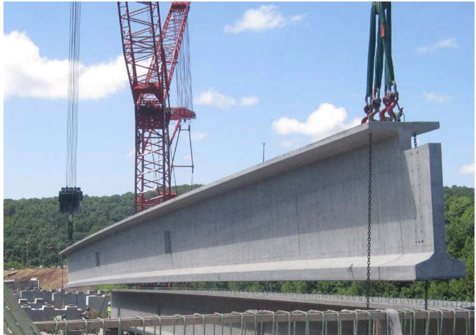
Figure 9.9.5 Placement of an AASHTO-PCI Bulb-Tee Beam
