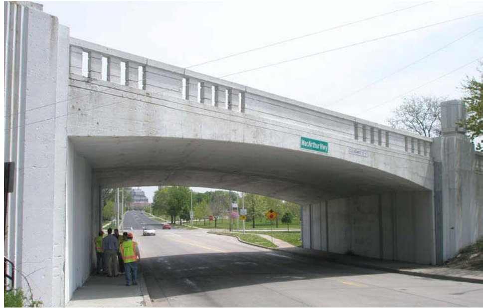
Figure 9.6.2 Single-span Rectangular Concrete Rigid Frame Bridge
