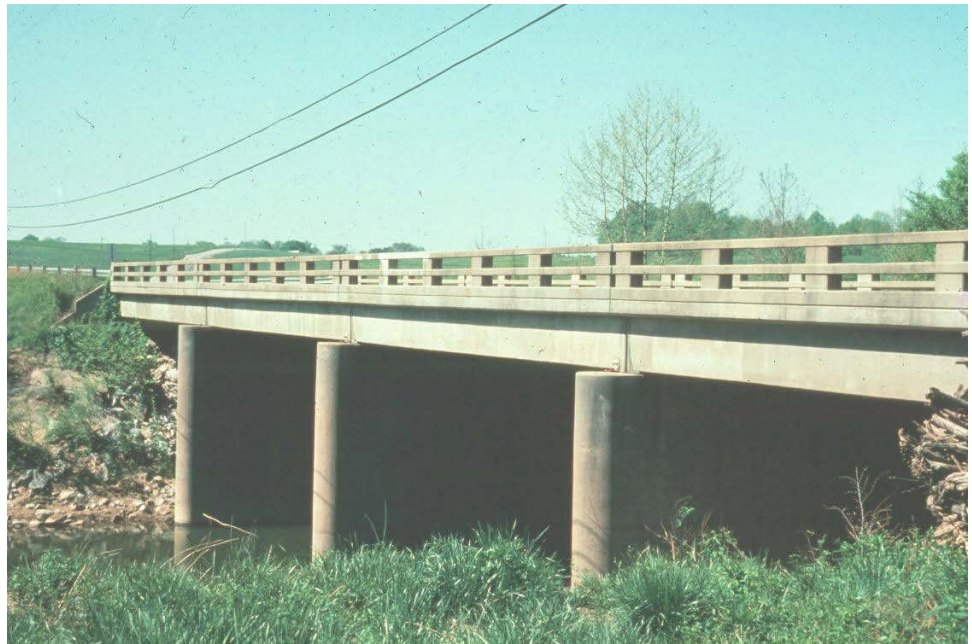
Figure 9.10.1 Typical Box Beam Bridge
