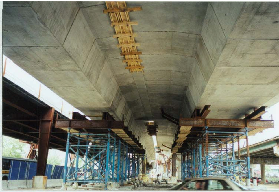
Figure 9.11.13 Adjacent Single Cell Boxes with Closure Pour
