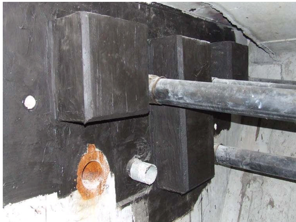
Figure 9.11.48 Box Girder Interior Diaphragm and Post-Tensioning Ducts
