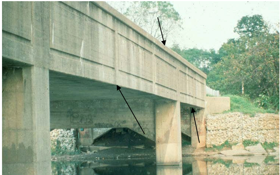
Figure 9.3.7 Typical Elevation View of a Through Two-Girder Bridge with Tension Zones Indicated
