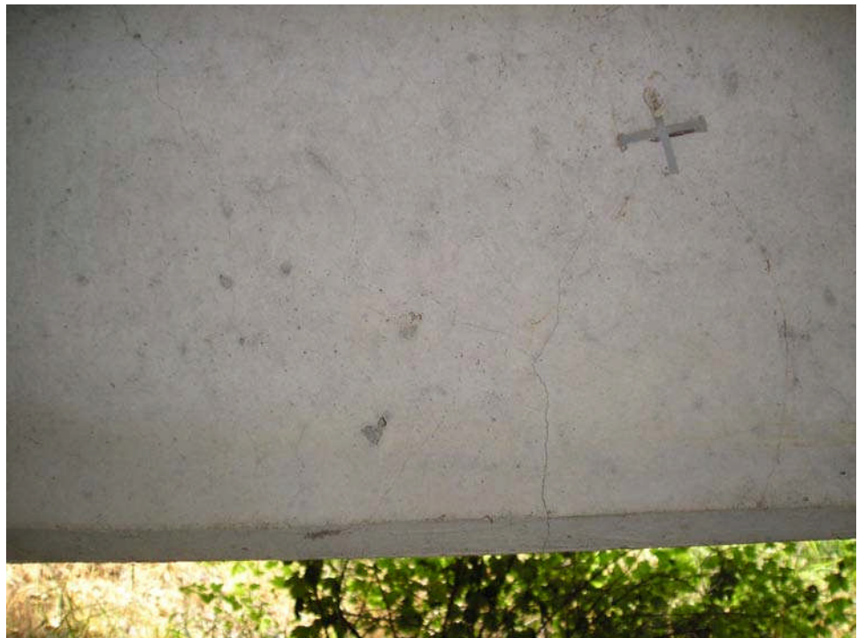
Figure 9.2.13 Flexure Cracks on a Tee Beam Stem
