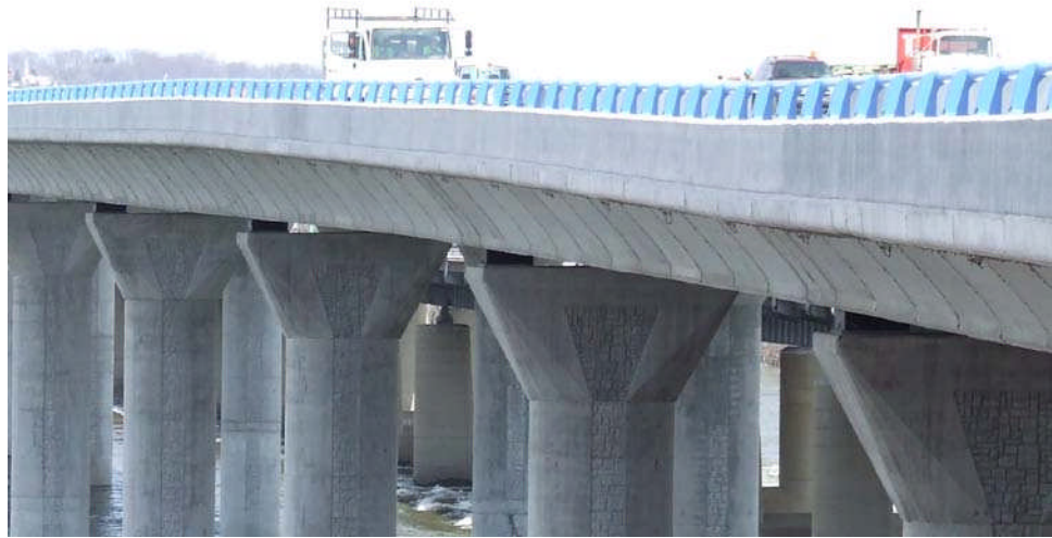
Figure 9.11.14 Segmental Concrete Bridge
