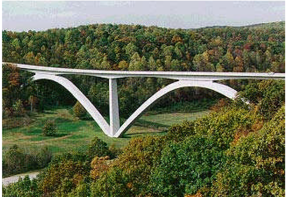
Figure 9.5.6 Precast Post-tensioned Concrete Arch without Spandrel Columns
