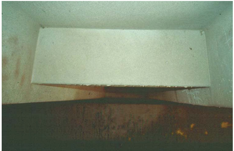
Figure 9.4.9 Close-up of Intermediate Diaphragm
