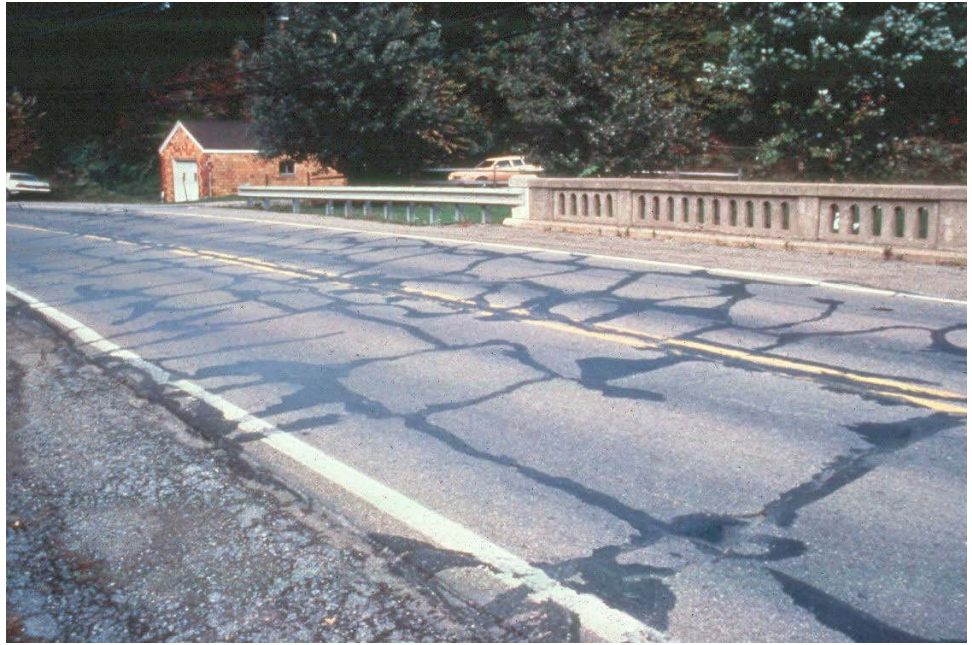
Figure 9.2.17 Asphalt Covered Tee Beam Deck
