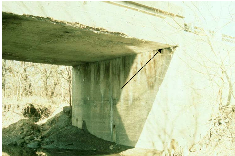
Figure 9.3.6 Bearing Area of a Through Two-Girder Bridge
