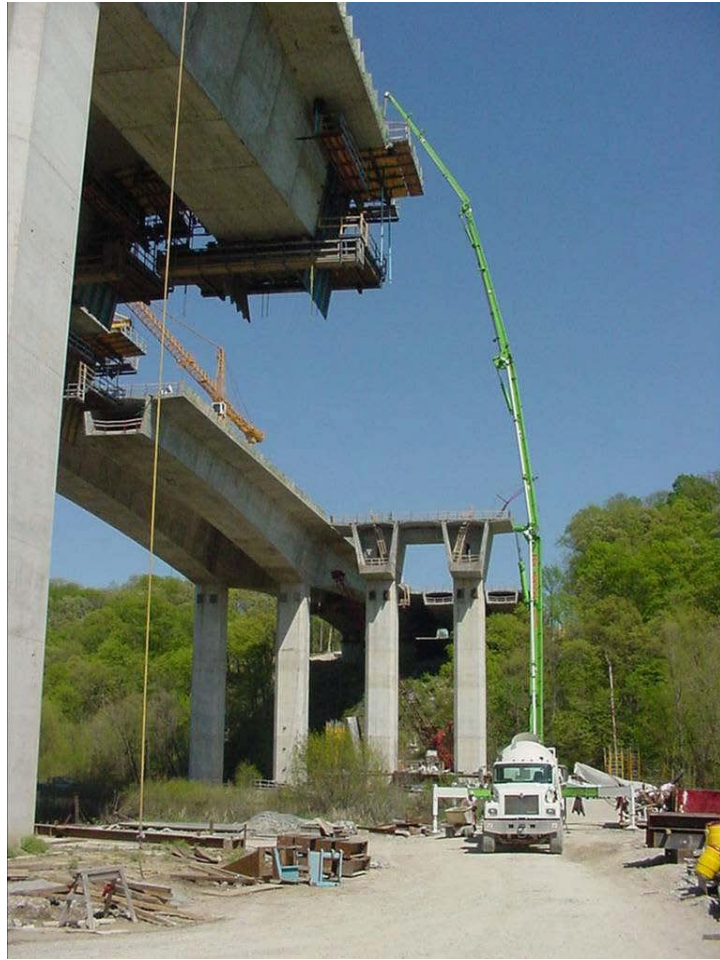
Figure 9.11.25 Progressive Placement Construction
