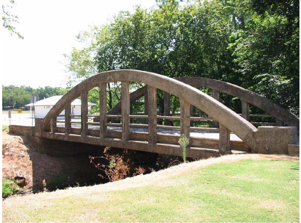
Figure 9.5.3 Concrete Through Arch Bridge
