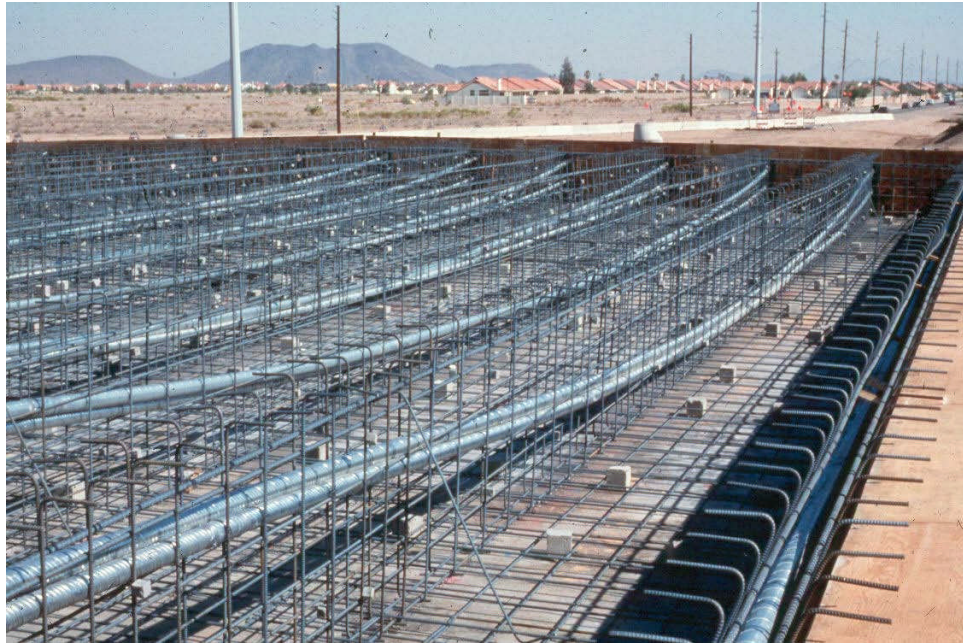
Figure 9.11.6 At-grade Formwork with Post-tensioning Ducts
