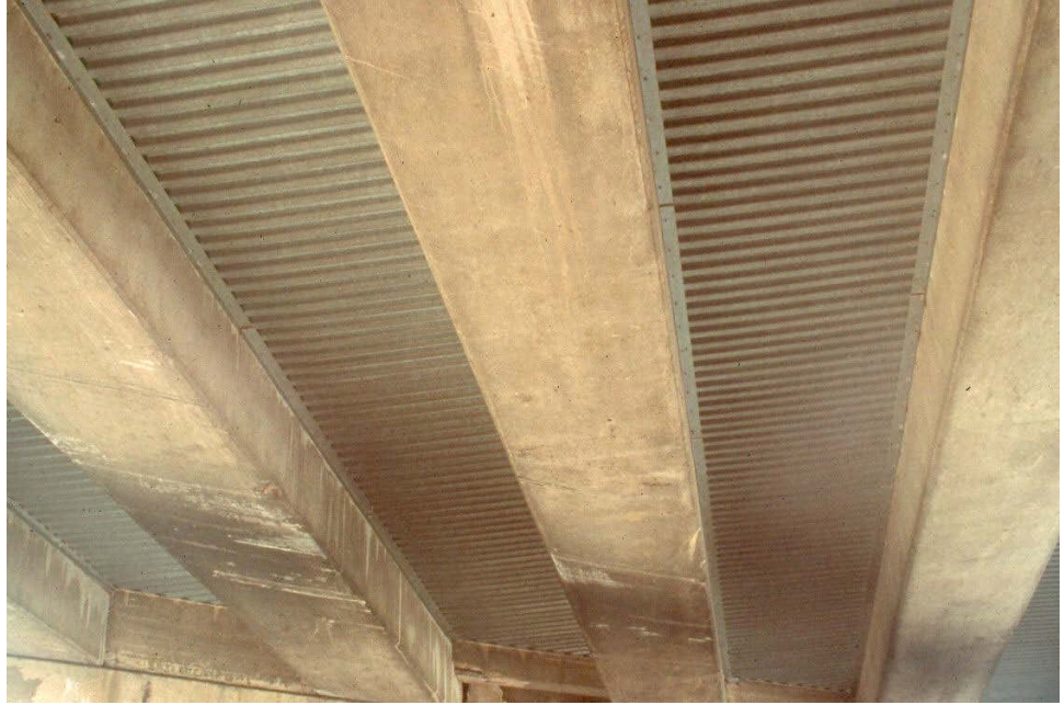
Figure 9.10.7 Underside of a Typical Spread Box Beam
