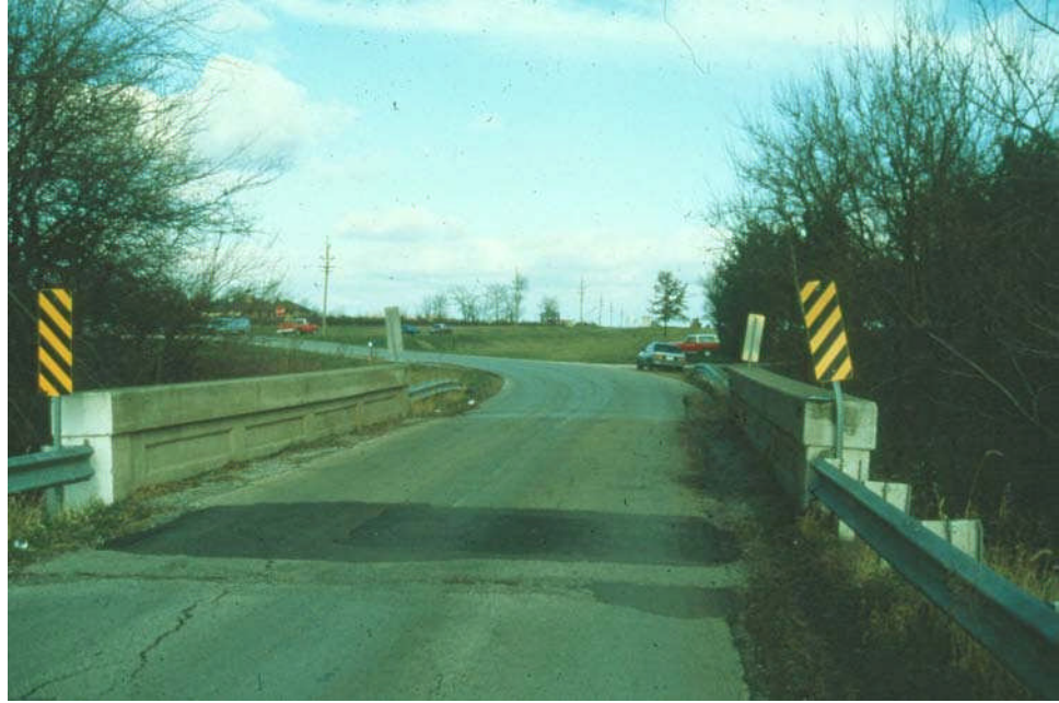
Figure 9.3.2 Concrete Through Two-Girder Bridge
