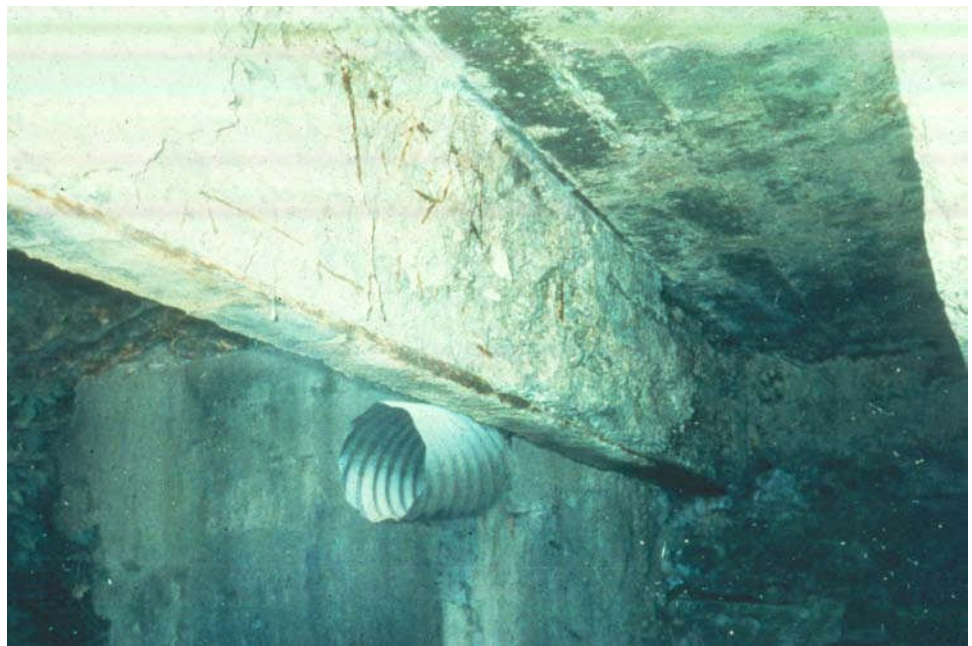
Figure 9.2.5 Concrete Encased Steel I-beam
