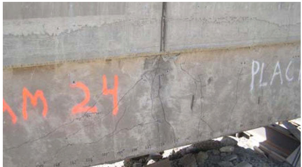
Figure 9.10.28 Cracking Near Barrier Joints
