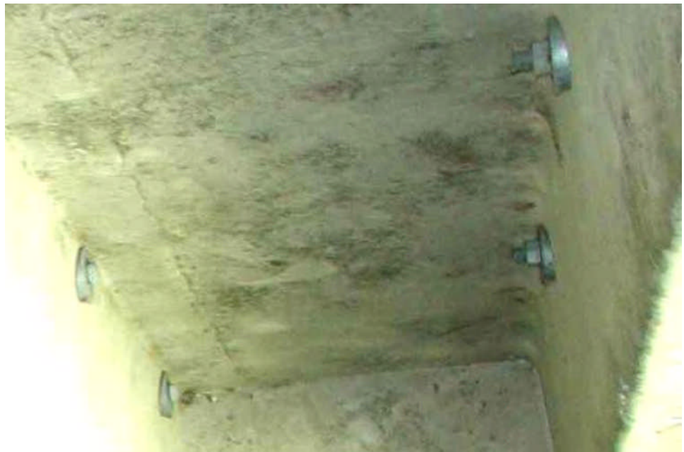
Figure 9.4.7 Stem Tie-Bolts
