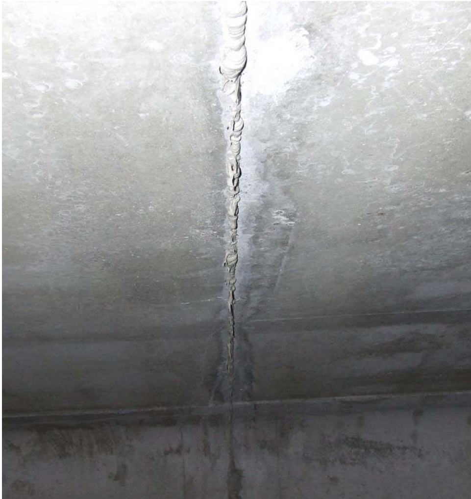
Figure 9.11.46 Close-up View of Box Girder Joint
