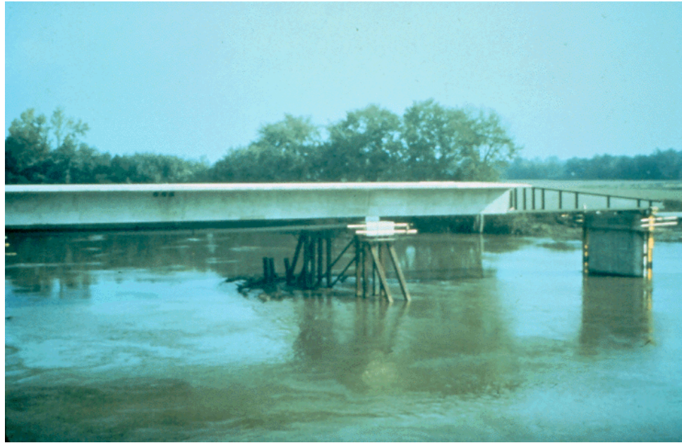
Figure 9.11.27 Incremental Launching Overview (Note Temporary Pile Bent)
