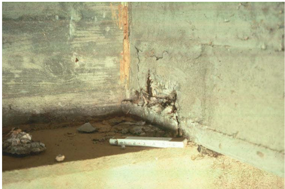
Figure 9.2.10 Deteriorated Tee Beam Bearing Area
