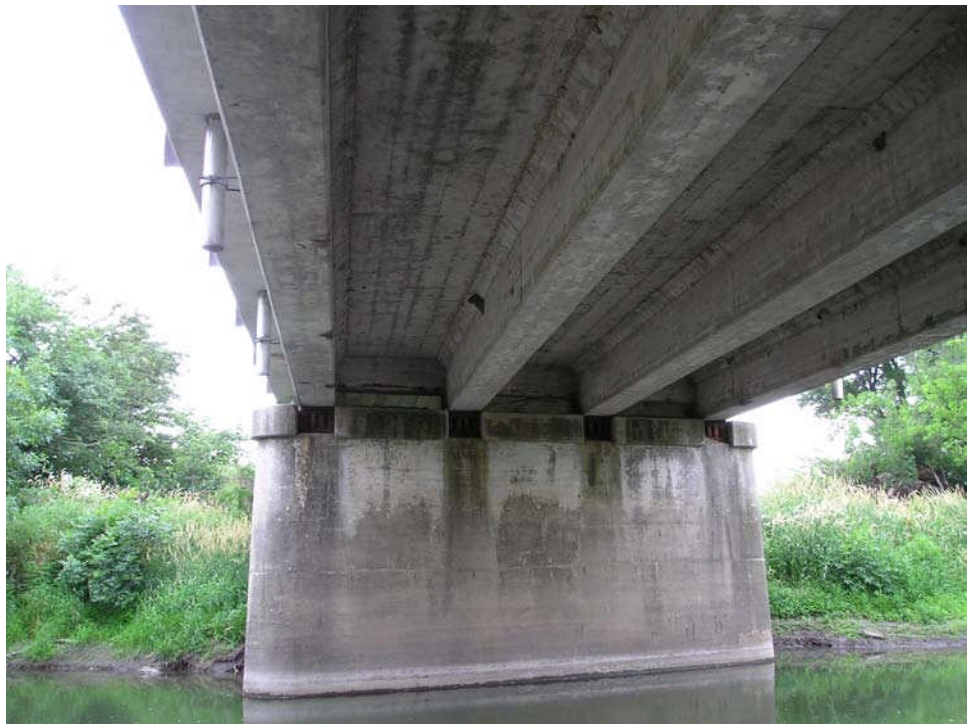
Figure 9.2.1 Simple Span Tee Beam Bridge
