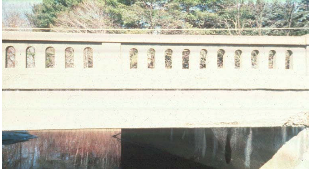
Figure 9.2.19 Deteriorated Tee Beam End Due to Drainage
