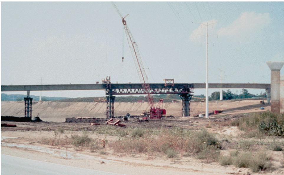
Figure 9.11.23 Span-by-span Construction (with Erection Truss)
