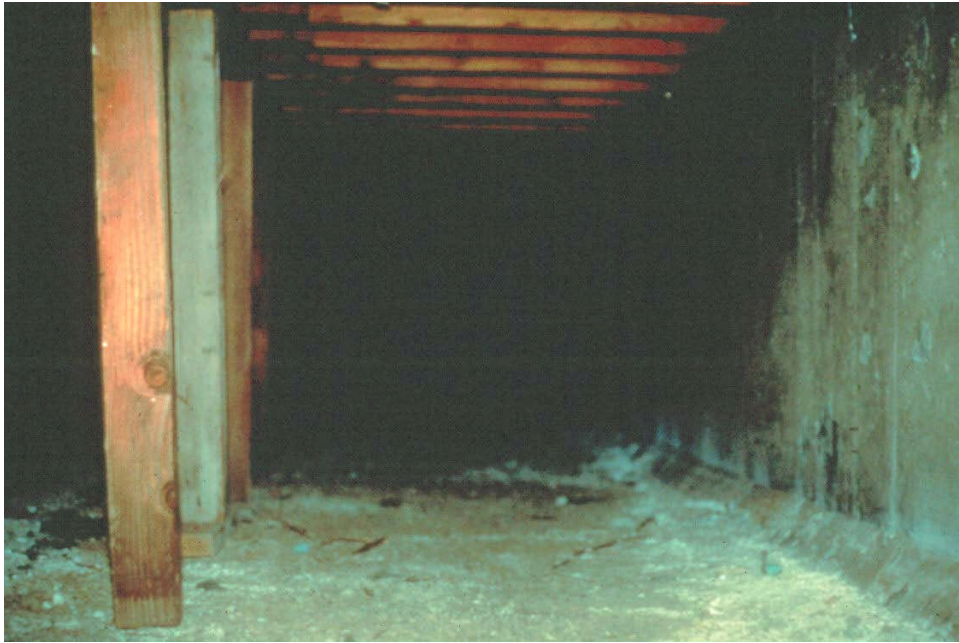
Figure 9.11.42 Interior Formwork Left in Place
