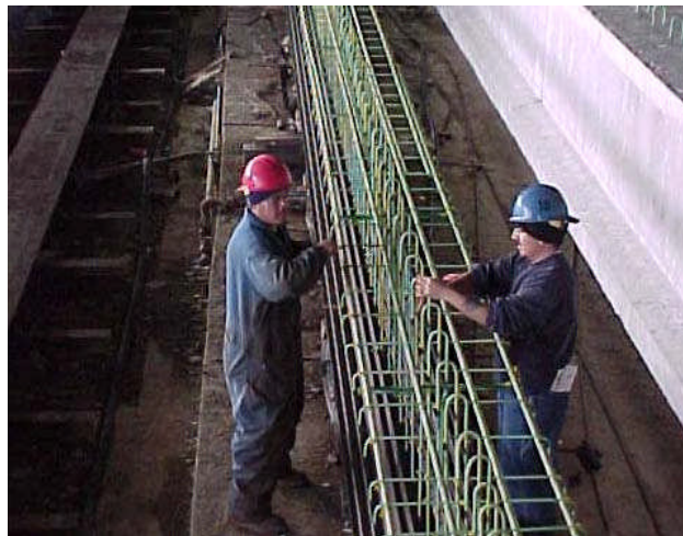
Figure 9.9.11 Extended Stirrups to Obtain Composite Action
