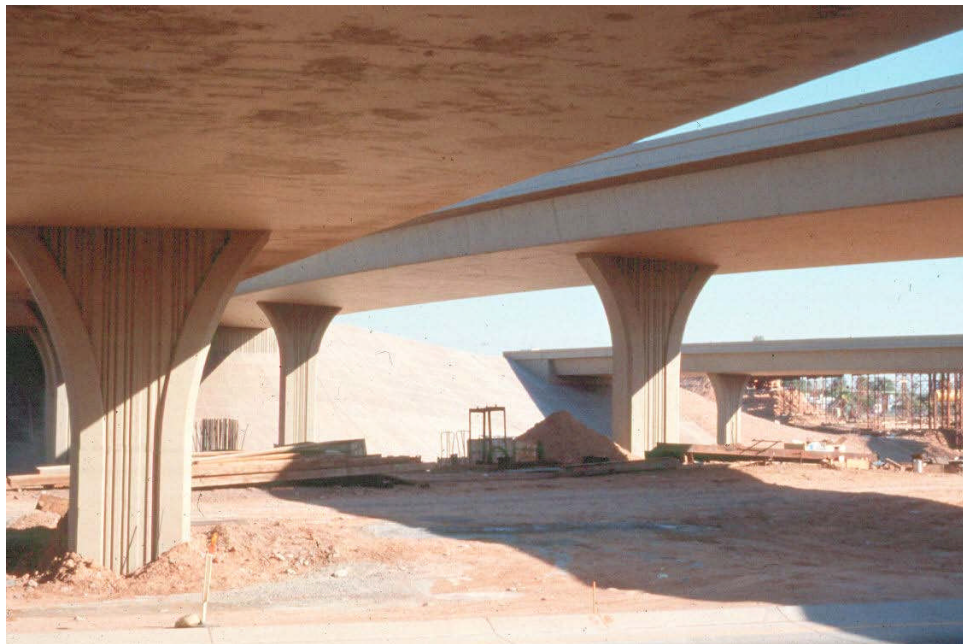
Figure 9.11.7 At-grade Casting – After Supporting Earth Removed
