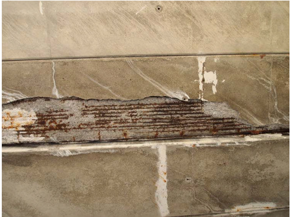
Figure 9.10.15 Spall and Exposed/Corroded Reinforcement
