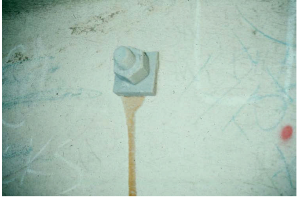
Figure 9.4.8 Close-up of Stem Tie-Bolt (Epoxy Resin)
