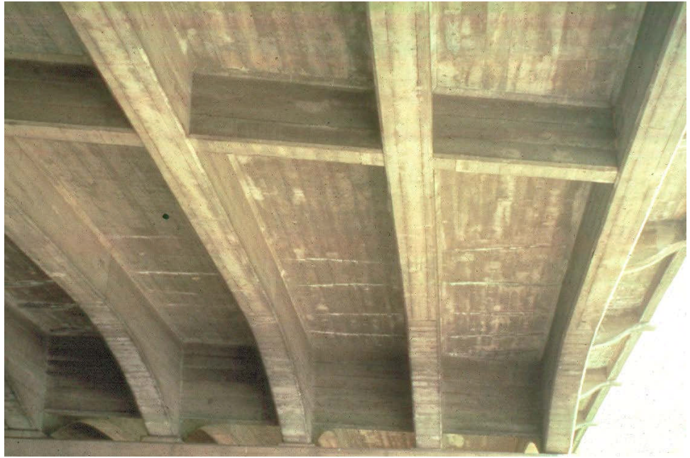
Figure 9.2.14 Flexure Cracks in Tee Beam Flange/Deck
