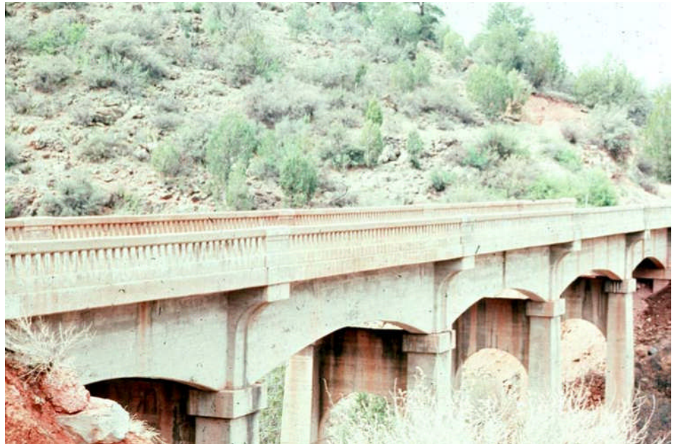
Figure 9.3.1 Concrete Deck Two-Girder Bridge
