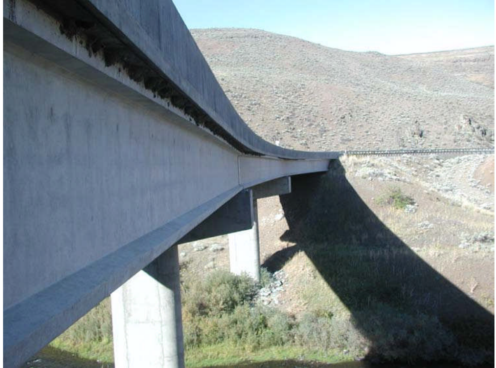
Figure 9.9.1 Prestressed I-beam Superstructure
