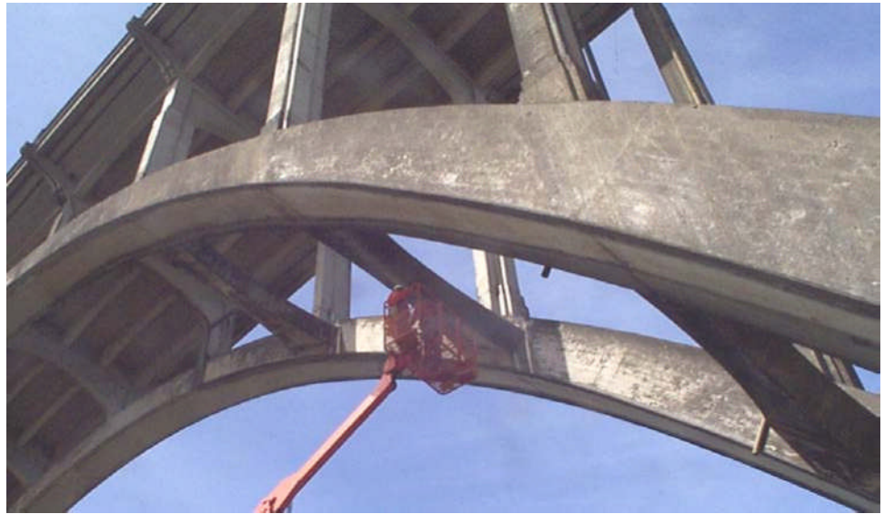
Figure 9.5.17 Inspection and Documentation of Arch Strut Deficiencies
