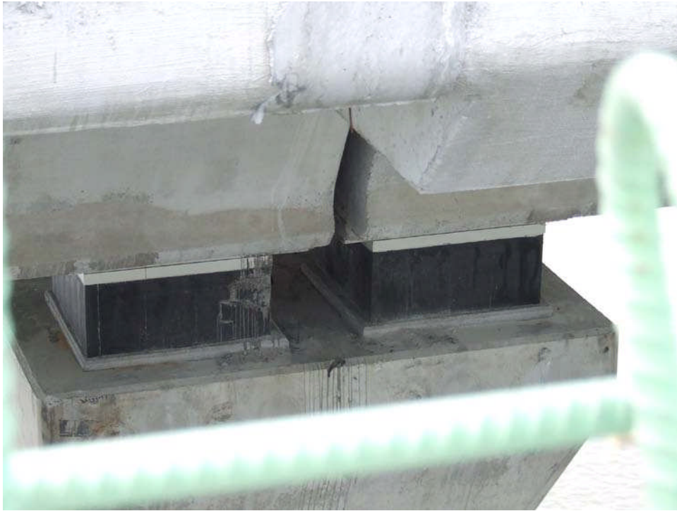
Figure 9.11.44 Segmental Box Girder Bearings at Intermediate Pier
