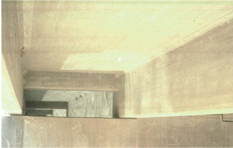
Figure 9.2.6 Tee Beam Primary and Secondary Members
