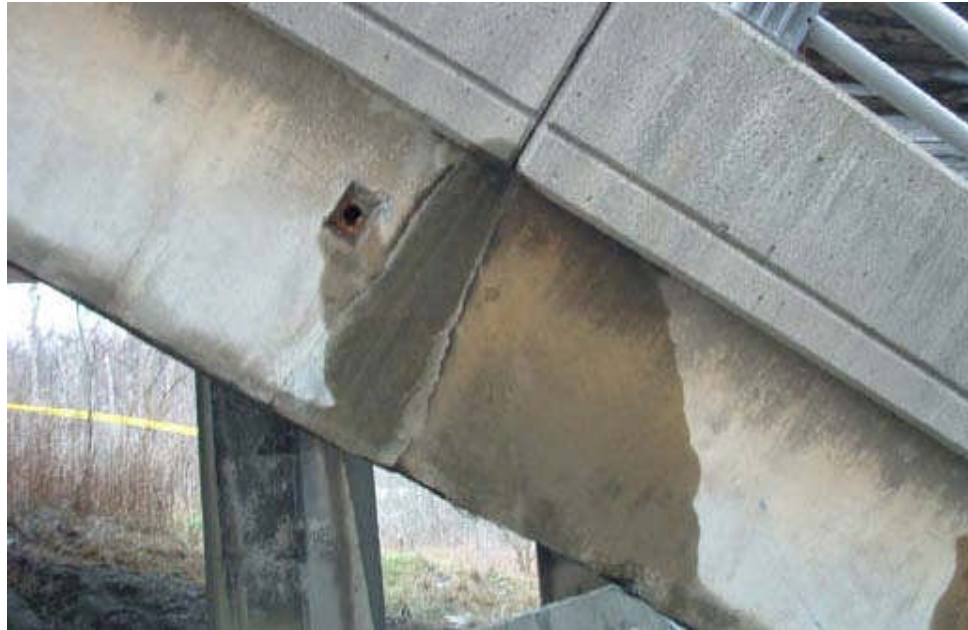
Figure 9.10. 29 Water Leakage Through Parapet Deflection Joints
