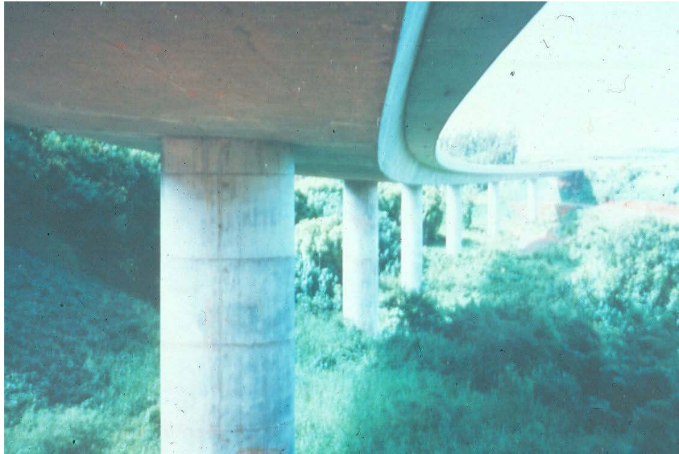
Figure 9.11.2 Cast-in-place Concrete Box Girder Bridge
