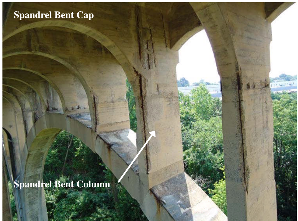
Figure 9.5.13 Spandrel Column Bent Cap Interface
