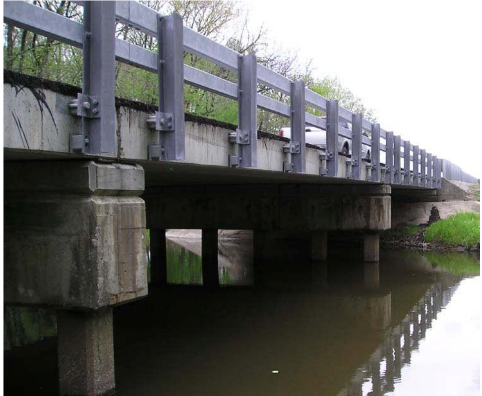
Figure 9.7.1 Typical Prestressed Slab Beam Bridge
