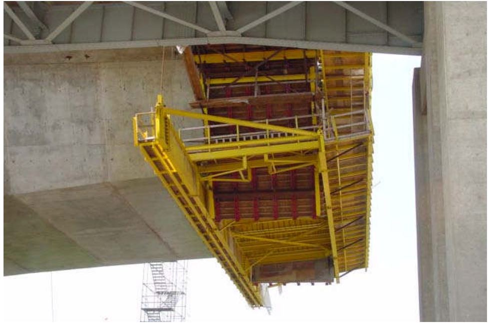
Figure 9.11.17 Cast-in-place Box Girder Segment
