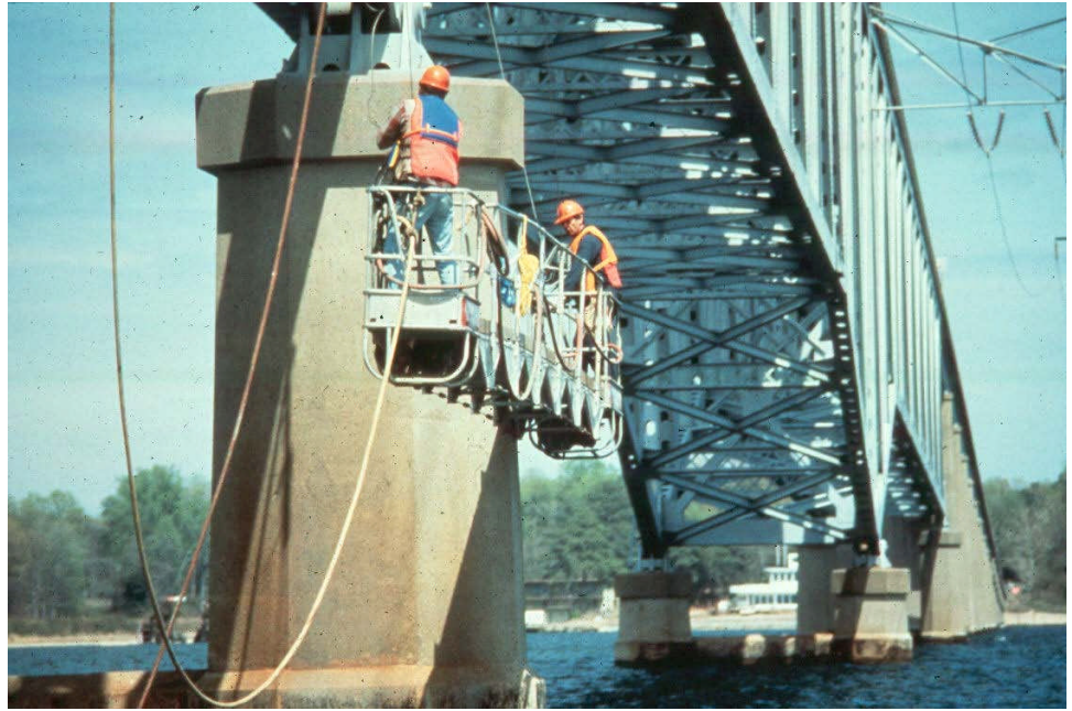
Figure 2.5.3 Rigging for Substructure Inspection
