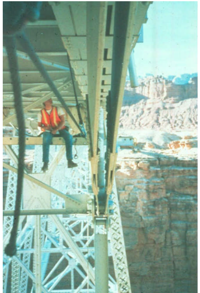
Figure 2.5.4 Rigging for Superstructure Inspection
