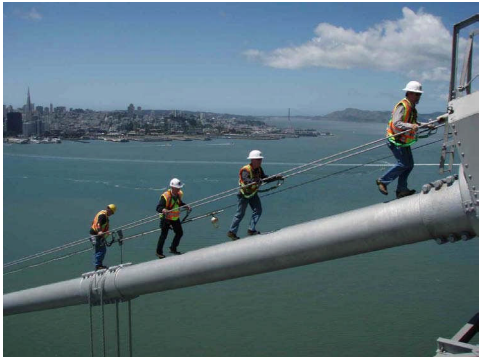
Figure 2.5.14 Handrail on Suspension Bridge
