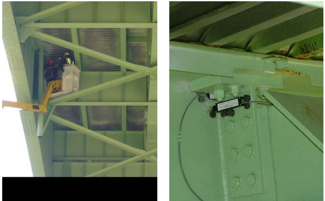
Figure 15.4.1 Installation of Sensors
