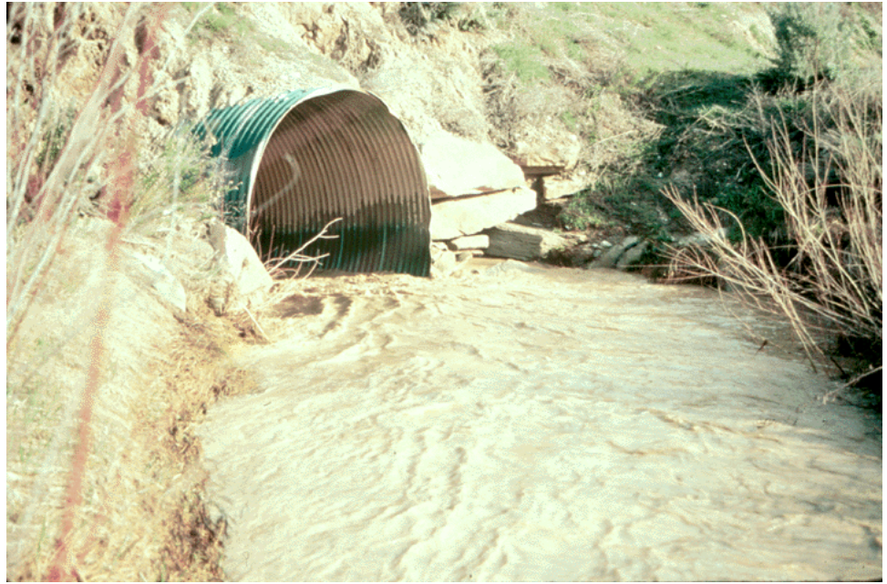
Figure 14.1.18 Culvert End Projection
