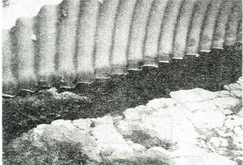
Figure 14.3.21 (Exhibit 79) Erosion Damage to Concrete Invert
