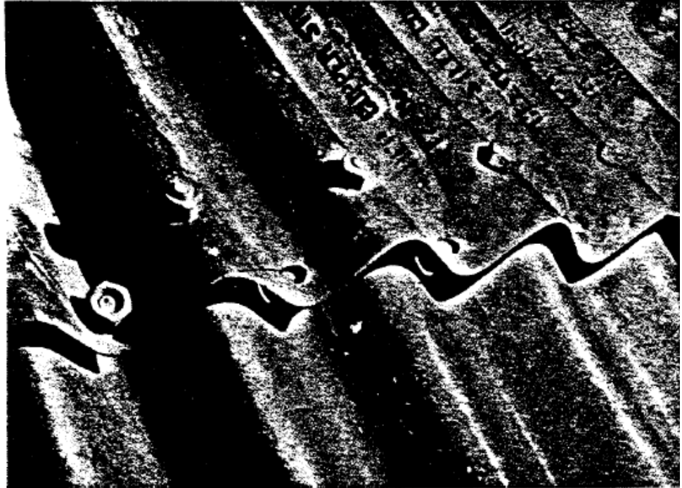
Figure 14.3.11 (Exhibit 69) Close-Up of Loose and Missing Bolts at a Cusped Seam; Loose Fasteners are Usually Detected by Tapping the Nuts with a Hammer
