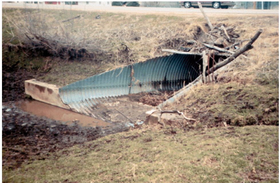
Figure 14.1.19 Culvert Mitered End
