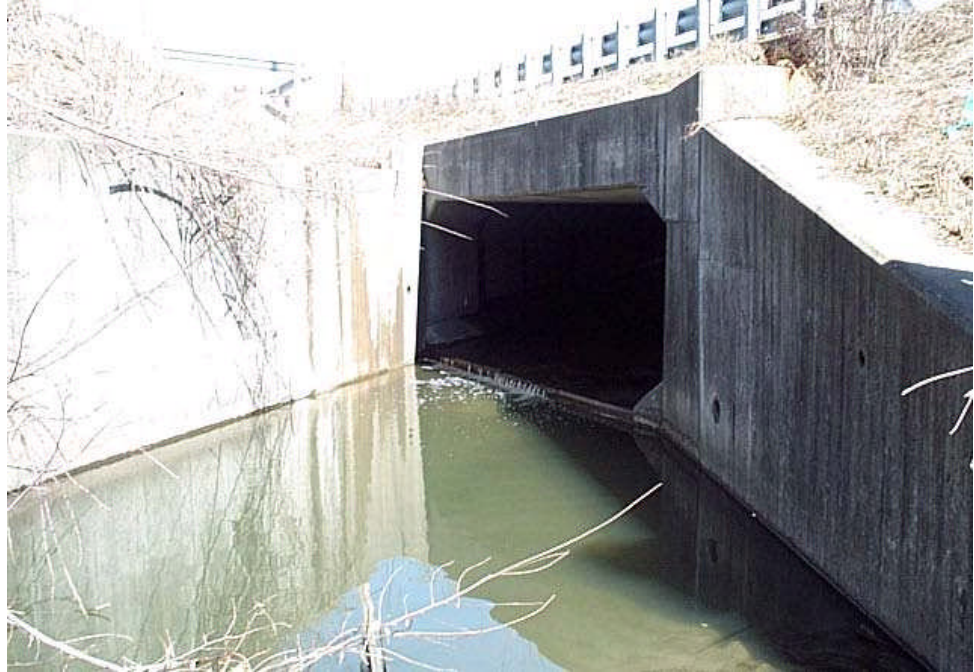
Figure 14.1.20 Culvert Skewed End
