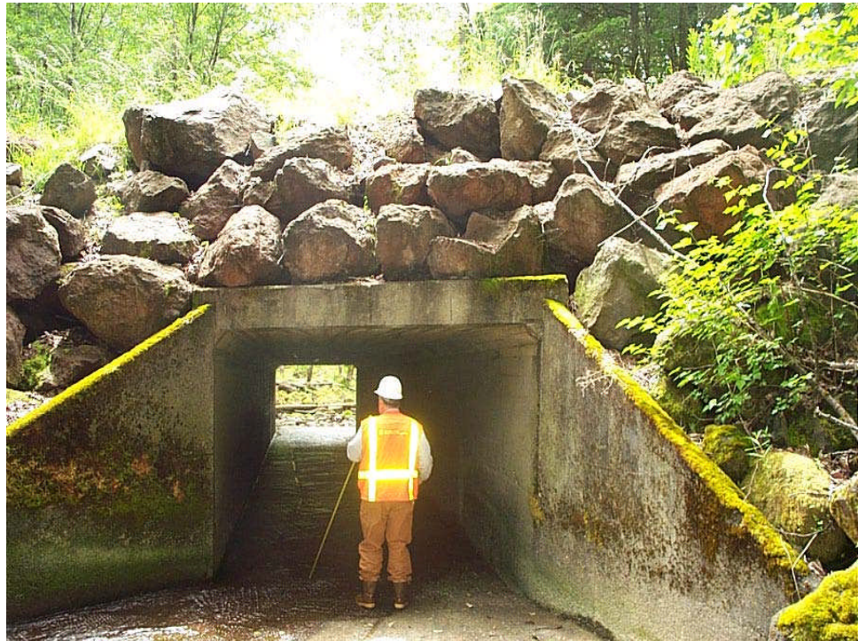
Figure 14.1.33 Potential for Tilted Wingwalls
