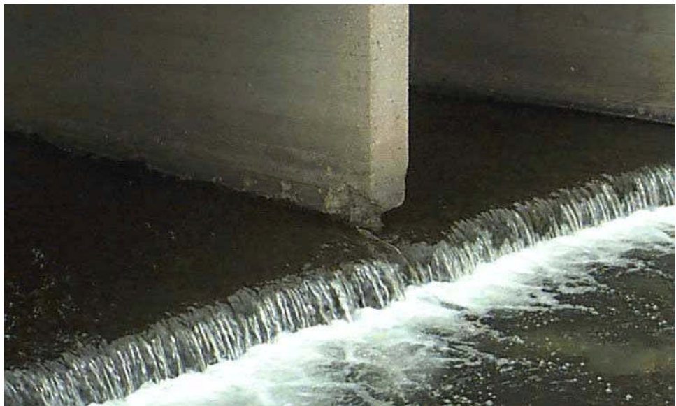
Figure 14.1.37 Energy Dissipater
