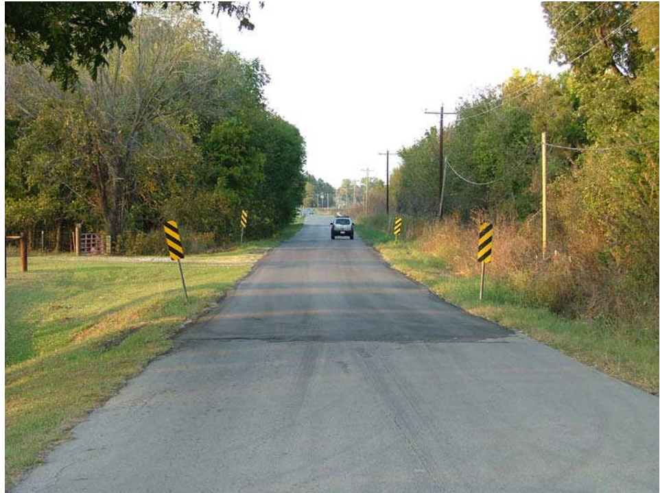
Figure 14.1.30 Repaired Roadway Over a Culvert
