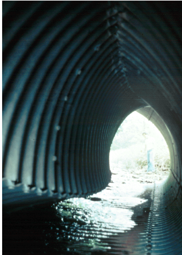
Figure 14.1.25 Bending or Shear Failure
