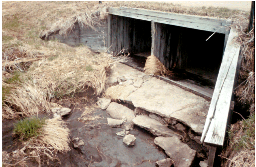
Figure 14.1.27 Scour and Undermining at Culvert Inlet
