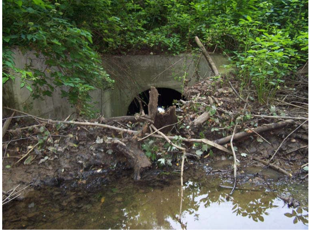
Figure 14.1.28 Debris and Sediment Buildup
