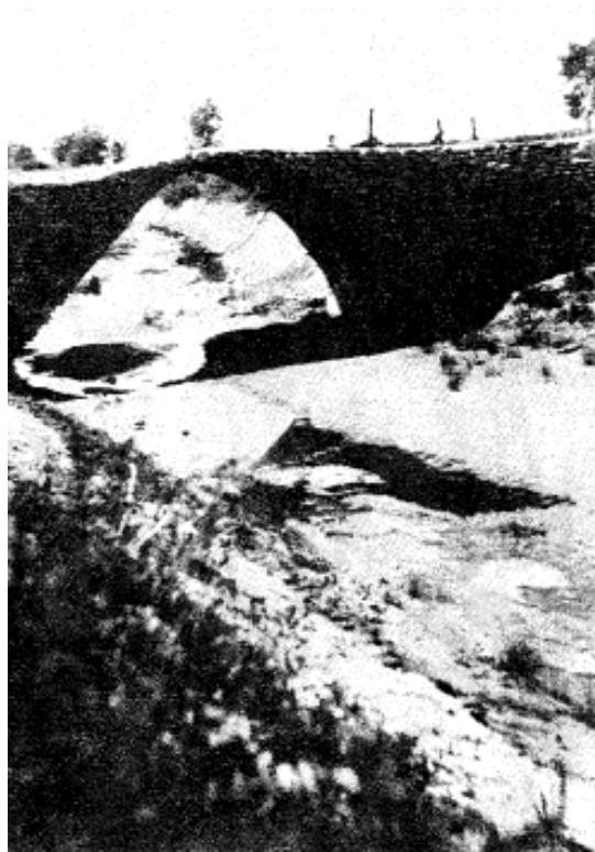
Figure 14.3.30 (Exhibit 88) Racked and Peaked Arch
