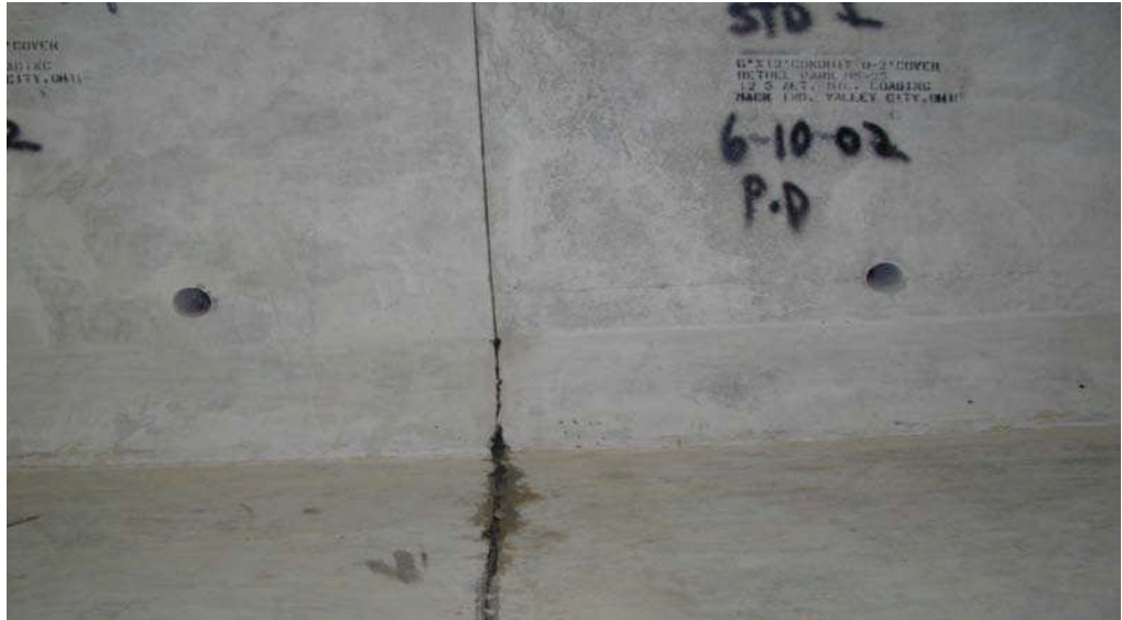
Figure 14.2.19 Precast Concrete Box Culvert Joint
