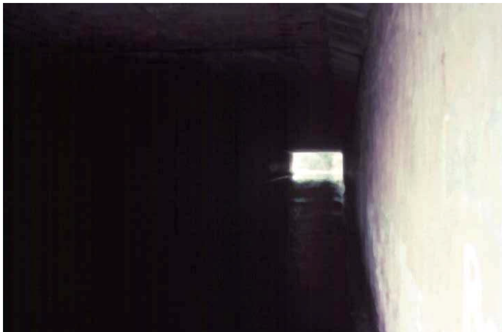
Figure 14.2.16 Sighting Along Culvert Sidewall to Check Horizontal Alignment
