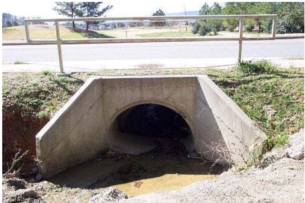
Figure 14.1.21 Culvert Headwall and Wingwalls
