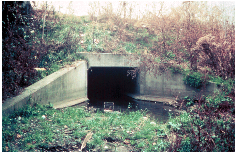
Figure 14.1.35 Culvert Headwall and Wingwall End Treatment
