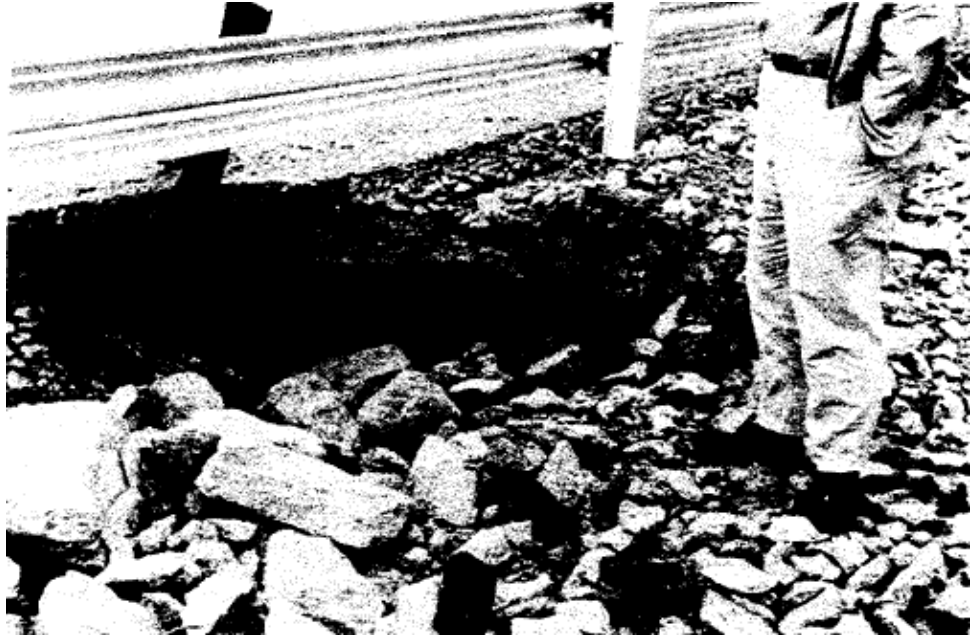
Figure 14.3.10 (Exhibit 68) Surface Hole Above Open Joint
