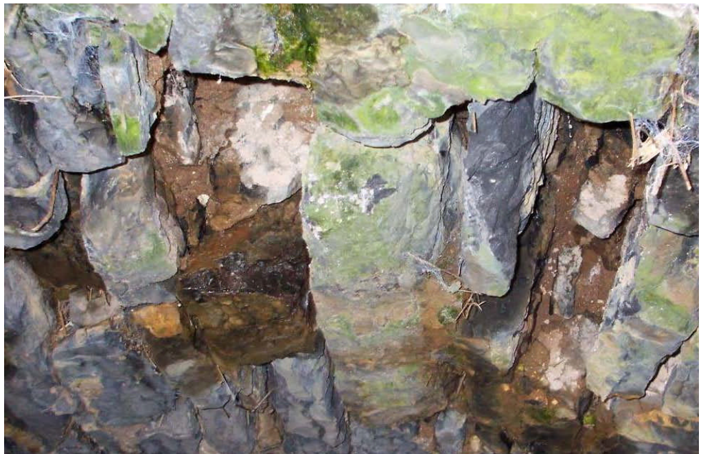
Figure 14.2.18 Missing Stones in Masonry Culvert
