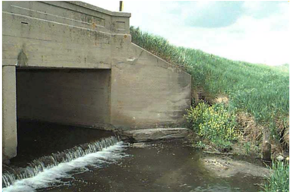
Figure 14.2.23 Cast-in-Place Concrete Headwall and Wingwall
