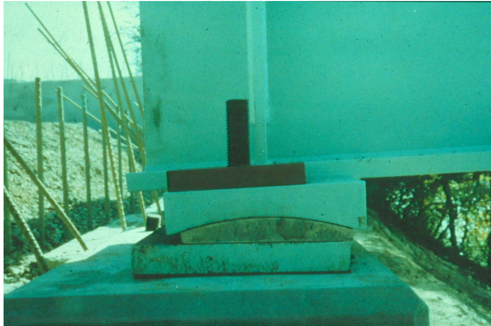
Figure 11.1.5 Bronze Sliding Plate Bearing
