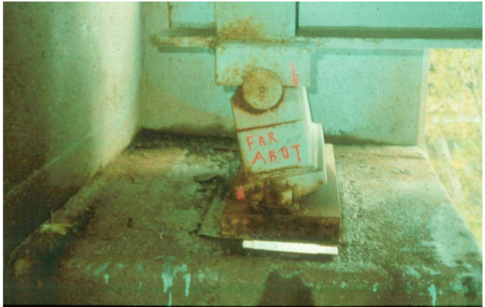
Figure 11.1.43 Broken Pintle on a Bearing
