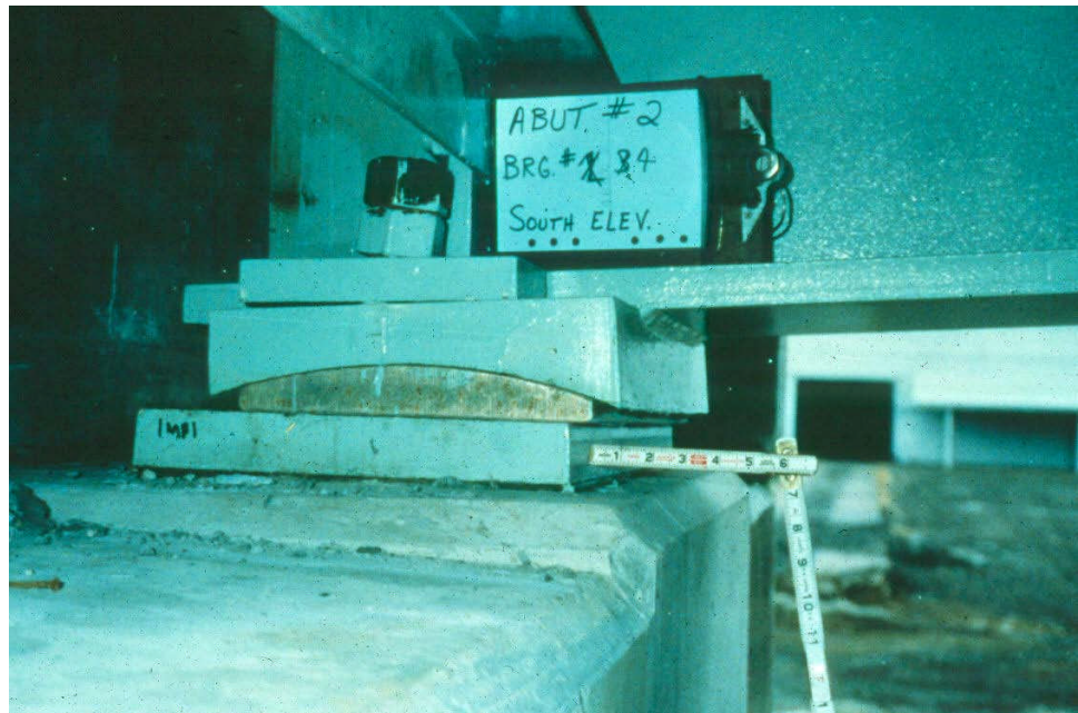
Figure 11.1.32 Longitudinal Misalignment in Bronze Sliding Plate Bearing
