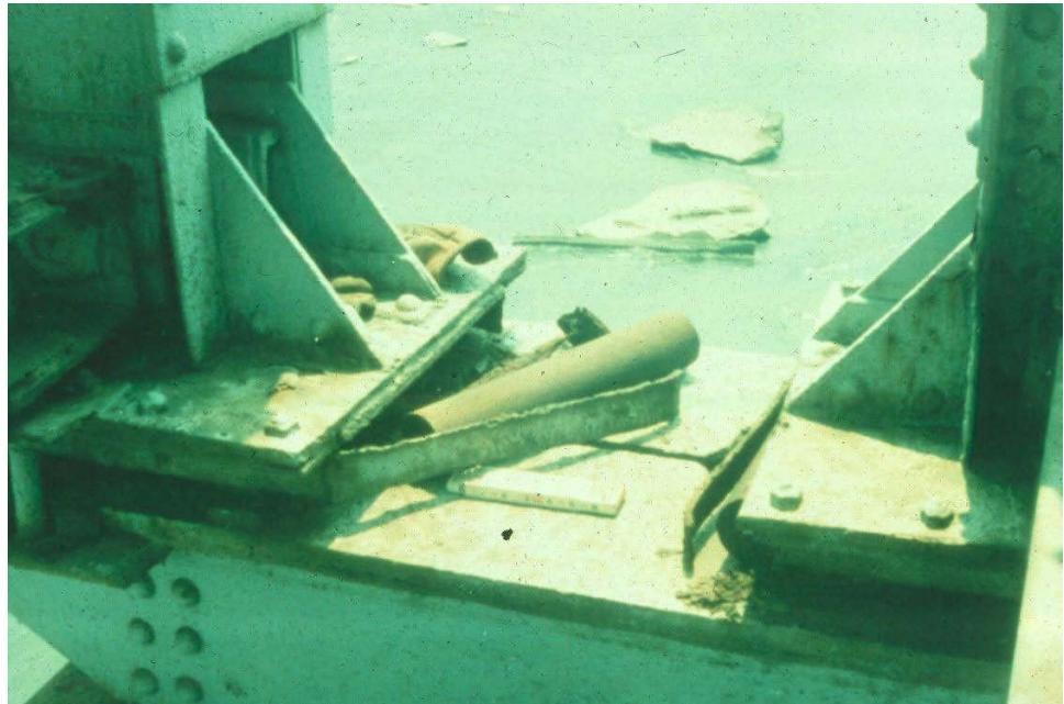
Figure 11.1.34 Damaged Roller Nest Bearing
