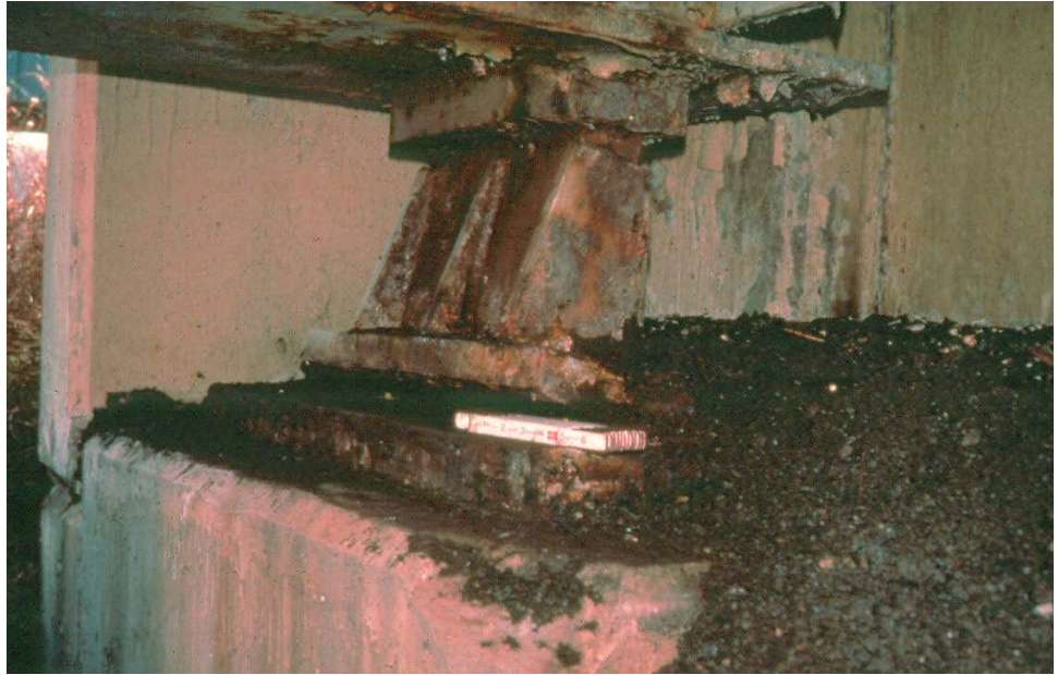
Figure 11.1.28 Heavy Corrosion on a Steel Rocker Bearing
