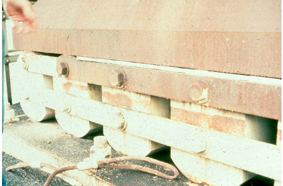
Figure 11.1.11 Segmental Rocker Nest Bearing
