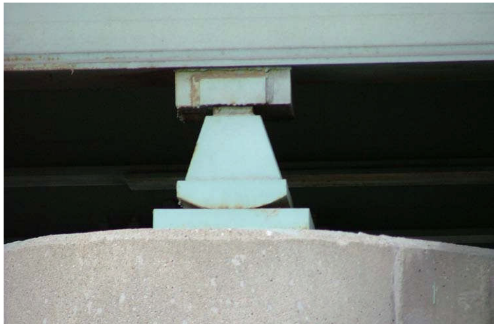
Figure 11.1.9 Rocker Bearing
