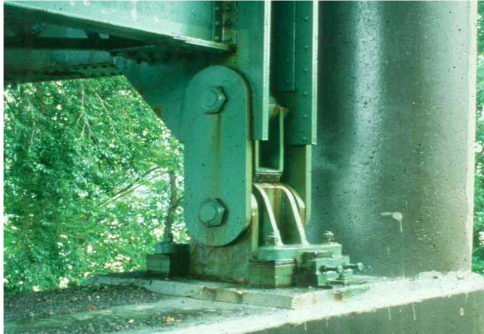
Figure 11.1.19 Pin and Link Bearing
