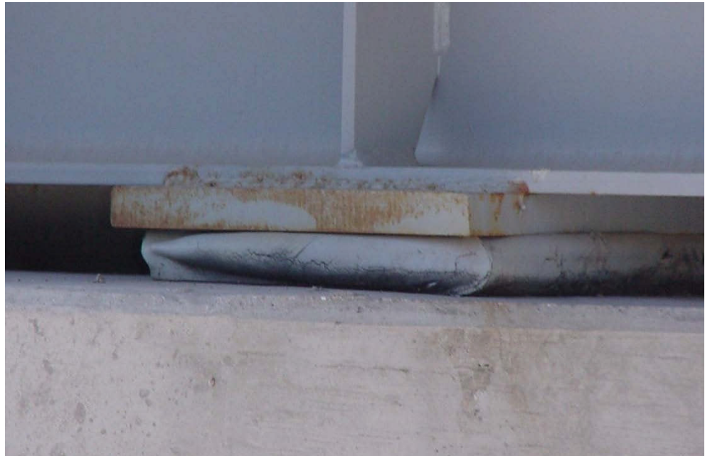
Figure 11.1.40 Neoprene Bearing Pad Excessive Bulging
