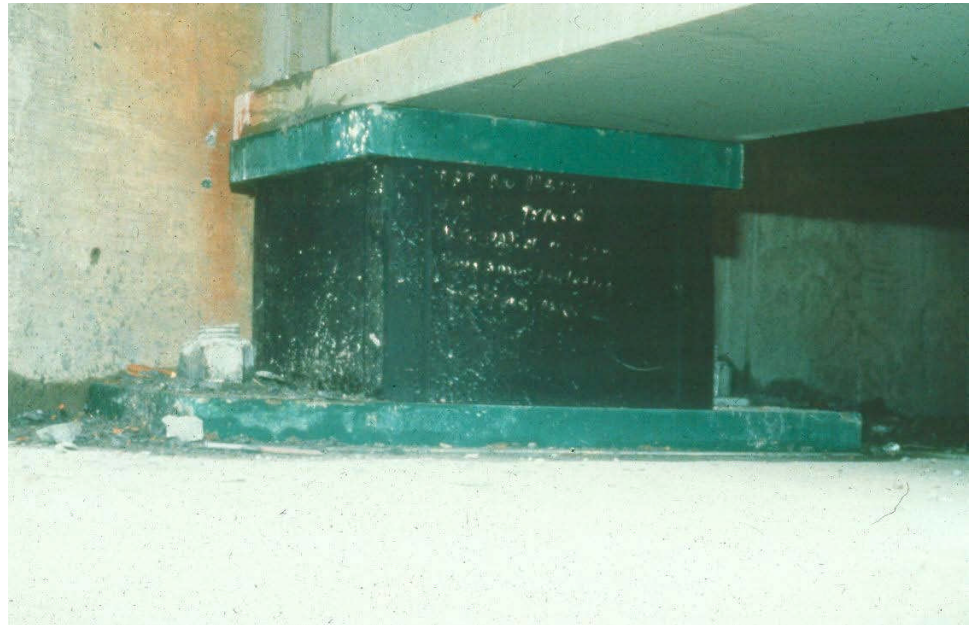
Figure 11.1.22 Lead Core Isolation Bearing
