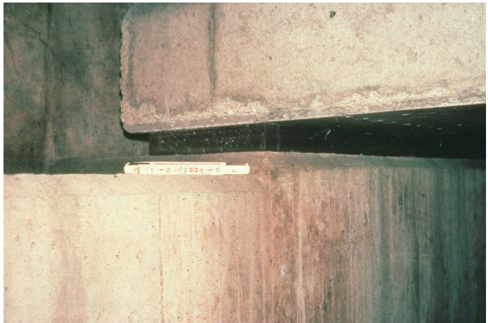
Figure 11.1.13 Plain Neoprene Bearing Pad
