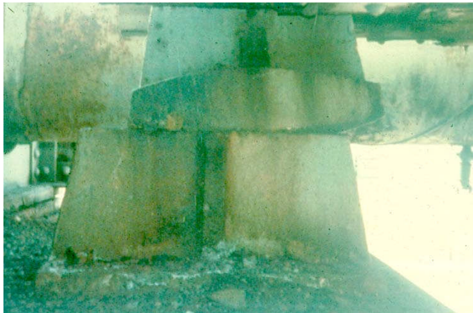
Figure 11.1.29 Rocker Bearing with Excessive Horizontal Movement
