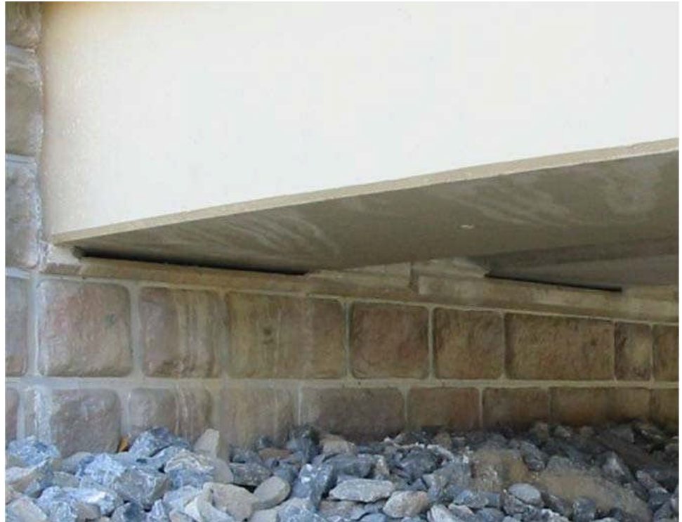
Figure 11.1.18 Enclosed or Concealed Bearing
