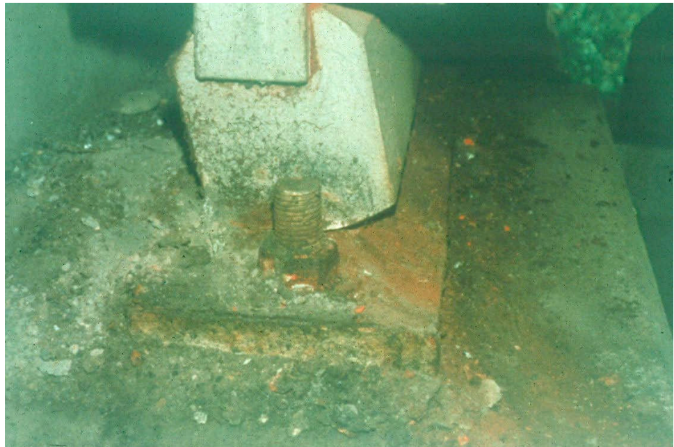
Figure 11.1.10 Segmental Rocker Bearing
