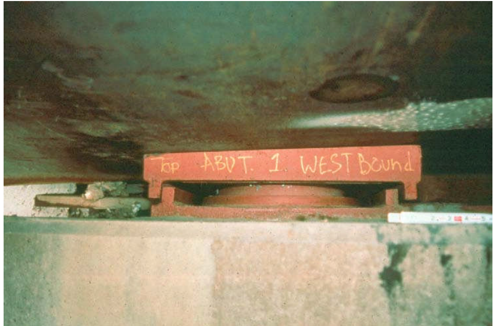
Figure 11.1.15 Neoprene Pot Bearing with Guide Bars
