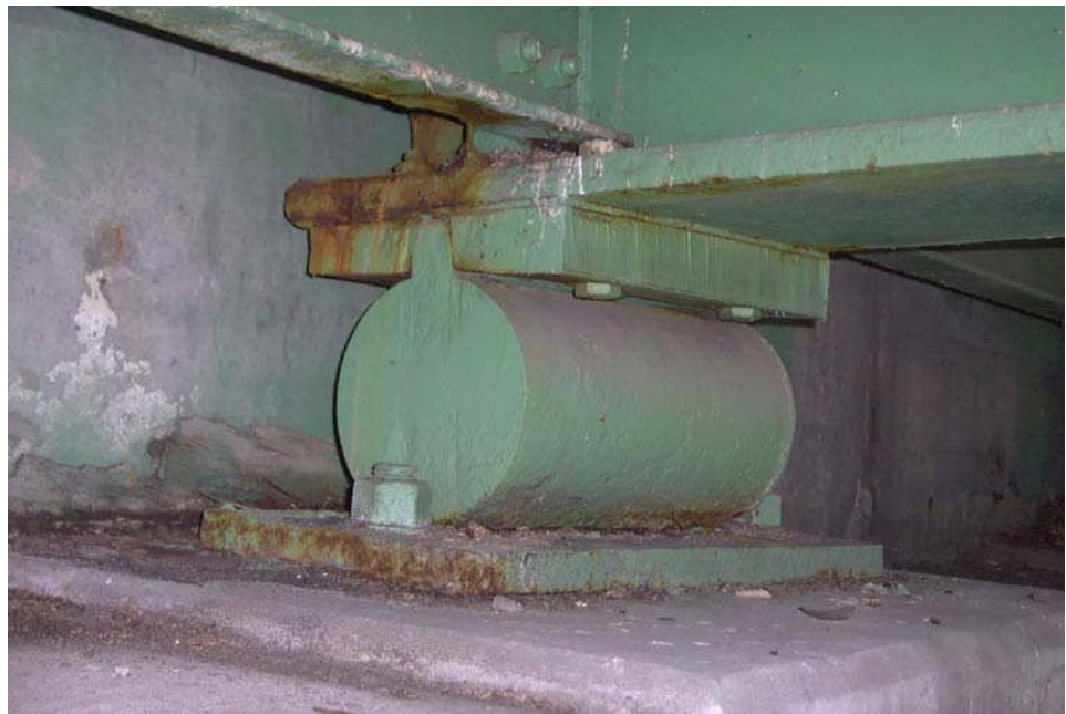
Figure 11.1.7 Single Roller Bearing
