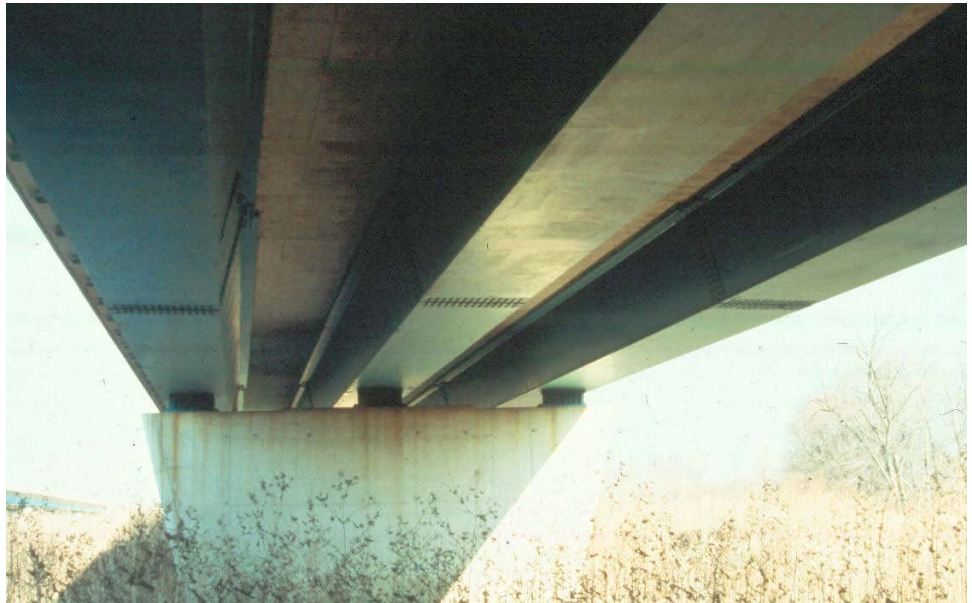
Figure 10.3.13 Redundant Box Girder Bridge
