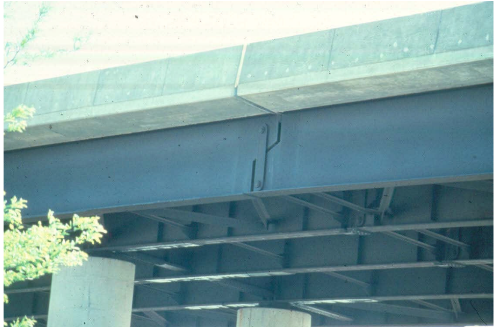
Figure 10.1.9 Fabricated Multi-girder Bridge with Pin & Hanger Connection
