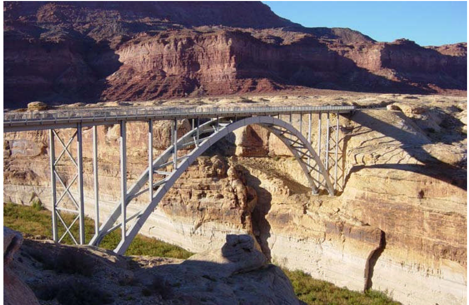
Figure 10.5.1 Deck Arch Bridge
