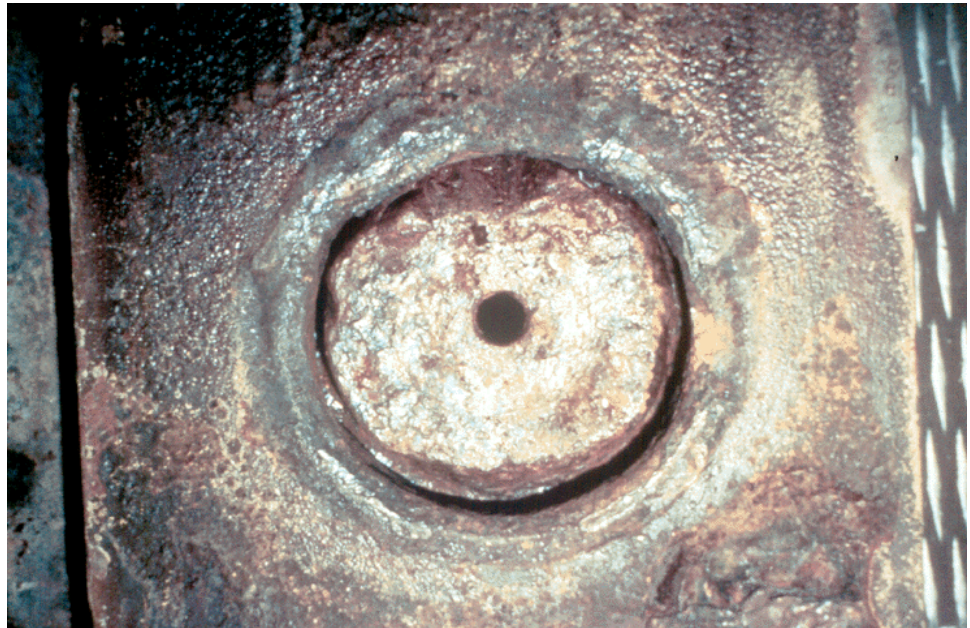
Figure 10.7.24 Corroded Pin-and-Hanger Assembly
