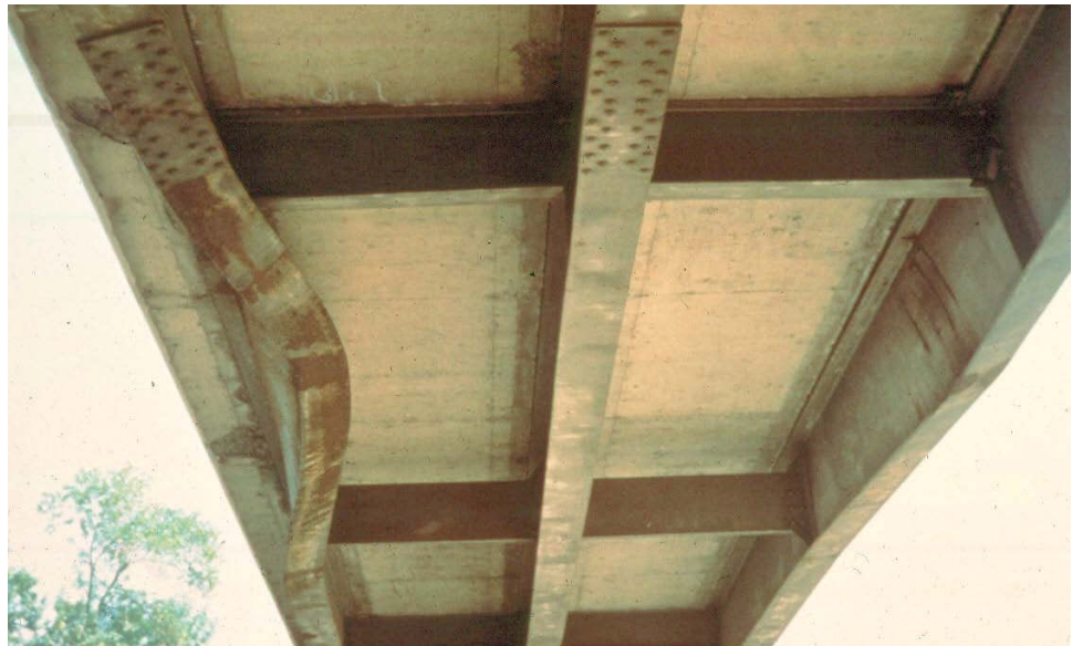
Figure 10.1.24 Collision Damage on a Fabricated Multi-Girder Bridge
