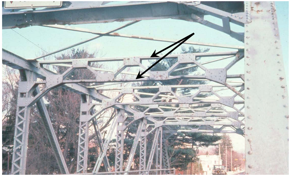
Figure 10.4.36 Sway Bracing
