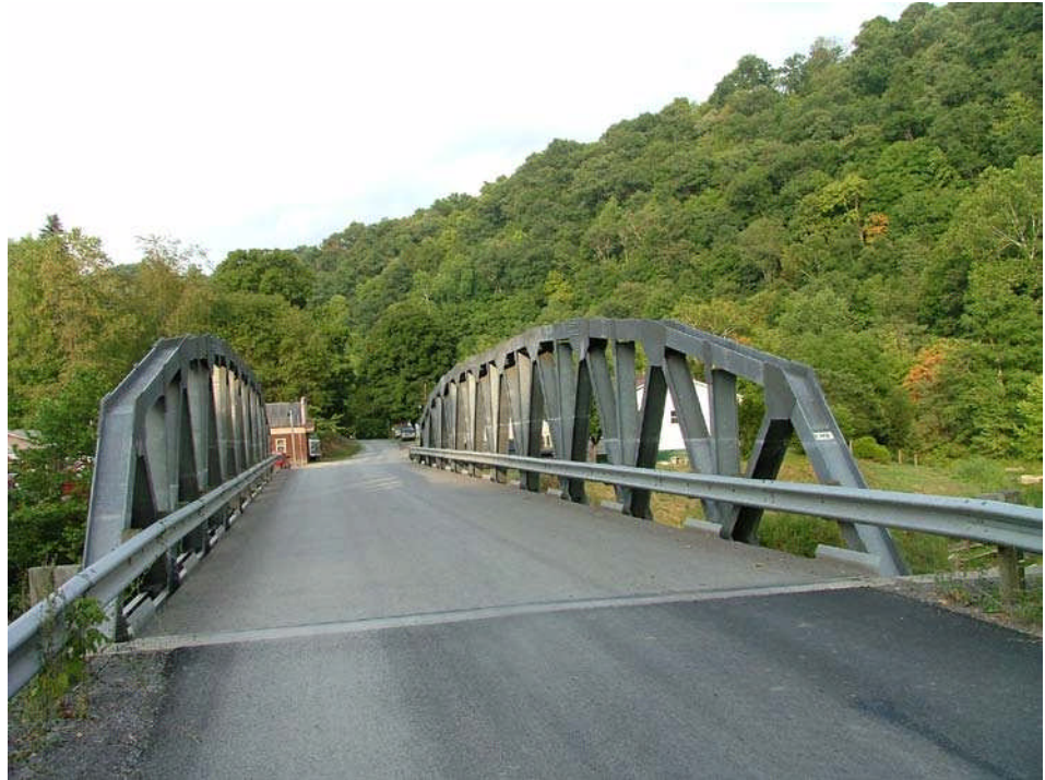
Figure 10.4.10 Single (Simple) Span Camel Back Pratt Truss
