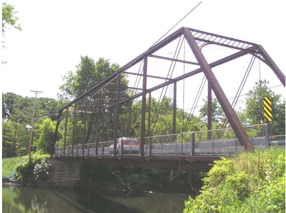
Figure 10.4.11 Single (Simple) Span Through Truss
