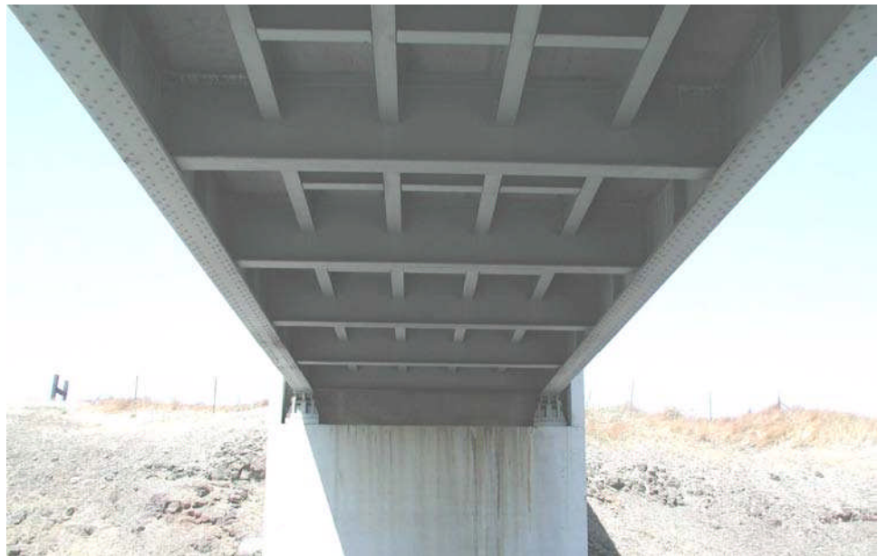
Figure 10.2.6 Two-Girder Bridge with Girder-Floorbeam-Stringer System
