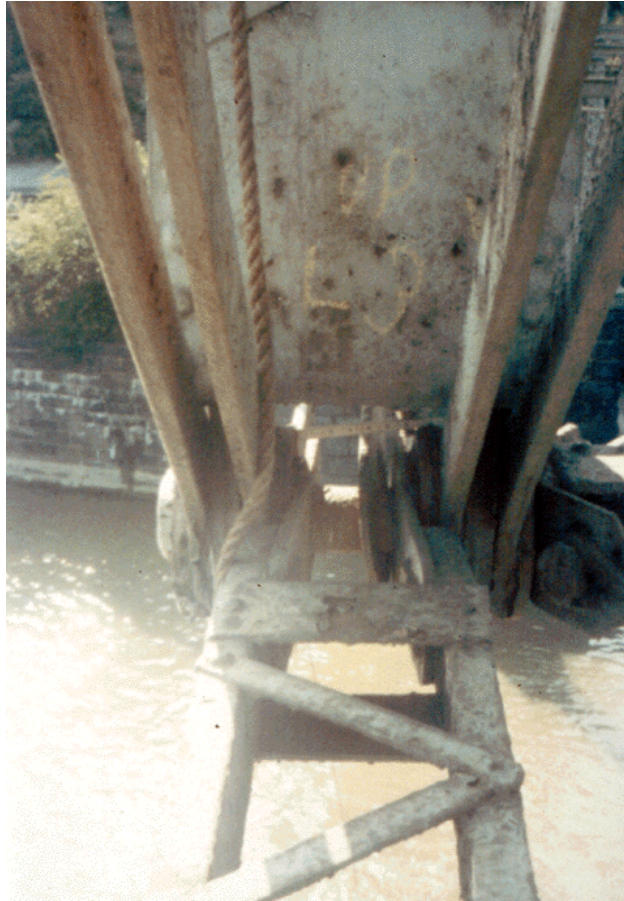
Figure 10.9.15 Loosely Packed Eyebars Connection
