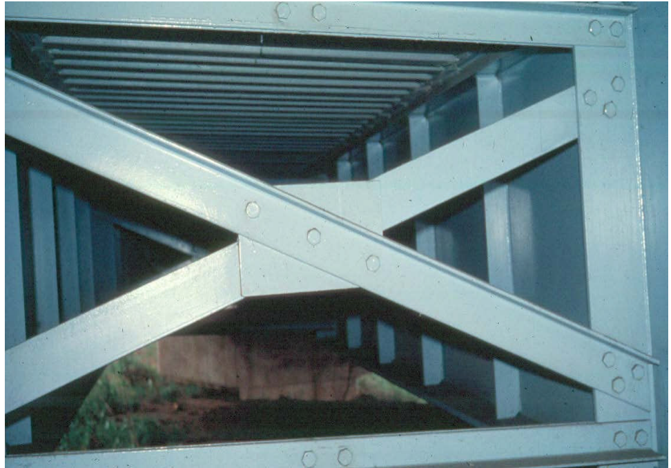
Figure 10.1.22 Intermediate Diaphragm
