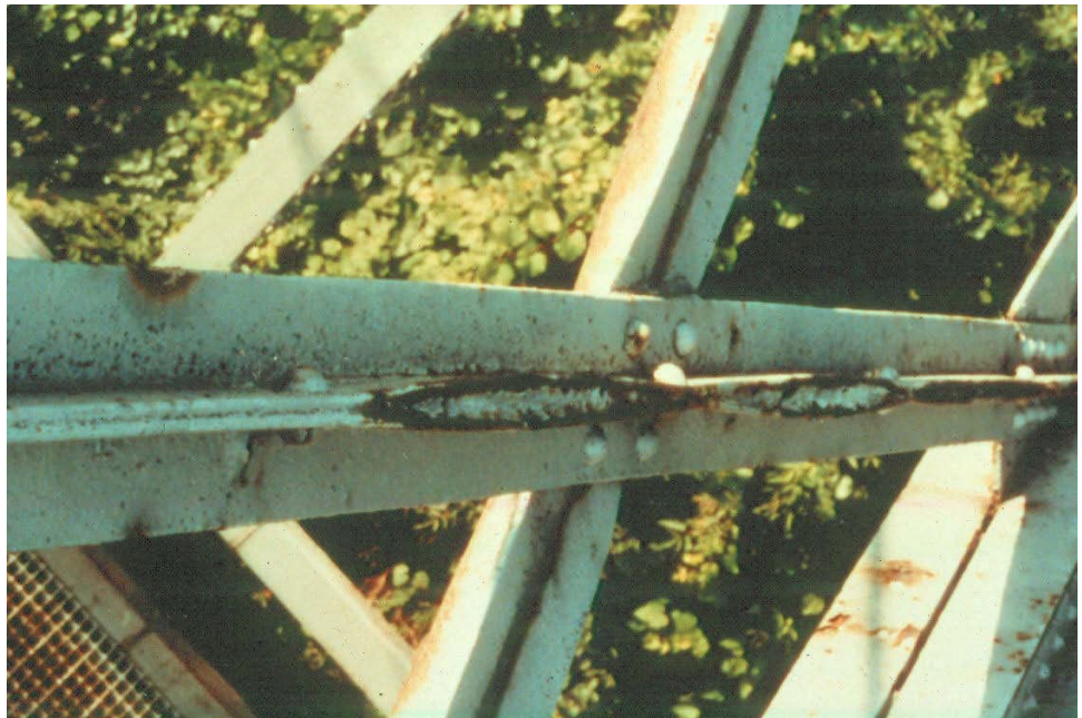
Figure 10.4.58 Sway Bracing with Pack Rust
