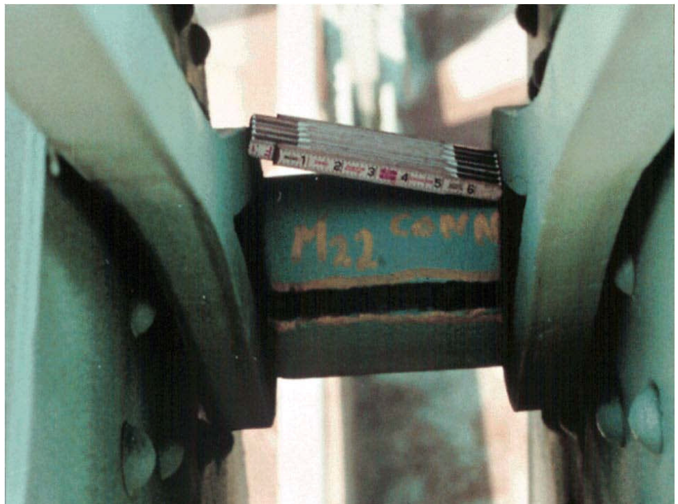
Figure 10.9.17 Steel Pin Spacer or Filling Ring
