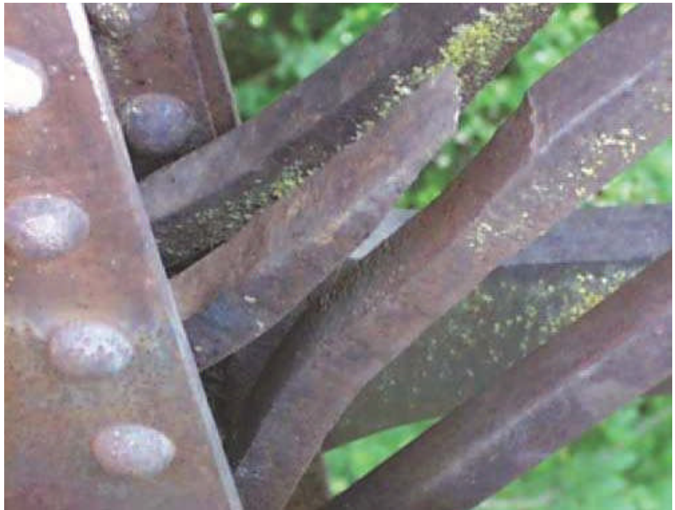
Figure 10.9.20 Forge Loop is Completely Apart
