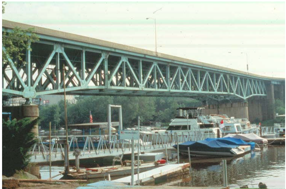
Figure 10.4.15 Cantilever Deck Truss
