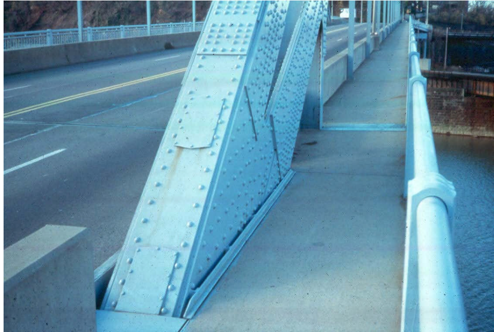
Figure 10.5.24 Through Arch Member Exposed to Traffic
