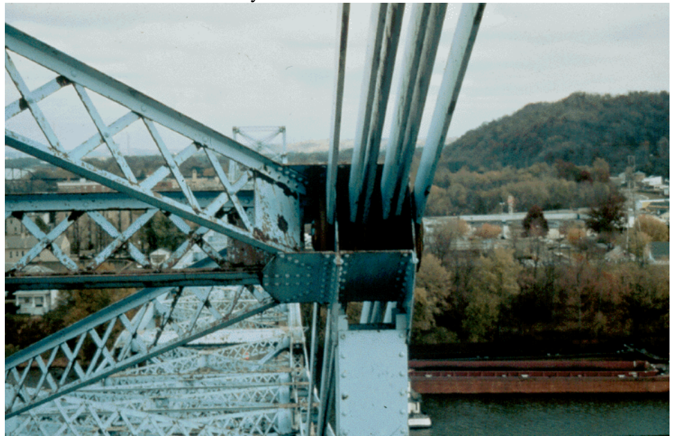
Figure 10.9.32 Fracture Critical Top Chord Truss Member: Internally Redundant Eyebars
