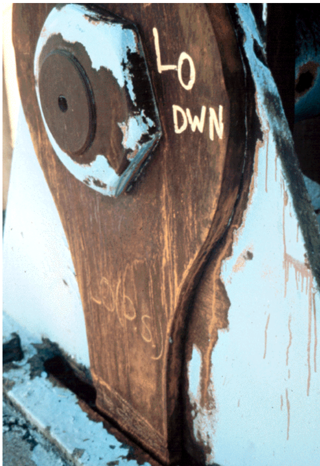
Figure 10.9.4 Anchorage Eyebars
