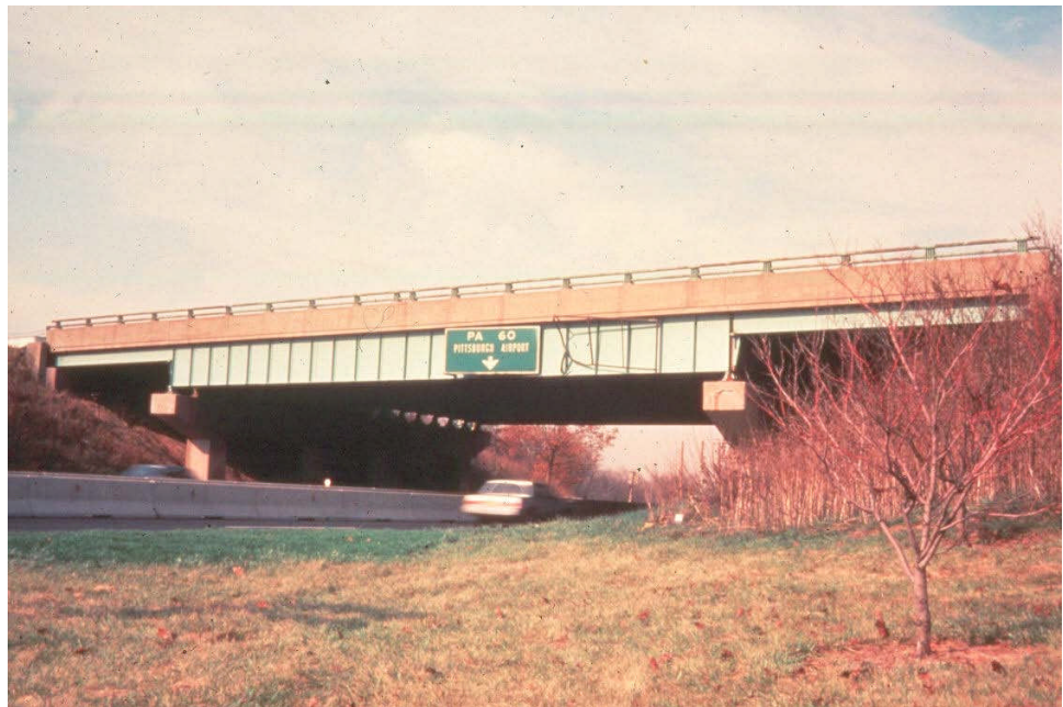
Figure 10.1.10 Combination Rolled Beams and Fabricated Girders
