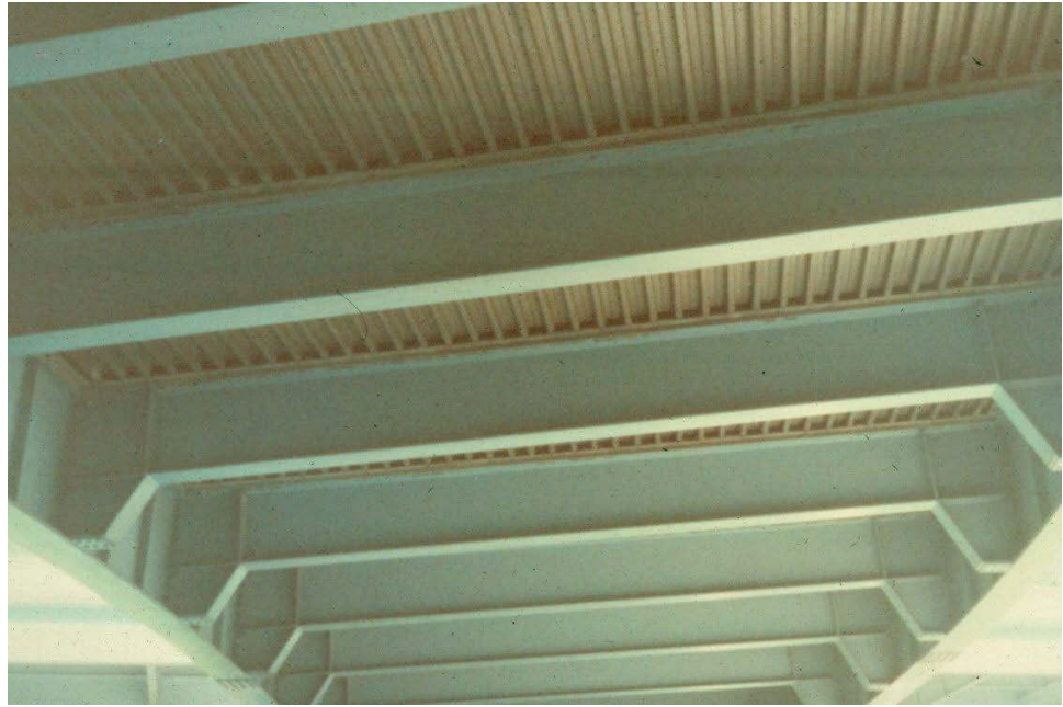
Figure 10.2.5 Two-Girder Bridge with Girder-Floorbeam System
