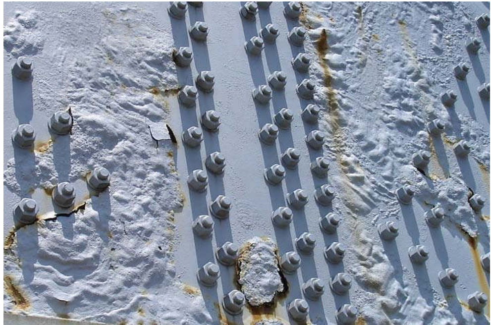
Figure 10.8.28 Gusset Plate with Paint Failure
