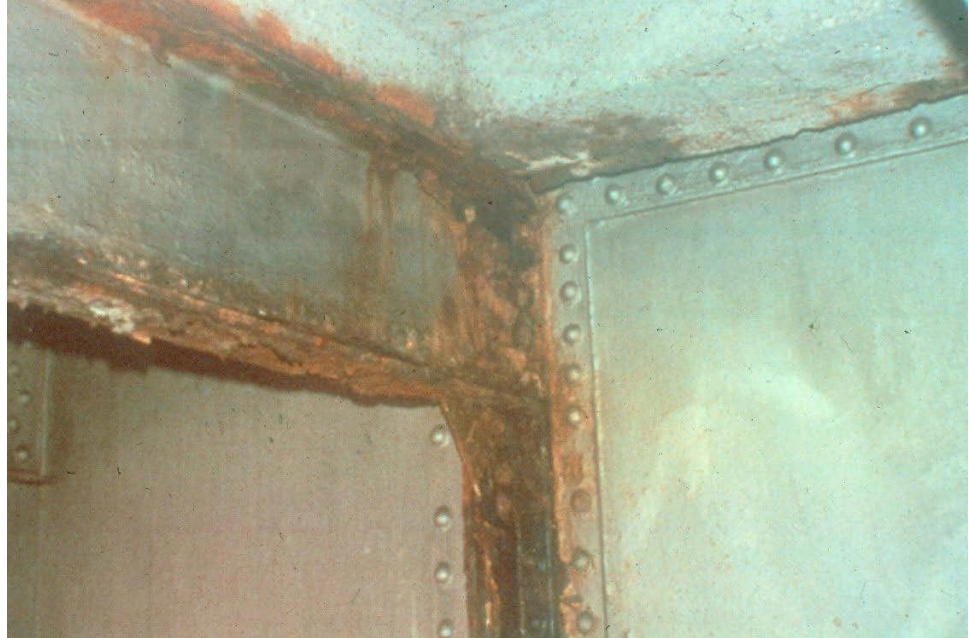
Figure 10.2.11 Shear Zone on a Deck Girder Bridge
