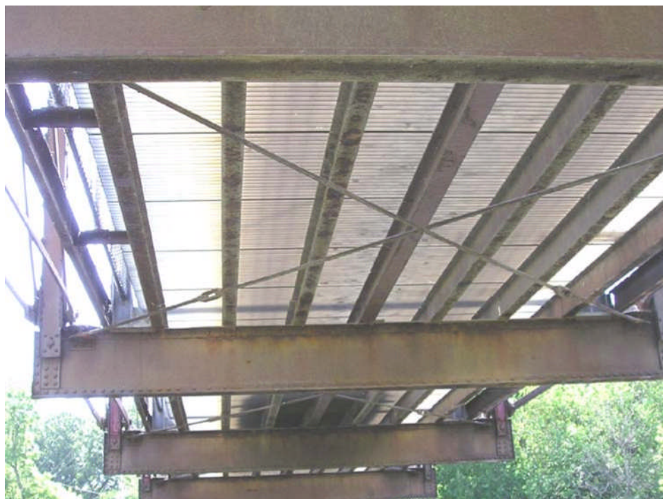
Figure 10.4.53 Corroded Stringers under an Open Grid Deck
