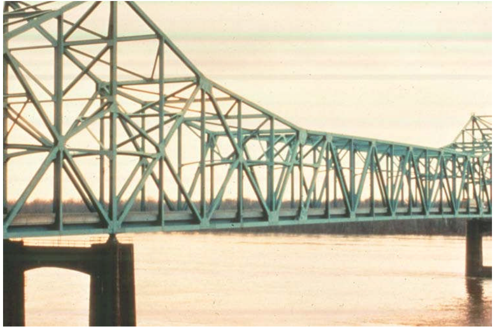
Figure 10.4.16 Cantilever Through Truss
