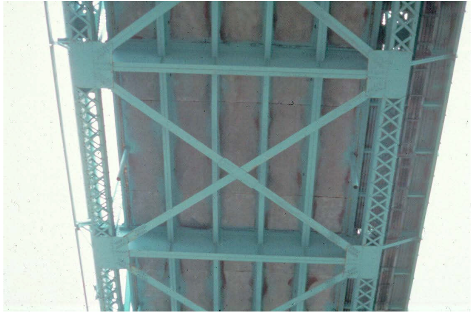
Figure 10.4.34 Lower Lateral Bracing
