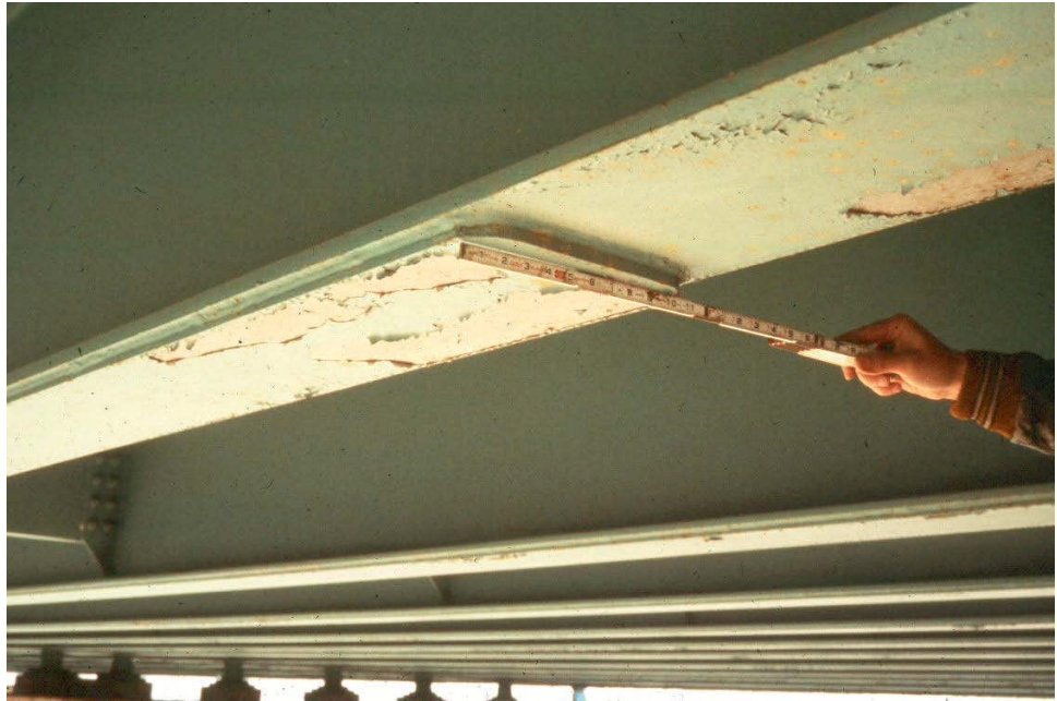
Figure 10.1.3 Rolled Multi-Beam Bridge with a Cover Plate
