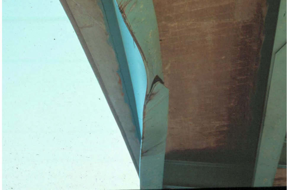
Figure 10.1.23 Collision Damage on a Rolled Multi-Beam Bridge
