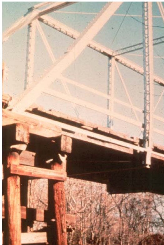
Figure 10.4.50 Buckled End Post
