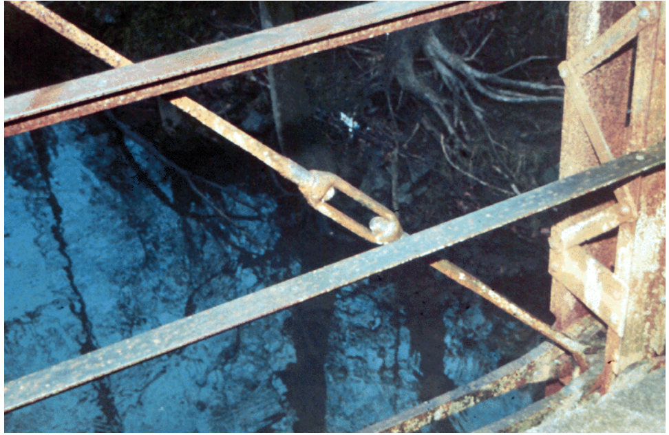
Figure 10.9.28 Turnbuckle on a Truss Diagonal
