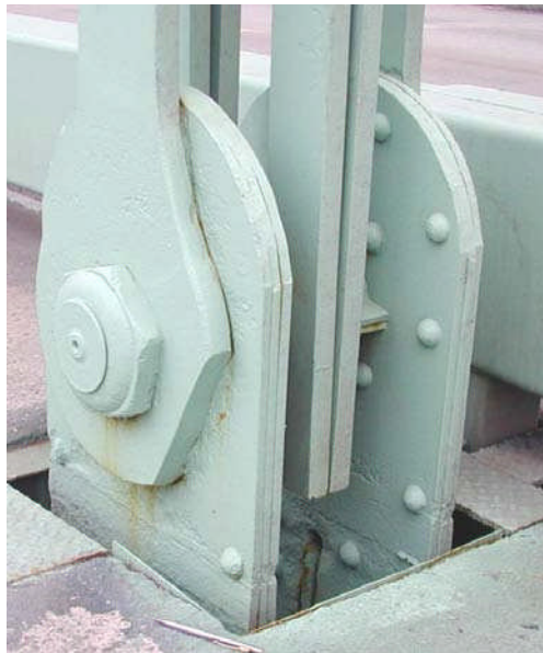
Figure 10.4.17 Pin-and-Hanger Assembly for Cantilevered Truss
