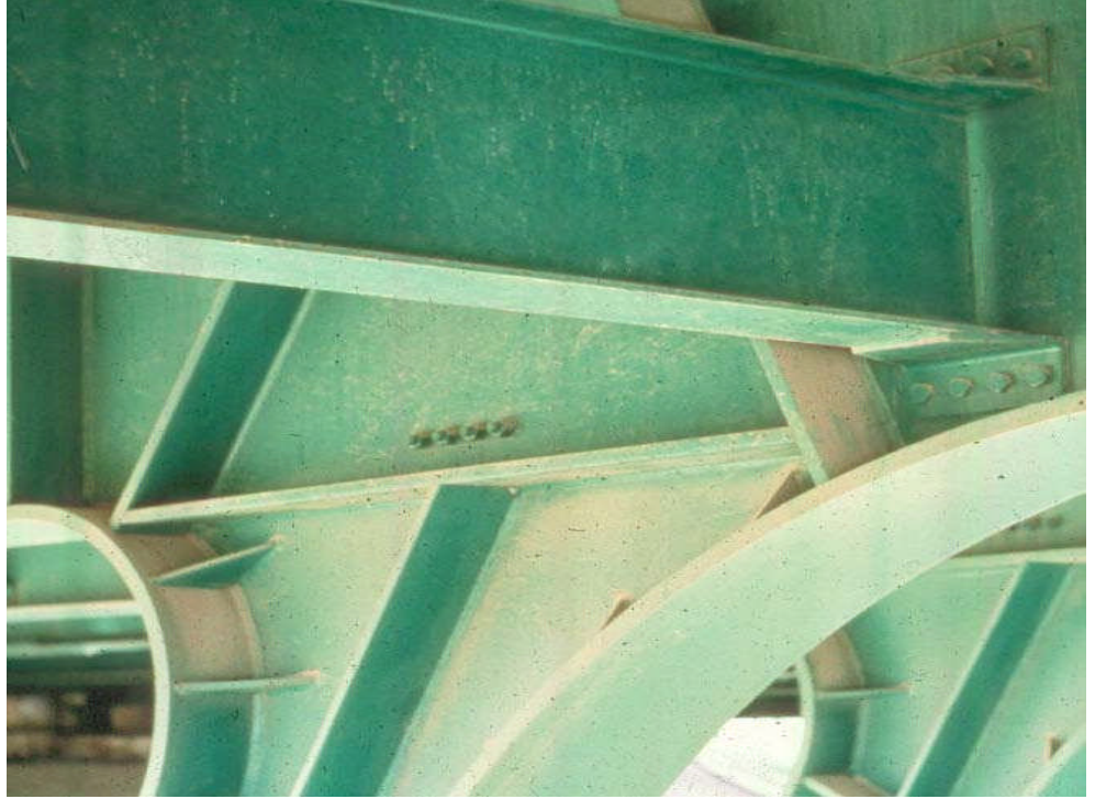
Figure 10.6.3 Connection Between Legs and Girder Portion
