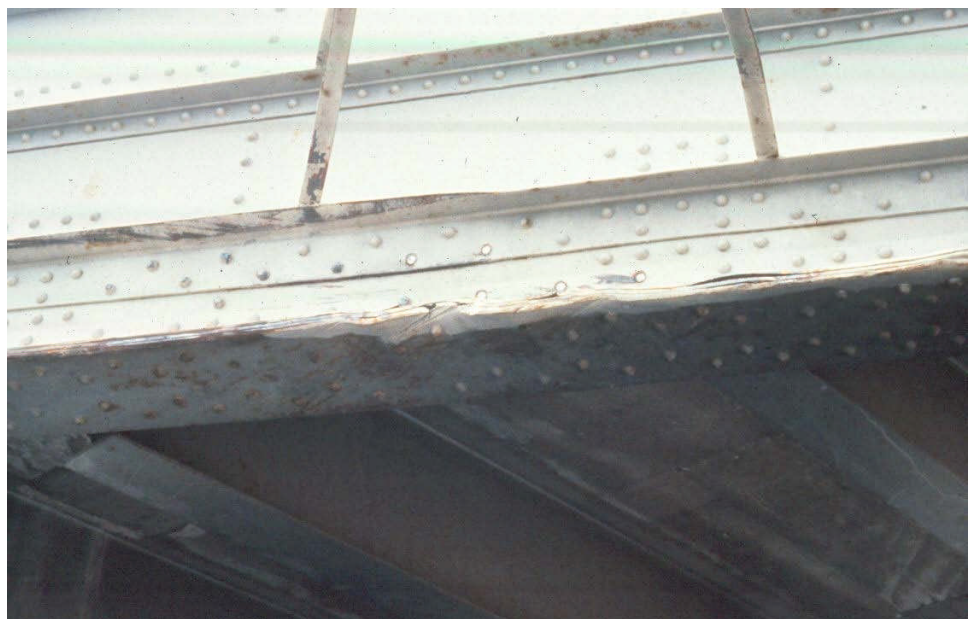
Figure 10.2.19 Collision Damage to a Through Girder Bridge
