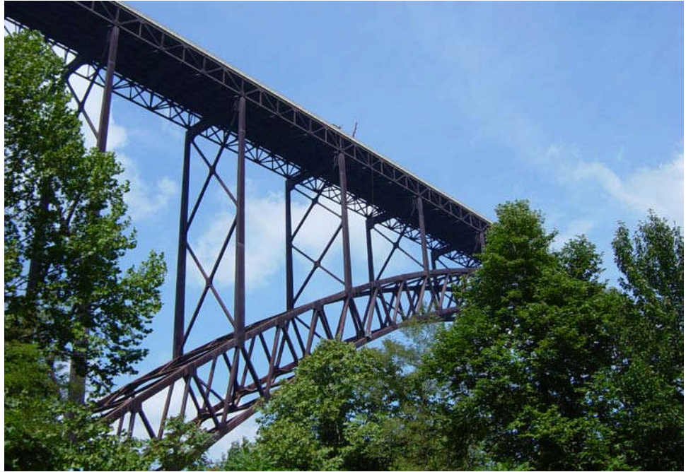
Figure 10.5.20 Braced Rib Deck Arch Showing Spandrel Columns
