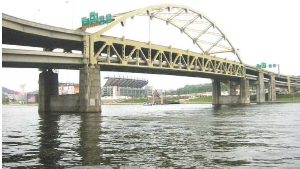
Figure 10.5.3 Tied Arch Bridge
