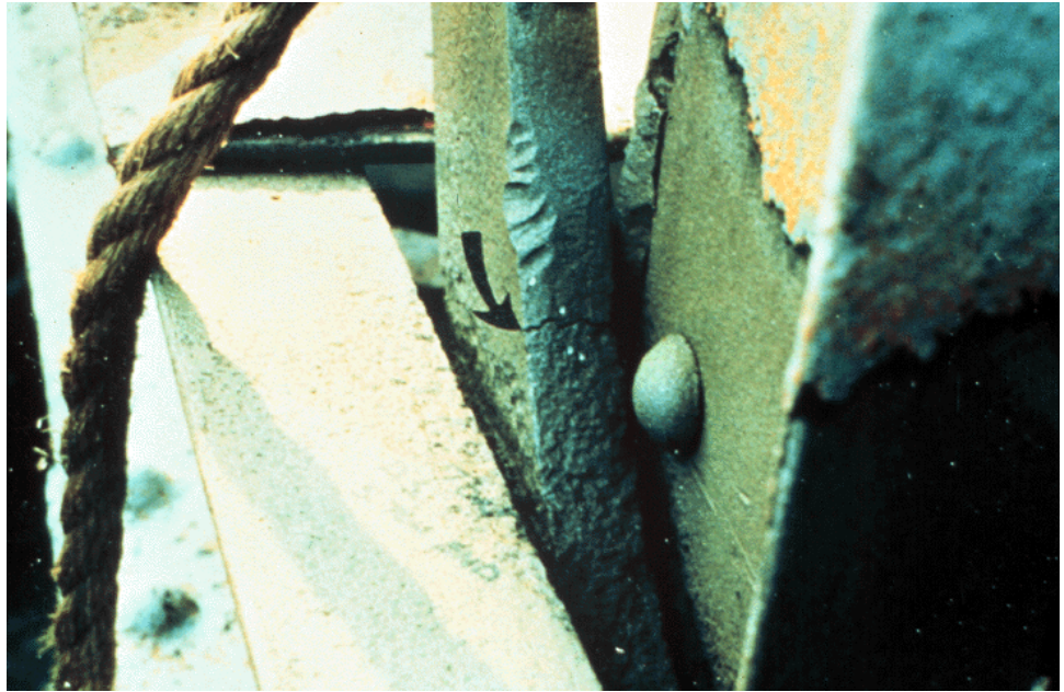
Figure 10.9.19 Close-up of the Forge Zone on an Eyebars (Arrow denotes crack)
