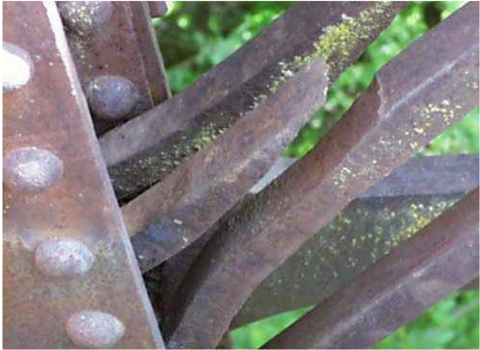
Figure 10.4.44 Cracked Forge Zone on a Loop Rod
