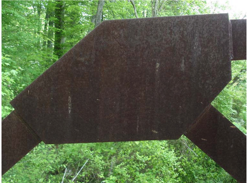
Figure 10.8.4 Steel Gusset Plate with Welded Connections
