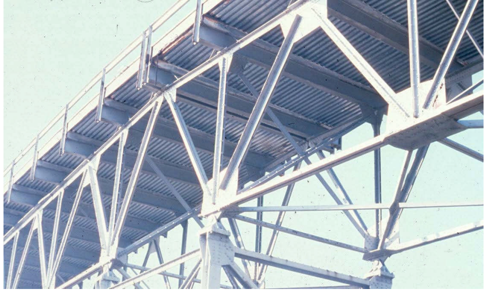
Figure 10.4.32 Floorbeam Floor System
