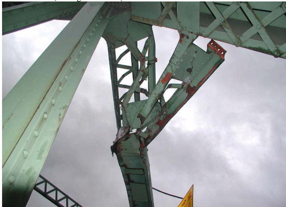
Figure 10.4.56 Collision Damage to Portal
