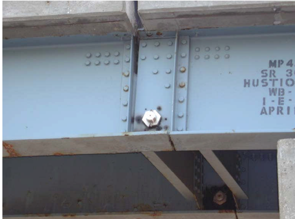
Figure 10.7.2 Single Pin with Riveted Pin Plate
