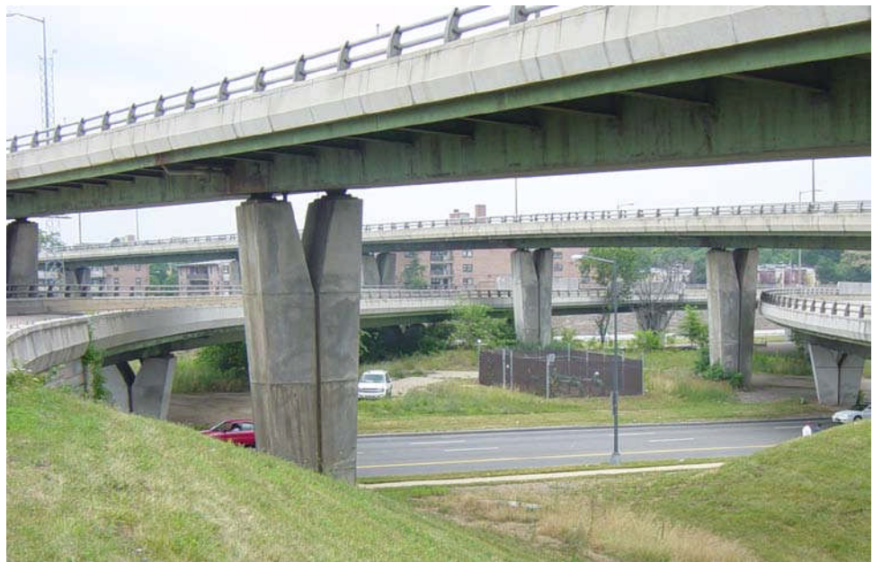
Figure 10.3.11 Continuous Box Girders
