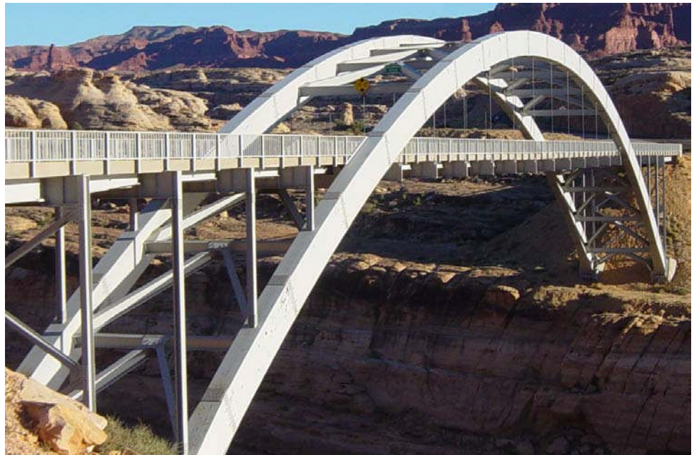
Figure 10.5.2 Through Arch Bridge
