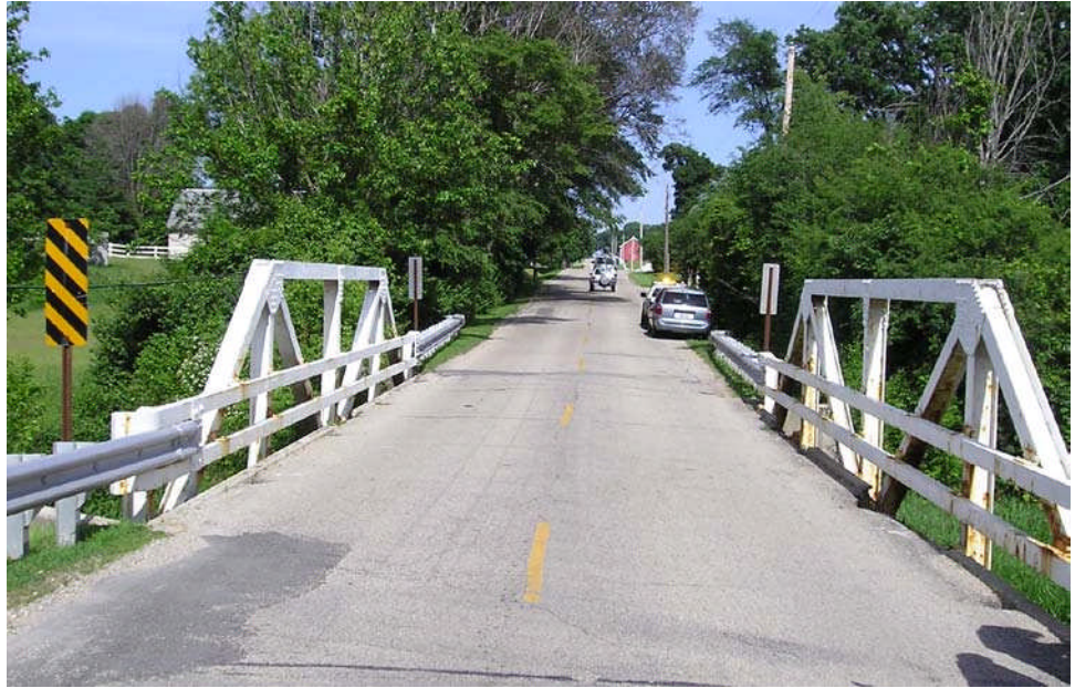
Figure 10.4.4 Pony Truss
