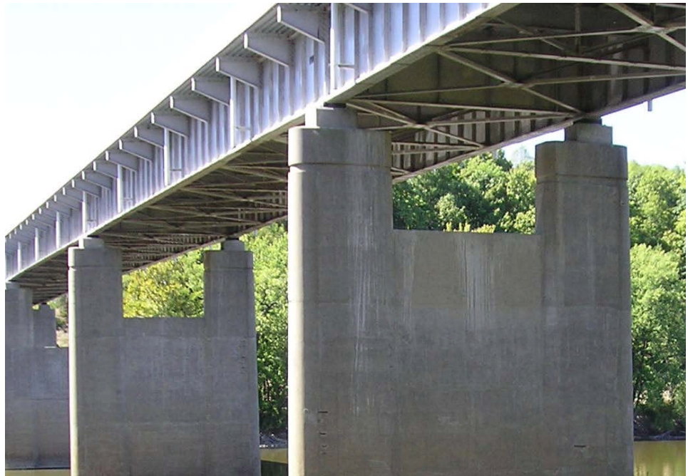
Figure 10.2.1 General View of a Deck Girder Bridge
