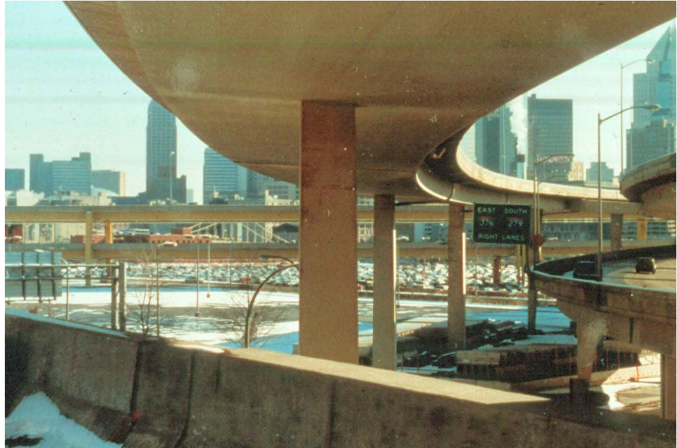
Figure 10.3.3 Box Girders With Multiple Interior Webs
