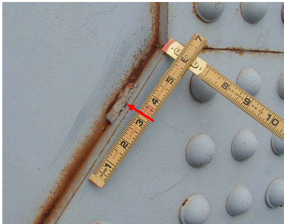
Figure 10.8.26 Partial Length Cracked Tack Weld
