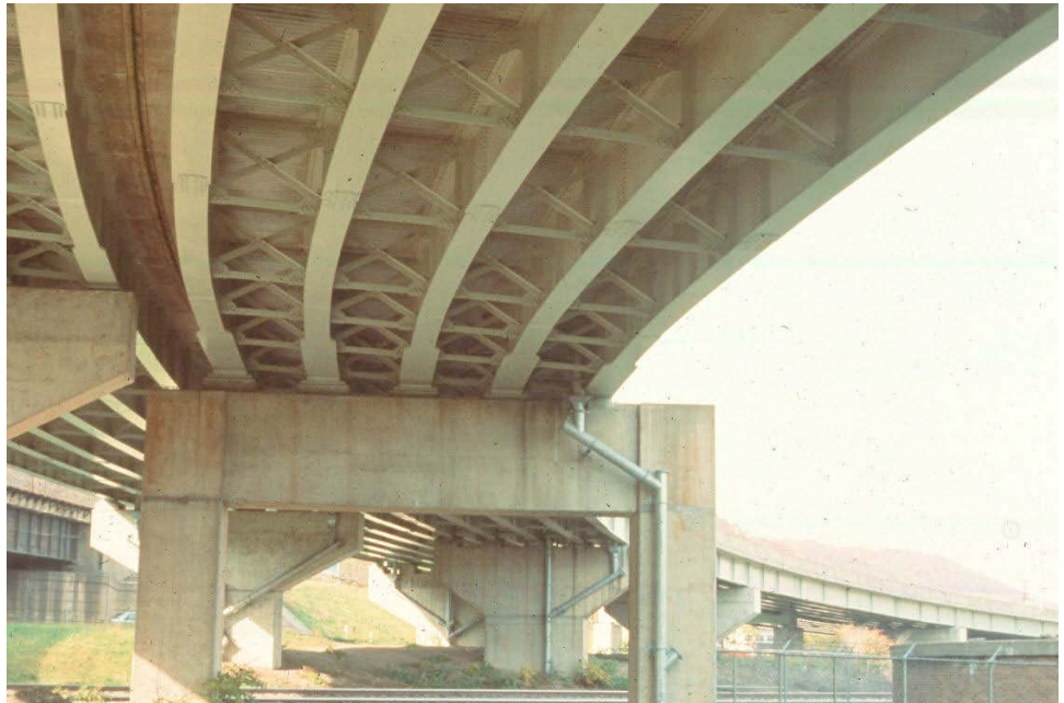
Figure 10.1.8 Curved Fabricated Multi-girder Bridge
