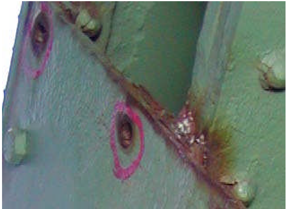
Figure 10.8.29 Missing Bolts on Gusset Plate
