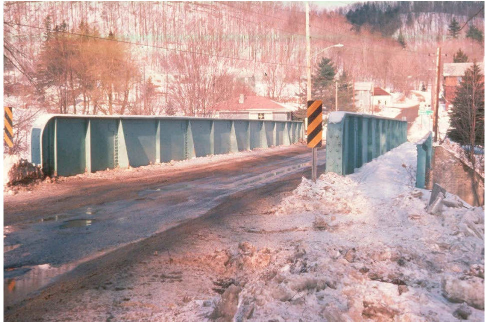
Figure 10.2.2 Through Girder Bridge
