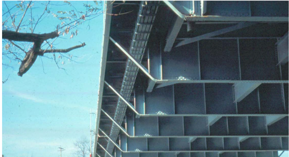
Figure 10.5.18 Floor System on a Through Arch
