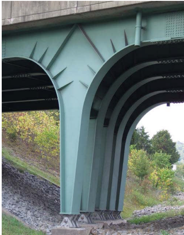
Figure 10.6.2 Typical Rigid Frame Constructed of Multiple Frames
