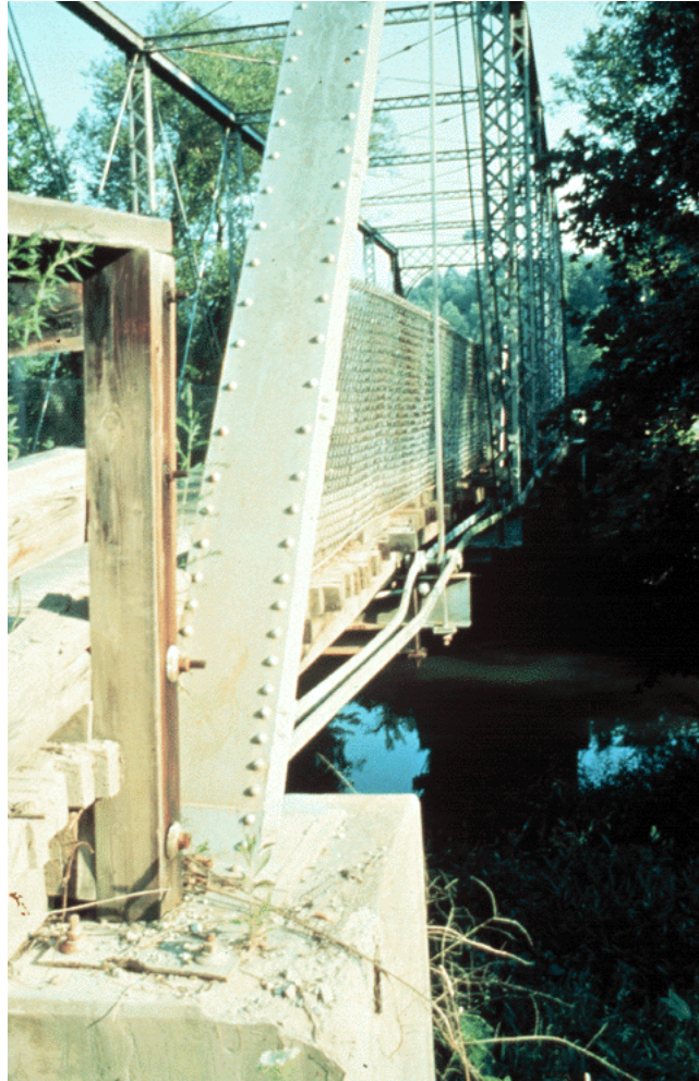
Figure 10.9.22 Buckled Eyebars due to Abutment Movement
