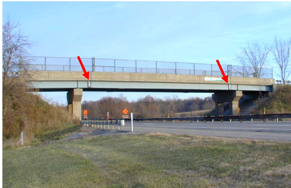
Figure 10.7.3 Pin-and-Hanger Assembly Locations Relative to Piers
