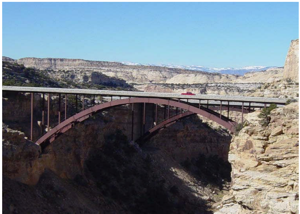
Figure 10.5.5 Solid Ribbed Deck Arch
