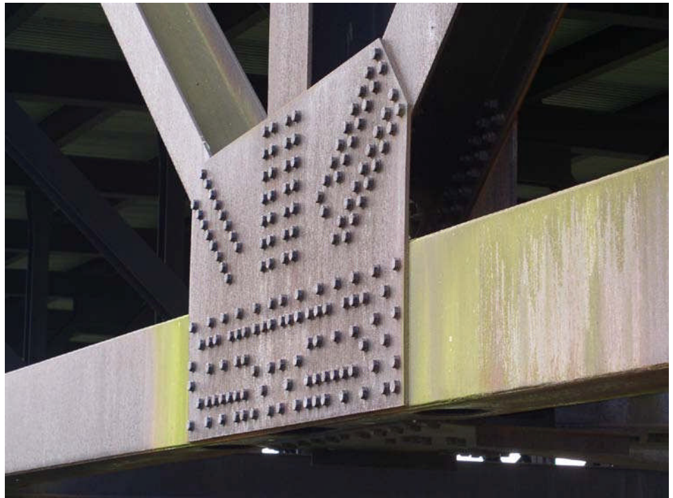
Figure 10.8.8 Gusset Plate Connecting Primary Load-Carrying Truss Members
