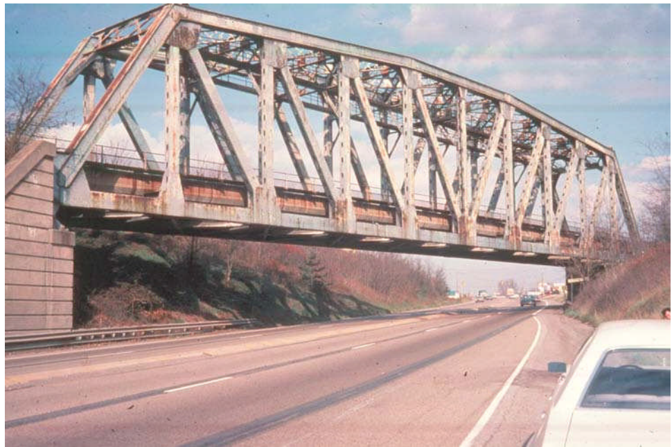
Figure 10.4.1 Simple Span Truss
