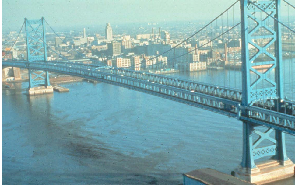
Figure 10.4.6 Suspension Bridge with Stiffening Truss
