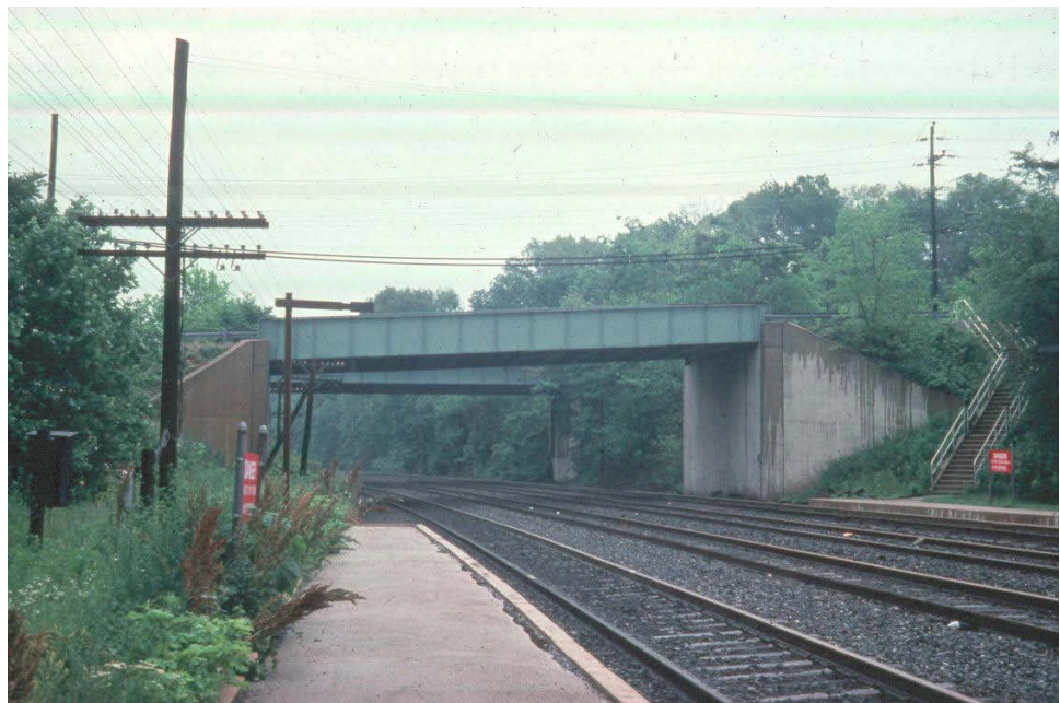
Figure 10.2.3 Through Girder Bridge with Limited Underclearance
