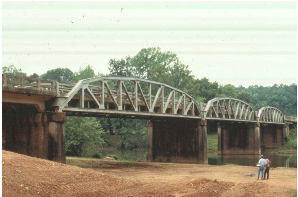
Figure 10.4.12 Multiple Span Pony Truss
