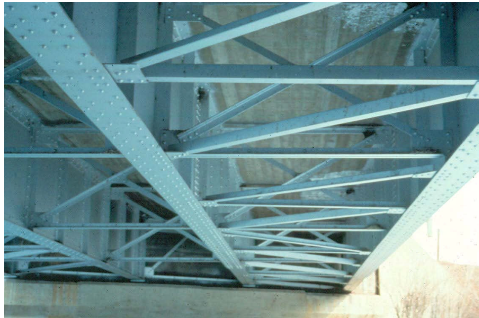
Figure 10.1.15 Straight Multi-Girder Bridge
