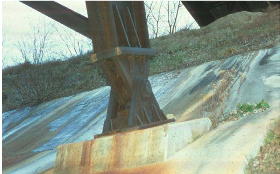
Figure 10.6.13 Bearing Area of a Two Frame Bridge
