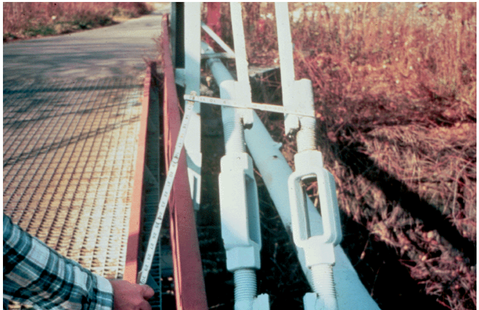
Figure 10.9.29 Welded Repair to Turnbuckles
