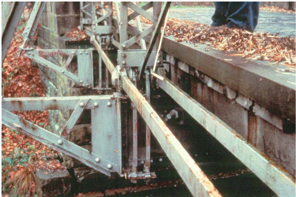
Figure 10.4.45 Bottom Chord with Eyebars
