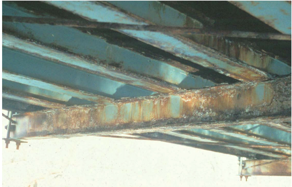
Figure 10.4.55 Corroded Floorbeams and Stringers
