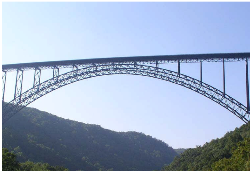
Figure 10.4.7 Deck Arch Bridge with Stiffening Truss
