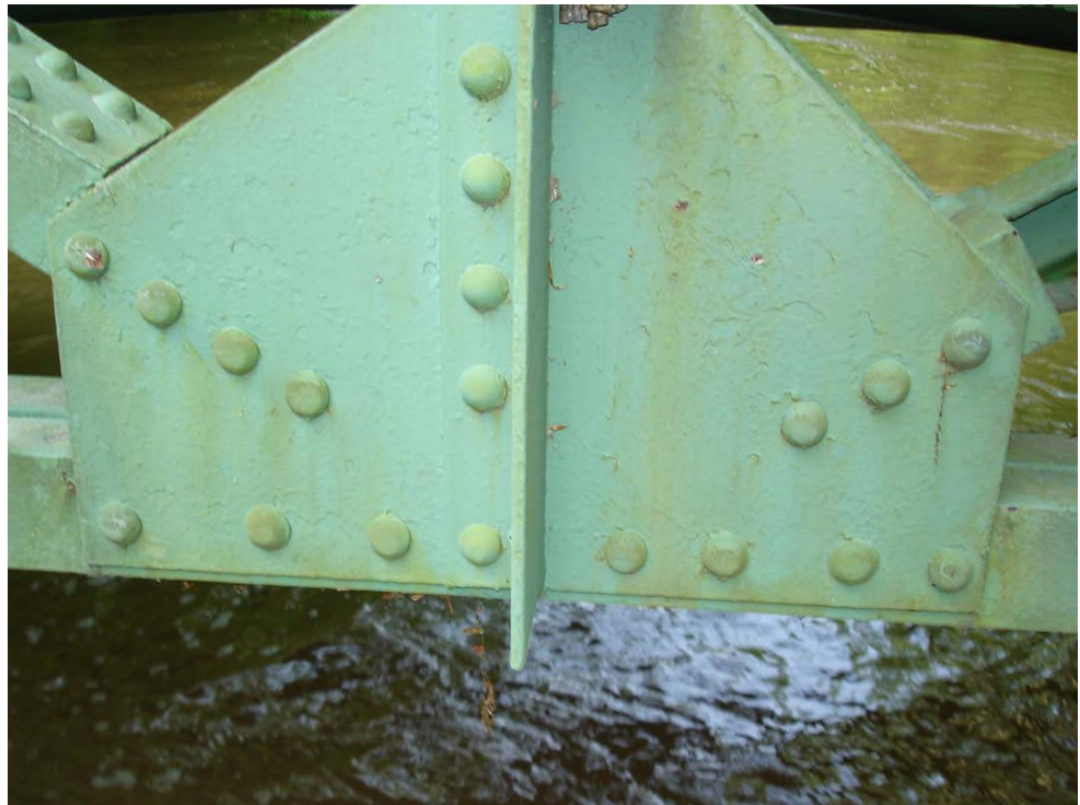
Figure 10.8.3 Steel Gusset Plate with Riveted Connections
