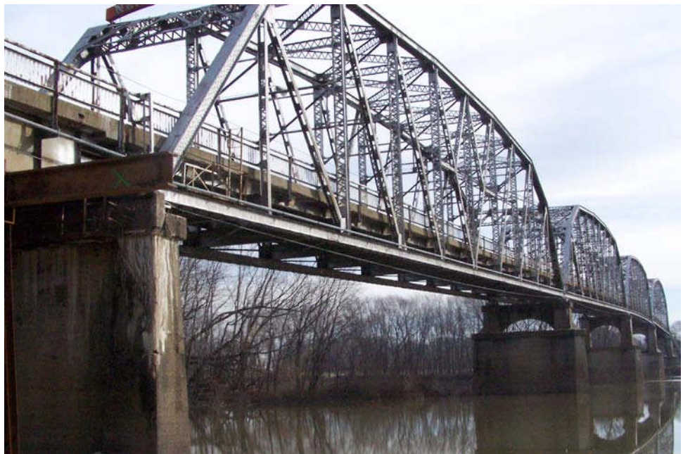
Figure 10.4.13 Multiple Span Through Truss
