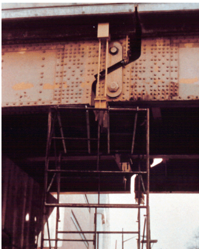
Figure 10.7.18 Alternate Hanger Link Retaining System
