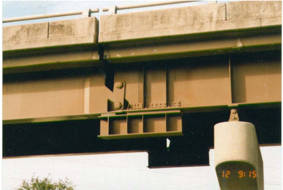
Figure 10.7.25 Underslung Catcher Retrofit
