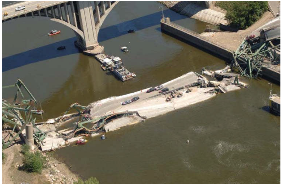
Figure 10.8.34 Collapsed I-35W Mississippi River Bridge
