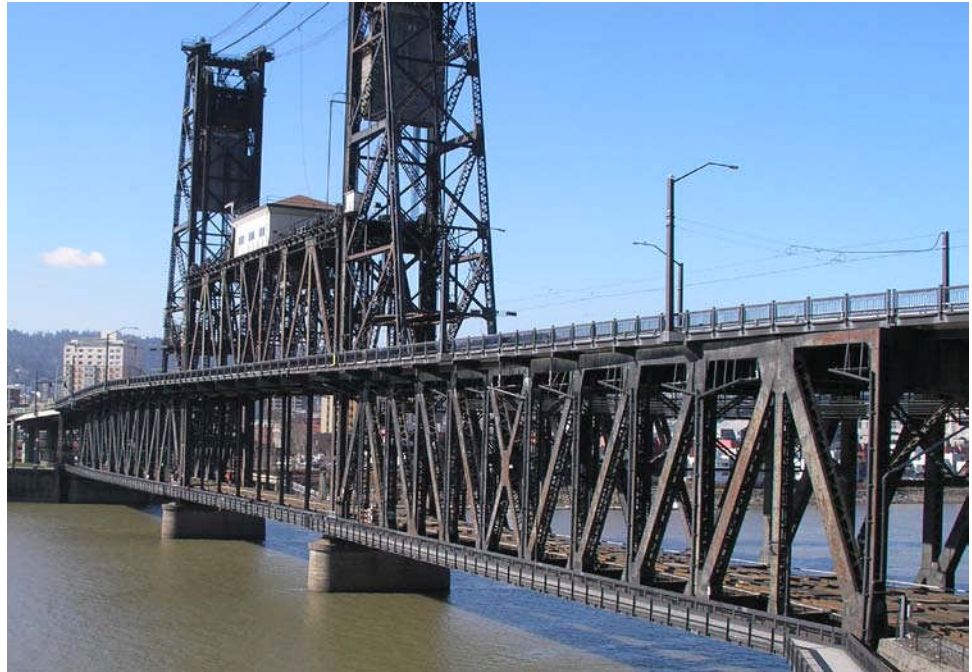
Figure 10.4.8 Vertical Lift Bridge
