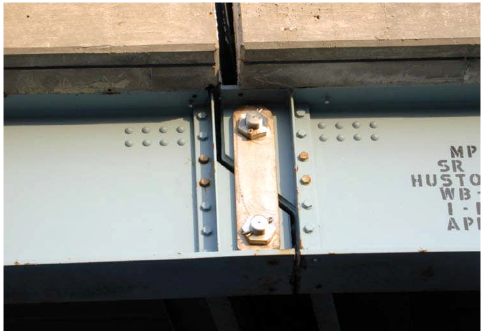
Figure 10.7.26 Stainless Steel Pin-and-Hanger Assembly
