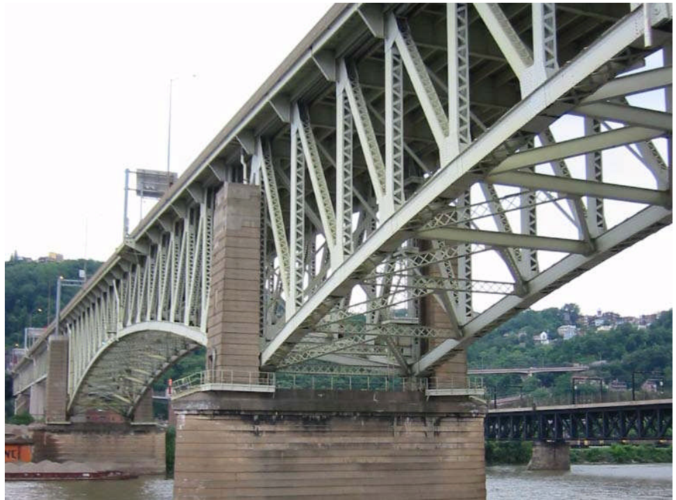
Figure 10.5.23 Bracing Members in Deck Arch Bridge
