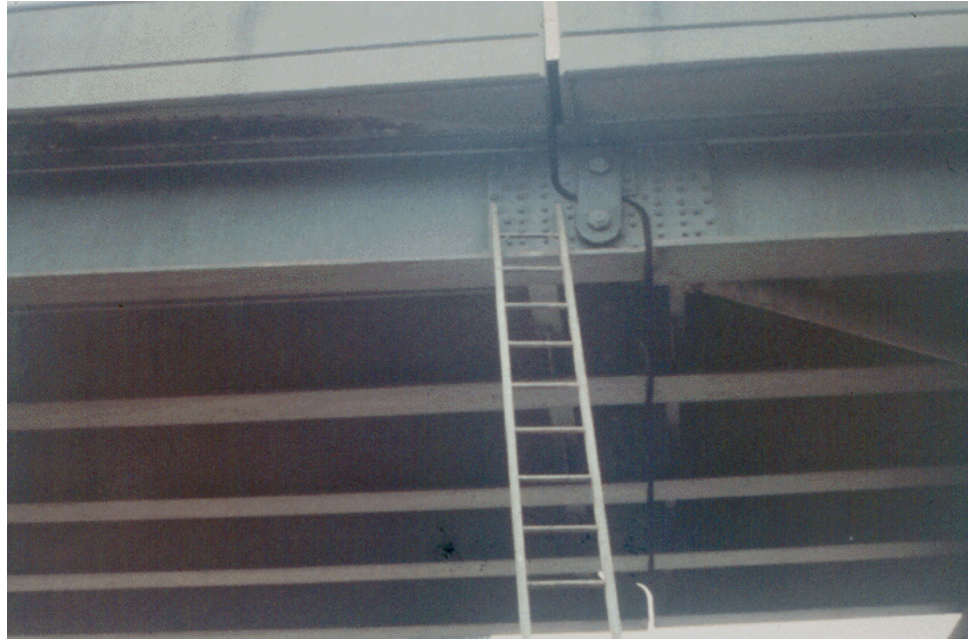
Figure 10.7.16 Multi-girder Bridge with Pin-and-Hanger Assemblies
