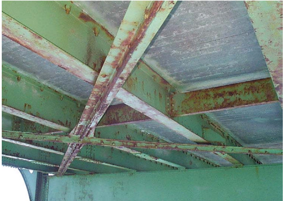
Figure 10.4.57 Lateral Bracing with Corrosion
