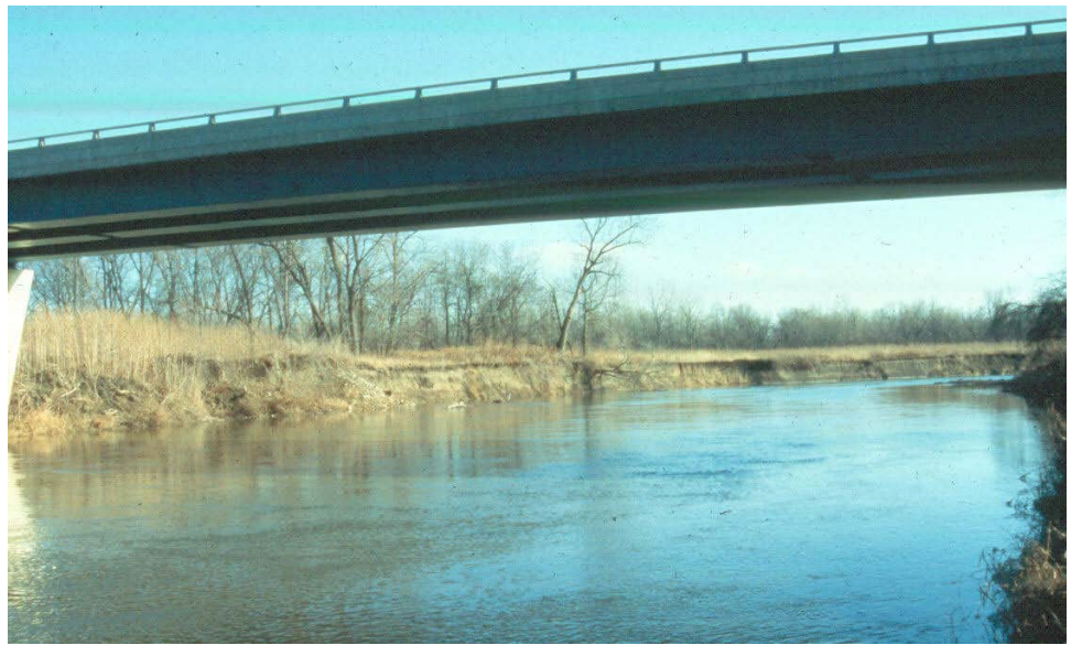
Figure 10.3.1 Simple Span Box Girder Bridge
