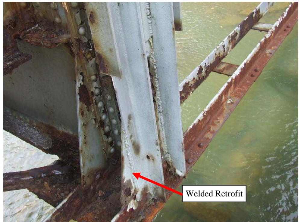
Figure 10.8.31 Poorly Designed Welded Retrofit
