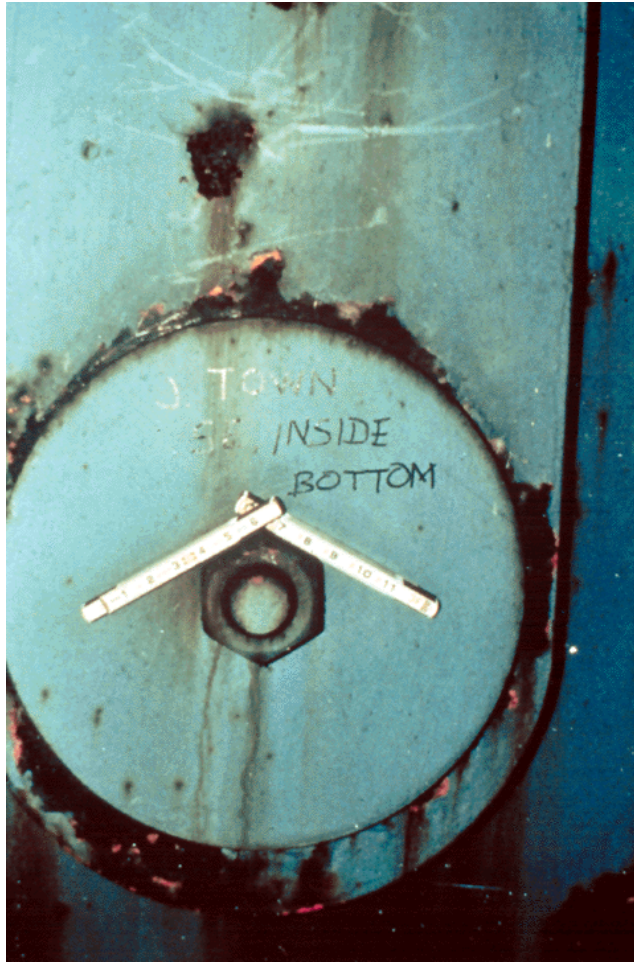
Figure 10.7.8 Pin Cap, Through Bolt and Nut
