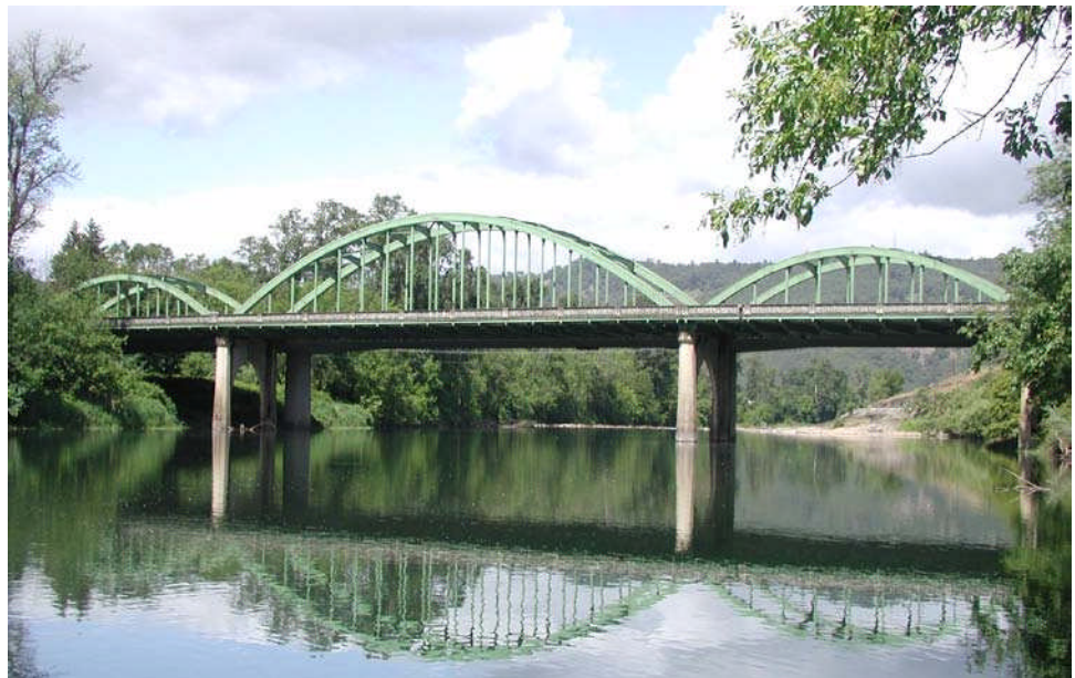
Figure 10.5.14 Three-Span Tied Arch Bridge
