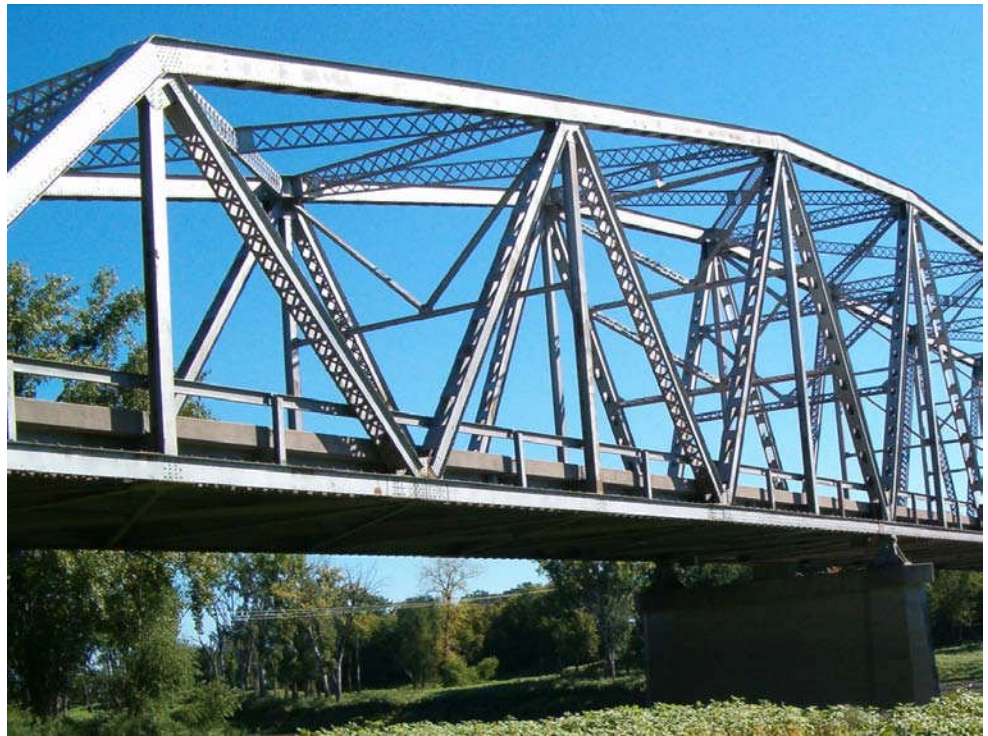
Figure 10.8.1 Steel Truss Superstructure with Gusset Plates
