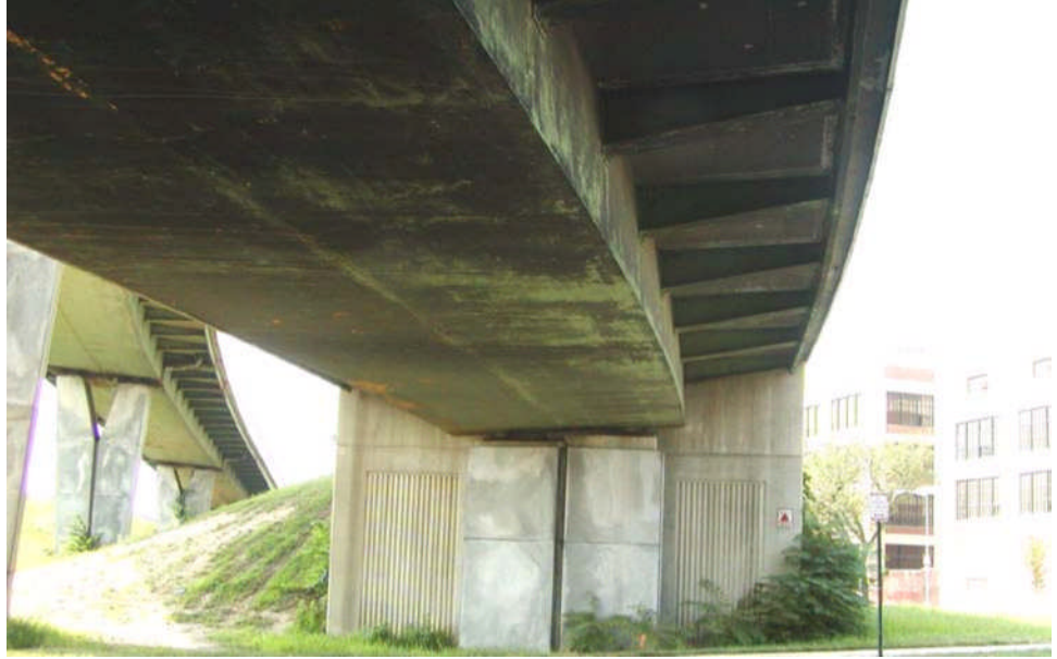
Figure 10.3.12 Non-Redundant Box Girder Bridges
