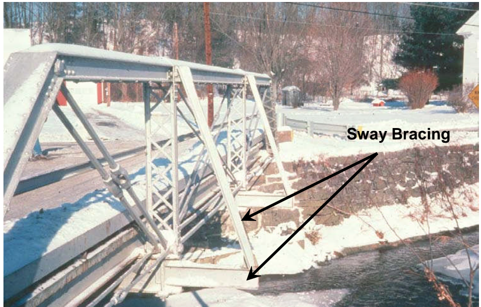
Figure 10.4.39 Pony Truss “Sway Bracing”
