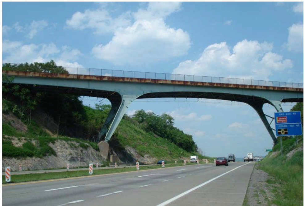
Figure 10.6.1 Typical Rigid K-frame Constructed of Two Frames
