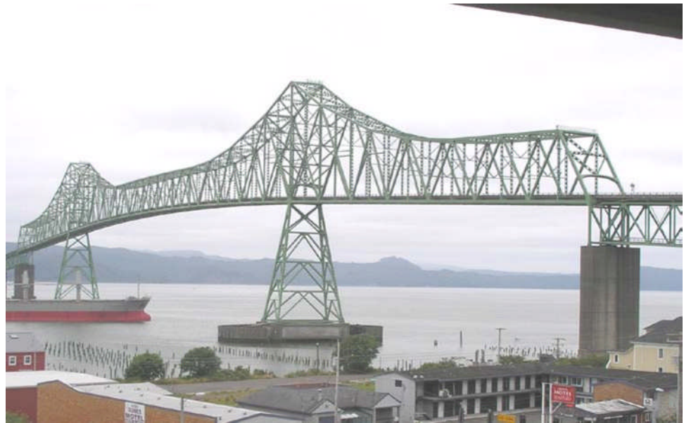
Figure 10.4.3 Through Truss
