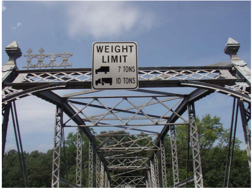
Figure 10.4.38 Portal Bracing with Attached Load Posting Sign
