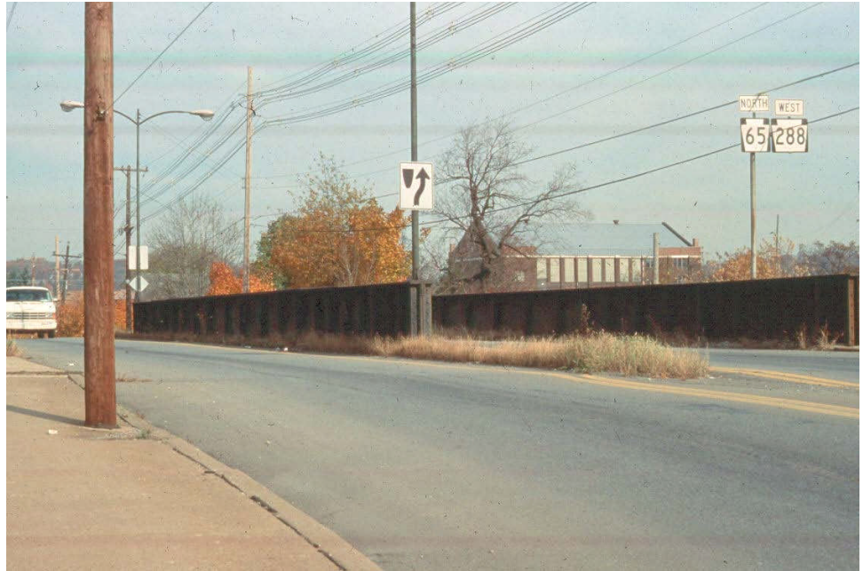
Figure 10.2.4 Through Girder Bridge with Three Girders
