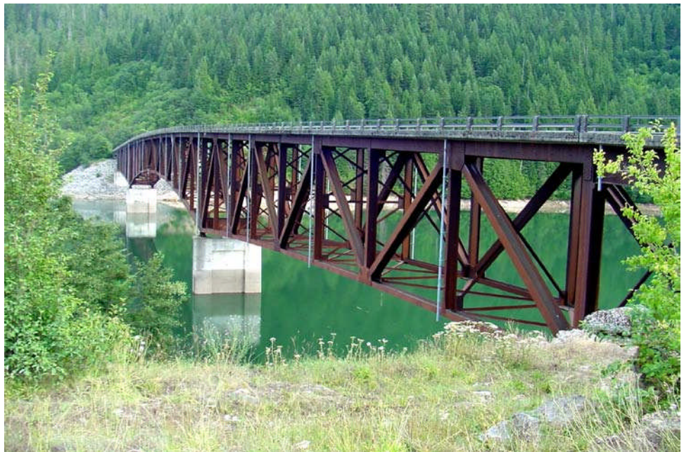
Figure 10.4.5 Deck Truss
