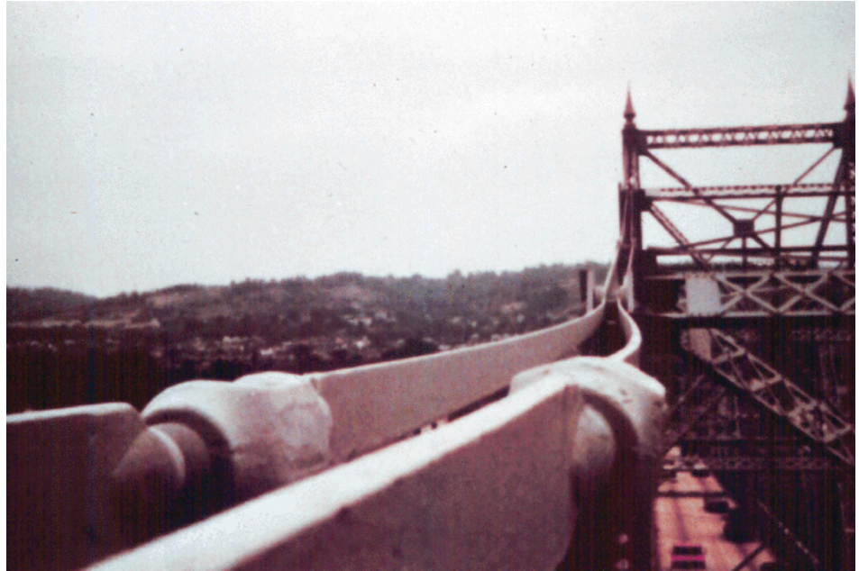
Figure 10.9.21 Bowed Eyebare Member
