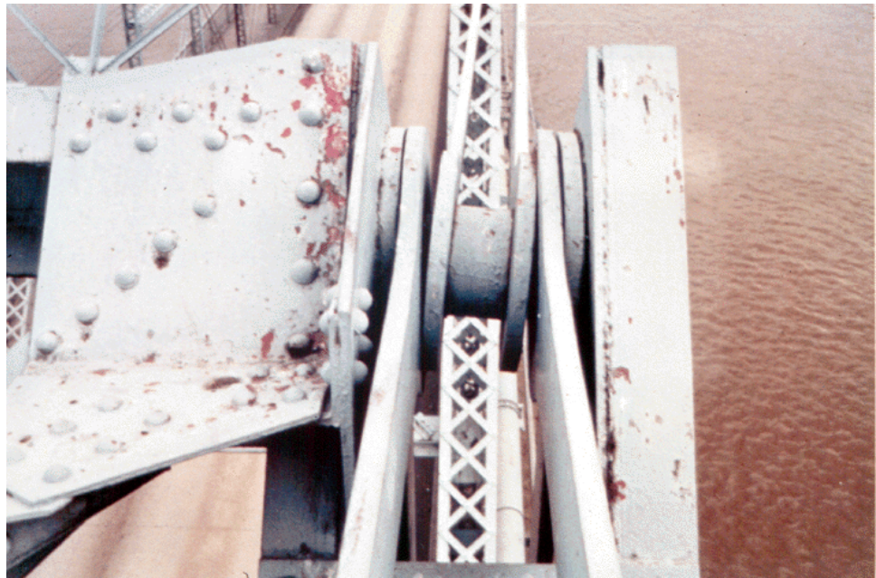
Figure 10.9.24 Asymmetry at an Eyebars Connection
