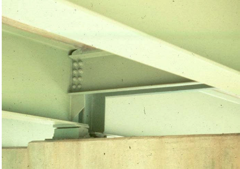
Figure 10.1.21 End Diaphragm
