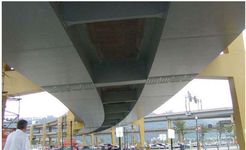
Figure 10.3.4 Spread Box Girders
