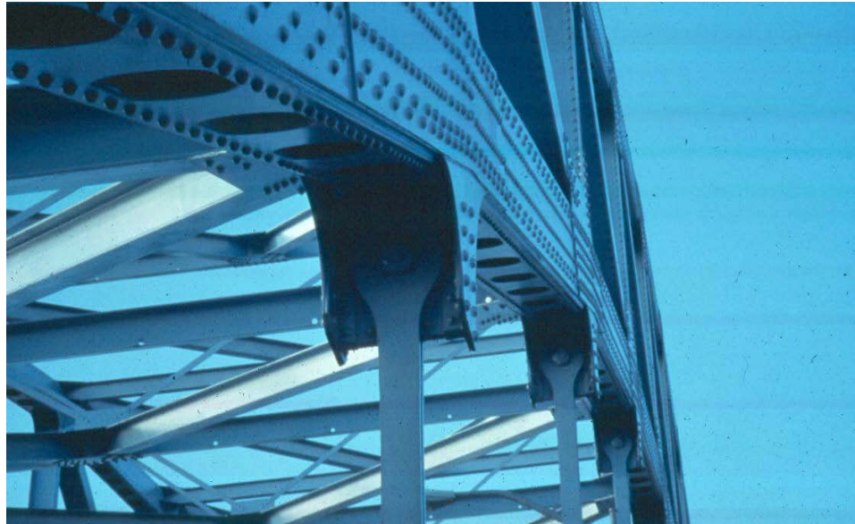
Figure 10.5.21 Hanger Connection on a Through Arch
