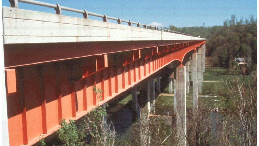
Figure 10.2.13 Flexural Zone on a Two-Girder Bridge
