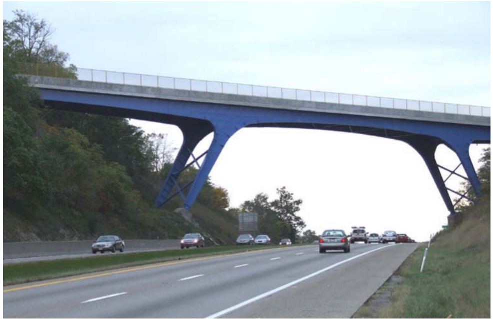
Figure 10.6.11 Fracture Critical Structure - No Load Path Redundancy
