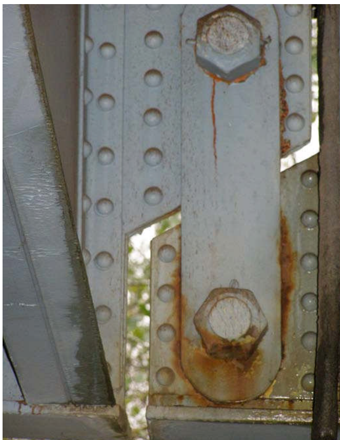
Figure 10.7.20 Rust Stains from Pin Corrosion
