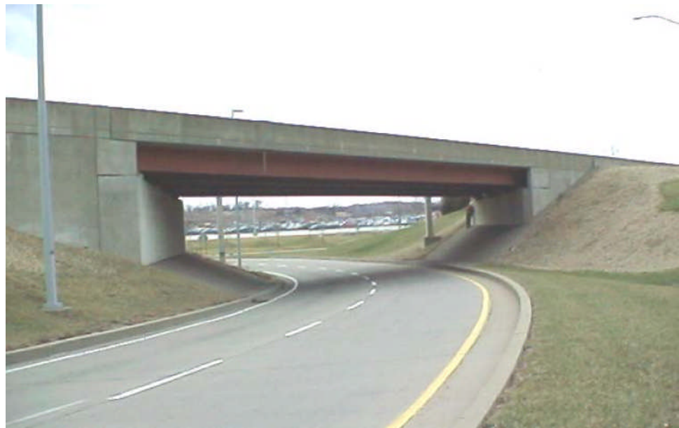
Figure 10.1.6 Single Span Fabricated Multi-girder Bridge
