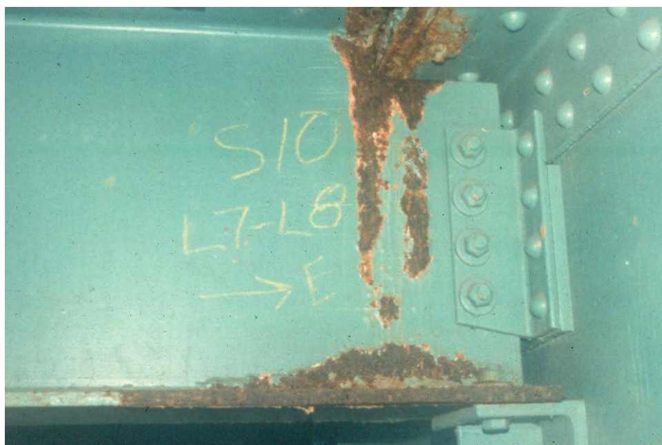
Figure 10.4.54 Corroded End of Stringer
