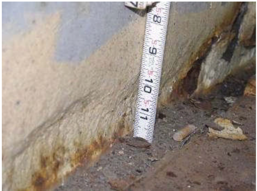
Figure 10.8.21 Inspector Using a Straightedge and Tape to Measure the Section Loss of the Gusset Plate
