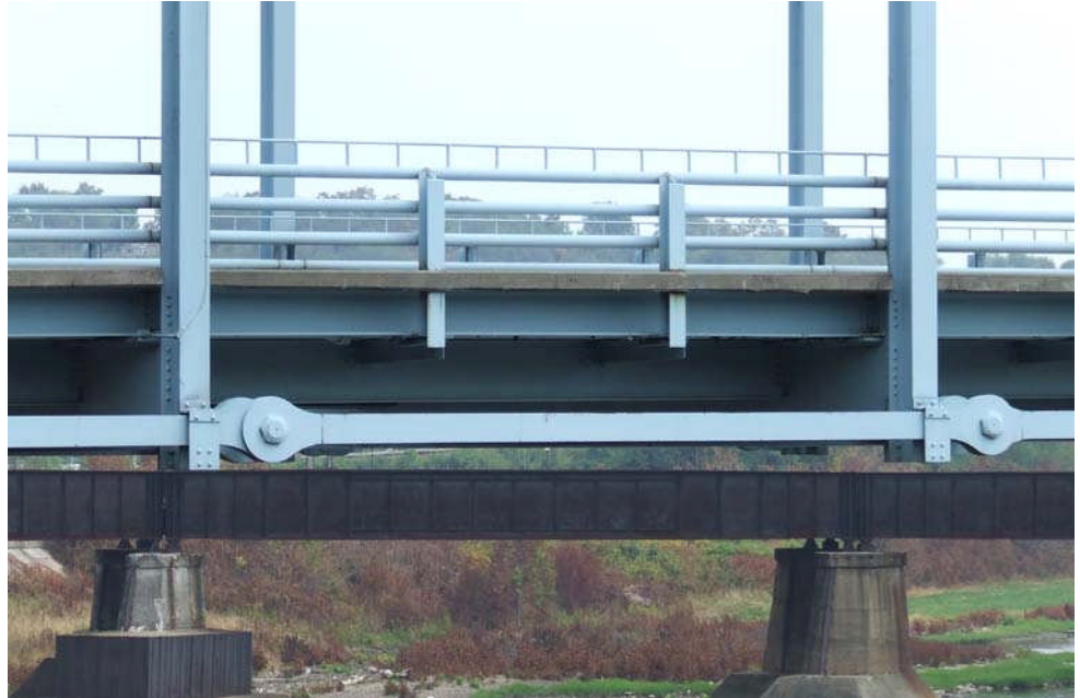
Figure 10.9.1 Typical Eyebare Tension Member on an Arch
