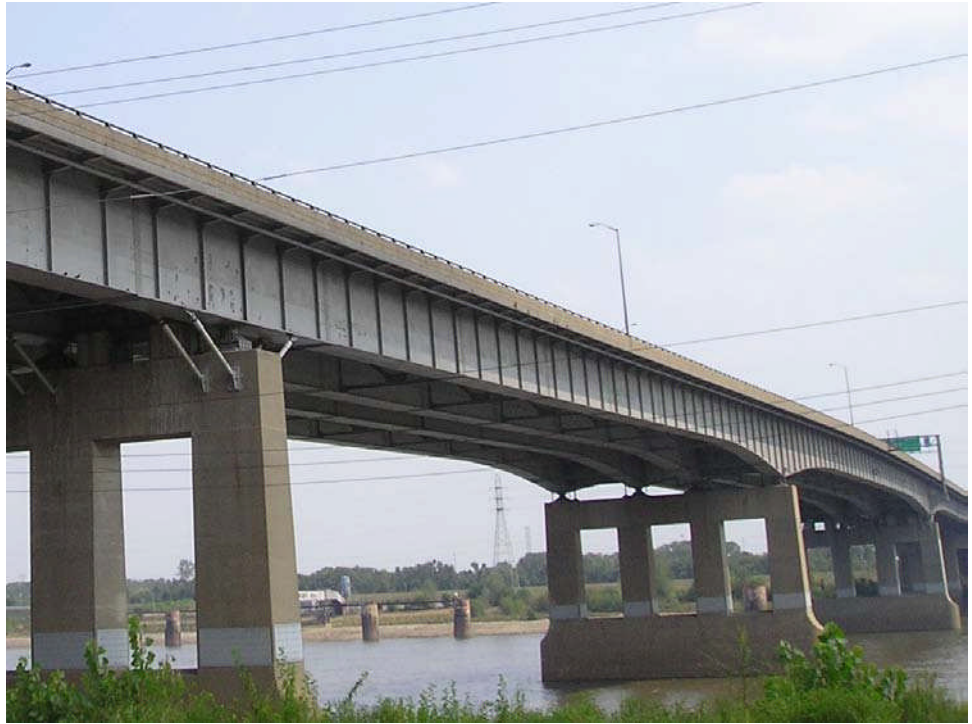
Figure 10.1.7 Continuous Span Fabricated Multi-girder Bridge
