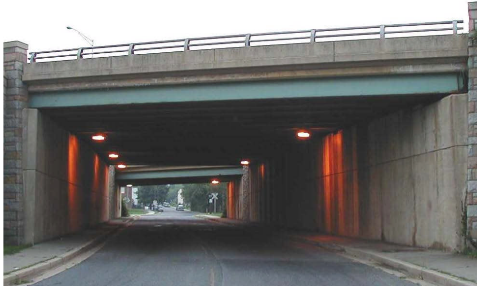
Figure 10.1.1 Simple Span Rolled Multi-Beam Bridge
