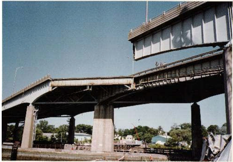
Figure 10.7.15 Mianus River Bridge Failure
