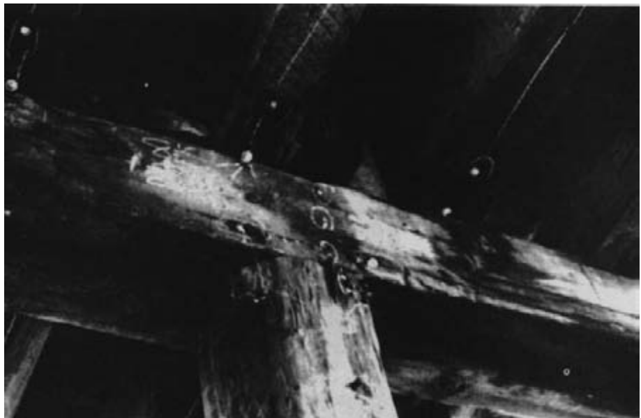
Figure 15-15 - Underside view of an intermediate bent cap after treatment was completed. Holes drilled for treatment application have been plugged with treated-wood dowels.
