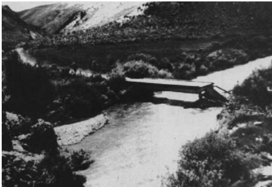
Figure 15-56. - Collapsed span and breached approaches of the existing bridge.
