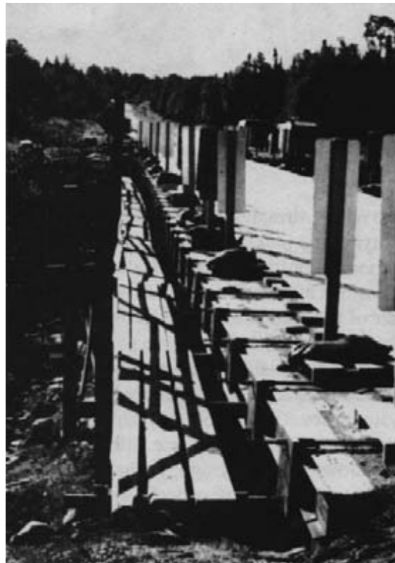
Figure 15-43. - Temporary plank surface placed over prestressing bars during construction at the Pickerel River Bridge.
