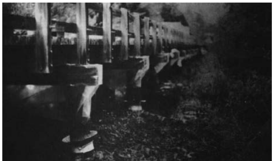
Figure 15-11. - Bridge draping for spillage protection, in place and ready for preservative injection.
