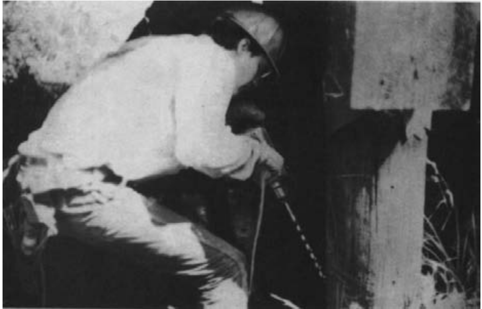
Figure 15-5. - Drilling holes for solid preservative cartridges.
