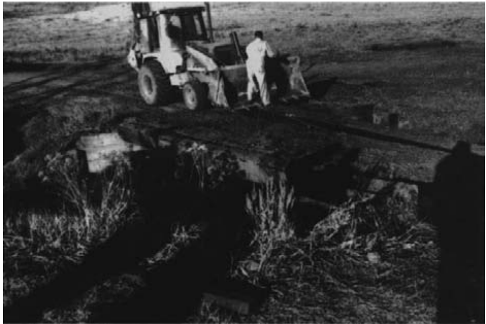
Figure 15-67. - The existing deck was carefully removed in sections to avoid damage to the treated-timber abutment caps.
