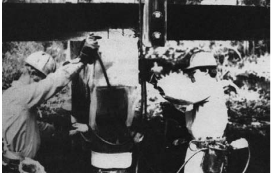
Figure 15-12. - Two-person crew injects liquid wood preservative solution into piles and caps. Note the safety backflow valve on the worker's belt.
