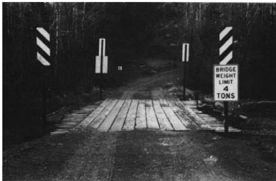
Figure 15-77. - The existing bridge was structurally deficient and load-posted. In addition, it was too narrow and lacked curbs and railing (photo courtesy of Wheeler Consolidated, Inc.).
