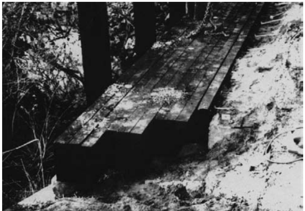
Figure 15-25. - A panel in final position. The ship-lap joint between the deck panel and first plank are interconnected with 5/8-inch-diameter by 13-inch-long drive spikes placed vertically through the joint.
