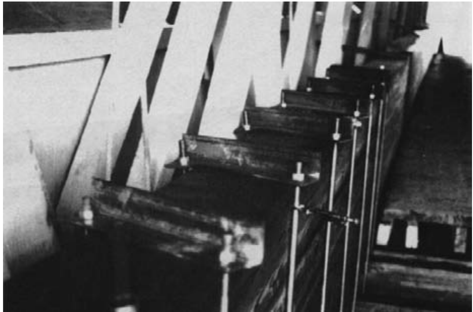
Figure 15-30. - Transverse glulam floorbeams were suspended from the tops of the girders by steel-rod hangers.
