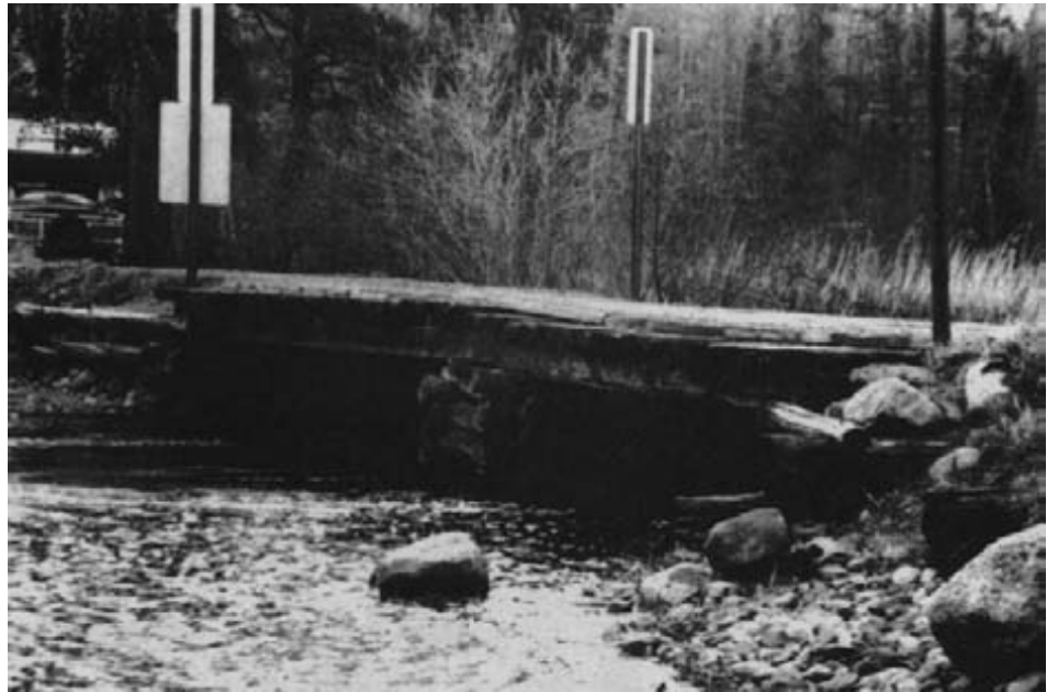
Figure 15-76. - The existing single-lane bridge was a simply supported, two-span, untreated-timber beam bridge supported by log cribbing (photo courtesy of Wheeler Consolidated, Inc.).
