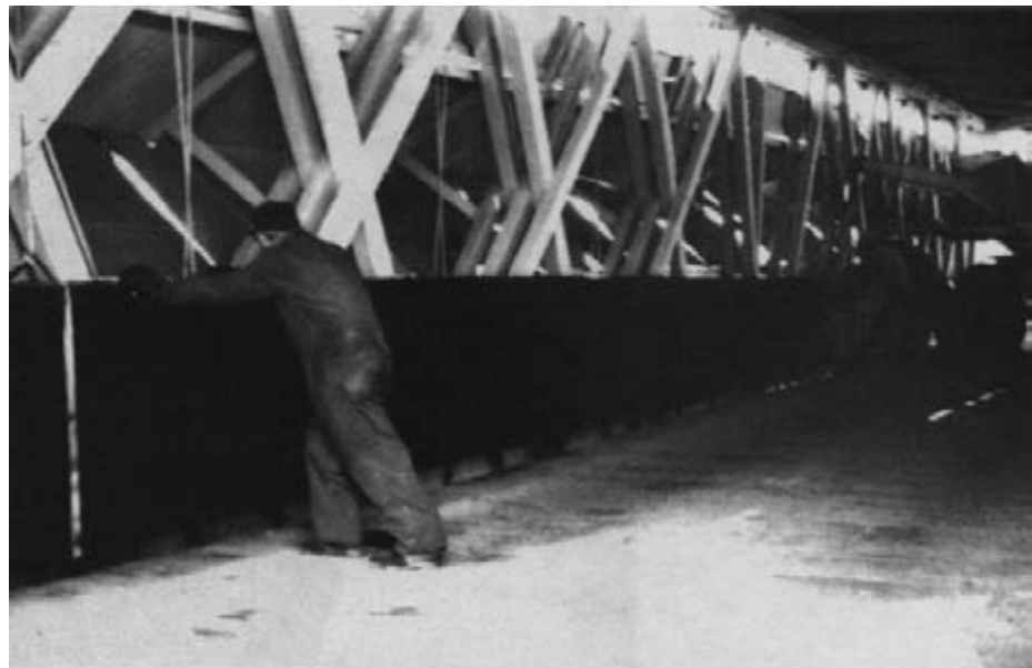
Figure 15-29. - Support for the roadway was obtained by installing two pressure-treated glulam girders inside the existing bridge, one along each side of the roadway.
