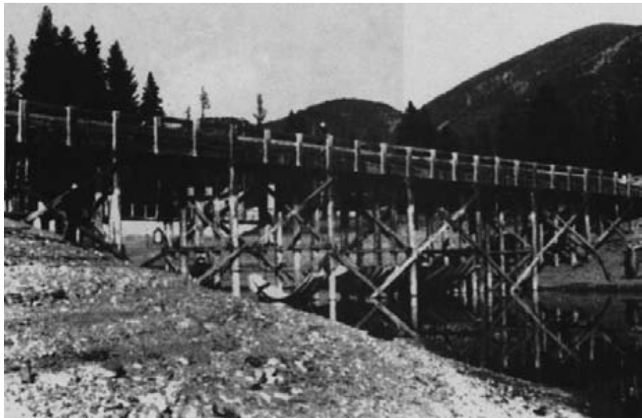
Figure 15-13. - View of the Sullivan Lake Outlet Bridge as in-place treatment was commencing. Note the canvas slings placed under the bridge to prevent water contamination should accidental spillage of treatment chemicals occur.
