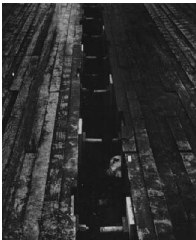
Figure 15-80. - Prestressing rods protruding from the two prefabricated deck panels before connection. The rod opposite each coupler was released and threaded into the coupler. After all couplings were made, the released rods were restressed, causing the deck panels to be stress-laminated together as an integral bridge deck.
