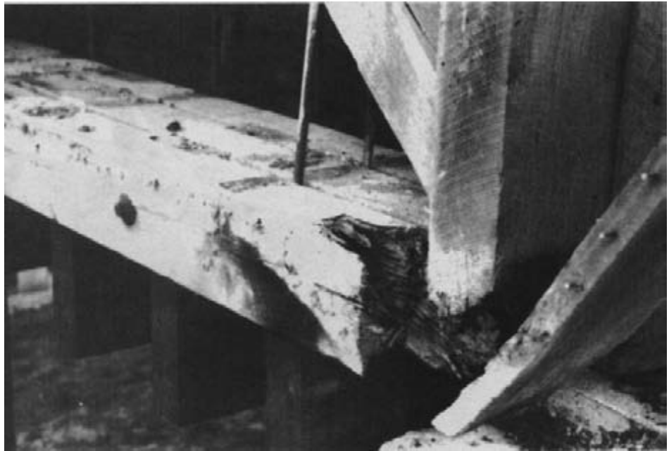
Figure 15-32. - Severe deterioration at each corner of the bridge was one cause of the poor truss alignment. New floorbeams were extended beyond the girders to help support each truss.
