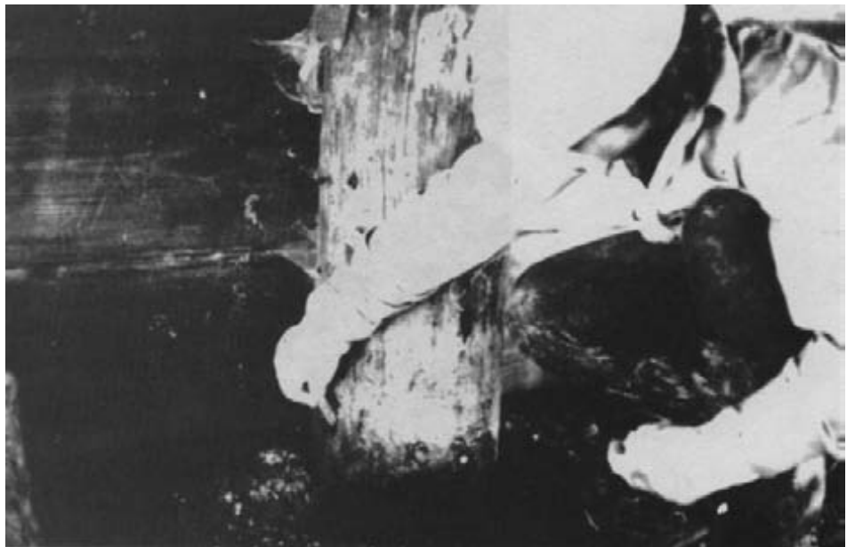
Figure 15-6 - Insertion of solid preservative cartridges into a timber pile. Note the use of rubber safety gloves.
