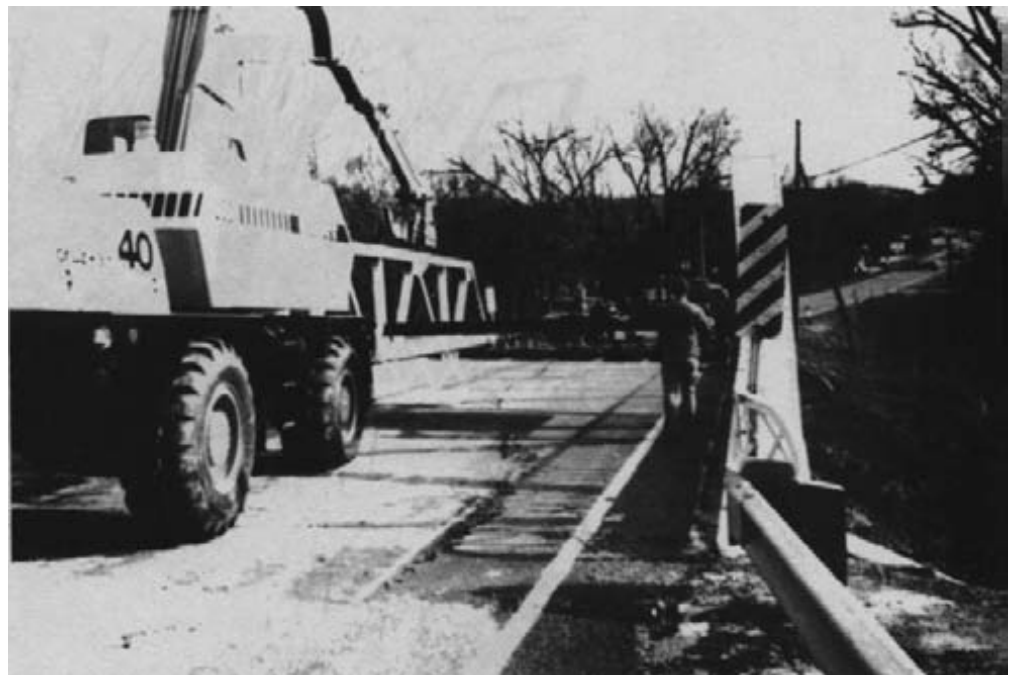
Figure 15-50. - New, prefabricated treated-timber deck panels were placed with a hydraulic excavator. The panels were designed to fit transversely on the stringers and were placed without removing the existing railing.
