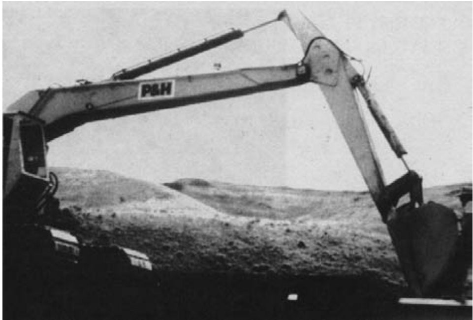
Figure 15-64. - Backhoe pushes panels together after dowels have been aligned. A large timber block was placed across the panel edge to prevent damage from the backhoe bucket.
