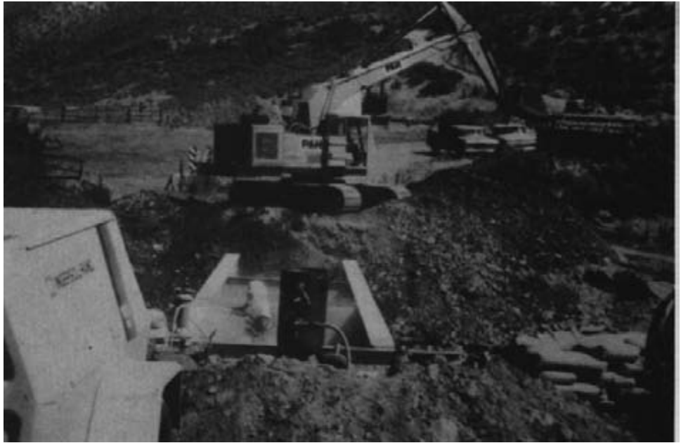
Figure 15-60. - Blast cleaning of the existing steel work in preparation for painting, while a backhoe removes material that was placed for the temporary repair.
