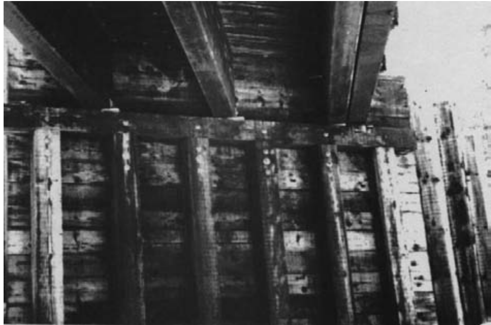
Figure 14-21. - A sister member in a glulam beam superstructure. The outside beam, which was damaged by a vehicle overload, could not be easily replaced. The sister member was added along the outside of the beam to restore the capacity to the structure.
