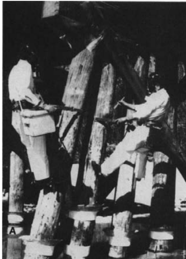
Figure 14-9. - Application of liquid fumigants. (A) Liquid fumigants applied with commercial equipment (photo courtesy of Osmose Wood Preserving, Inc.).
