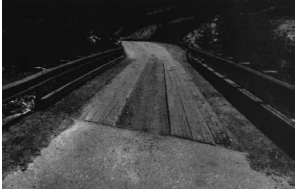
Figure 14-2. - Dirt and debris on the deck surface can trap moisture and lead to premature deterioration. Material such as this should be removed periodically as part of a good preventative maintenance program.
