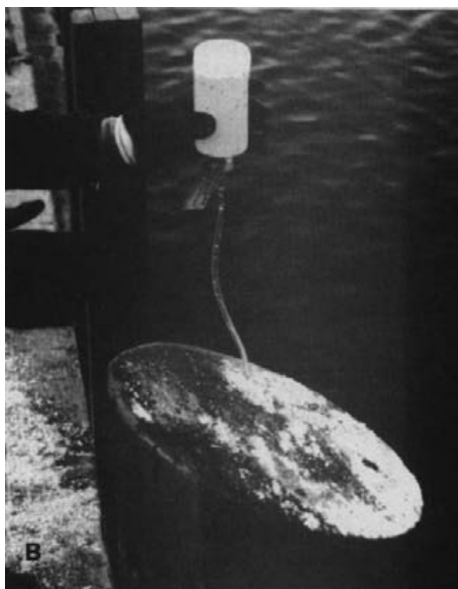
Figure 14-9. - Application of liquid fumigants (continued). (B) Liquid fumigants applied from a polyethylene squeeze bottle (photo courtesy of Jeff Morrell, Oregon State University).
