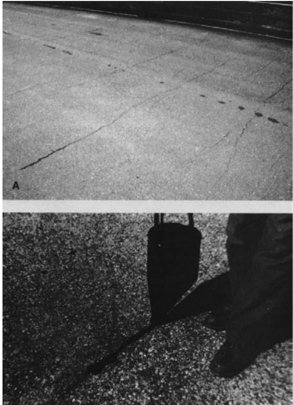
Figure 14-4. - (A) Minor cracking in an asphalt wearing surface from differential deck deflections. (B) Sealing the cracks with an asphalt emulsion slurry.
