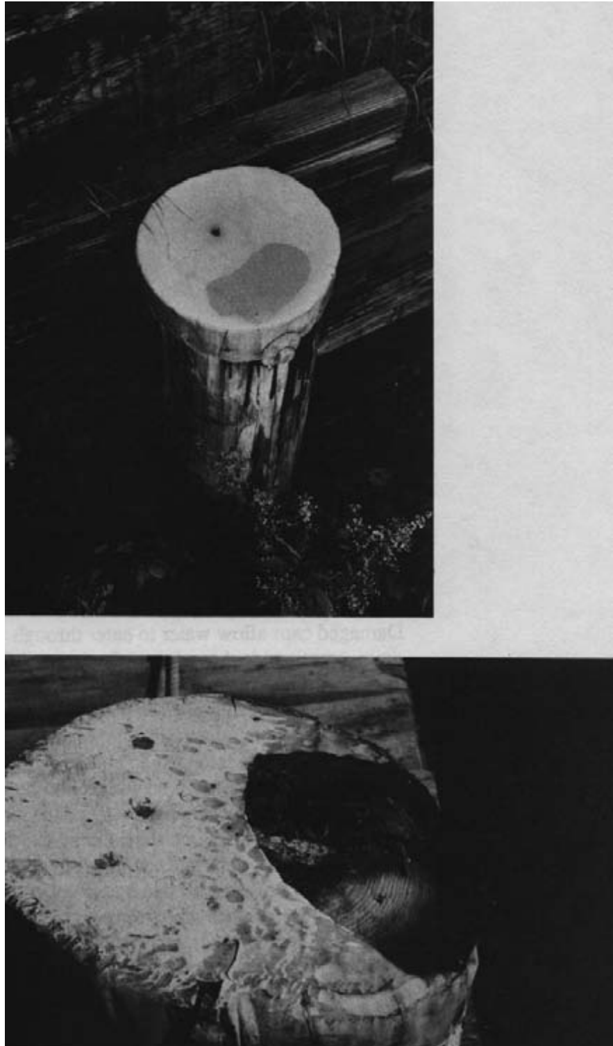
Figure 13-42. - (Top) Damaged metal pile caps allow water to enter, but restrict air circulation and drying. (Bottom) Pile decay is exposed when the damaged cap is removed.
