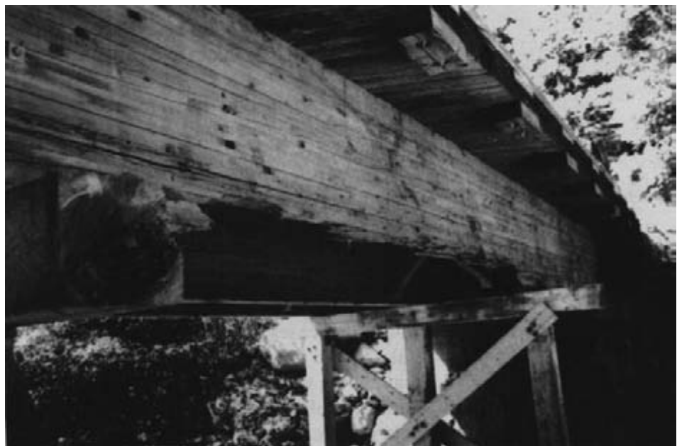
Figure 13-19. - Severe mechanical damage to a glulam bridge caused by debris flow during high stream levels.
