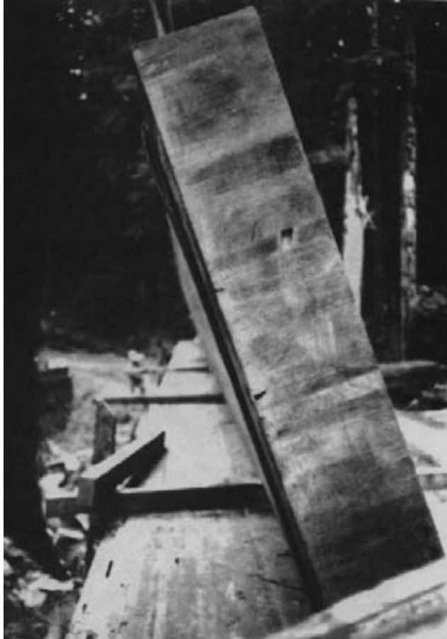
Figure 12-7. - A large glulam bridge beam is tipped from its horizontal storage position before being lifted into place on edge (photo courtesy of Tim Chittenden, USDA Forest Service).
