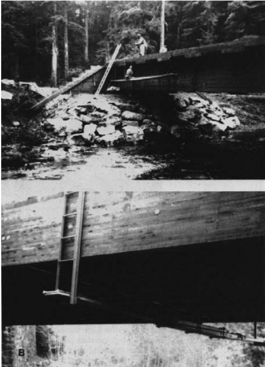
Figure 12-12. - Typical scaffolding configurations for accessing the underside of a glulam beam bridge. (A) Along the deck overhang (photo courtesy of Tim Chittenden, USDA Forest Service). (B) Between beams (photo courtesy of Western Wood Structures, Inc.).
