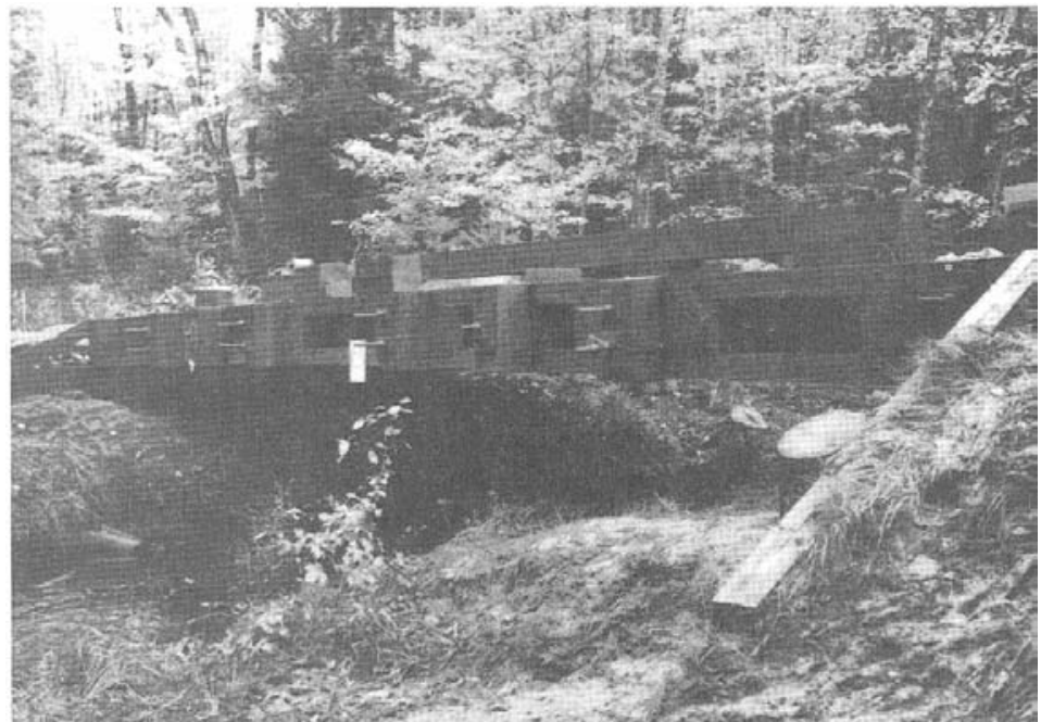
Figure 9-6. - (Top) Drawing of a stress-laminated parallel-chord truss. (Bottom) Prototype stress-laminated parallel-chord bridge built on the Hiawatha National Forest (shown during construction).
