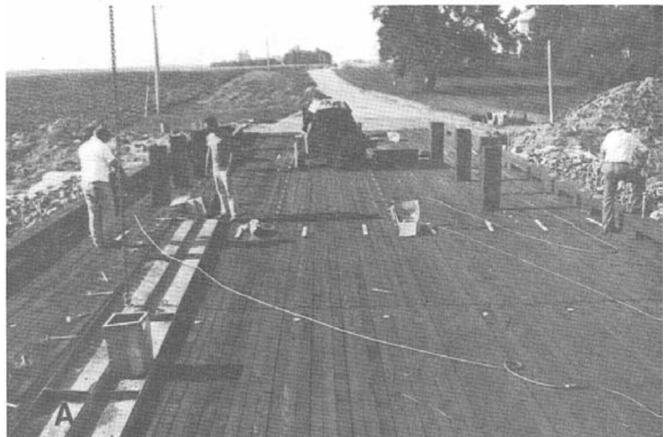
Figure 8-12. - Panelized longitudinal nail-laminated deck bridges. (A) During construction. (photos courtesy of Wheeler Consolidated, Inc.).
