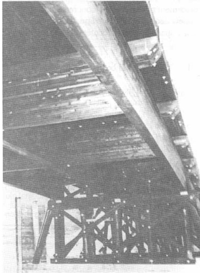
Figure 8-19. - Longitudinal glulam deck on transverse glulam floorbeams.
