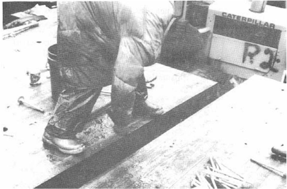
Figure 7-28. - Bituminous sealer is spread on the edges of glulam deck panels to waterproof the panel joints.
