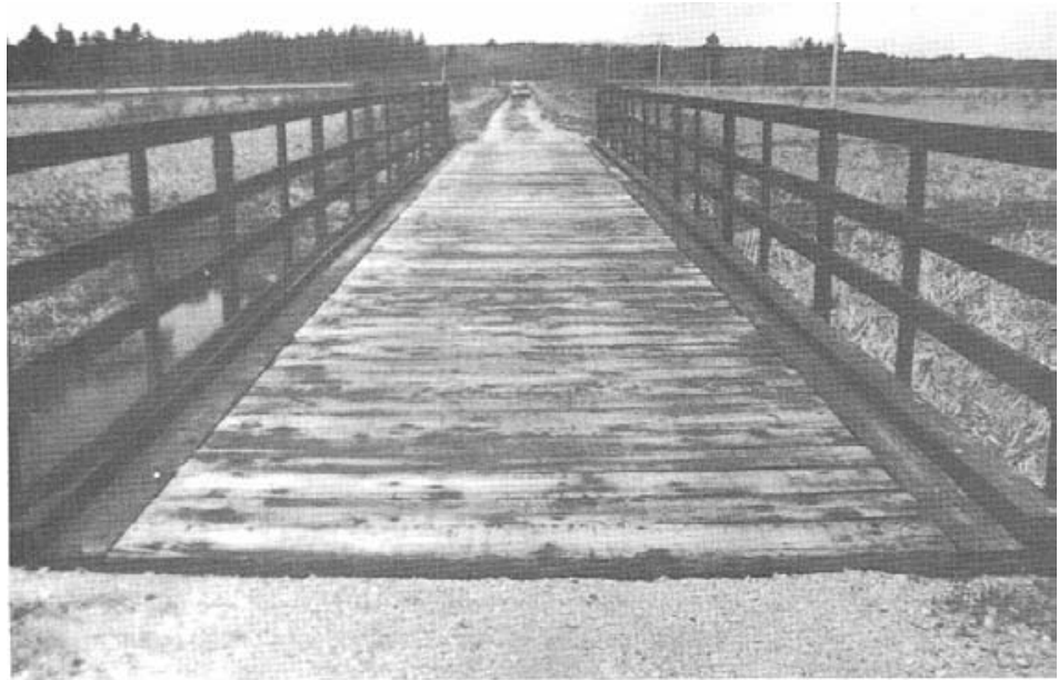
Figure 7-41. - Transverse plank deck on a single-lane, low-volume road (photo courtesy of Wheeler Consolidated, Inc.).
