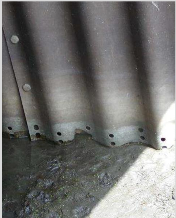
Condition State 4 Failed seam on an aluminum box culvert
