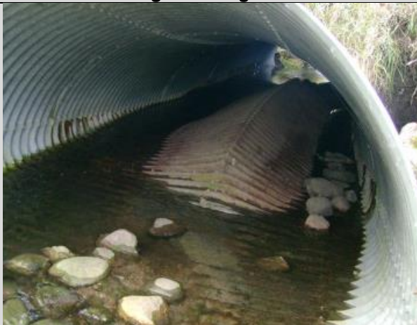
Condition State 4 Severe barrel distortion
