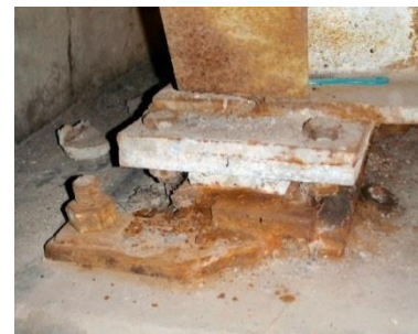
Corroded (possibly frozen) sliding plate bearing
