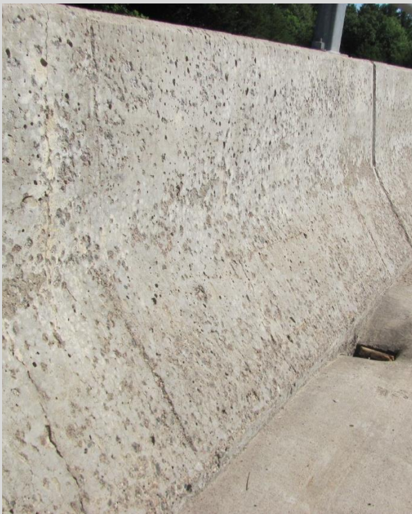
Condition State 2 Scale on a concrete J-barrier
