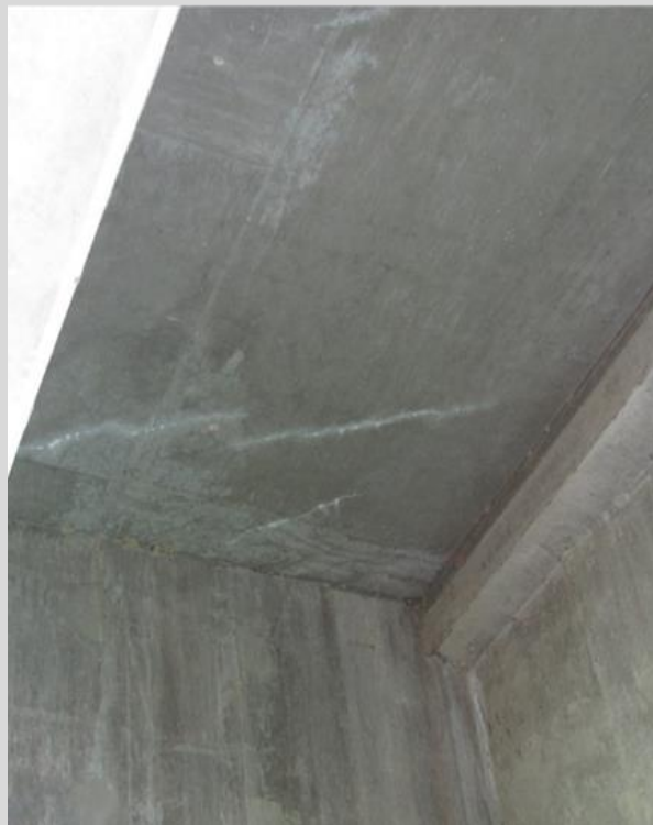
Condition State 2 Diagonal crack on the underside of a concrete deck with light leaching (efflorescence)
