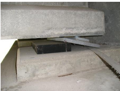
Severe malfunction of an elastomeric bearing
