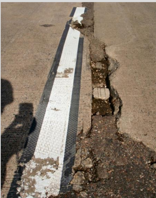
Condition State 4 Severe spall along centerline of a concrete approach panel
