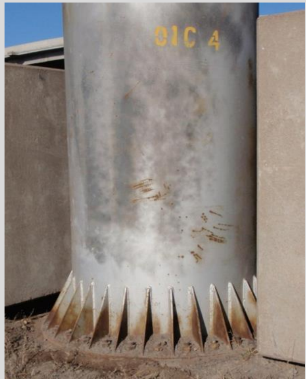
Condition State 2 Paint failure and surface corrosion on a steel column
