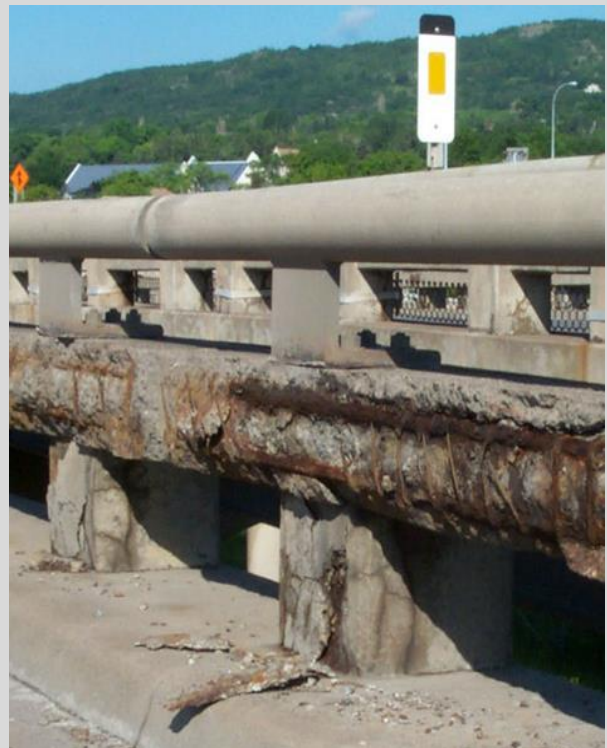
Condition State 4 Severe spalling on the concrete rail base of a combination railing
