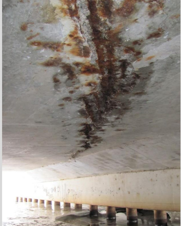
Condition State 4 Severe spalling (more than 3" deep) on the underside of a concrete deck
