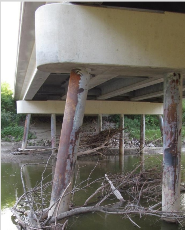
Condition State 2 Paint failure and surface corrosion on a CIP Pile
