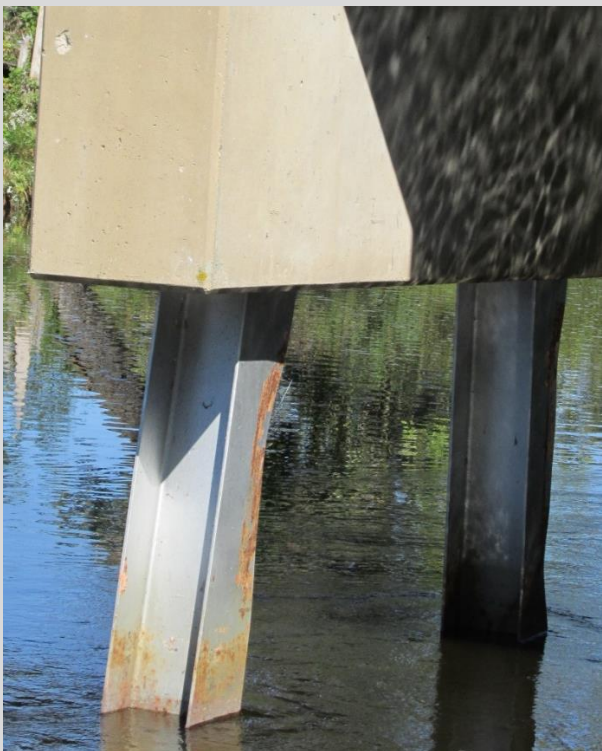
Condition State 2 Impact damage (bent flange) on a steel H-pile
