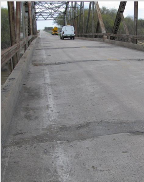
Condition State 4 Extensive deck deterioration (bituminous patching) along transverse poured deck joints
