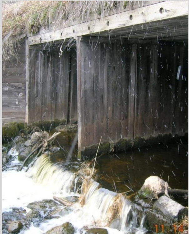
Condition State 2 Evidence of decay along the waterline of a timber box culvert
