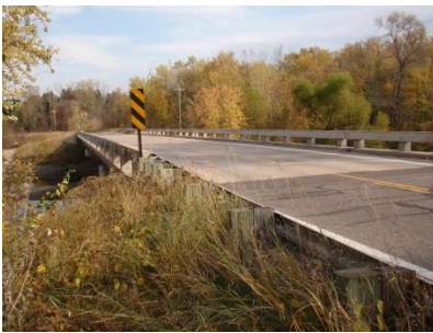
1. Roadway across Bridge
