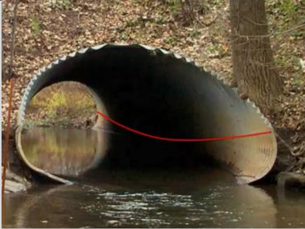
Condition State 3 Significant longitudinal deflection
