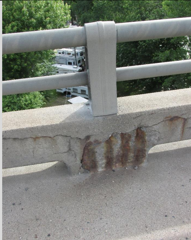
Condition State 3 Spalling (exposed rebar) on the concrete parapet of a combination railing
