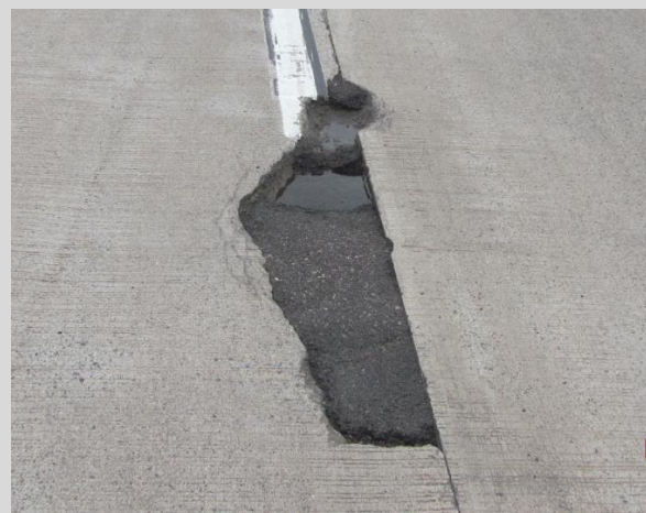
Condition State 4 Failed bituminous patch on a low slump overlay
