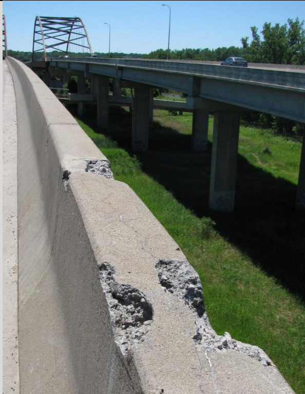
Condition State 3 Spalling/scaling along the top of a concrete J-barrier
