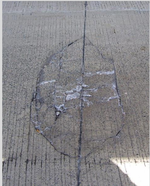
Condition State 4 Cracking and delamination adjacent to a transverse poured deck joint
