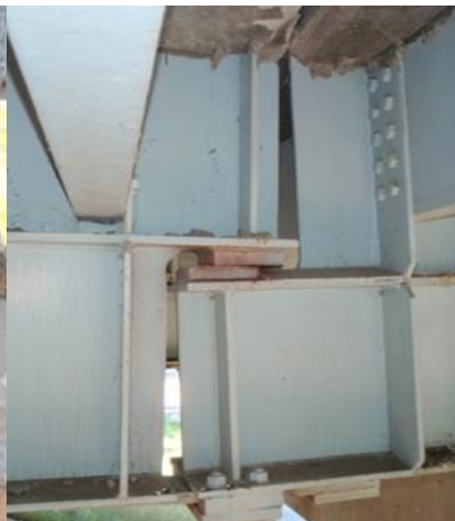
Misaligned hinge bearing
