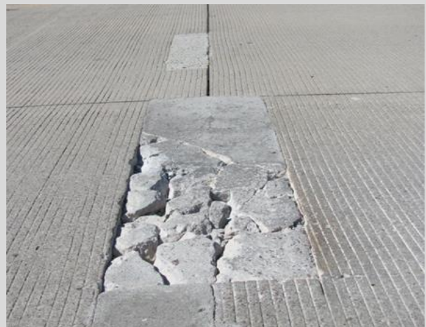
Condition State 4 Failed patch on low slump concrete overlay
