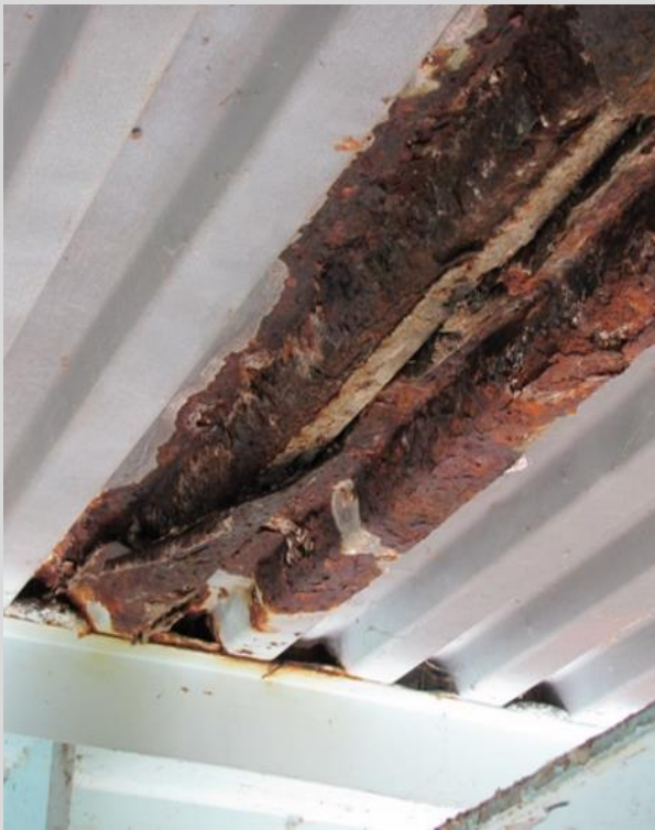
Condition State 3 Steel stay-in-place forms on underside of concrete deck rusted through
