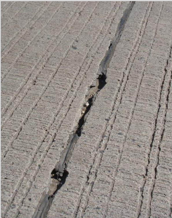
Condition State 3 Section of poured seal missing
