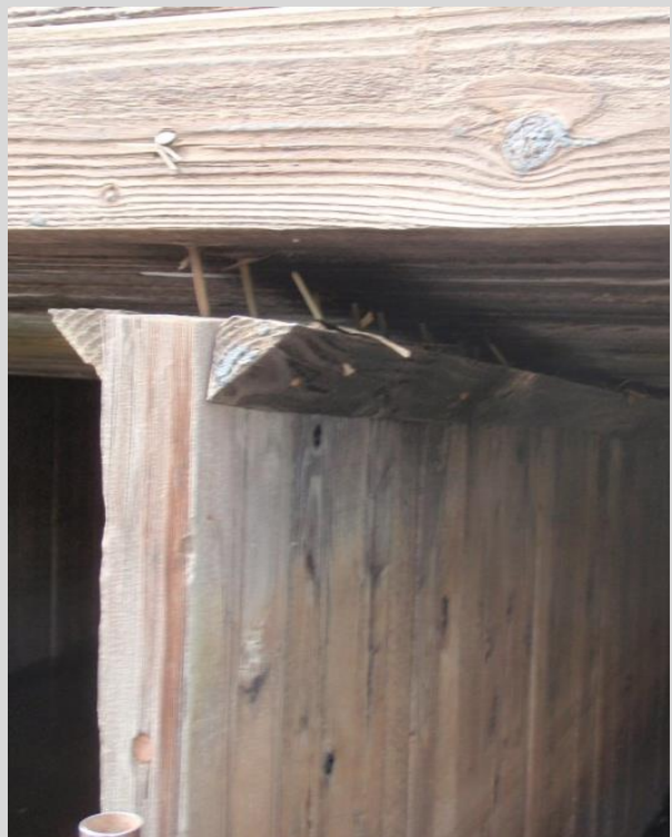
Condition State 4 Separation (connection failure) between wall and ceiling on a timber box culvert
