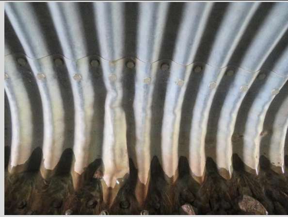
Condition State 4 Severe buckling of corrugations in sidewall
