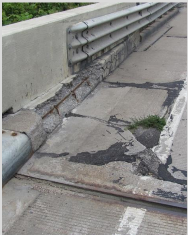
Condition State 4 Concrete approach panel fractured at the corner
