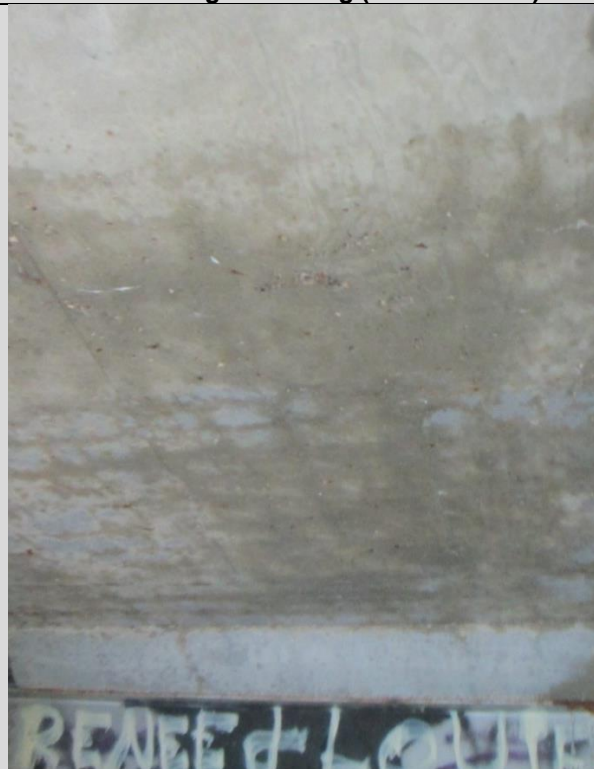
Condition State 2 Light water saturation on the underside of a concrete deck
