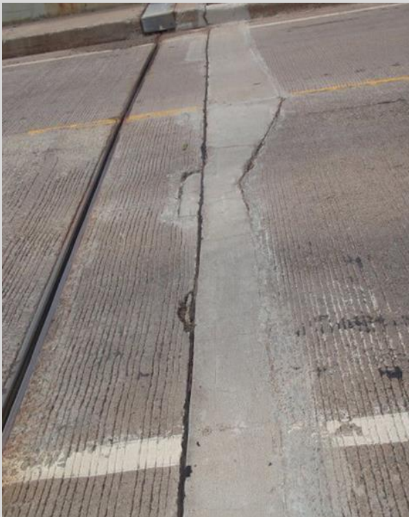
Condition State 2 Concrete patch on a concrete approach panel (along the end block joint)
