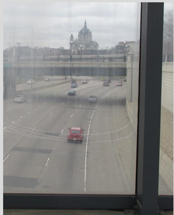
Condition State 3 Cracks in a transparent panel
