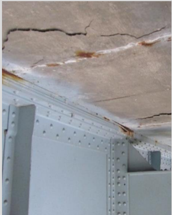
Condition State 4 Delaminated and loose concrete on the underside of a concrete deck (over traffic - safety hazard)
