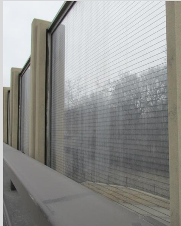
Condition State 1 Transparent Noise Barrier is dirty (no permanent loss of transparency)
