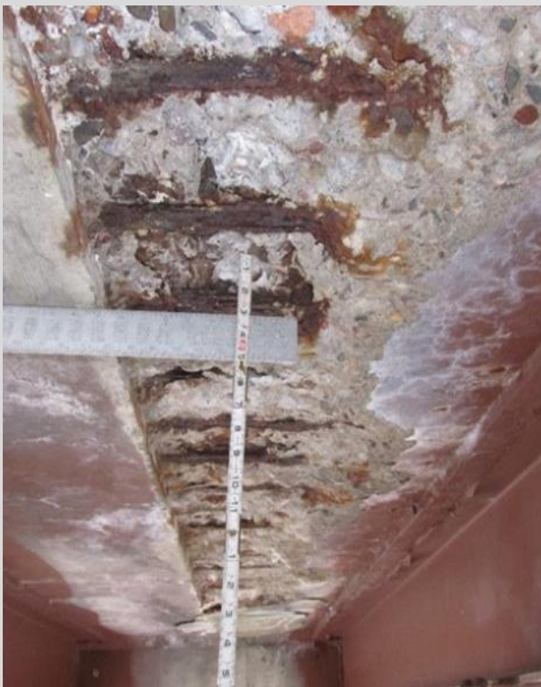
Condition State 4 Severe spalling (more than 3" deep) on the underside of a concrete deck
