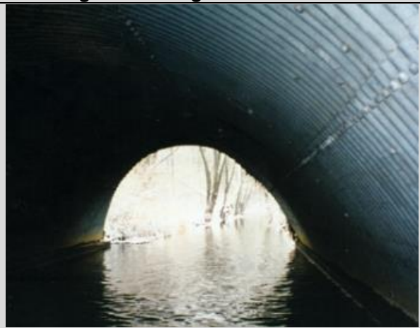
Condition State 3 Asymmetrical barrel distortion
