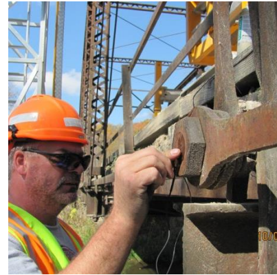
Ultrasonic Examination of a Pinned Truss Connection
