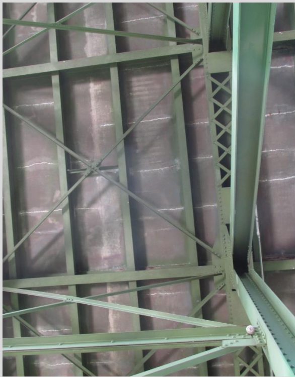
Condition State 2 Transverse crack on the underside of a concrete deck with light leaching (efflorescence)
