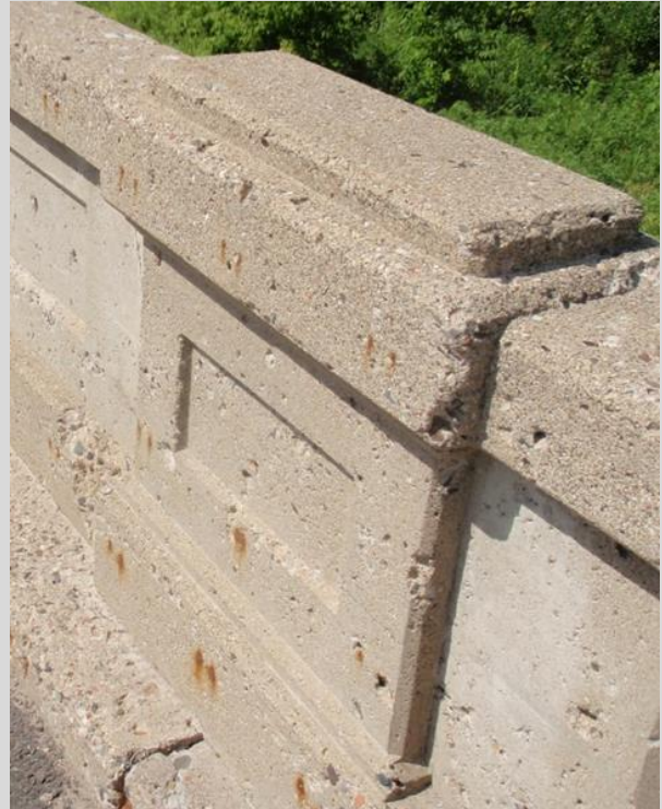
Condition State 2 Scale and pot-outs on a concrete parapet railing
