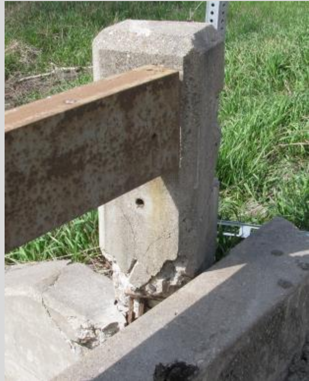
Condition State 4 Severe spall and fracture on a concrete end post
