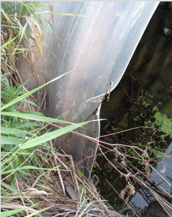
Condition State 3 Torn edge on an aluminum box culvert
