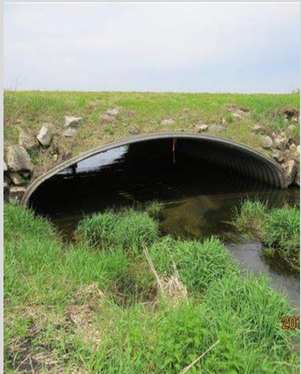
Condition State 1 Aluminum Box Culvert
