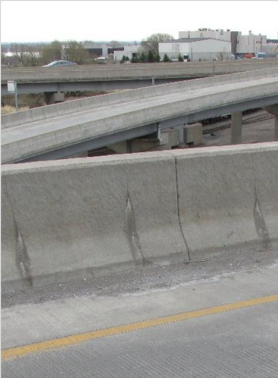
Condition State 2 Vertical cracks with light leaching in a concrete J-barrier
