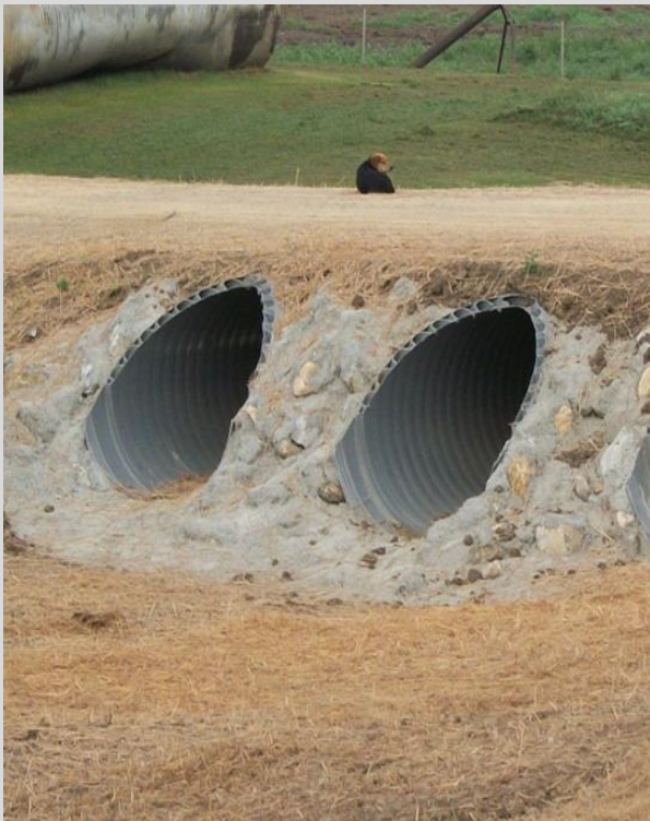
Condition State 1 Plastic pipe culvert (DWPE – Double Wall Polyethylene)
