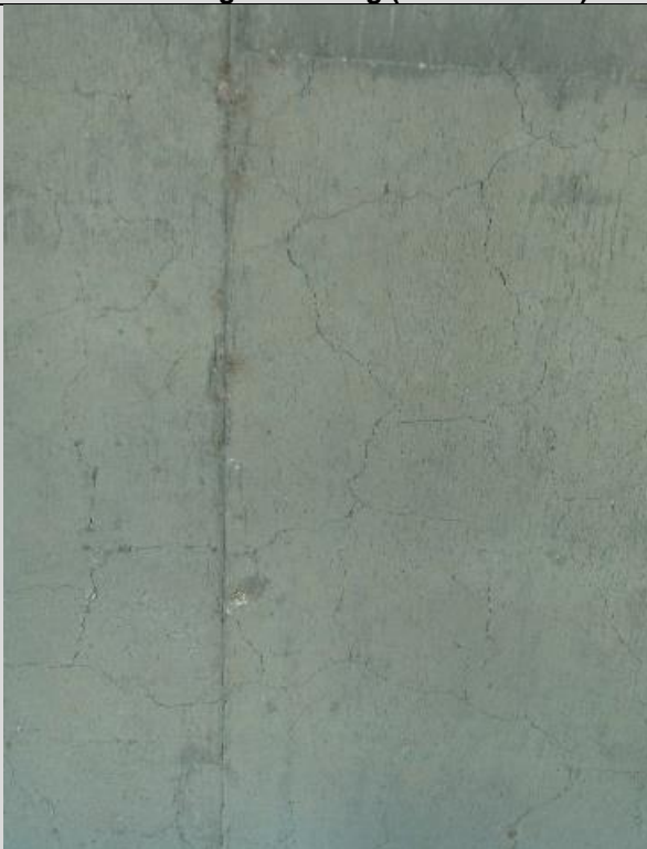
Condition State 2 Map cracking (moderate width) on the underside of a deck with no leaching or water saturation
