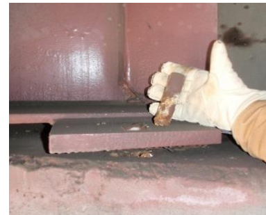
Anchor bolt failure on a fixed bearing
