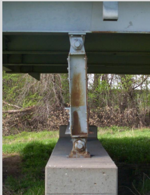
Condition State 2 Paint failure and surface corrosion on a pinned steel column
