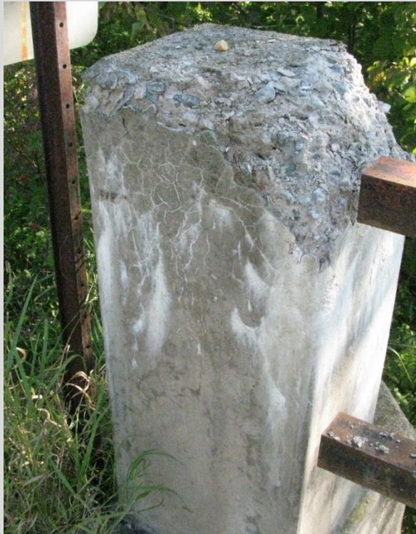
Condition State 3 Scale/spall on a concrete end post
