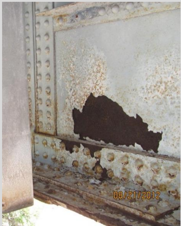
Condition State 4 Paint system failure (exposed steel)
