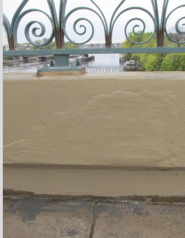
Condition State 2 Repair patch on a concrete parapet of a combination railing
