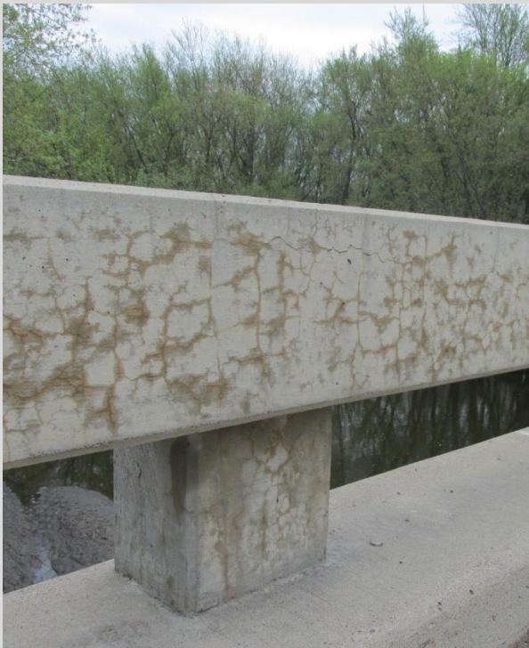
Condition State 2 Map cracking on a concrete post & beam railing
