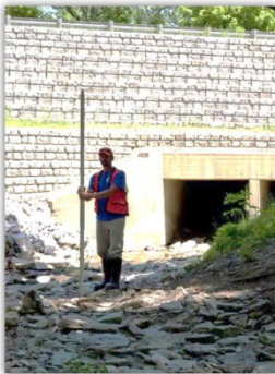
Figure 1-3. Highway failures can occur across a gradient of stream settings, as seen by this ~$250,000 repair at a crossing with a cobble-bed channel draining ~2.6 km 2 , adapted from Hawley et al. (2013).
