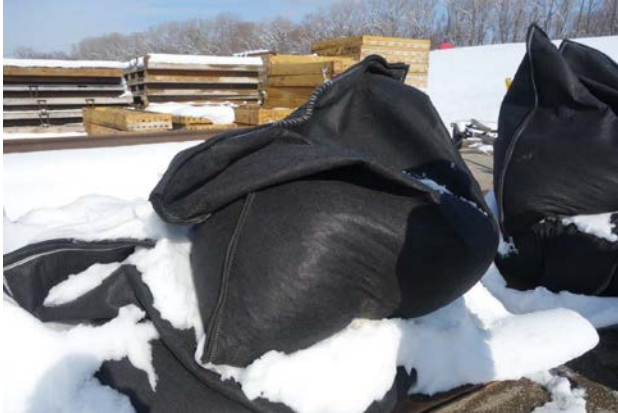
Finished filled Geobag, and installation of Geobag
