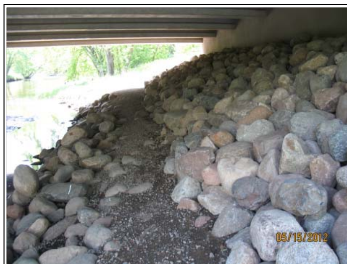
Figure 3.1. Photo of Bridge 48030 left abutment prior to grout installation.
