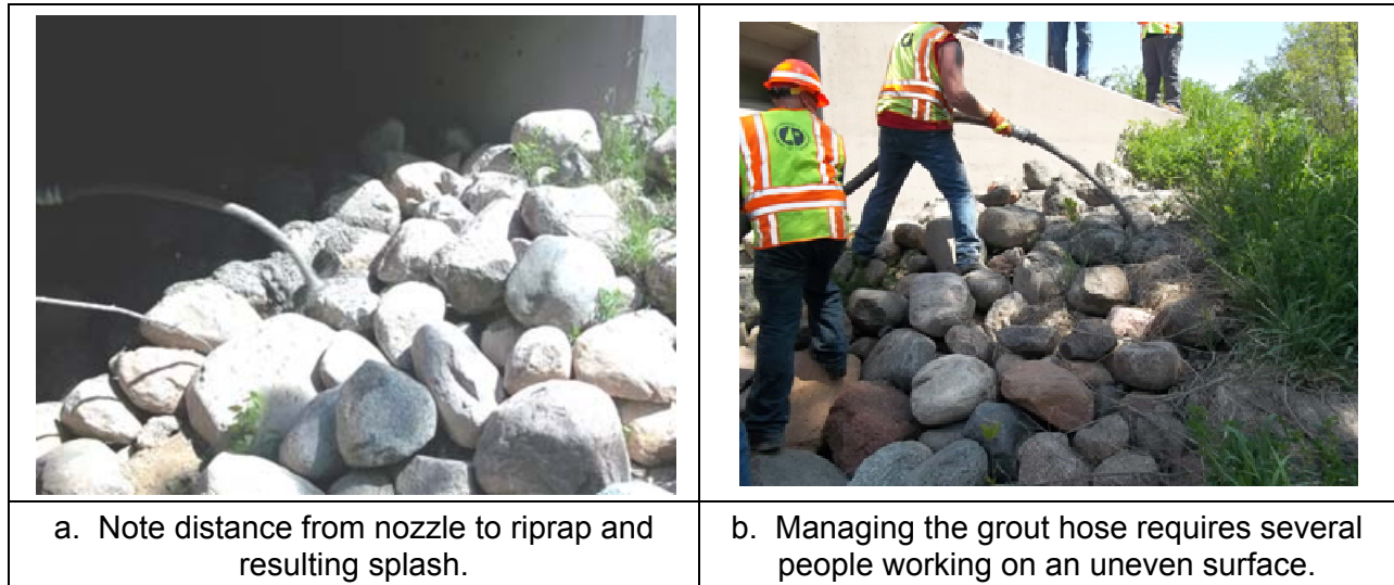
Figure 3.6. Placement of grout at Bridge # 48030.
