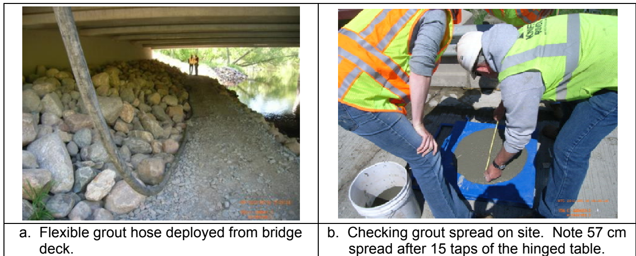
Figure 3.5. Matrix Riprap grout installation setup in Milaca, MN.
