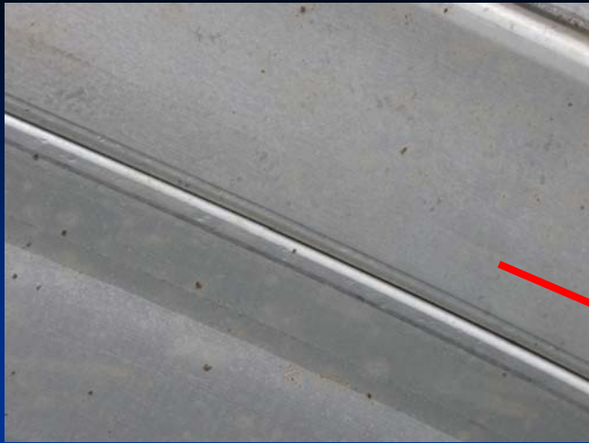
photo 0678 - aluminized type 2- spiral rib corrugation
