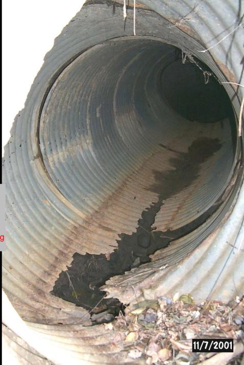
The hole in the pavement may also show up somewhere upstream of the hole in the pipe.
