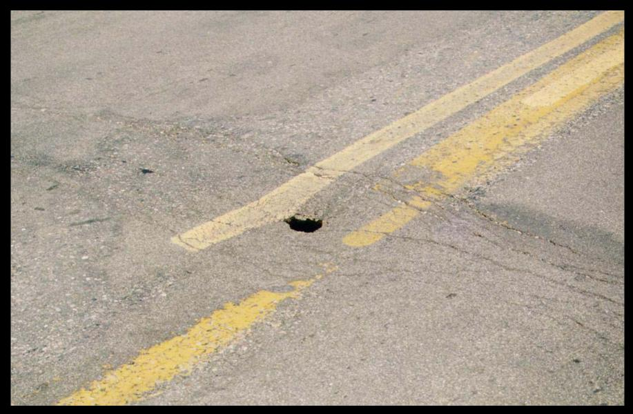
The hole in the pavement may look small. The void below it is the real concern. Holes, joint separations and piping in culverts and storm drain pipes cause voids under road pavement.
