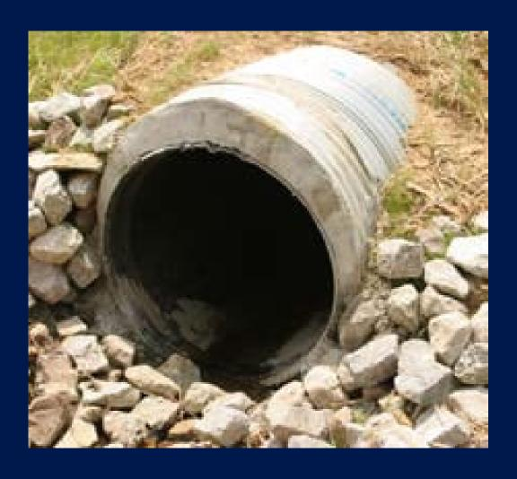
Like Snap-Tite or butt-fused HDPE liner has grout between original pipe and liner.
