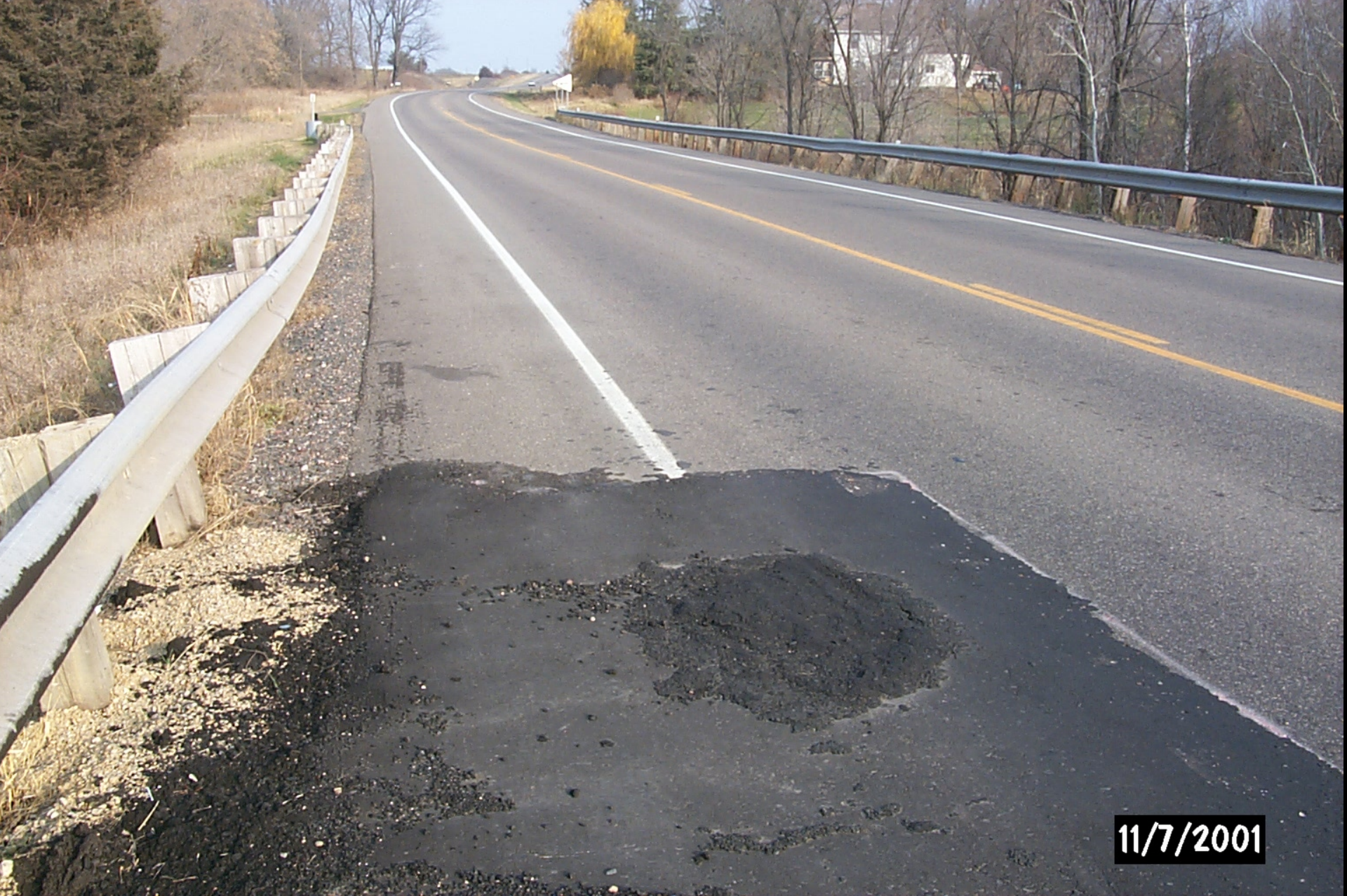
2 successive patches on the bituminous pavement point to a problem below the road's surface.
