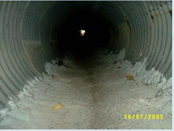
Paved Invert repair, done in 1971, on steel plate culvert still looks good in 2015. Has a channel that keeps most flows away from galvanized steel sides. 2005 Photo from Bergstrand, D1
