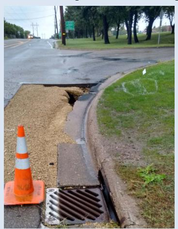
Fill road Voids is a temporary fix. The underlying pipe had holes that caused the void in road. Photo at MnDOT Oakdale Office
