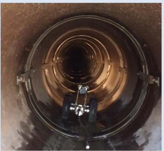
Joint Repair with Internal Bands and heavy-duty pipe ties. Photo from D3 Troy Gratke
