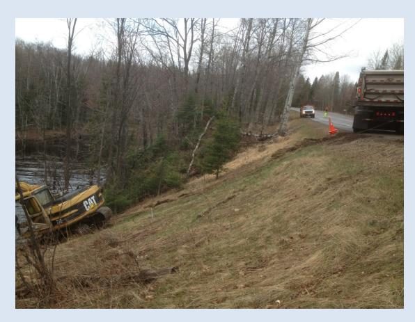
Beaver dam at RP 318.8 RT on TH 23. The box culvert is about 8' and the dam was about 7.5'. Not the best spot for the excavator to work in. We used tree about 14 inch in diameter and 25 feet long to break it loose.
