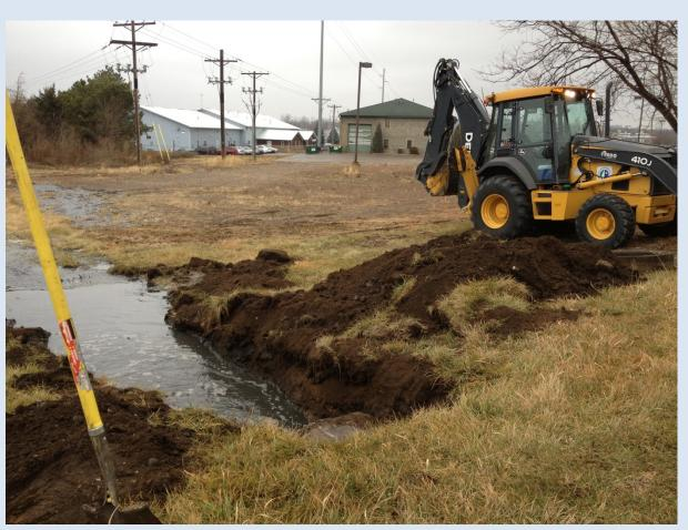
"Cleaning" focuses on the culvert end. Use "Ditch Cleaning" if the largest cost is in the ditch, even if aprons were also cleaned. Photo from D6 Adam Miller
