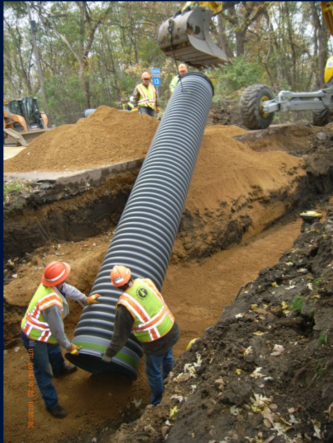
Trench New Pipe
