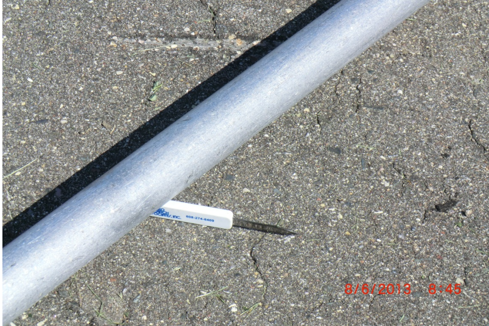
Y49 CTA1 001 (Medium-Severity Rutting)
