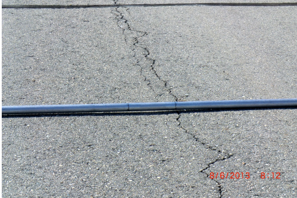
Y49 RY1533 001 (Low-Severity L&T Cracking and Rutting)
