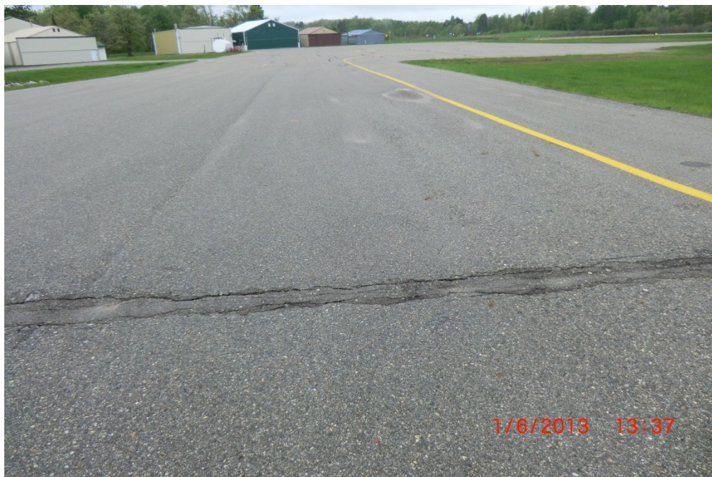
XVG TLC 001 (High-Severity L&T Crack)
