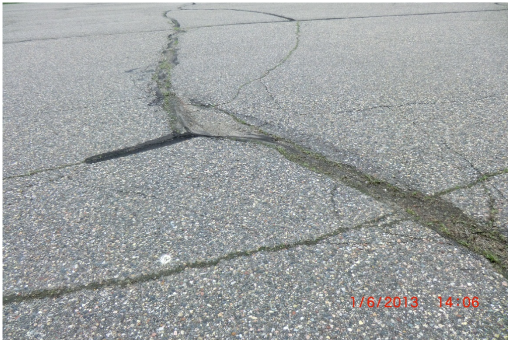
XVG APA 001 (High-Severity L&T Crack)
