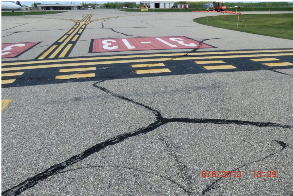
TVF CTA3 002 (Prior to Rehabilitation)
