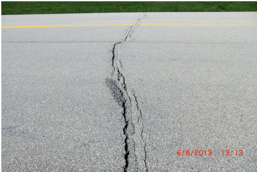
TVF PTB 001 (High-Severity L&T Crack)
