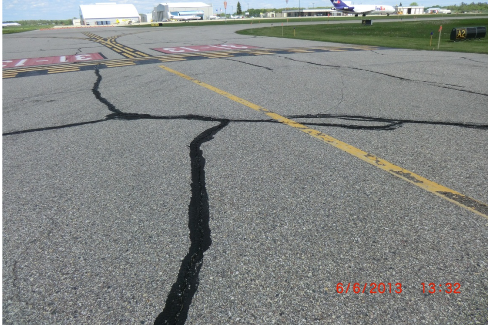
TVF CTA2 002 (Prior to Rehabilitation)
