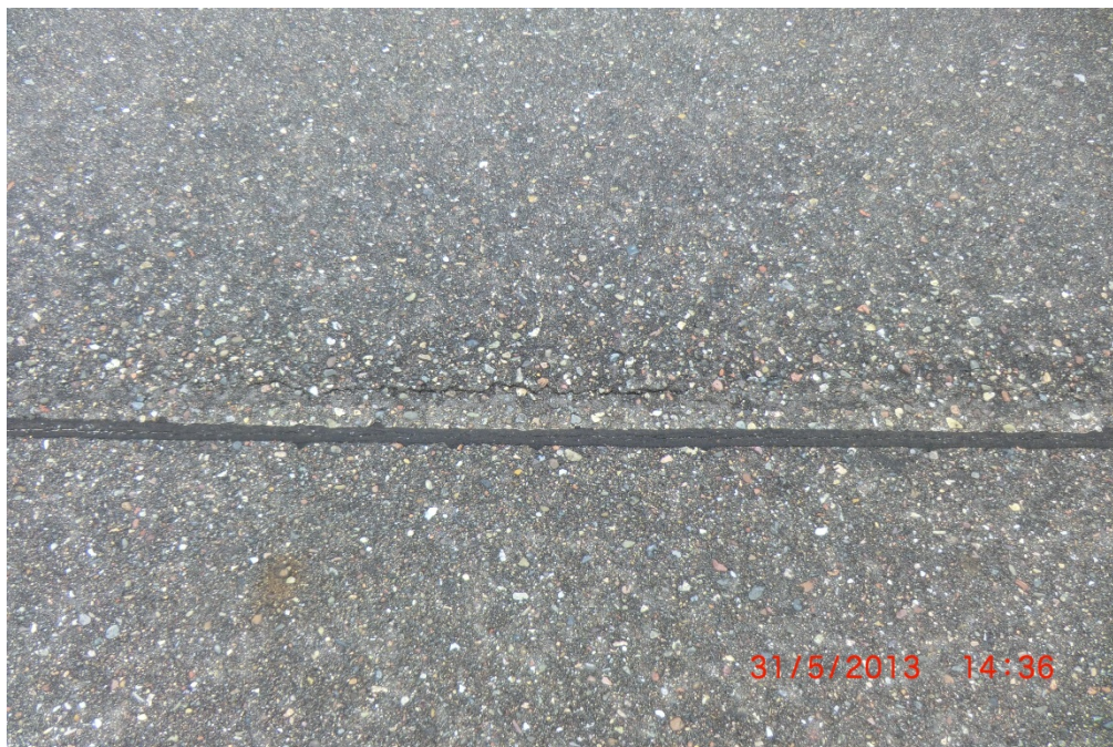
SAZ RY1432 001 (Secondary Crack)
