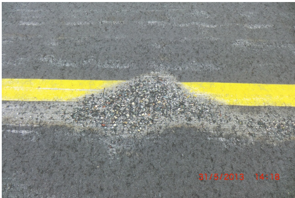
SAZ CTB 002 (Medium-Severity Raveling)
