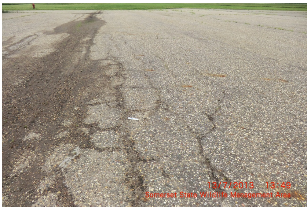
OWA TLA 002 (Medium-Severity Alligator Cracking)
