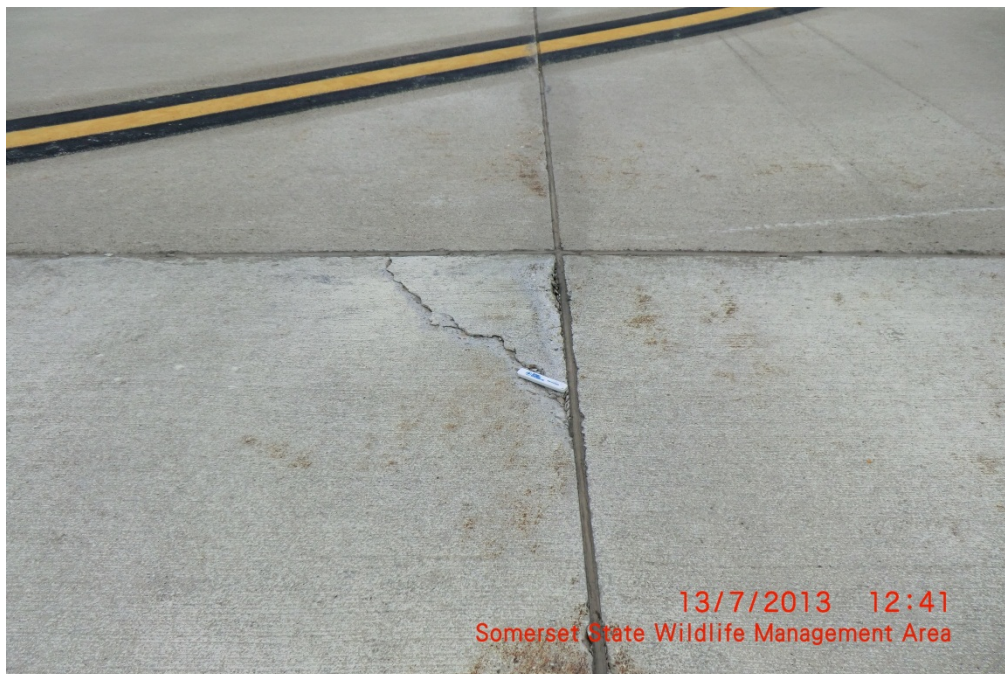
OWA PTA 002 (Medium-Severity Corner Spall)
