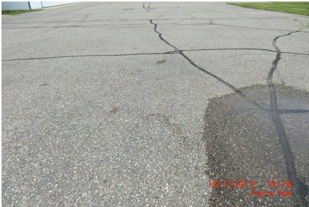
OWA APA 004 (PCI = 14, Medium and High-Severity Raveling Not Visible in Photo)
