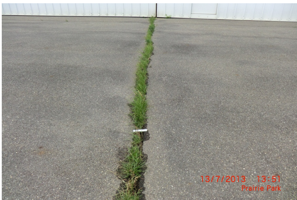
OWA TLA 001 (High-Severity L&T Crack)
