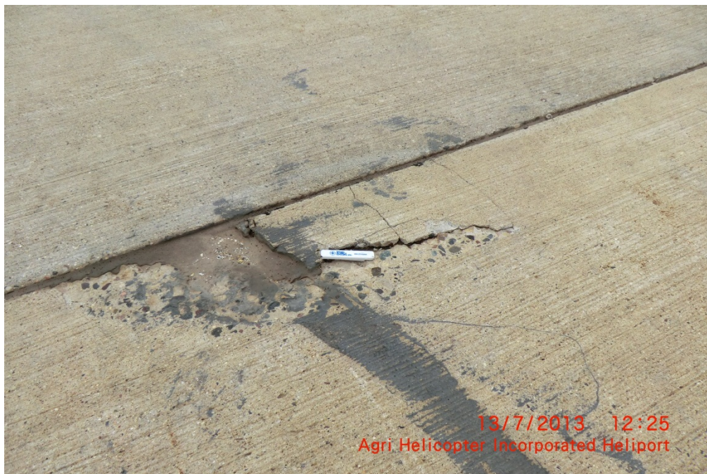
OWA CTA2 002 (High-Severity Joint Spall)
