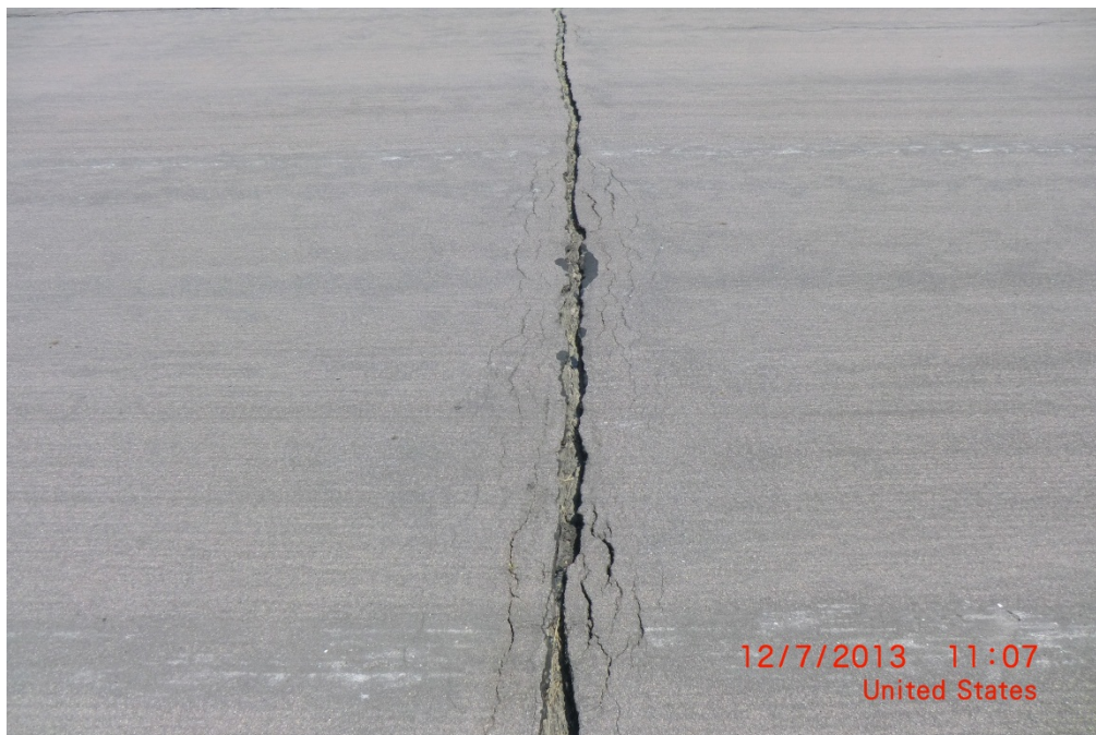
MJQ RY1331 003 (High-Severity L&T Crack)
