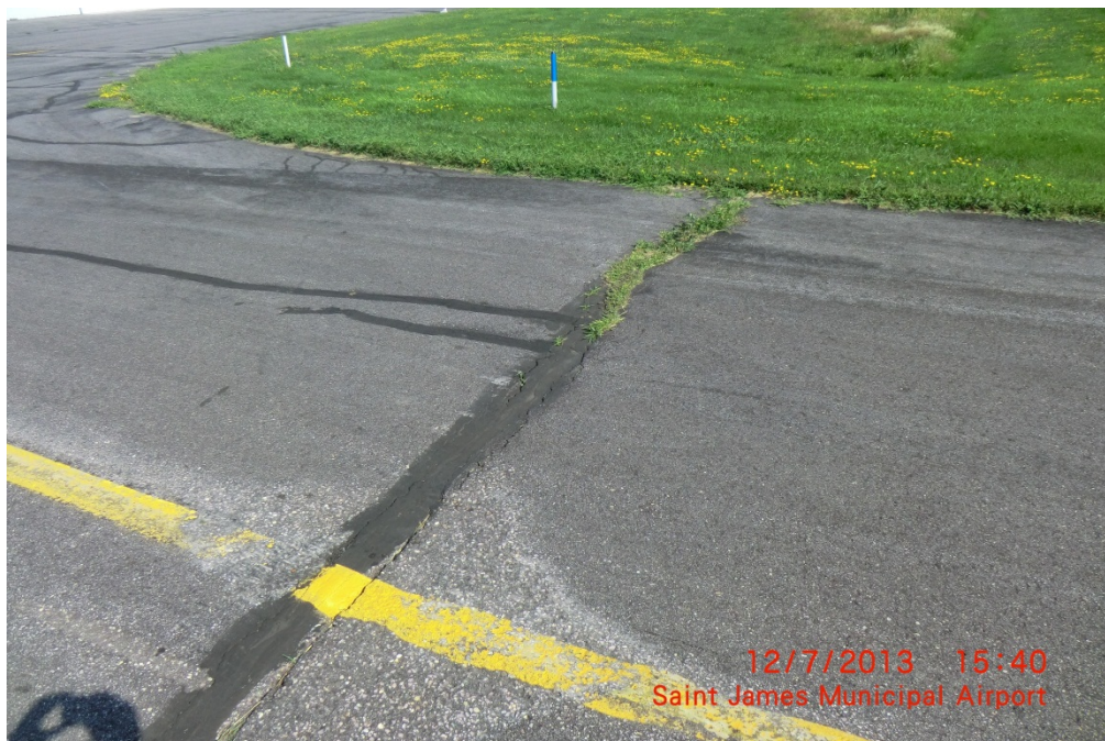
JYG CTB 001 (High-Severity L&T Crack)
