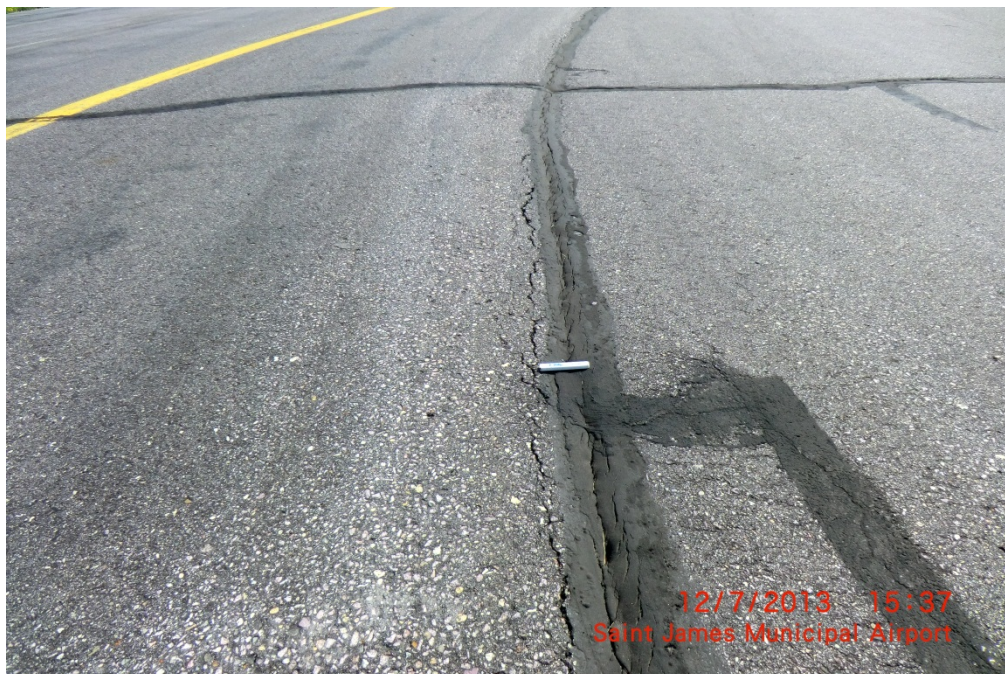
JYG PPTA 003 (Medium-Severity Alligator Cracking)
