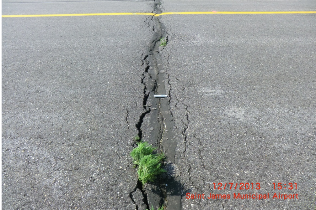
JYG CTA 002 (High-Severity L&T Crack)
