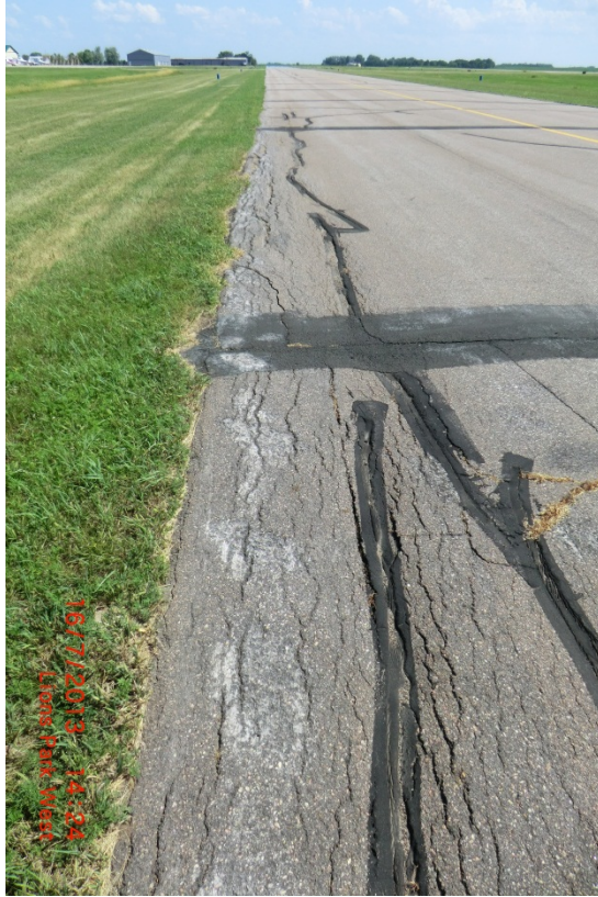
HCD PTA 003 (Alligator Cracking and Swelling)
