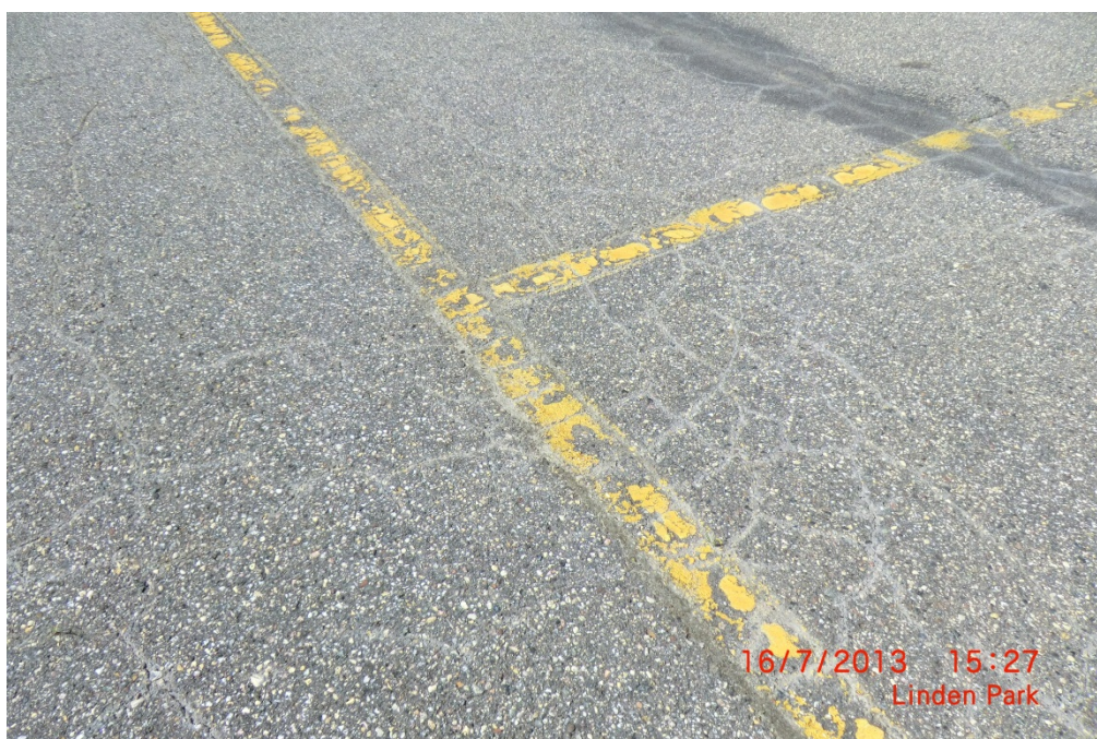
HCD APB 001 (Medium-Severity Alligator Cracking)
