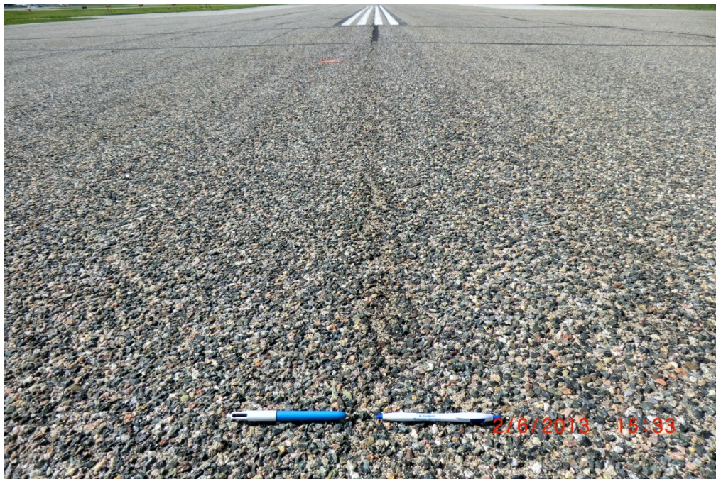
GPZ RY1634 001 (Low-Severity L&T Crack)
