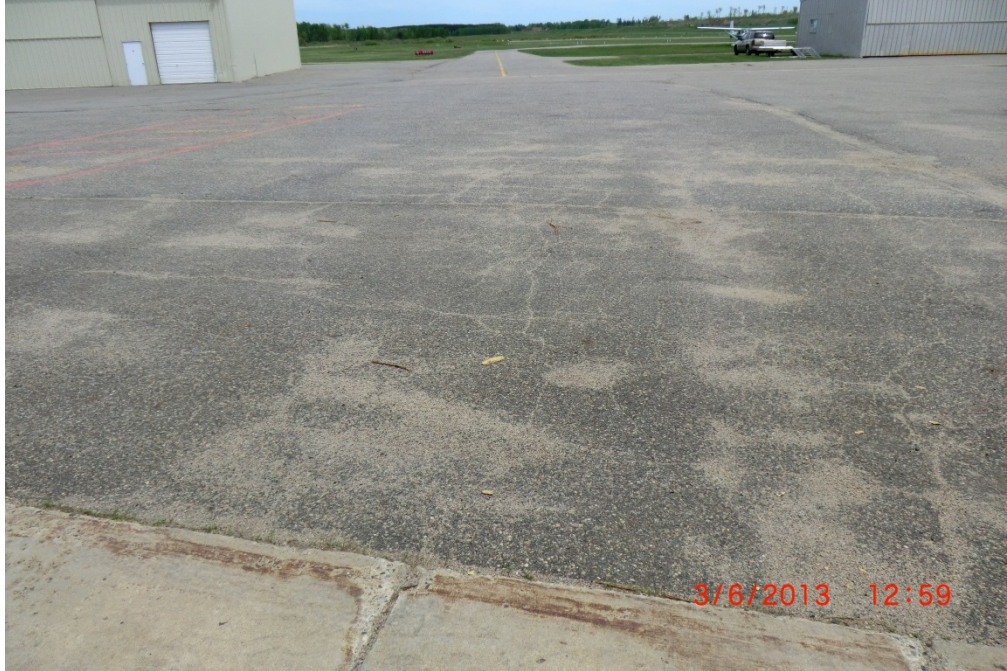
GPZ TLD 001 (Prior to Reconstruction)
