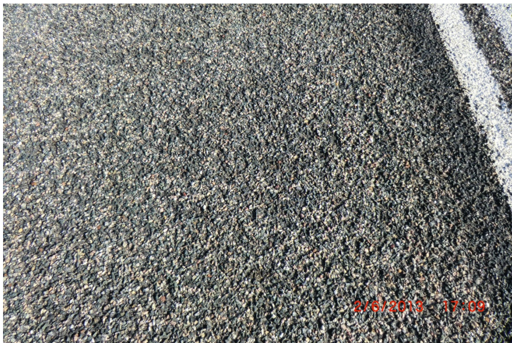
GPZ RY1634 003 (Medium-Severity Raveling)
