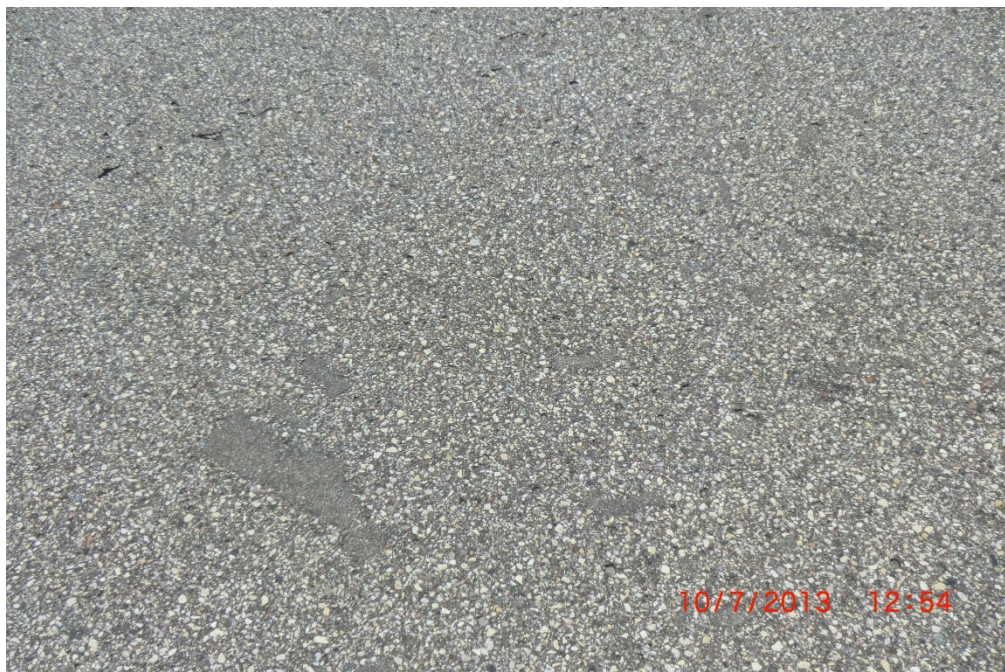
DXX RY1432 001 (Low-Severity Raveling and Weathering)
