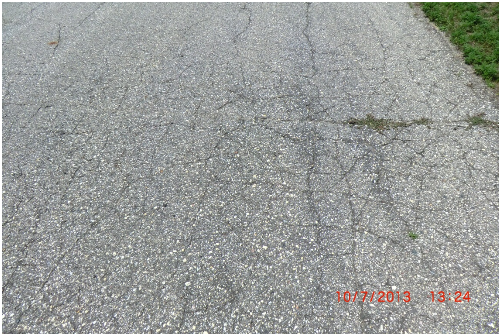
DXX TLA 002 (Medium-Severity Alligator Cracking)
