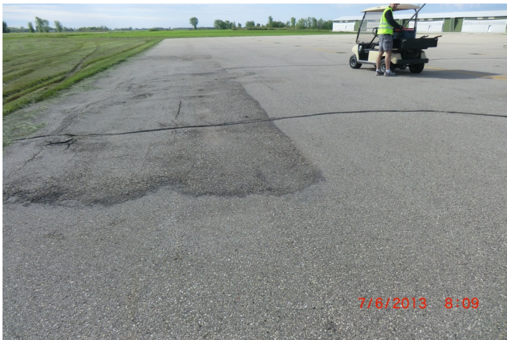
D81 APA 001 (Low-Severity Swelling)
