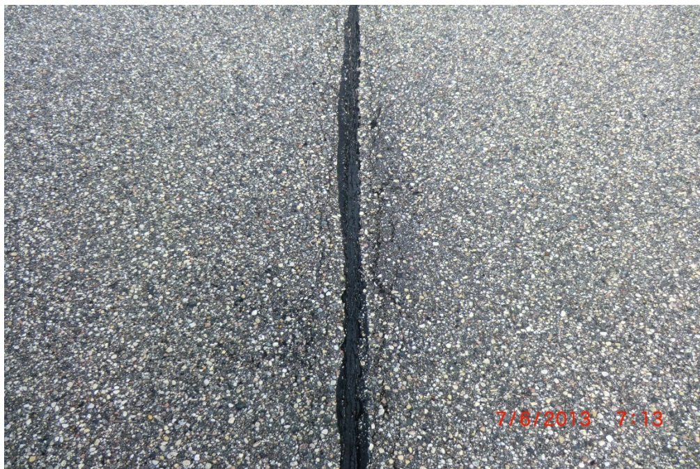
D81 RY1533 001 (Medium-Severity L&T Crack)
