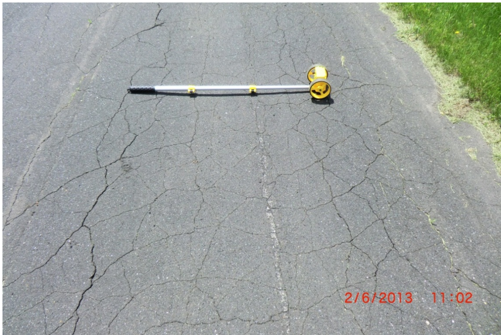
AIT TLC 001 (Medium-Severity Alligator Cracking and Rutting)
