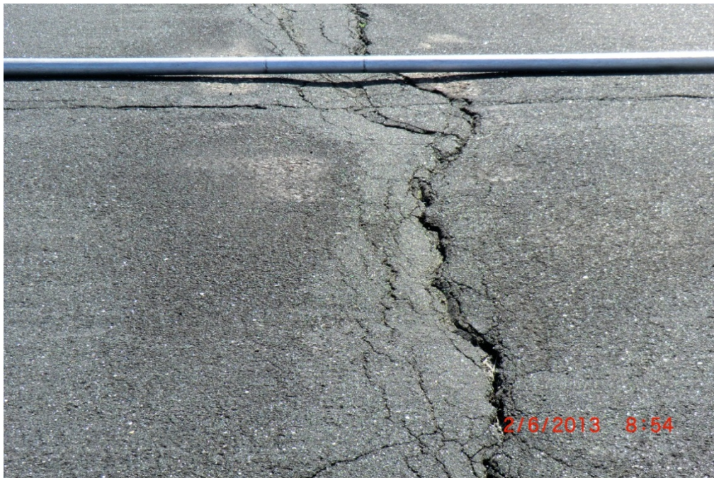
AIT RY1634 001 (Crack with Medium-Severity Depression)
